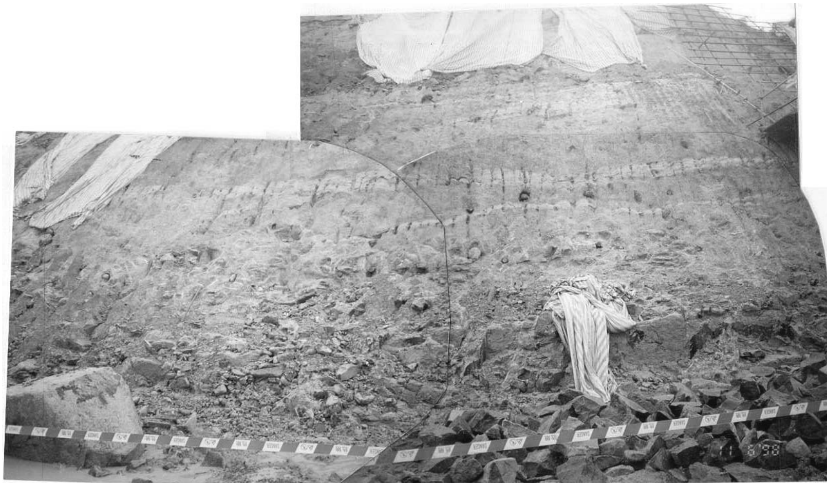
Plate 5 – View of Temporary Cut Slope Surface with Temporary Soil Nails without Nail Head (Photograph taken on 11 June 1998 and Reproduced from GEO Site Record. See Figure 32 for Location.)
