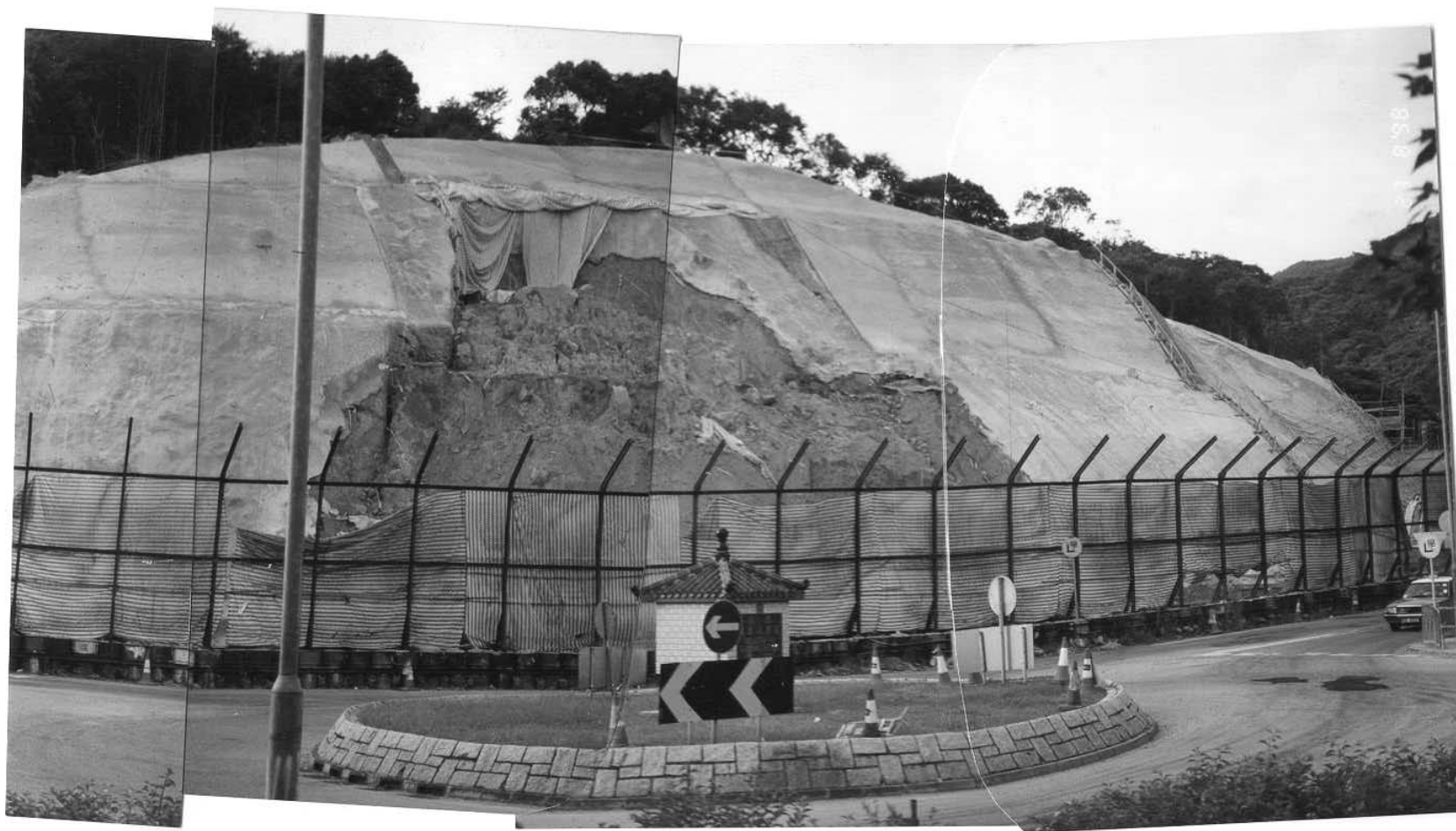
Plate 7 – General View of the Southern Landslide after Shotcreting the Adjacent Areas (Photograph taken on 27 August 1998. See Figure 32 for Location.)
