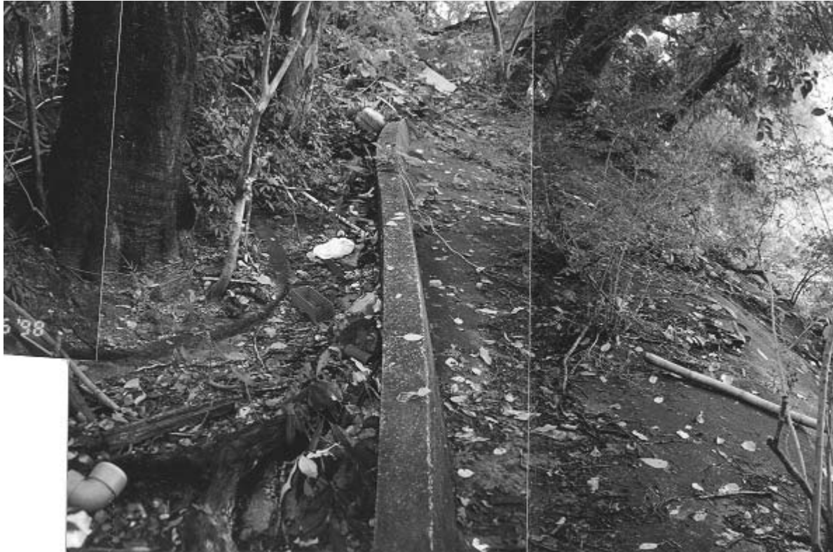
Plate 7 – Blocked Drainage 8 m above Slope No. 11SW-D/C1007 (Photographs taken on 5 June 1998)
