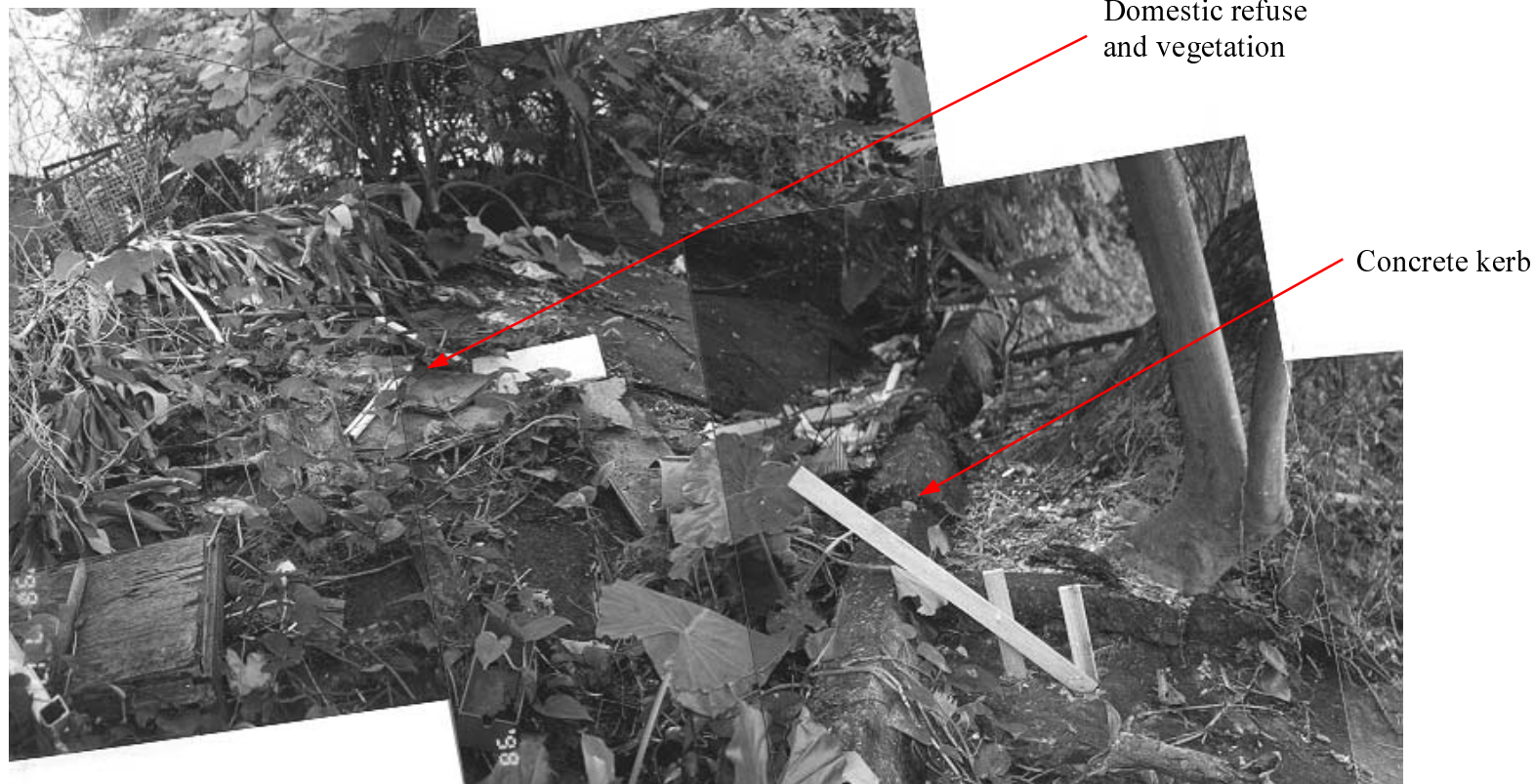
Plate 8 – Dislodged and Partially Broken Section of Concrete Kerb (Photographs taken on 17 July 1998)
