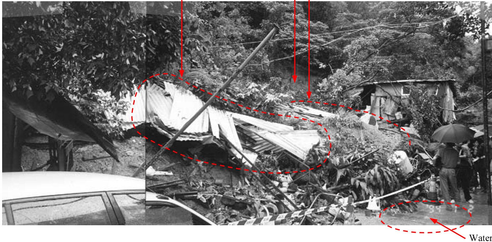
Plate 4a – General View at the Toe of the Scar of Landslide No. 2 showing the Damaged Storage Building. Note the Water at the Toe of the Debris (Photographs taken on 11 June 1998)
