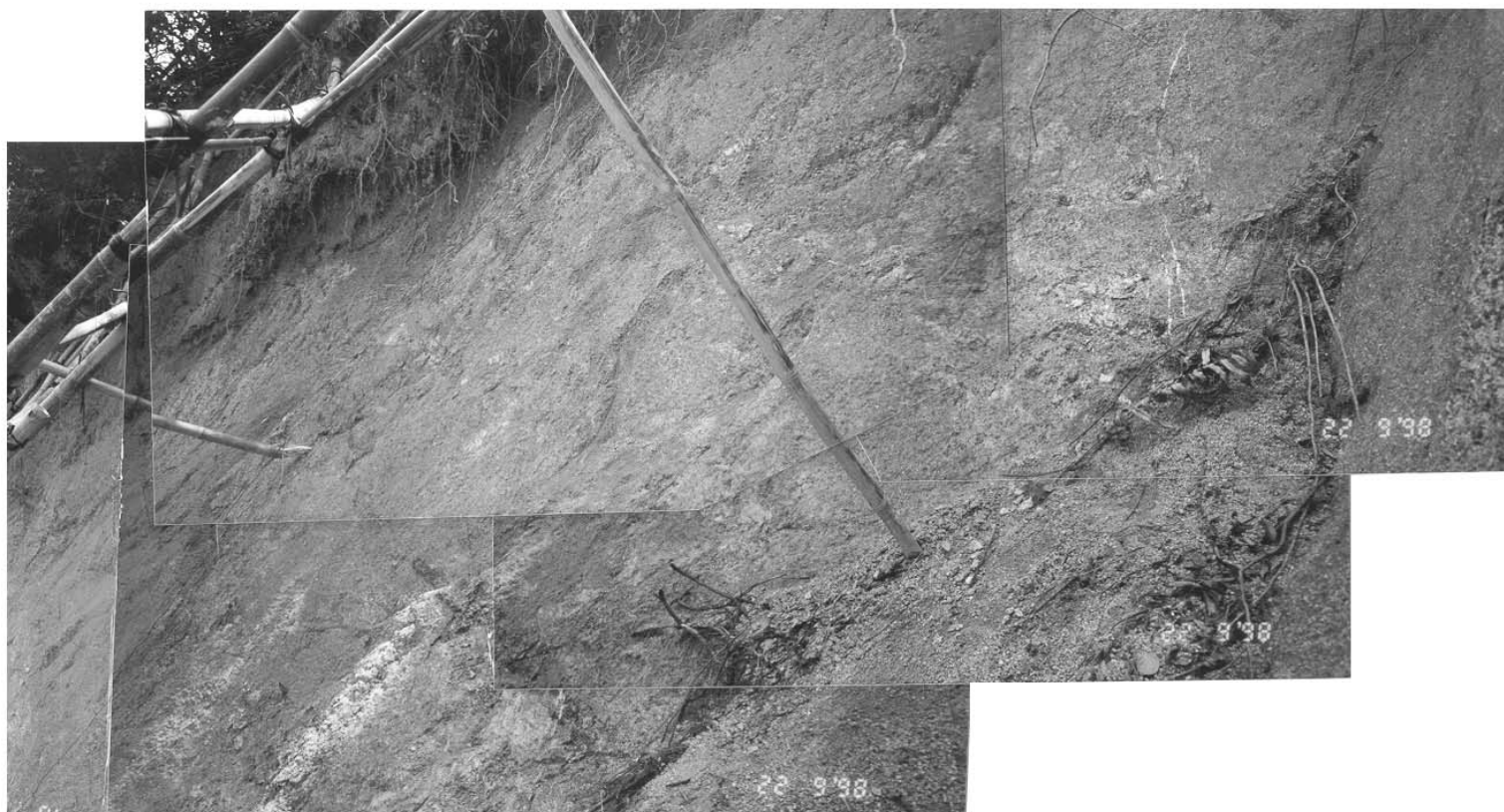
Plate 5 – Close-up View of the Eastern Failure Plane (Photograph taken on 22 Septembe 1998)
