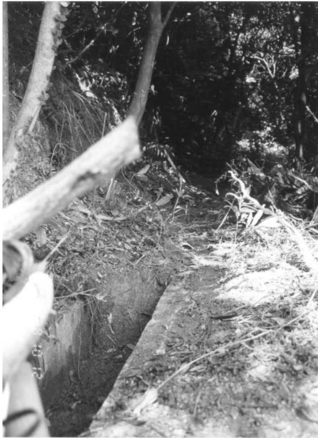
Plate 11 – View of the Drainage Channel above the Western Side of the Landslide (Photographs taken on 12 October 1998)
