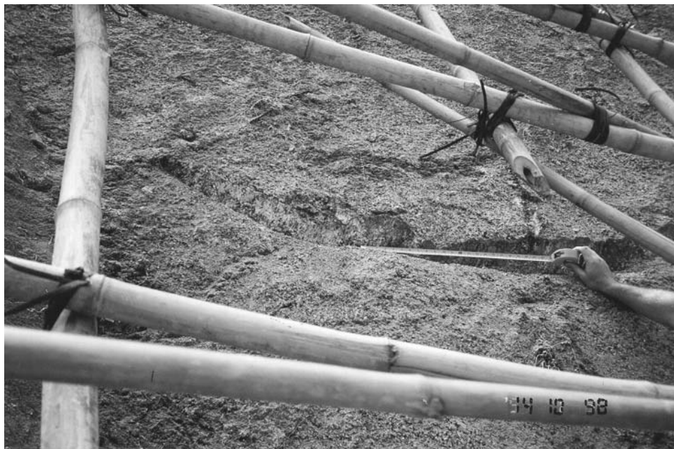
Plate 15 – View of Kaolin Infilled Joint Surfaces Exposed in the Soil Cut Slope (Photographs taken on 14 October 1998)
