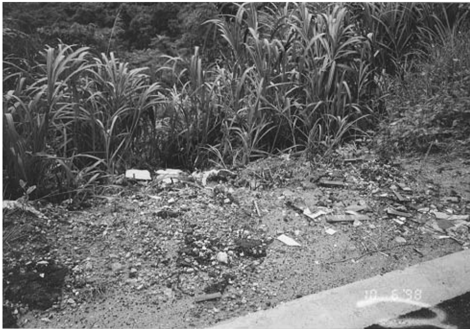
Plate 17 – View East Over Crest of Fill Slope to South of Landslide Scar. Warning Lettering on Pavement (Refer Plate 16) Visible in Lower Right of Frame. Note Appearance of Recent Overland Flow on Soft Verge. (Photograph Taken on 10 June 1998)
