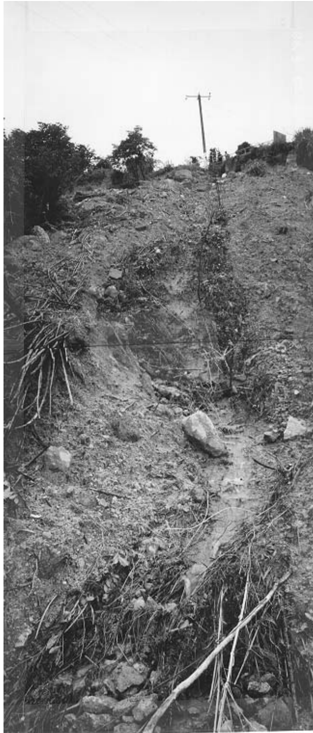
Plate 12 – View West Towards Main Scarp From Within Main Eroded Gully in Deposition Zone. Intact Vegetation Exposed in Eroded Gully. (Photograph Taken on 10 June 1998)
