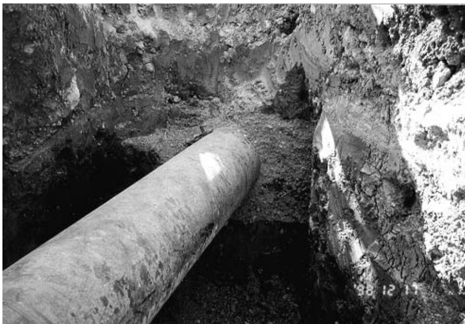
Plate 31 – View South Along 400 mm Diameter Water Main From Within WSD Trench Associated with Main Diversion Works. Note Granular Pipe Bedding Material and Layering in Fill Exposed in Sides of Excavation. (Photograph Taken on 17 December 1998)
