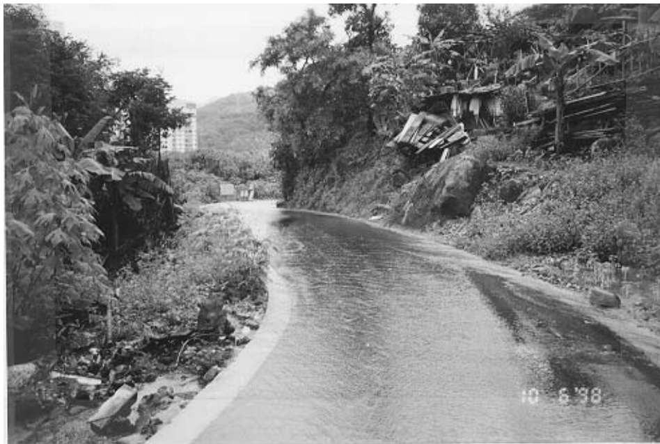
Plate 22 – View South-East Along Au Tau Village Road From Intersection of Road and Stream Course “B”. Note Substantial Overland Flow Along Road. (Photograph Taken on 10 June 1998)
