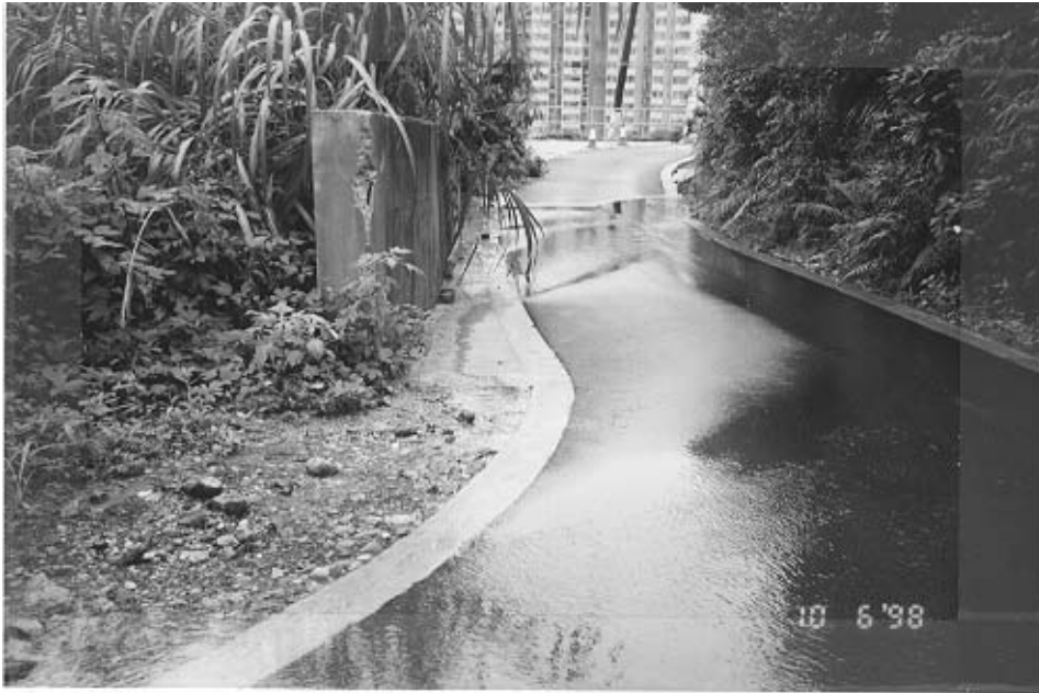
Plate 19 – View East Towards Apron on Outside of Bend in Au Tau Village Road Above Location of Landslide. Note Overland Flow on Road in Foreground and Continued Flow To East. (Photograph Taken on 10 June 1998)
