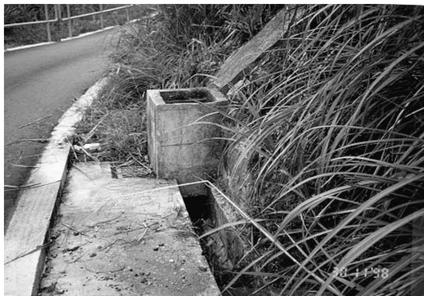
Plate 28 – Catchpit Located Behind Landslide Scar on Opposite Side of Au Tau Village Road. Note 300 mm U-Channel on Road Apron and Stepped U-Channel Providing Discharge to Crest Drainage of Cut Slopes Above Entering Catchpit. (Photograph Taken on 30 November 1998)
