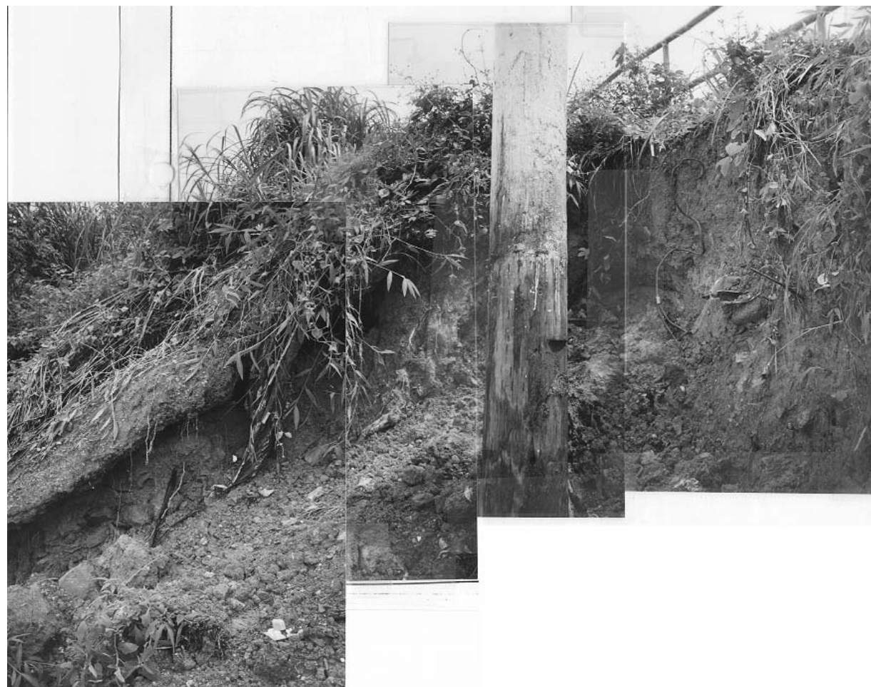
Plate 8 – View of Southern Flank of Landslide Near Main Scarp Indicating Loose Nature of Fill Material and Layering Parallel to Slope Face. (Photograph Taken on 10 June 1998)
