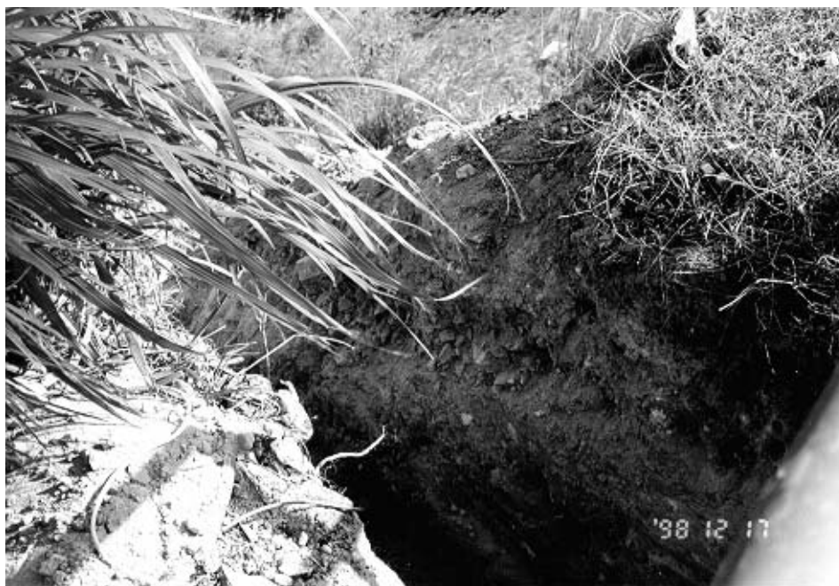
Plate 32 – View North-East Across WSD Trench Associated with Diversion Works for 400 mm Diameter Water Main Exposed in Landslide Scar. Note Variation and Layering in Fill Material Parallel to Slope Face. (Photograph Taken on 17 December 1998)
