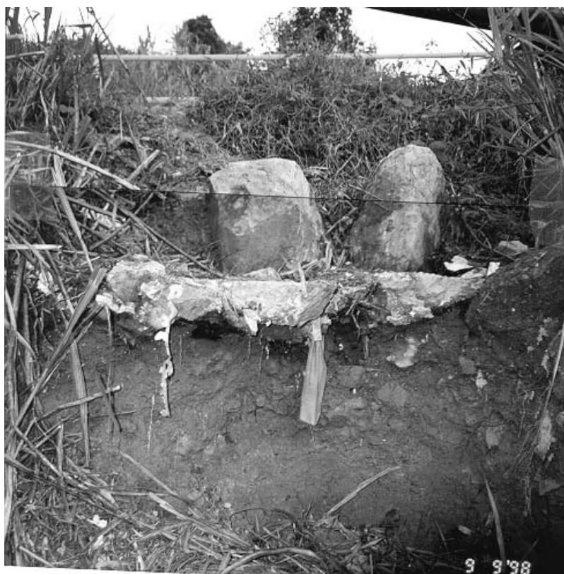
Plate 27 – Close-Up of Main Scarp of Narrow Washout to South of Landslide Scar (Refer Plate 17). Purpose of Concrete Slab is Unknown. Note Undermining Beneath. (Photograph Taken on 9 September 1998)
