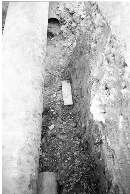
Plate 30 – View North Along Trench Excavated to Expose 400 mm Diameter Water Main Behind Landslide Scar Associated with WSD Diversion Works to Re-Locate Main Away From Slope Crest. Note Section of 150 mm Diameter PVC Pipe Removed During Trench Excavation. (Photograph Taken on 17 December 1998)
