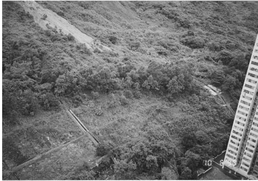
Plate 5 – View West From Yan Lam House, Tsui Lam Estate, Indicating Runout of Debris Relative to Rock Slopes Adjacent to Choi Lam House. (Photograph Taken on 10 June 1998)
