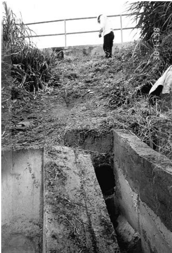
Plate 29 – Outlet to 225 mm Diameter Pipe Draining Catchpit Opposite Landslide Scar (refer Plate 28) Exposed in Slope to North of and Below Concrete Apron. Stepped Channel Extends to North. Concrete Structure Adjacent to Channel Associated with 1992 Water Main Installation by WSD. (Photograph Taken on 30 November 1998)
