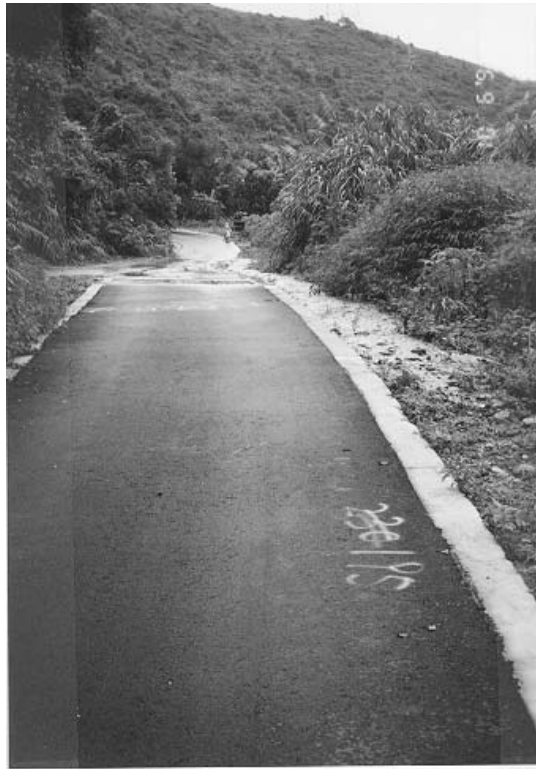
Plate 21 – View North Along Au Tau Village Road to West of Landslide Indicating Overland Flow From Stream Course “B”. Flow Discharges into Valley Below Road on Right of Frame. (Photograph Taken on 10 June 1998)
