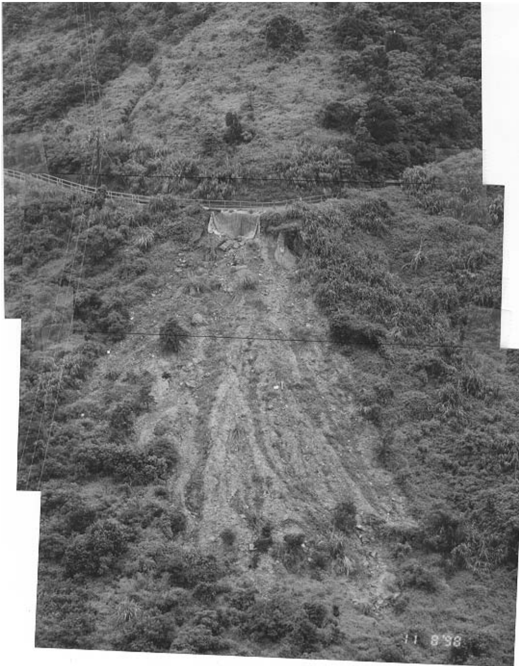
Plate 24 – View West from Choi Lam House Across Landslide Scar. Re-Vegetation in Debris Deposition Zone Provides Indication of Gully Erosion. Locations and Original Toe-Line of Fill Slope No. 11NE-D/F284 Prior to Failure. (Photograph Taken on 11 August 1998)
