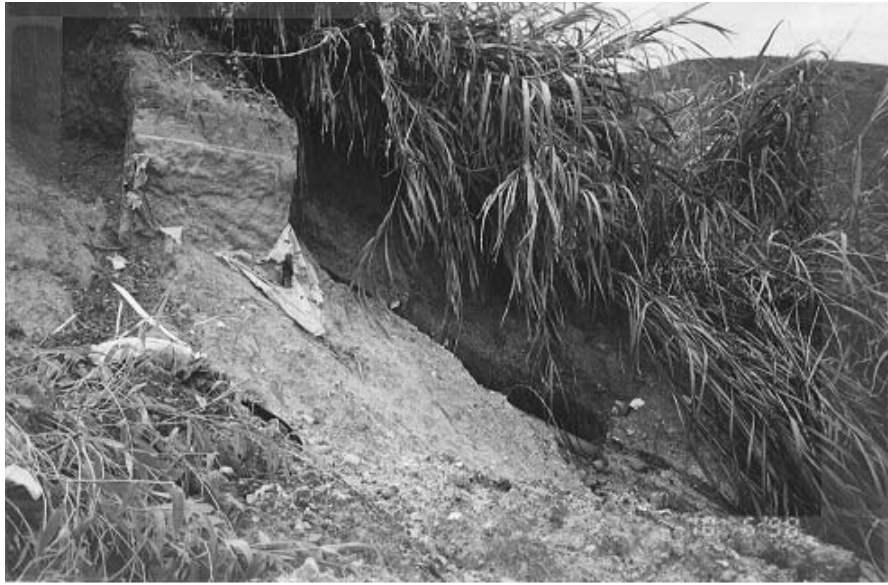
Plate 9 – View of Exposed Pipework on Northern Flank of Landslide Scar. 400 mm Diameter Water Main and 150 mm Diameter PVC Pipes Visible. Broken Section of PVC Pipe Leaking Water Obscured. (Photograph Taken on 10 June 1998)
