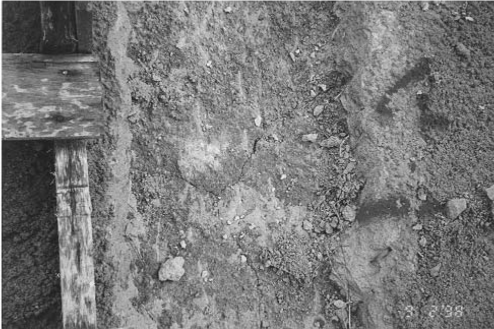
Plate 44 – Strip S1 Showing Cracking in Previous Hard Surfacing 4 m Down Face From Crest (Photograph Taken on 2 September 1998)
