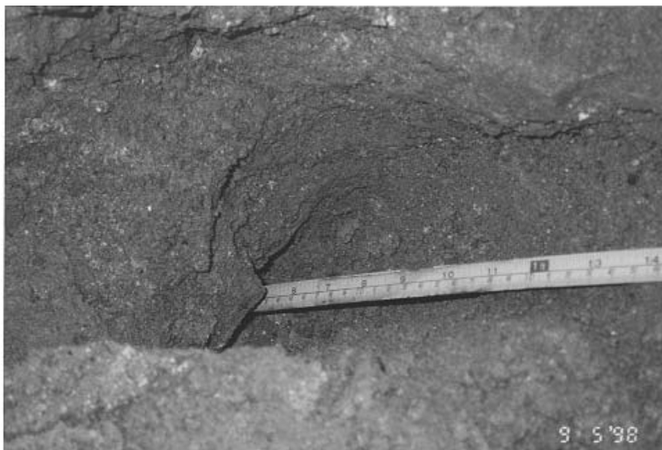
Plate 60 – Strip S3(A) Showing Close-Up of Void. Tape Measure Reads Approximately 300 mm (Photograph Taken on 5 September 1998)
