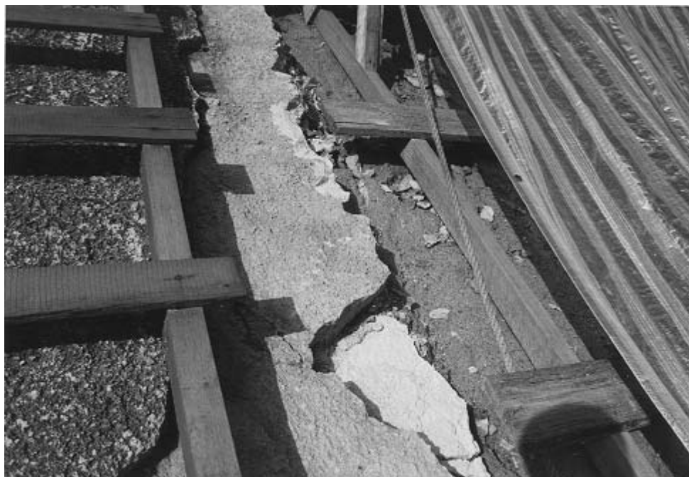
Plate 39 – View of North-western Edge of Shotcrete Strip. Note Previous Application of Hard Surfacing Beneath Shotcrete (Photograph Taken on 5 May 1998)
