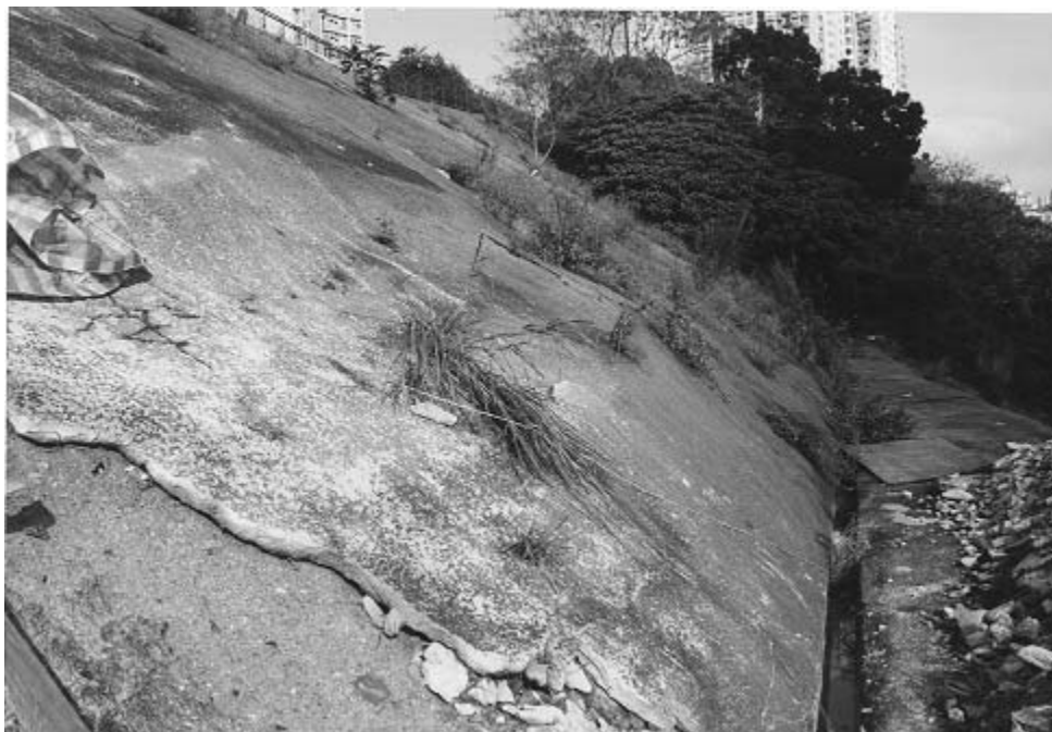
Plate 38 – View South-east Along Upper Berm. Shotcrete Strip Visible in Foreground. Note Break in Slope Angle and Uneven Form of Shotcrete. Note Also Shotcrete Directly Overlying Fill (Photograph Taken on 5 May 1998)
