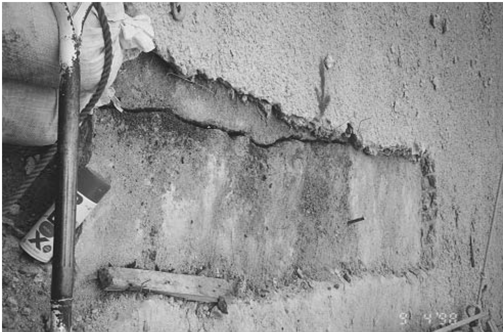
Plate 46 – Strip S1(A) Showing Crack Exposed in Horizontal Strip Extended Across Slope From Strip S1 7.5 m Below Crest (Photograph Taken on 4 September 1998)
