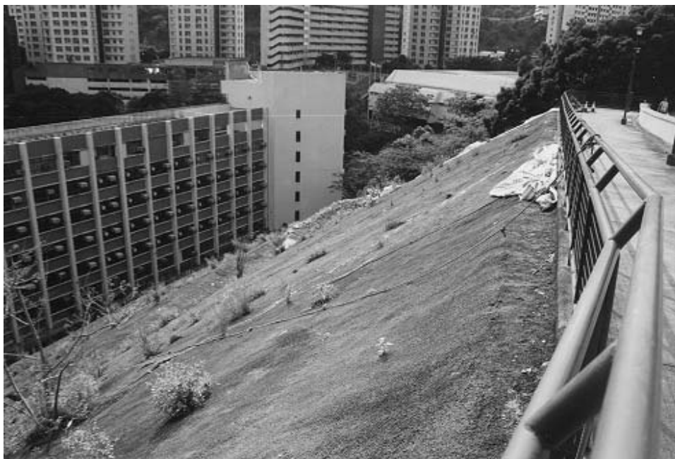
Plate 35 – View North-west Across Upper Batter. Note Cracking on Slope Face and Distortion in Hand Rail (Photograph Taken on 5 May 1998)
