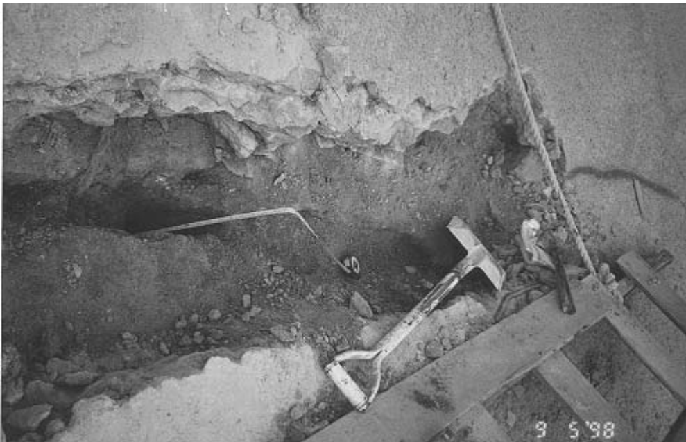
Plate 59 – Strip S3(A) Showing Voiding in Fill Exposed Beneath Hard Surfacing. Crack Width Approximately 100 mm Throughout, Soft Infill Between Voids (Note Multiple Layers of Hard Surfacing) (Photograph Taken on 5 September 1998)
