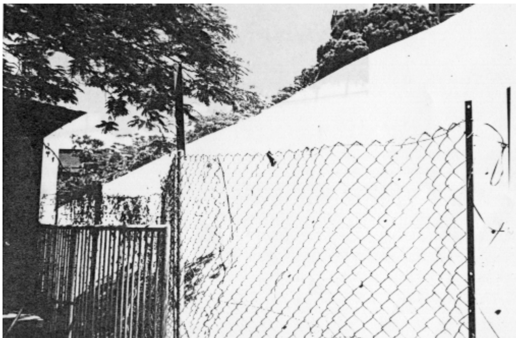
Plate 18 – View North-east From Toe of Slope Indicating Newly Shotcreted Slope. Weepholes Visible in Shotcrete (Photograph Taken on 13 June 1995)
