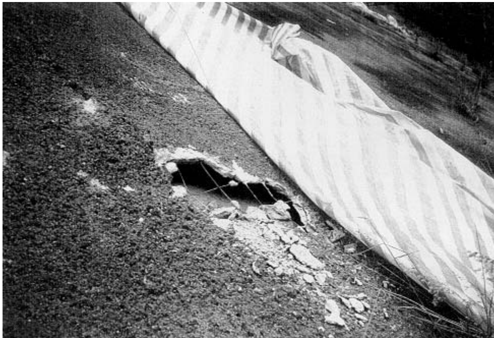
Plate 24 – View of North-western Zone of Bulging in Shotcrete with Inspection Hole Broken in. Note Absence of Free Water (Photograph Taken on 14 April 1998)
