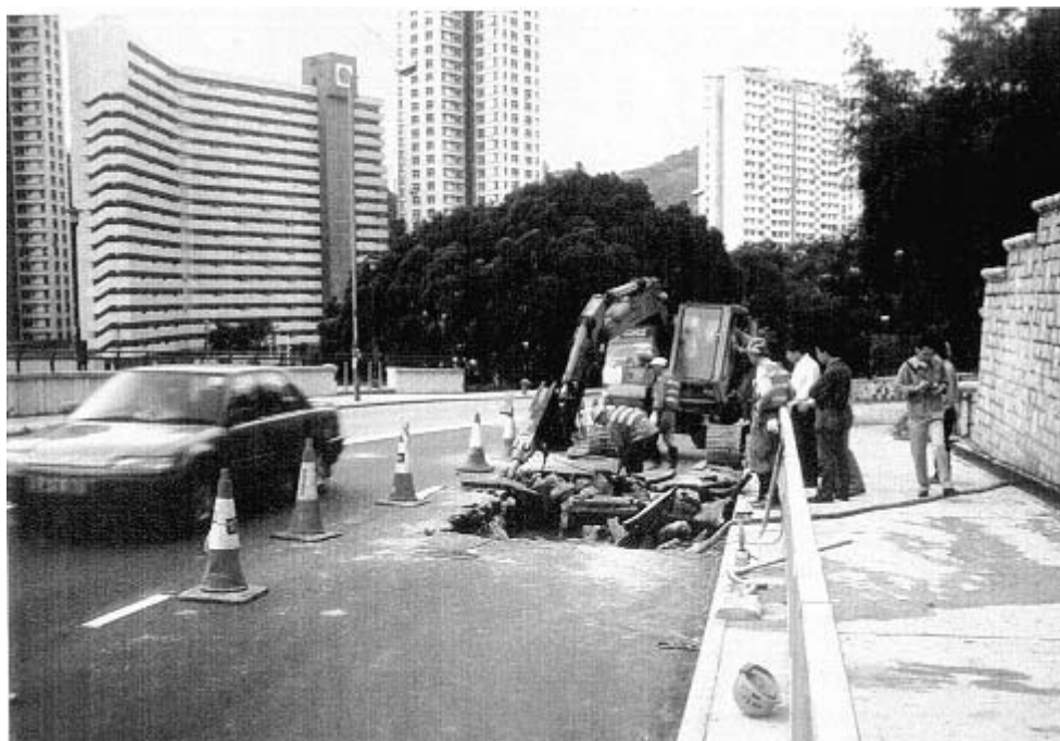
Plate 26 – View North-west Along Northern Side of Hiu Kwong Street. Exploratory Pit Open at Location of Leak in Water Main. Note Free Water Visible in Pit and Blue Hose Pipe for De-Watering (Photograph Taken on 14 April 1998)
