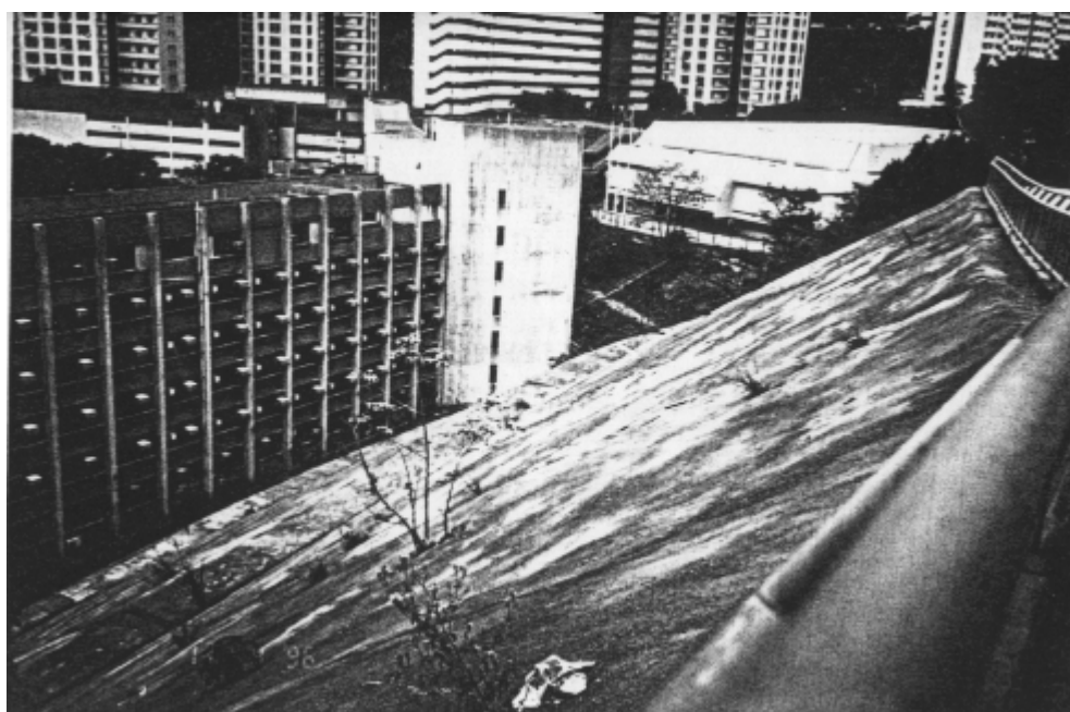
Plate 19 – View North-west Along Crest of Slope. Note Possible Cracking in Foreground. Note Also Distortion in Hand Railing at Crest on Right (Photograph Taken on 11 April 1996)
