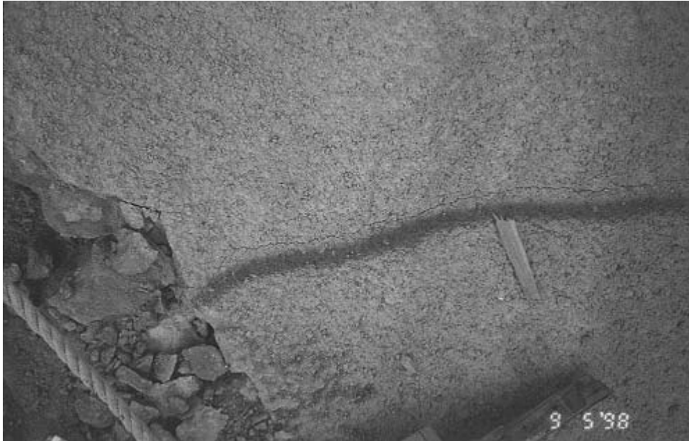
Plate 58 – Strip S3(A) Showing Cracking in 1998 Application of Shotcrete Beyond Extent of Strip (Photograph Taken on 5 September 1998)
