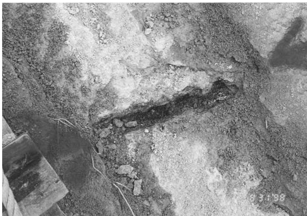
Plate 55 – Strip S3 Showing Cracking Exposed in Previous Hard Surfacing Approximately 4 m Below Crest. Note Darker Organic Fill in Middle Ground (Photograph Taken on 31 August 1998)
