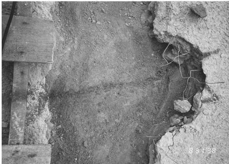
Plate 53 – Strip S2 Showing Fill Exposed Beneath Hard Surfacing, 17 m Above Upper Berm. Note Apparent Extension of Crack into Fill (Area Chased, But No Sign of Cracking in Fill Observed) (Photograph Taken on 31 August 1998)
