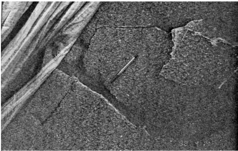
Plate 23 – Cracking in Shotcrete at North-western Zone of Bulging (Photograph Taken on 14 April 1998)
