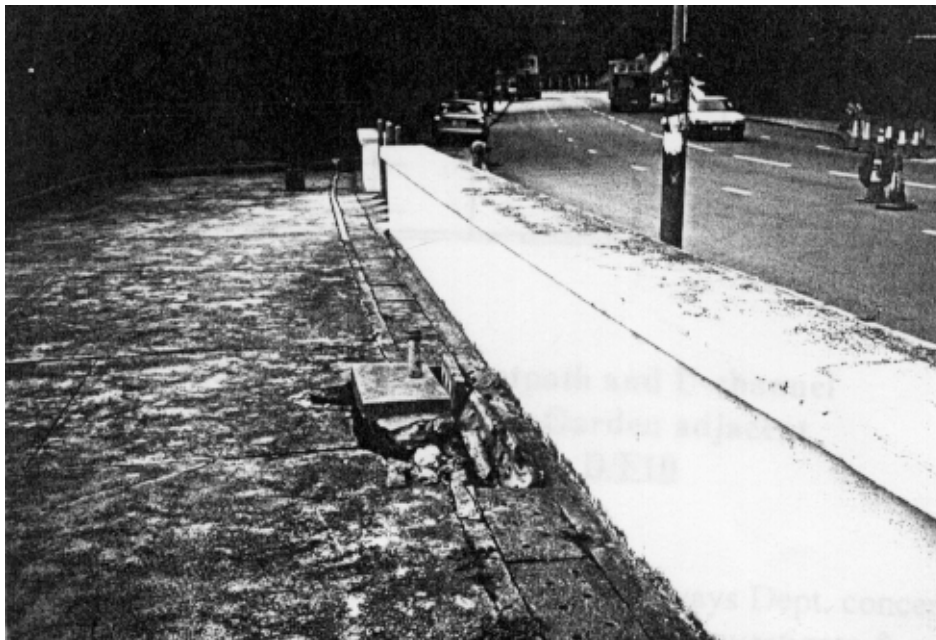
Plate 25 – View North-west Along USD "Open Space" Behind Crest of Slope at North-western End Indicating Concrete Plinth Standing Proud of Surrounding Pavement (Photograph Taken on 14 April 1998)
