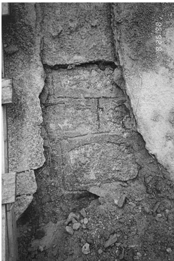
Plate 62 – Strip S4 (Middle Batter) Showing Stone Pitching Exposed Below 1995 Application of Shotcrete at Toe of Batter. Note Differential Movement Between Previous Hard Surfacing and Stone Pitching at Interface (Photograph Taken on 26 August 1998)
