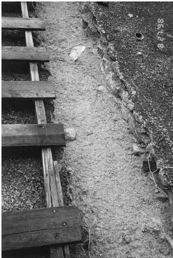
Plate 64 – Strip S4 (Middle Batter) Showing Cracking in Previous Hard Surfacing Approximately 16 m Above Lower Berm. Note Organic Fill and Rootlets (Photograph Taken on 26 August 1998)
