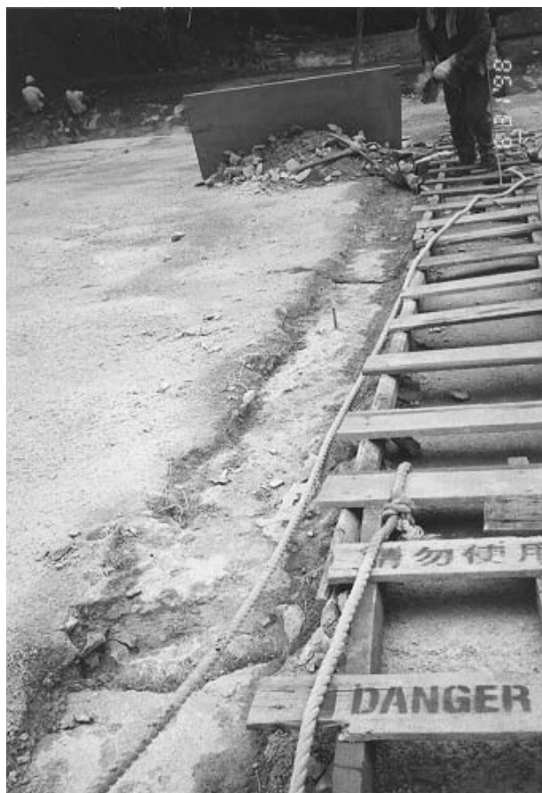
Plate 54 – Strip S3 Showing Cracking Exposed in Previous Hard Surfacing. Crack in Foreground Approximately 0.2 m Below Crest. Crack in Middle Ground Approximately 4 m Below Crest (Photograph Taken on 31 August 1998)
