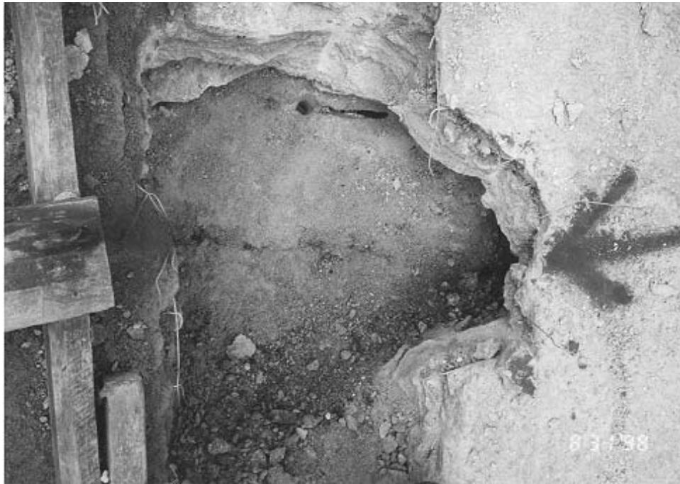
Plate 56 – Strip S3 Showing Fill Exposed Behind Hard Surfacing at Crack Location. Note Staining of Fill Along Line of Crack in Hard Surfacing. Note Void Beneath Surfacing on Right Hand Side. Slot at Top of Exposure is Crack Infill (Photograph Taken on 31 August 1998)
