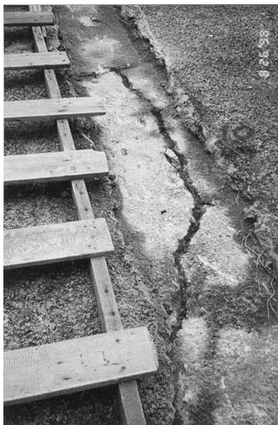
Plate 63 – Strip S4 (Middle Batter) Showing Cracking in Previous Hard Surfacing Below 1995 Application of Shotcrete Approximately 16 m Above Lower Berm. Note Organic Infill and Rootlets (Photograph Taken on 26 August 1998)
