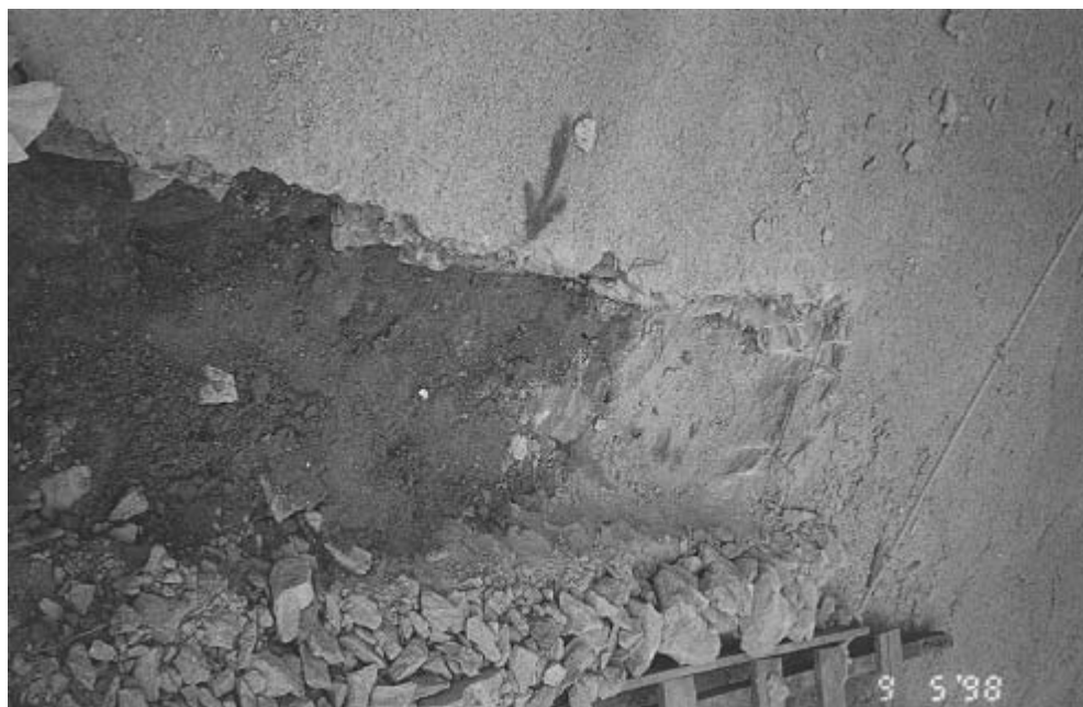
Plate 47 – Strip S1(A) Showing Fill Exposed Below Hard Surfacing (Photograph Taken on 5 September 1998)
