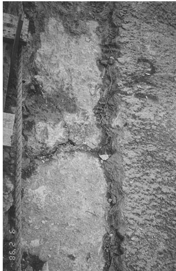
Plate 43 – Strip S1 Showing Cracking in Previous Hard Surfacing 2 m Down Face From Crest (Photograph Taken on 2 September 1998)
