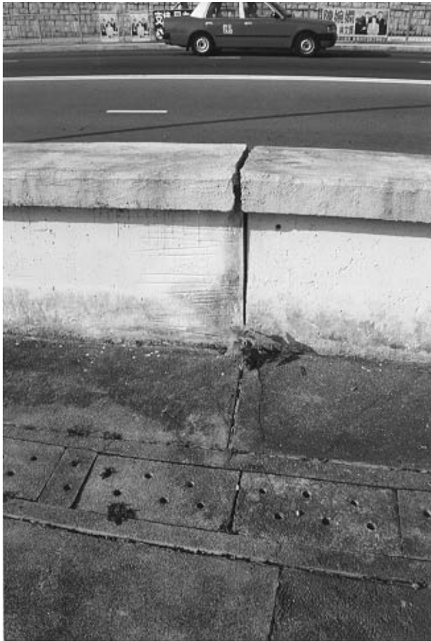
Plate 36 – Cracking at Construction Joint in Parapet Wall (Photograph Taken on 5 May 1998)
