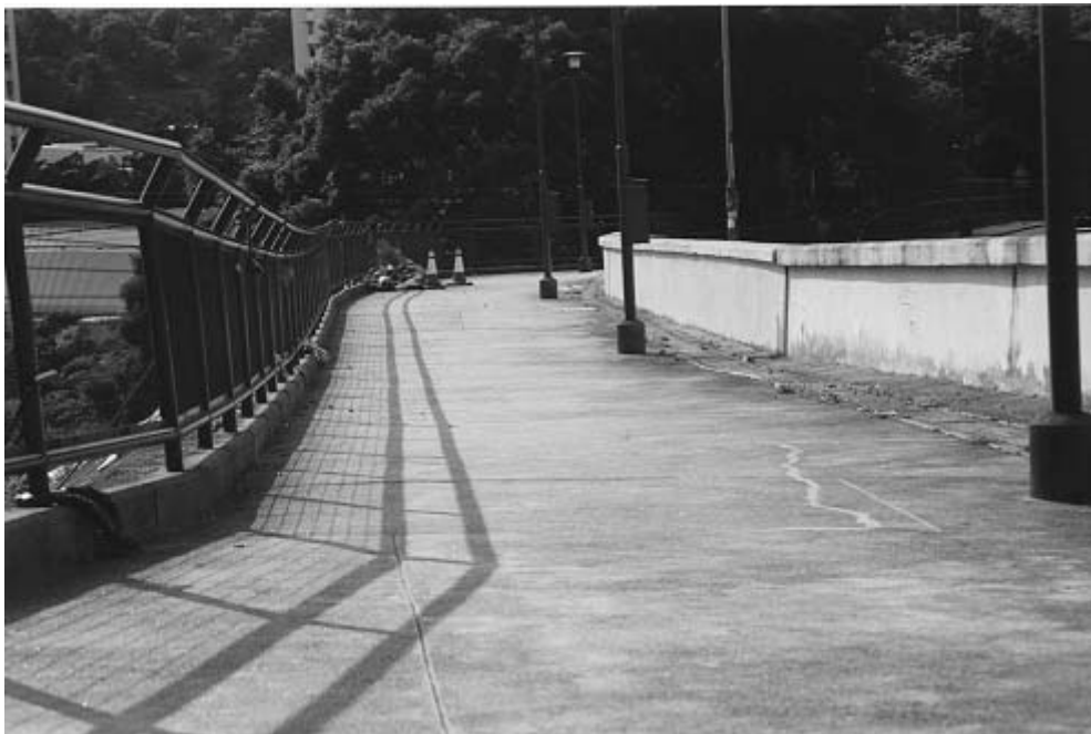
Plate 33 – View North-west Along USD "Open Space" Behind Crest. Note Distortion in Hand Railing and Concrete Parapet Wall. Note Also Repaired Cracking in Pavement in Right Foreground (Photograph Taken on 5 May 1998)
