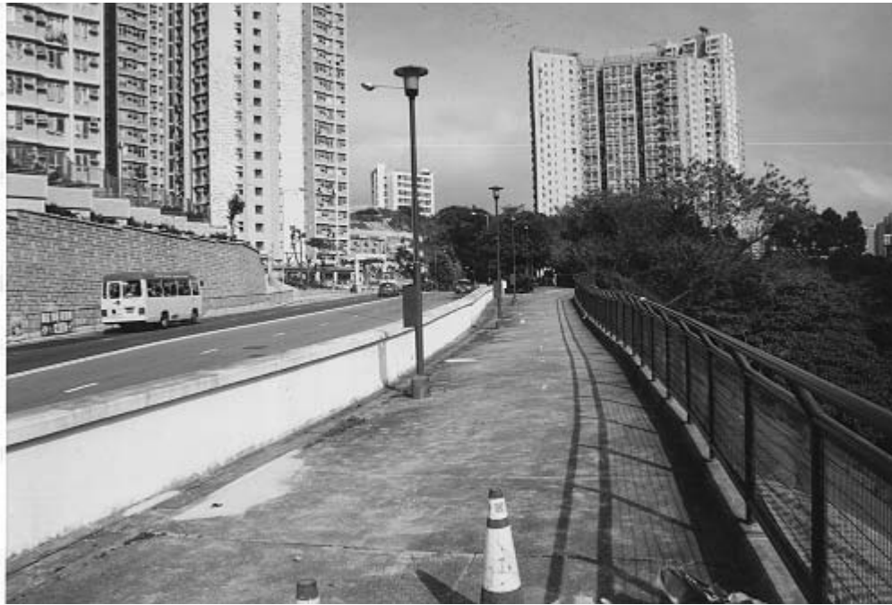
Plate 32 – View South-east Along Open Space Behind Crest. Note Distortion in Hand Railing and Concrete Parapet Wall. Repaired Location of Concrete Plinth Visible in Left Foreground. Repaired Road Pavement at Location of Leaking Main Visible Behind PLB in Left Middle Ground (Photograph Taken on 5 May 1998)
