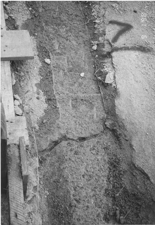
Plate 42 – Strip S1 Showing Cracking in Previous Hard Surfacing 7.5 m Down Face From Crest (Photograph Taken on 1 September 1998)
