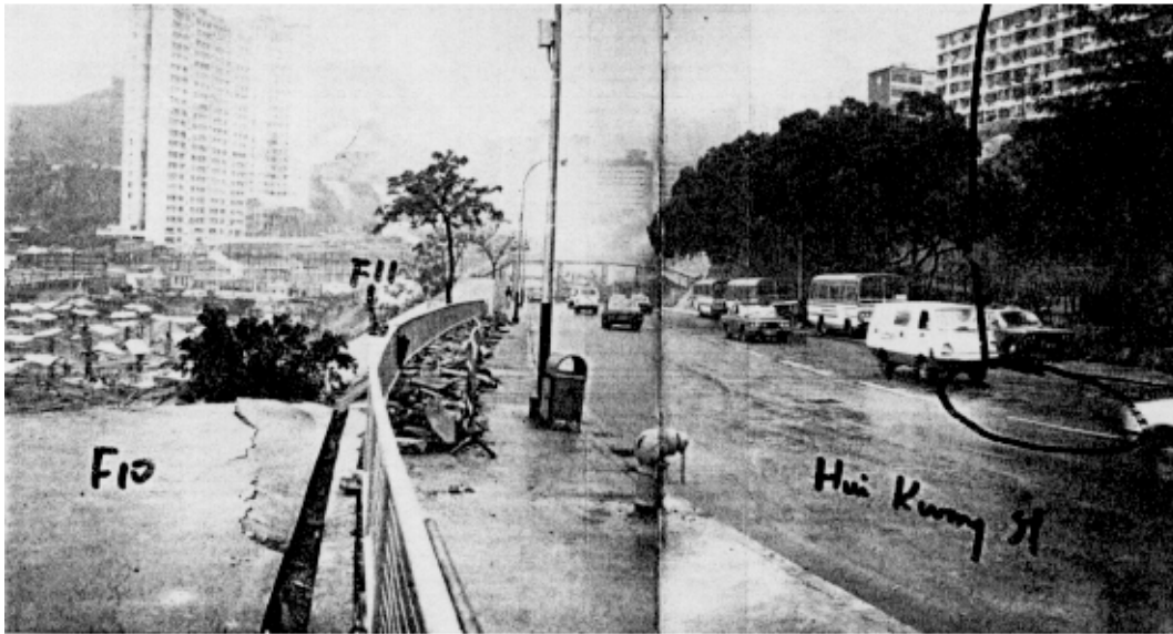
Plate 6 – View North-west Along Crest of Slope No. 11NE-D/F10 Following "Washout" of Fill Reportedly by Leaking Water Main (Photograph Taken on 5 April 1984)
