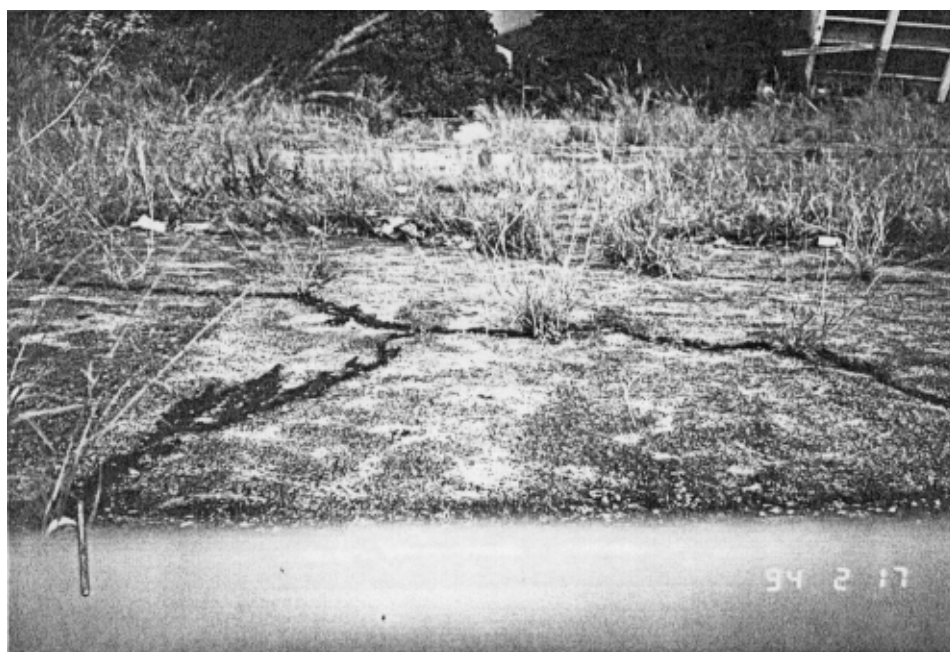
Plate 11 – View North-east From Toe of Slope Indicating Vegetation and Cracking on Hard Surfacing (Photograph Taken on 17 February 1994)
