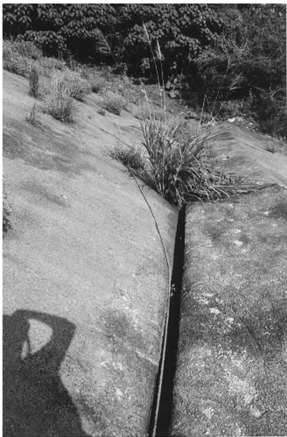
Plate 30 – View South-east Along Upper Berm at South-eastern End of Feature. Note Shotcrete Extending Over Lip of Channel and Vegetation Growing From Beneath Shotcrete (Photograph Taken on 5 May 1998)
