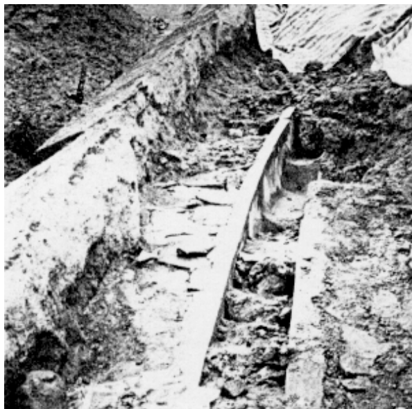
Plate 9 – View North-east Towards Crest of Slope at Location of "Washout" Indicating Old Surface Channel and Hard Surfacing Below 1977 Remedial Works Revealed During 1984 Remedial Works (Photograph Taken on 25 April 1984)
