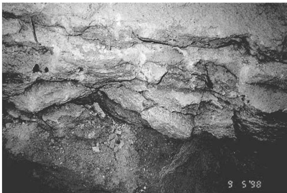
Plate 61 – Strip S3(A) Showing Close-Up of Multiple Layering of Hard Surfacing. Total Thickness Approximately 250–350 mm (Photograph Taken on 5 September 1998)
