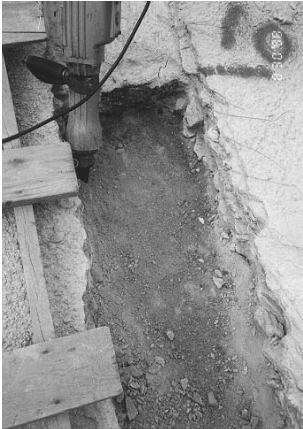
Plate 52 – Strip S2 Showing Fill Exposed Below Hard Surfacing 10 m Above Upper Berm. Note Numerous Layers of Hard Surfacing and Organic Deposit on Upper Face of Crack (Photograph Taken on 30 August 1998)
