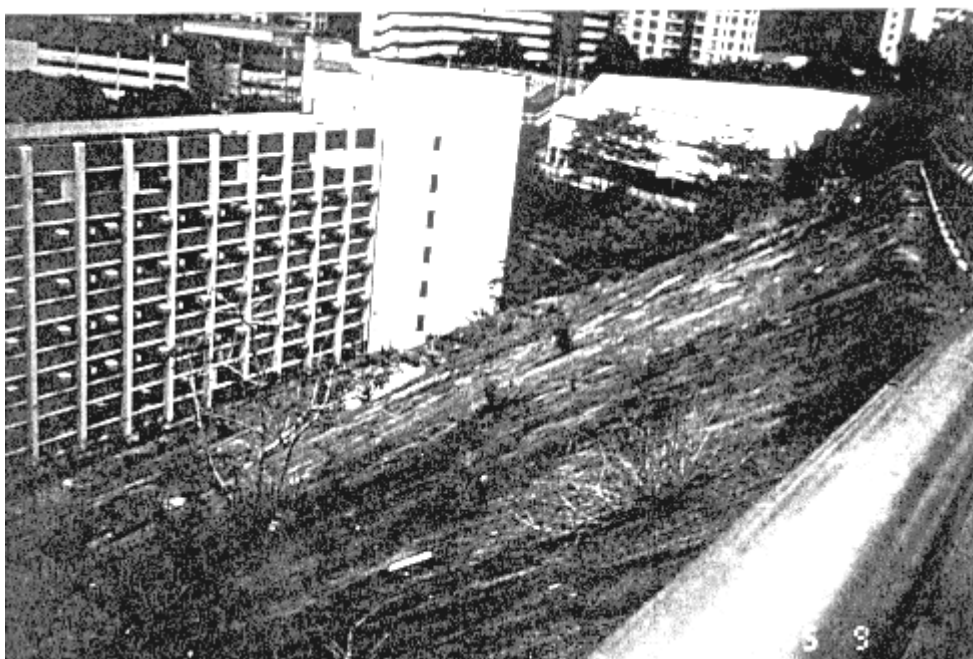
Plate 21 – View North-west Along Crest of Slope. Note Distortion in Hand Railing Along Crest (Photograph Taken on 9 May 1997)
