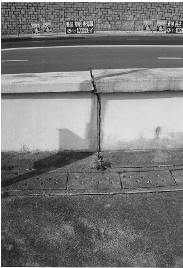
Plate 34 – Cracking at Construction Joint in Parapet Wall (Visible in Plate 33) (Photograph Taken on 5 May 1998)
