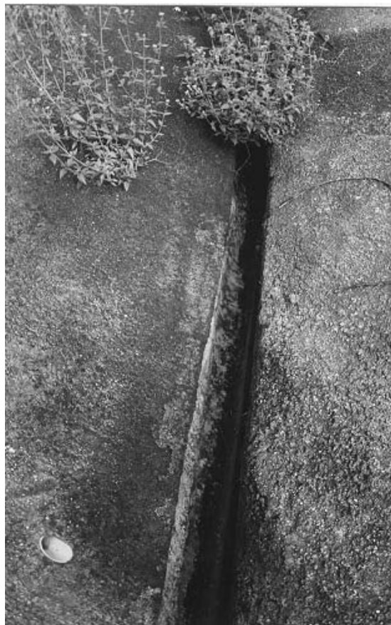
Plate 31 – View of Shotcrete Extending Beyond Lip of Channel on Upper Berm. Note Also Vegetation Growing From Beneath Shotcrete (Photograph Taken on 5 May 1998)
