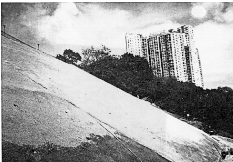
Plate 17 – View South-east Along Lower Berm. Re-Surfacing Works in Progress. Note Slight Convex Shape of Slope at Toe in Profile (Photograph Taken on 26 May 1995)
