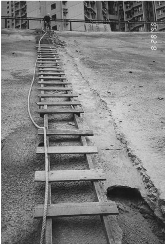
Plate 48 – Strip S2 – View From Upper Berm. Note Void Behind Previous Hard Surfacing Approximately 1 m Above Berm (Photograph Taken on 28 August 1998)
