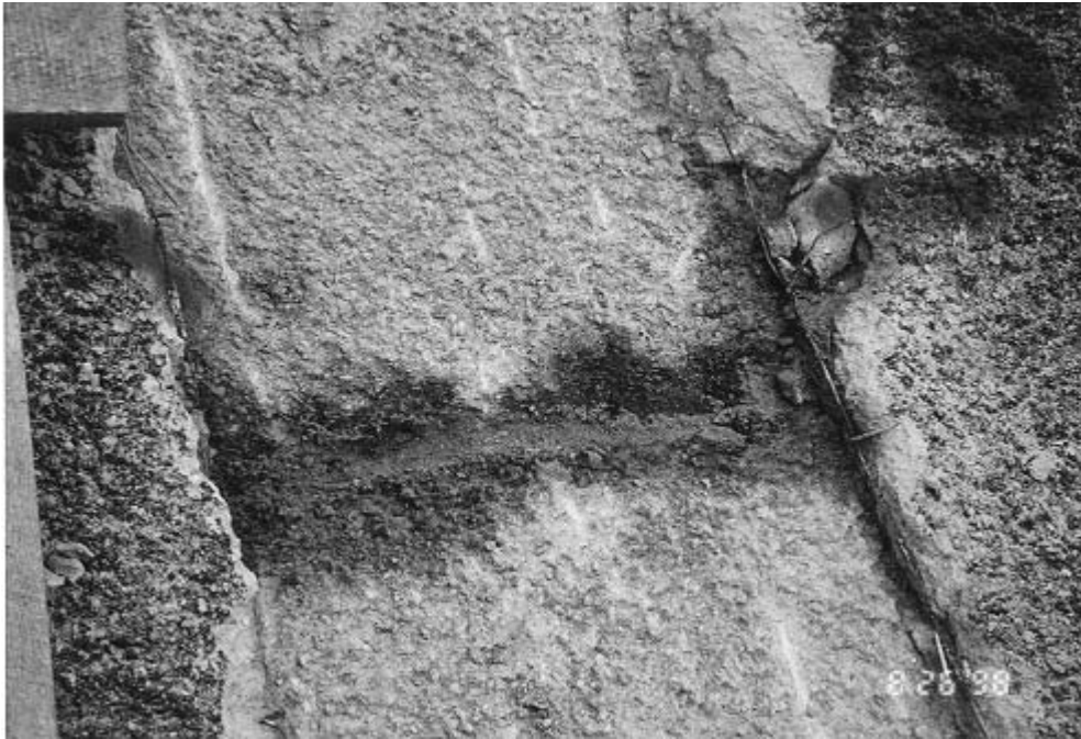
Plate 64 – Strip S4 (Middle Batter) Showing Cracking in Previous Hard Surfacing Approximately 16 m Above Lower Berm. Note Organic Fill and Rootlets (Photograph Taken on 26 August 1998)
