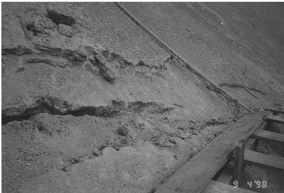
Plate 57 – Strip S3(A) Showing Cracking in Previous Hard Surfacing and Voiding Beneath Exposed Below 1998 Application of Shotcrete, Approximately 4 m Below Crest (Photograph Taken on 4 September 1998)
