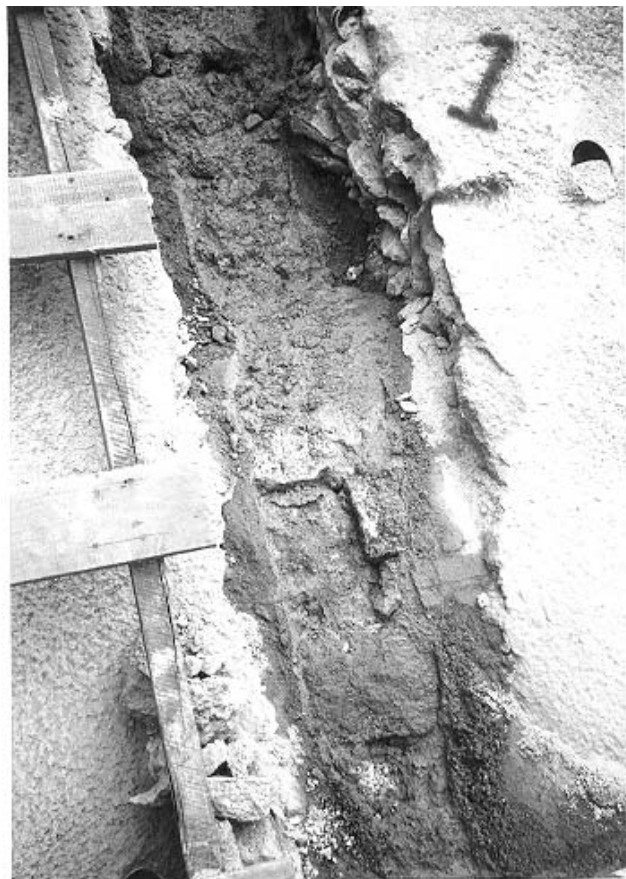
Plate 49 – Strip S2 Showing Stone Pitching Exposed Below 1998 Hard Surfacing. Note Numerous Layers of Surfacing (Photograph Taken on 29 August 1998)
