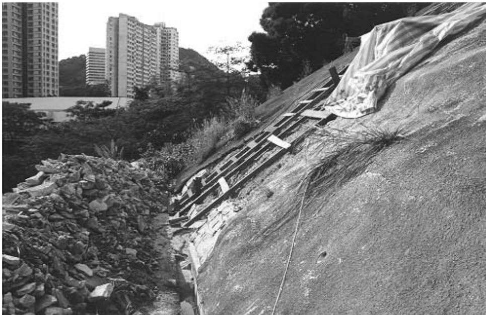
Plate 37 – View North-west Along Upper Batter Across Shotcrete Strip, North-western End of Feature. Note Stone Pitching Exposed and Cracking in Shotcrete Along Break in Slope. Note Also Convex Form of Stone Pitching and Void Between Shotcrete and Stone Pitching (Photograph Taken on 5 May 1998)
