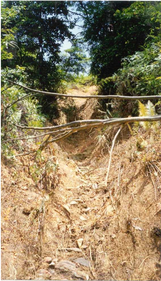
Plate 7 – Ephemeral Stream Course Below the Toe of the Surface of Rupture (Photograph taken on 17 June 1998)
