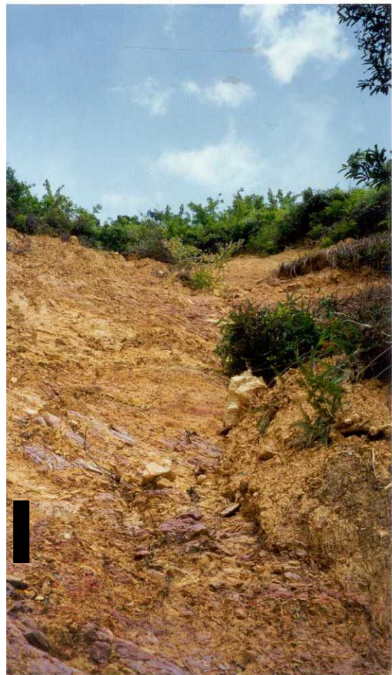
Plate 6 – View of Toe of Surface Rupture and Dense Vegetation Towards the Lower Portion of the Slope (Photograph taken on 17 June 1998)
