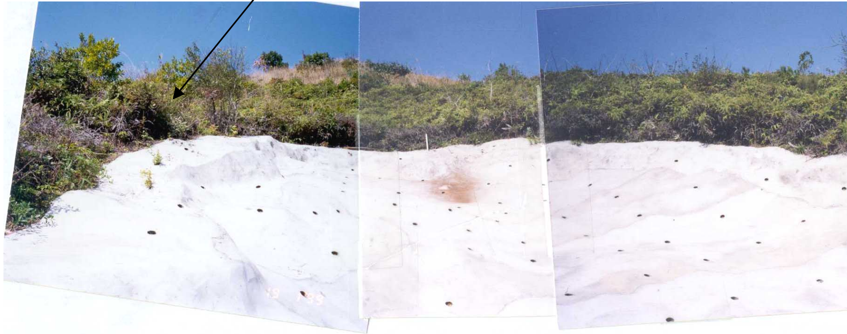
Plate 11 – Top of the Landslide Scar Following the Application of Chunum Surface Protection (Photograph taken on 19 January 1998)
