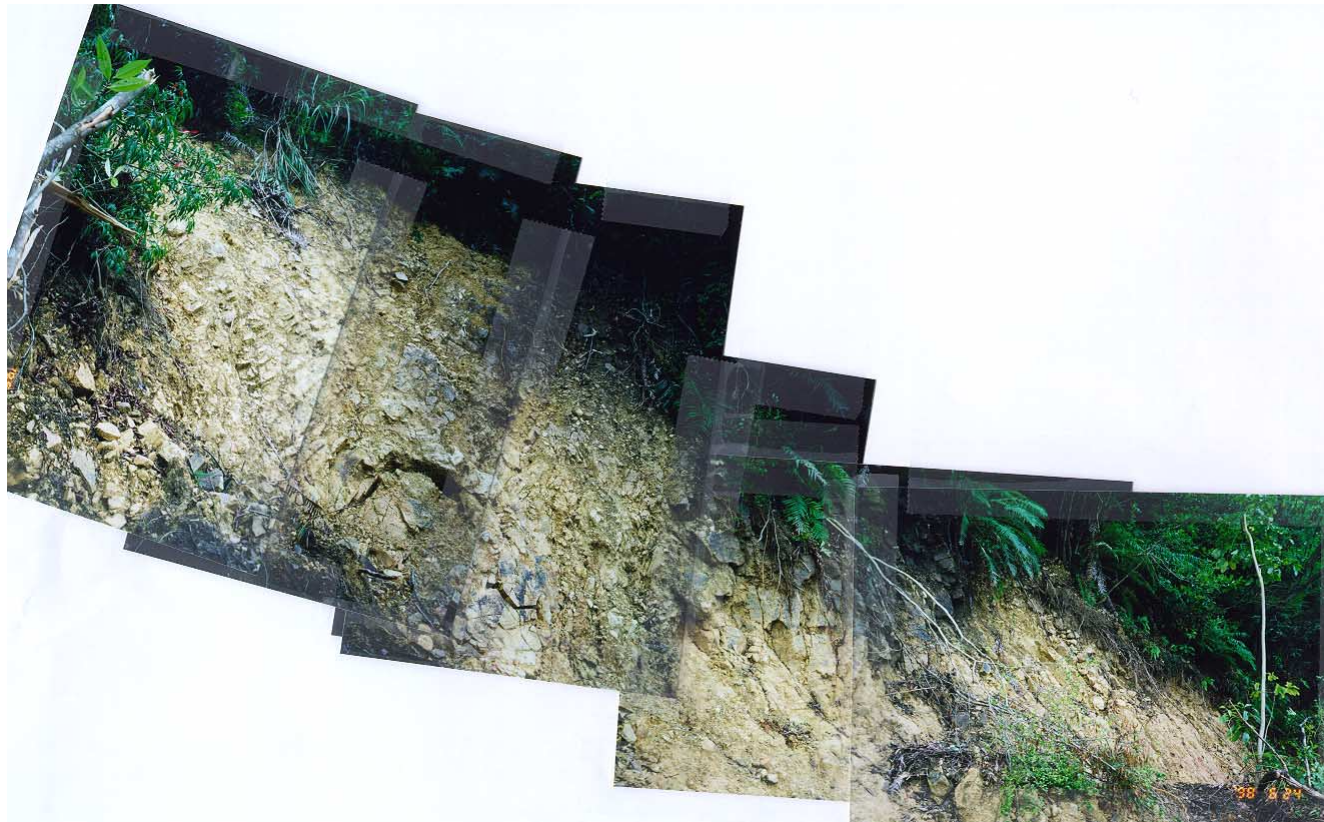
Plate 20 – Lower Landslide Backscarp – Dominant Westward dipping Joint Set Evident (Photographs taken on 24 June 1998)
