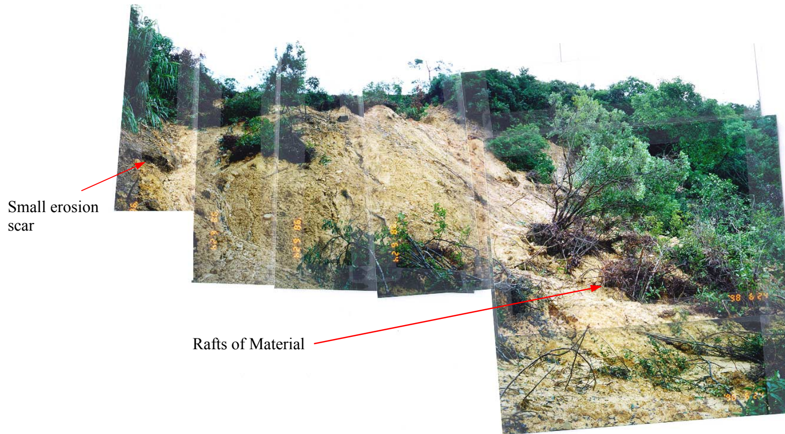
Plate 7 – General View of the Landslide Looking up to the Small Spur-type Feature from Below. Note the Rafts of Material in the Foreground as well as the Erosion Channels that have formed within the Landslide Debris (Photographs taken on 24 June 1998)
