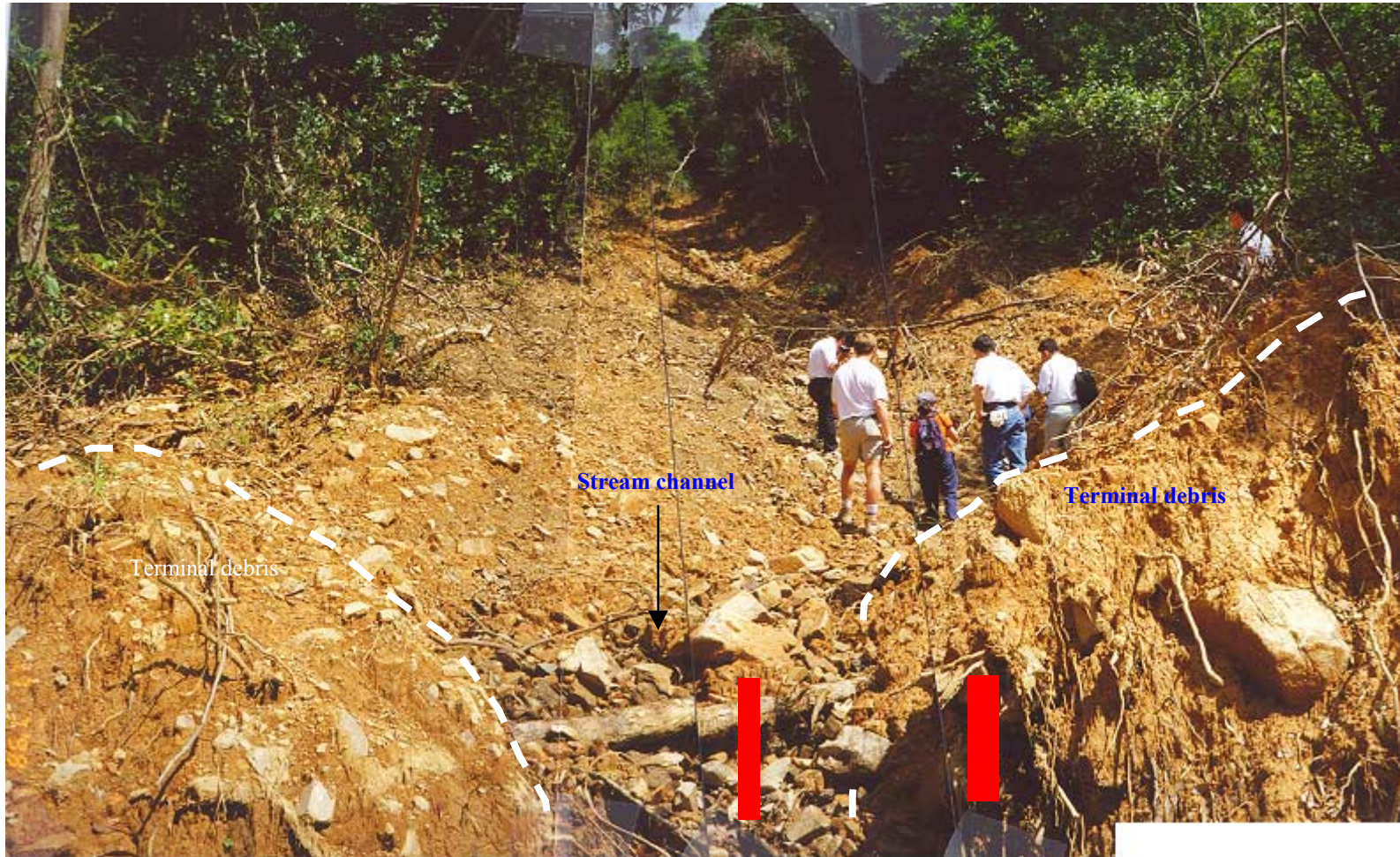
Plate 10 – View of Channel Cut through Terminal Debris above Toe Retaining Wall
