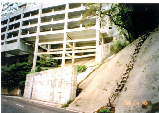
Plate 10 - Reinforced Concrete Boulder Barrier at Baguio Villa
