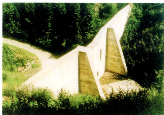
Plate 5 - Reinforced Concrete Barrier with Counterforts (Czerny, 1998)
