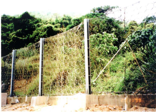
Plate 8 - Steel Boulder Fence in Fanling Area 49A
