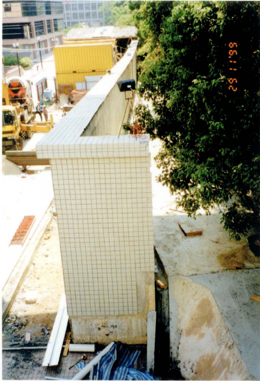
Plate 12 - 5-m High Reinforced Concrete Barrier at Kowloon Medical Rehabilitation Centre
