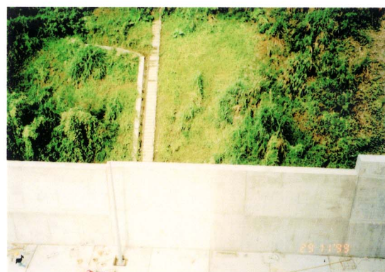
Plate 11 - Reinforced Concrete Landslide Debris/Boulder Barrier in Fanling Area 49A
