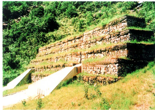
Plate 9 - Gabion-type Boulder Barrier Constructed at Yiu Hing Estate, Shaukeiwan
