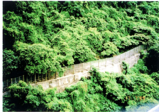
Plate 7 - Steel Boulder Fence below Seymour Cliff, Midlevels
