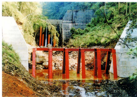
Plate 3 - 5-m High Slit Dam in Japan (Kawaken, 1998)
