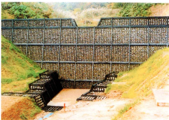
Plate 4 - Gabion-type Check Dam in Japan (Kawaken, 1998)
