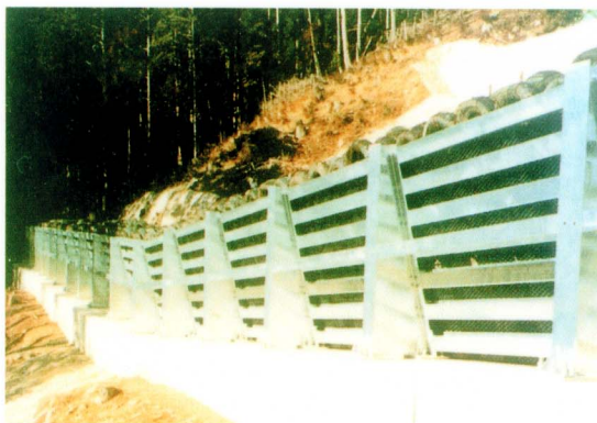
Plate 15 - Use of Rubber Tires to Soften Impact on Barrier (Kawaken, 1998)
