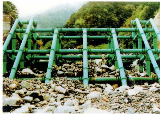
Plate 2 - Grid-type Steel Sabo Structure on Komu River in Japan (Kawaken, 1998)
