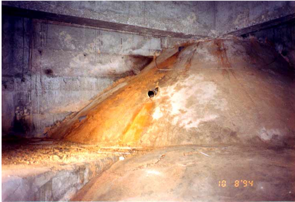
Plate M14 - The Ground underneath Block D Adjoining the Yard Area, with Signs of Seepage through the Weepholes, before Excavation of Trial Pit No. TP 35 (Photograph taken on 10 August 1994)
