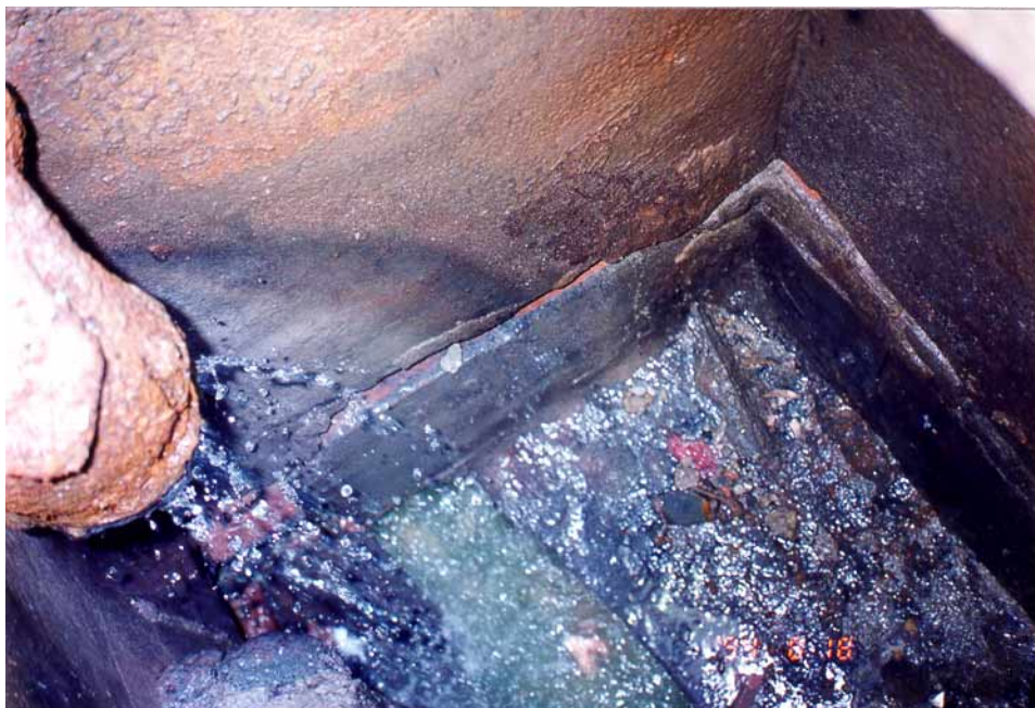
Plate M12 - Foulwater Manhole No. 34 with a Crack near the Base (Photograph taken on 18 August 1994)
