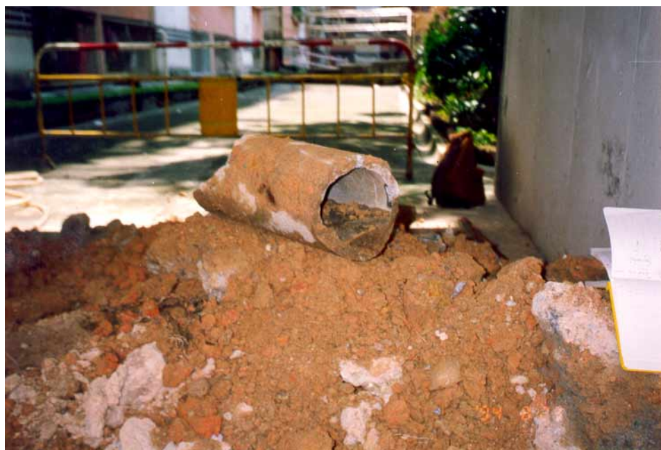
Plate M13 - Part of the Defective Stormwater Drain between Gully No. GT15a and Manhole No. 15 in the Yard Area (Photograph taken on 23 August 1994)
