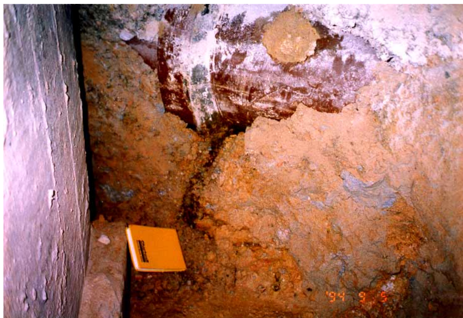
Plate M11 - Part of the Foulwater Sewer with Minor Leakage between Manhole No. 77 and the Landslide Scar (Photograph taken on 5 September 1994)
