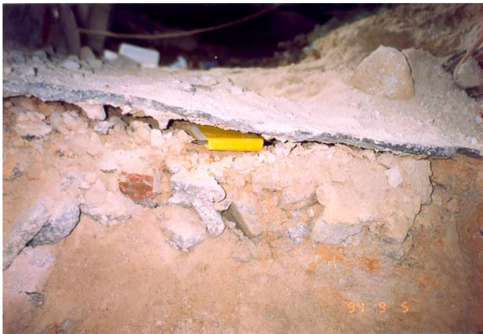
Plate M16 - Loose Fill near the Surface of the Ground underneath Block D (Photograph taken on 5 September 1994)
