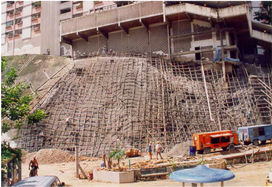
Plate M7 - View of the Landslide after Shotcreting on 29 July 1994
