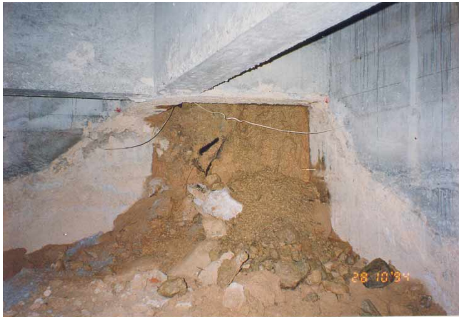
Plate M15 - The Ground below the Yard Area Exposed after Exposed after Excavation of Trial Pit No. TP 35 (Part of the ground collapsed when a field permeability test was carried out in drillhole No. BH12 sunk in the yard area. Photograph taken on 28 October 1994)
