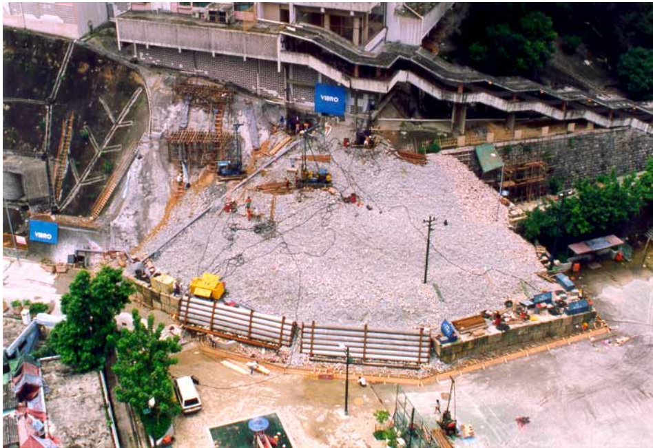
Plate M8 - View of the Landslide after Completion of Emergency Repair Works and during Ground Investigation (Photograph taken on 13 August 1994)
