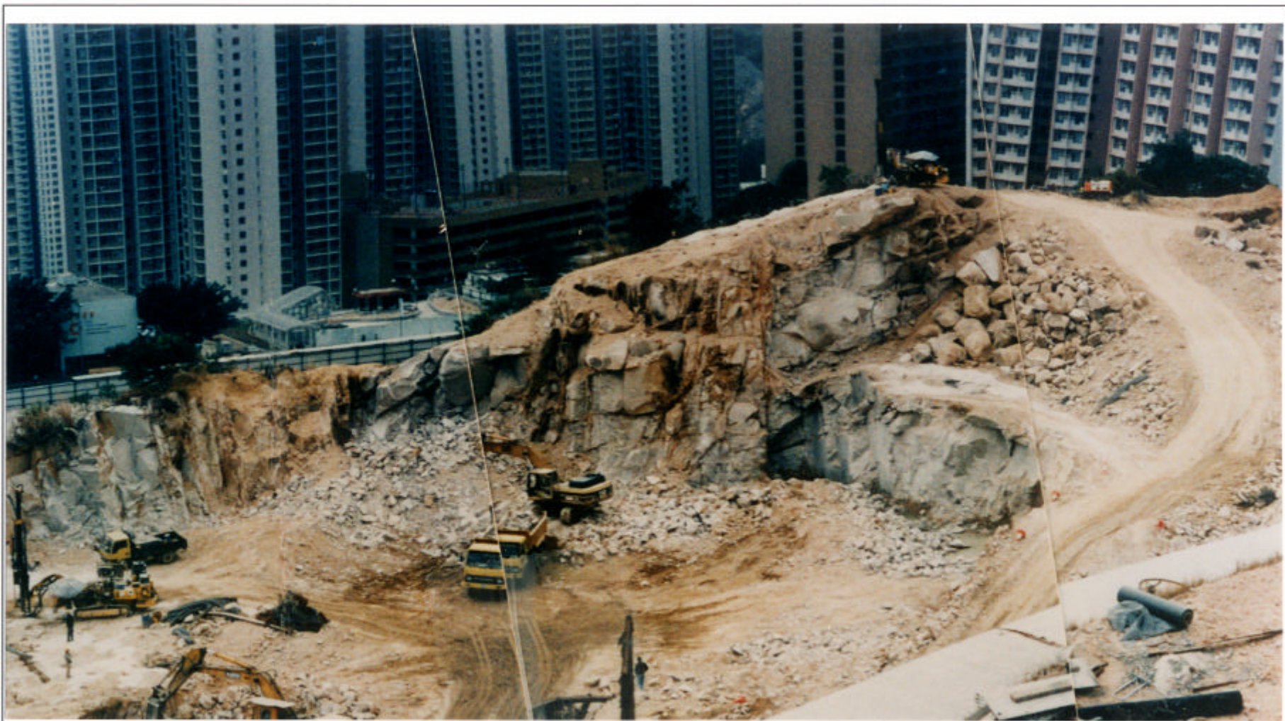
Plate 8 - An Enlarged View of the Crest and the Cut Face at the Back of the Failed Slope before the Failure (Extracted and Enlarged from Plate 7)
