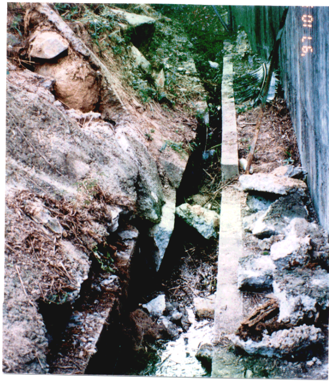
Plate 6 - Bulging and Collapse of Slope Toe (Photograph Taken on 30 October 1997)
