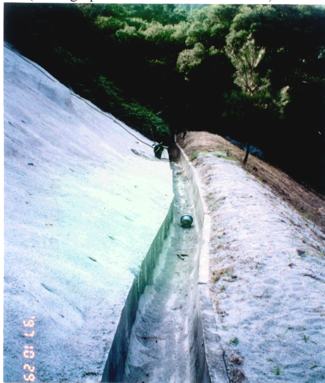
Plate 5 - Displacement of U-Channel along Lower Berm (Photograph Taken on 29 October 1997)
