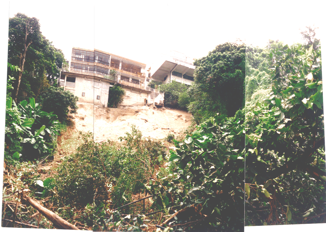
Plate 6 - Upslope View of the Landslide Scars (Photograph Taken on 11 July 1997) (Note the Undermining of the Stairwell in the Centre of the Photograph)
