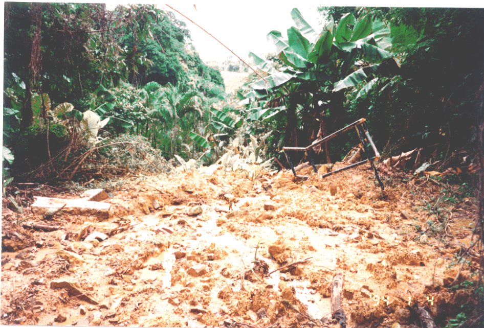
Plate 5 - Hand Railings Found Near the Toe of the Debris (Photograph Taken on 17 June 1997)
