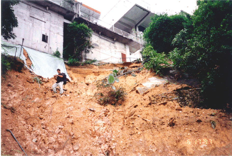
Plate 2 - View of the Main Scarp of the Landslide of 4 June 1997 (Photograph Taken on 17 June 1997) (Note the Plastic Pipes Attached to the Front Wall of the Podia as Indicated by the White Arrow)
