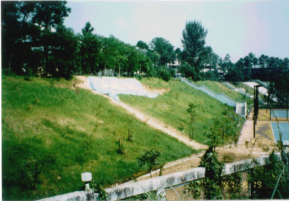
Plate 1 - View North Showing Failure B comprising 35 m-long Scarp on the Fill Slope (Photograph Taken on 19 August 1997)
