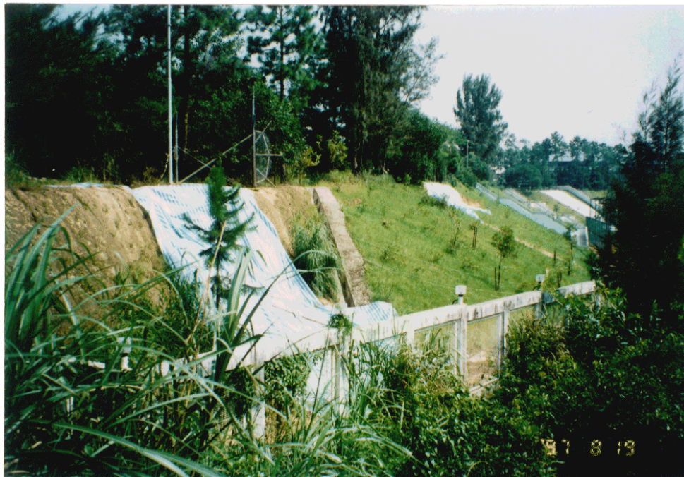
Plate 2 - View North Showing Failure A on the Cut Slope with the Fill Slope Shown in the Background (Photograph Taken on 19 August 1997)
