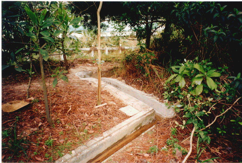
Plate 5 - U-channel Constructed between the Existing Drainage Channels at the Crest of the Fill Slope During Remedial Works (Photograph Taken on 24 February 1998)
