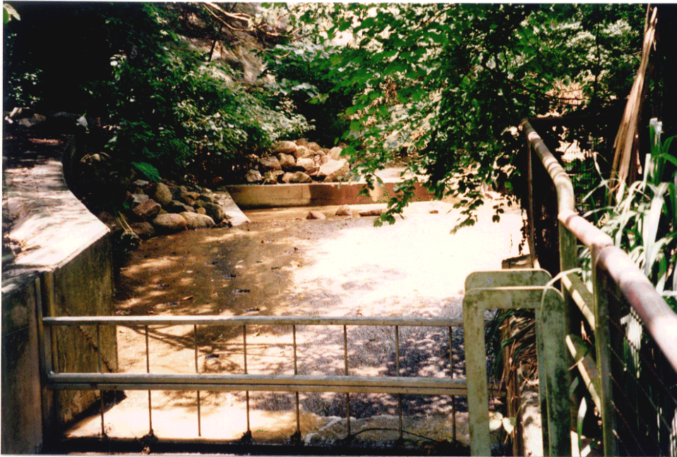
Plate 4 - View of the Entrance to the Drainage Cascade, Showing the Steel Grill Gate (Photograph Taken on 16 June 1998)
