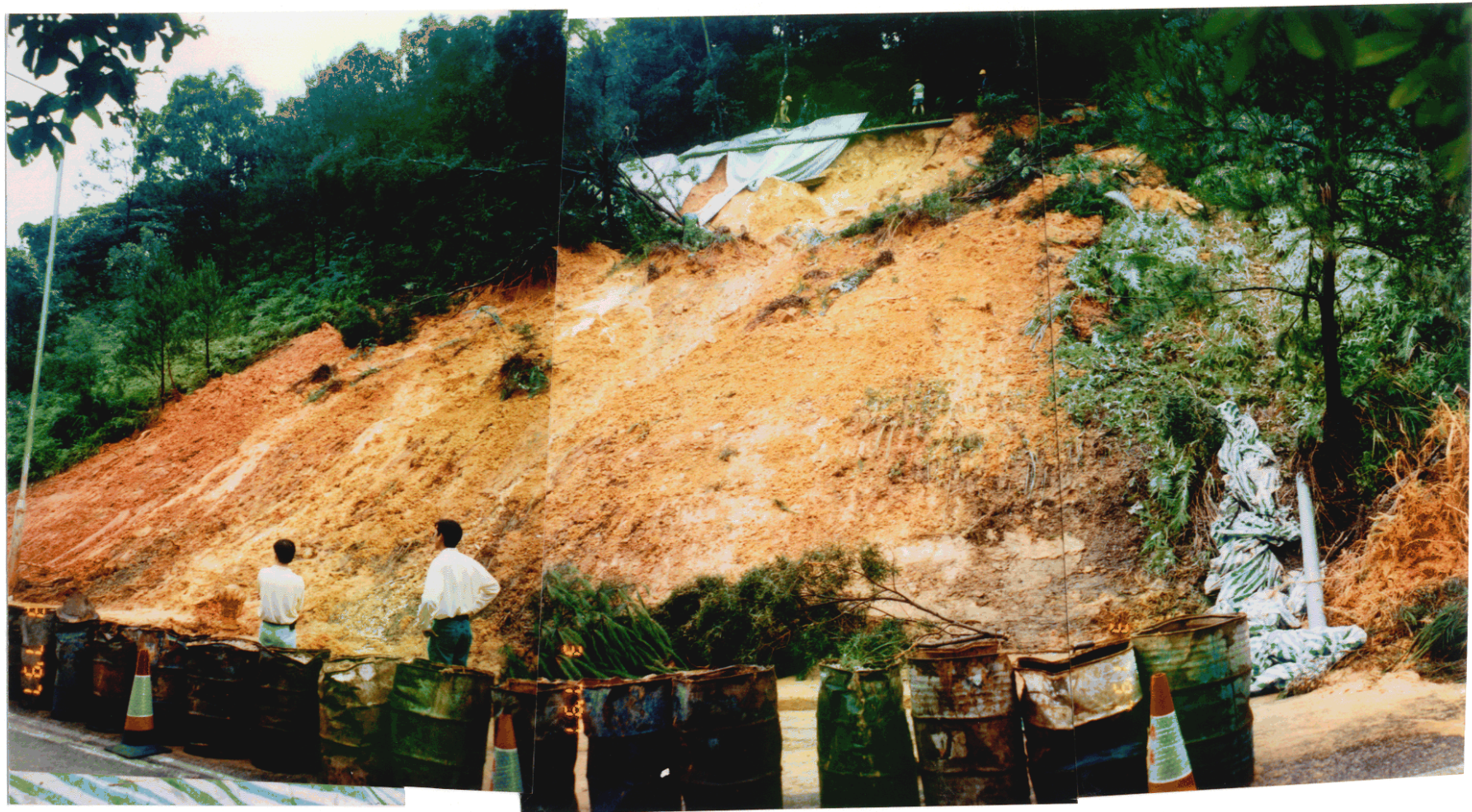
Plate 5 - View of the Landslide (Photograph Taken on 3 July 1997. Note the Colour Change Across the Site from Orangish Red Residual Soil to Orangish Yellow Completely Decomposed Volcanics)
