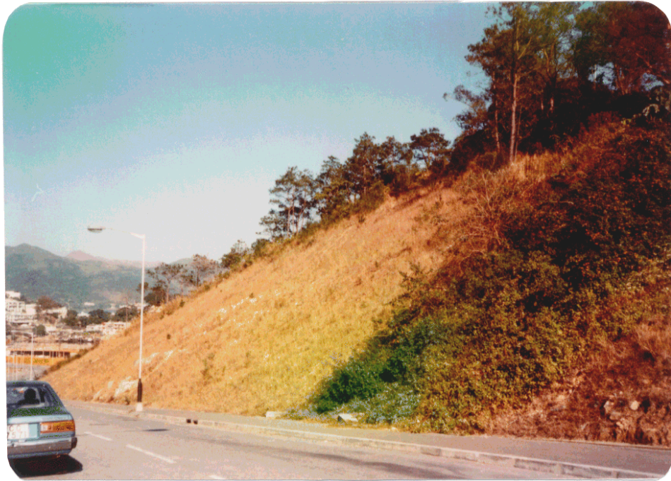
Plate 4 - Site Record Photograph Showing "Lush Growth Where There is a Perennial Discharge into Cracked Surface Water Drains" (Photograph Taken on 14 January 1981)
