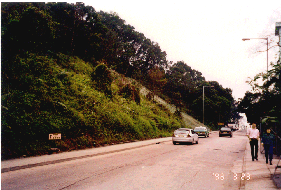
Plate 1 - View of Hong Tsuen Road and Adjacent Cut Slope No. 8SW-C/C3 After Urgent Repair Work was Completed (Photograph Taken on 23 March 1998. Note the Photograph is Looking Southwest and the Landslide Occurred Where the Slope is Shotcreted, Near the Lamp Post)
