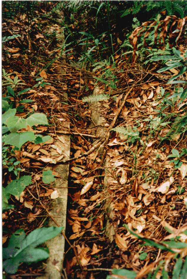
Plate 2 - Partly Blocked Drainage U-channel on the Second Bench Adjacent to the Southwest Flank of the Landslide (Photograph Taken on 23 March 1998)
