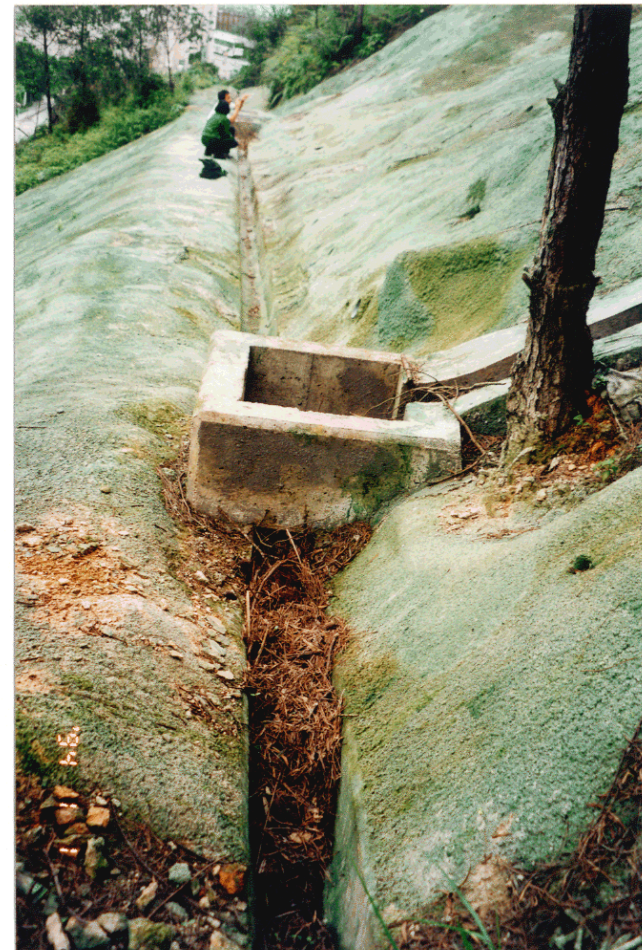
Plate 3 - Drainage U-channel Partially Blocked by Vegetation at a Catchpit (Photograph Taken on 23 March 1998. Note the Blockage Occurred after Repair Works were Completed)
