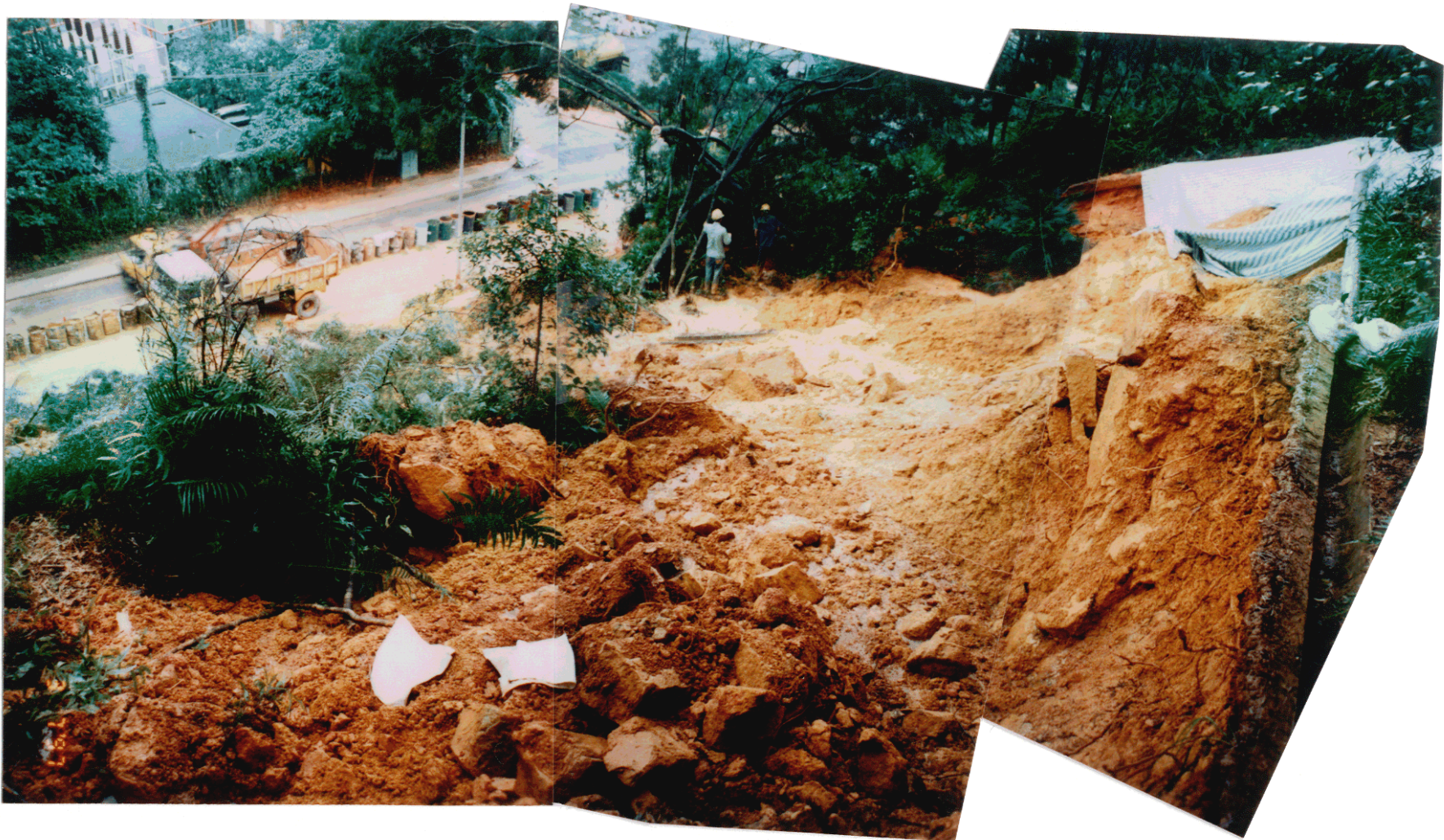
Plate 9 - View of the Main Scarp Looking North (Photograph Taken on 3 July 1997. Note the Exposed Corestone Comprising Jointed Moderately Decomposed Volcanics in the Main Scarp and the Issue of Groundwater)
