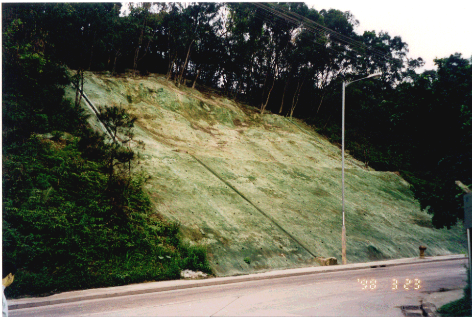
Plate 10 - View of Slope No. 8SW-C/C3 after Urgent Repair Work was Completed (Photograph Taken on 23 March 1998. Note the Landslide Scar Visible on the Upper Part of the Slope and Daylighting at the First Bench)
