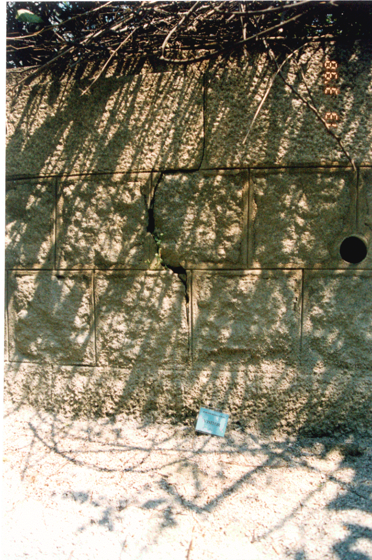
Plate 6 - Crack in the Retaining Wall above the Landslide (Photograph Taken on 13 March 1998)
