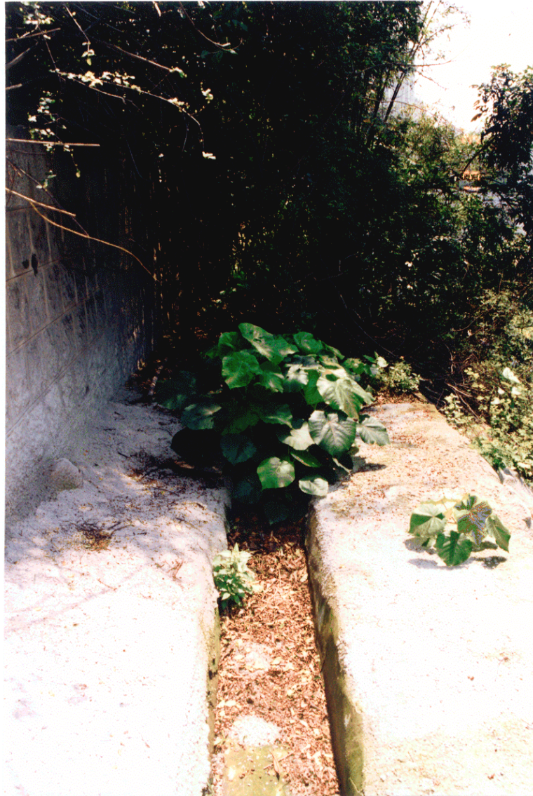
Plate 5 - U-channel at the Crest of the Slope with Infilling of Vegetation (Photograph Taken on 13 March 1998)
