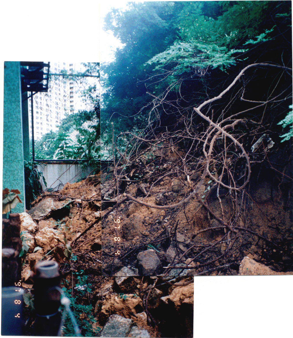
Plate 1 - Landslide Debris between the Slope and School Wall (Photograph Taken on 4 August 1997)
