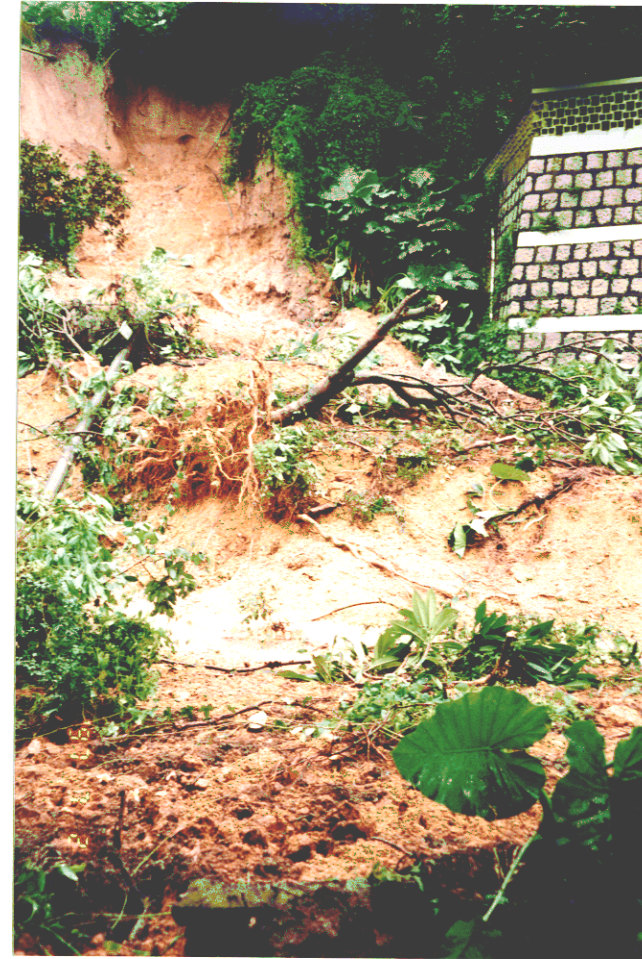
Plate 5 - View of the Western Flank of the Main Landslide Showing a Section of Masonry Retaining Wall within the Landslide Debris (Photograph Taken on 2 July 1997)
