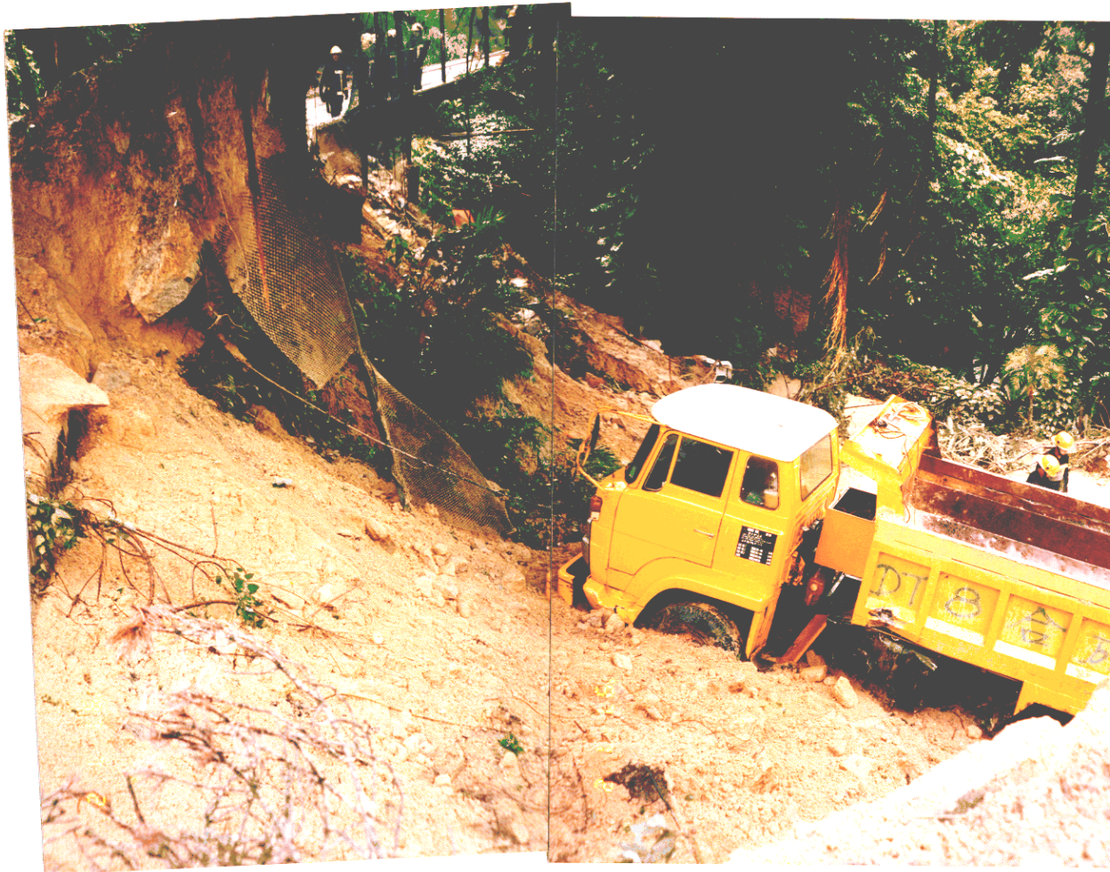
Plate 6 - View from the Elevated Road to No. 369 Riviera Apartments Showing the Dump Truck which was Carried by the Landslide down the Slope below Castle Peak Road (Photograph Taken on 2 July 1997)
