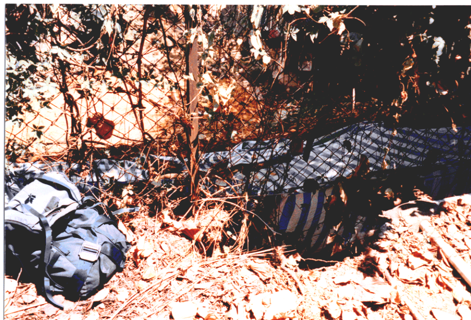
Plate 7 - View Showing the Undermining of the Lower Platform at the Crest of the Slope behind the Girls Toilet Block of Kwai Chung Public School (Photograph Taken on 15 May 1997) (Note the Two Water Supply Pipes in the Right-Hand Corner of the Photograph)
