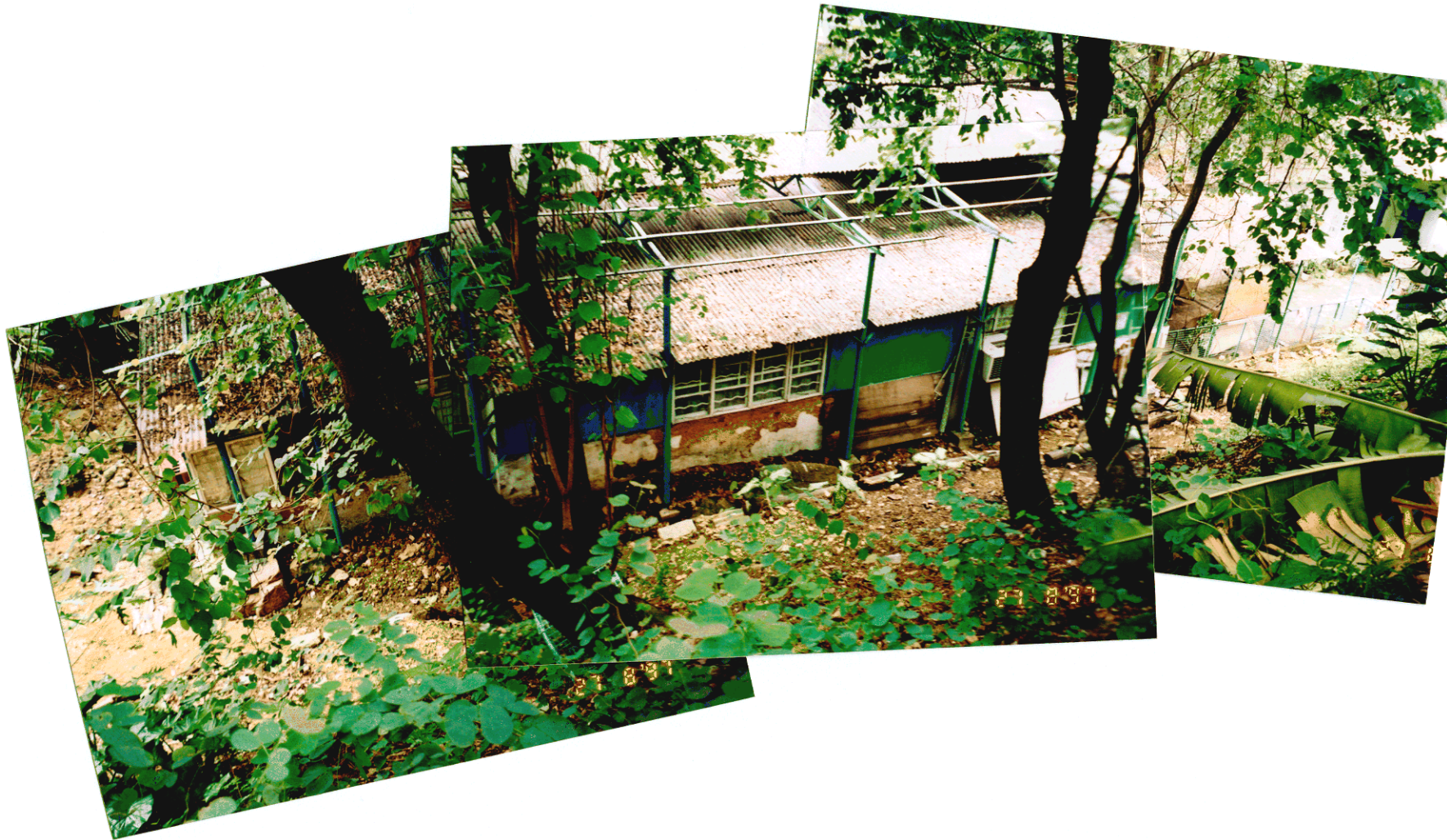
Plate 3 - View Downslope to Glorious Praise Christian Centre Showing the Open Ditch at the Toe of the Slope (Photograph Taken on 27 August 1997)
