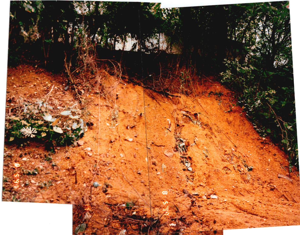
Plate 1 - View of the Landslide Showing the Debris on the Slope (Photograph Taken on 9 May 1997) (Note the Main Scarp is Obscured at the Crest of the Slope)
