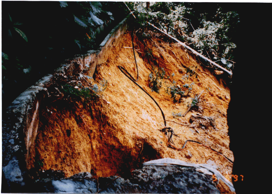
Plate 2 - View of 500 mm U-Channel at the Crest of the Landslide (Photograph Taken on 5 June 1997)
