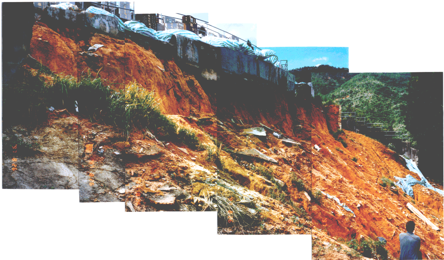
Plate 6 - The Main Scarp of Landslide B (Photograph Taken on 26 August 1997) (Note the Smooth Surface of the Pre-existing Slope)
