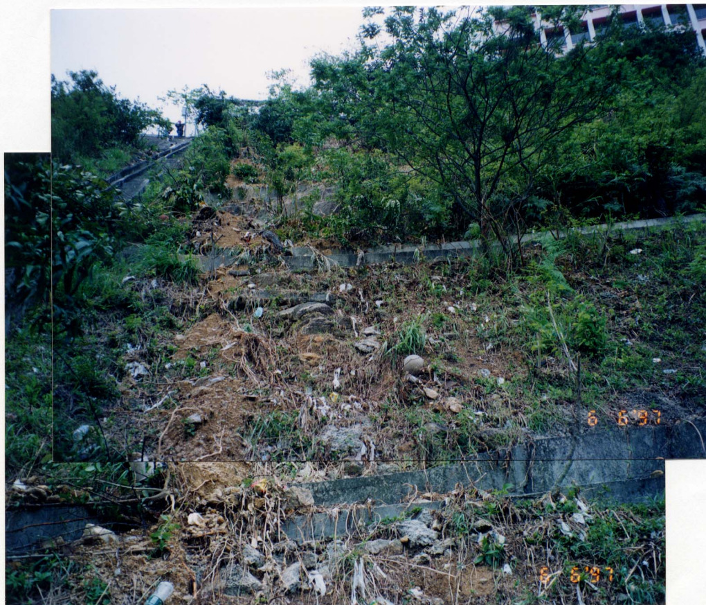
Plate 6 - Upslope View of the Landslide Run-out Track (Photograph Taken on 6 June 1997)
