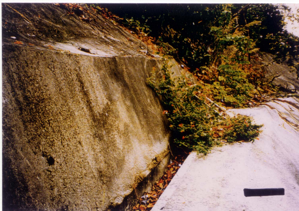
Plate 8 - Partial Obstruction of U-Channel above the Landslide Scar (Photograph Taken on 6 June 1997)
