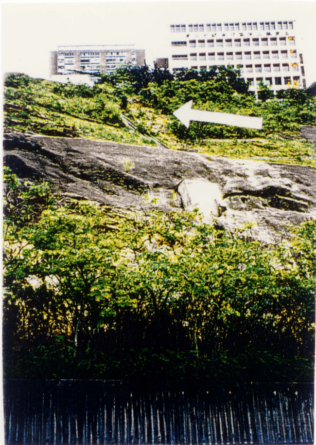
Plate 2 - Close View of Slope No. 11NW-A/C7. The Arrow Shows the Landslide Run-out Track (Photograph Taken on 6 June 1997)
