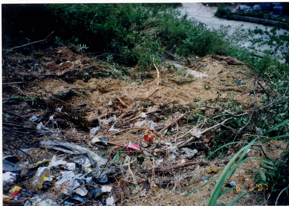
Plate 5 - Landslide Debris at the Toe of the Soil Portion of Slope No. 11NW-A/C7 (Photograph Taken on 6 June 1997)
