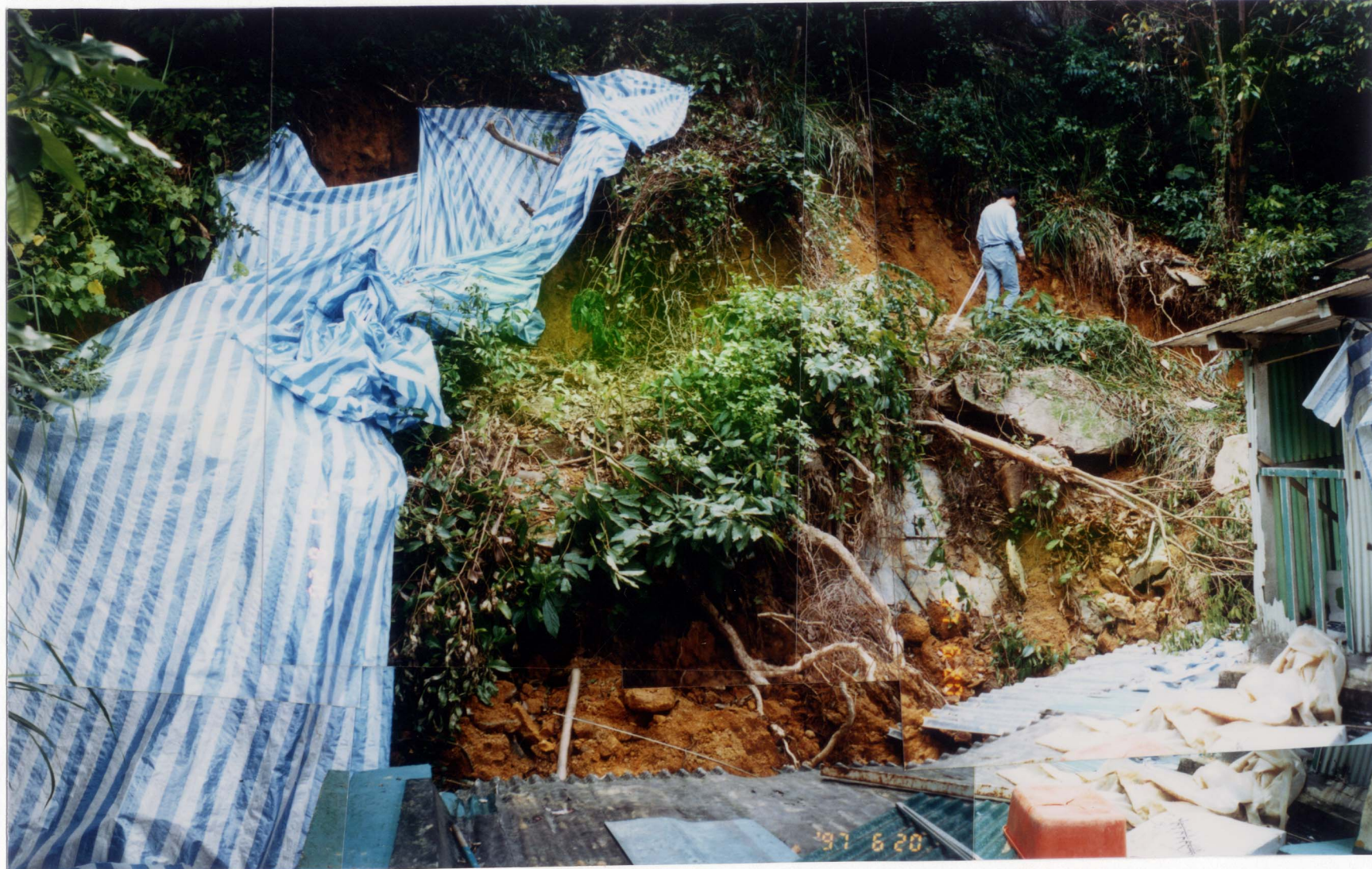
Plate 6 - View of Landslide A (Photograph Taken on 20 June 1997. Note the Entire Slope Shown in Plate 2 has Failed)
