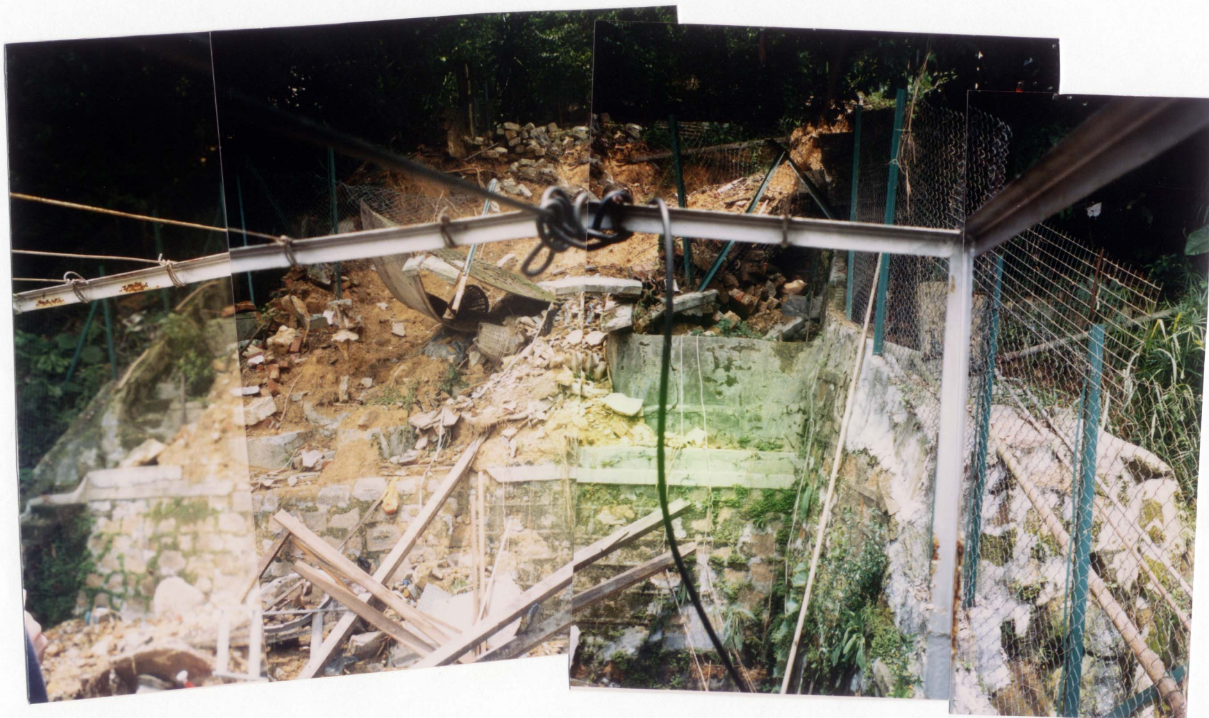
Plate 9 - View of Landslide C (Photograph Taken on 6 June 1997. Note that the Fill Platform was Located Near the Top of the Landslide Scar)
