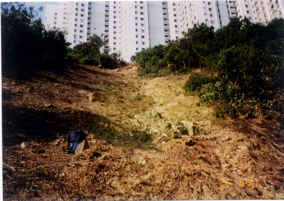
Plate 4 - View Looking Up Run Out Track (Photograph Taken on 26 May 1997)
