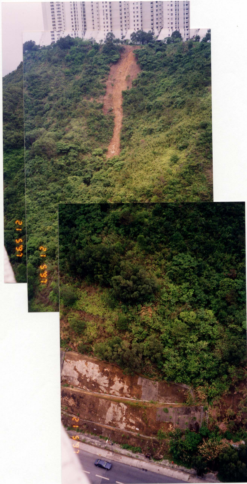
Plate 1 - General View of Landslide (Photograph Taken on 21 May 1997)
