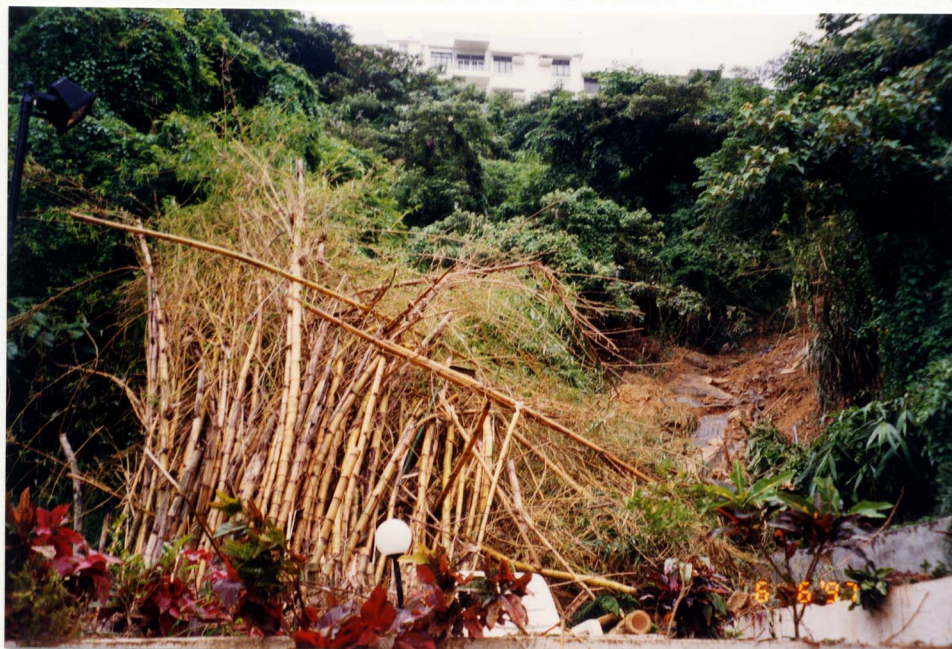
Plate 4 - Upslope View of the Gully at Incident No. MW97/6/12 (Photograph Taken on 6 June 1997. Note the Intact Raft of Landslide Debris Covered by Bamboo)
