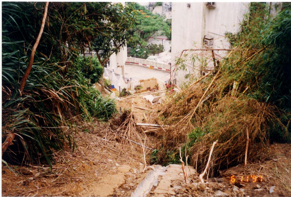
Plate 3 - Southwestern View of the Lower Part of the Gully Showing the Distribution of Landslide Debris from Incident No. MW97/6/12 (Photograph Taken on 11 June 1997. Note the Vegetation Pile on the Right of the Frame and the Debris on the Patio Areas of Woodcrest Hill)
