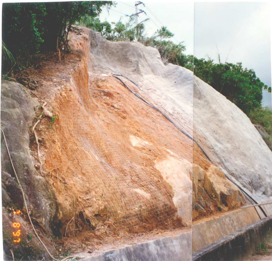
Plate 2 - Landslide 'B' on the Tai Lam Chung Catchwater Cut Slope No. 6SE-D/CR135 (Photograph Taken on 7 August 1997)
