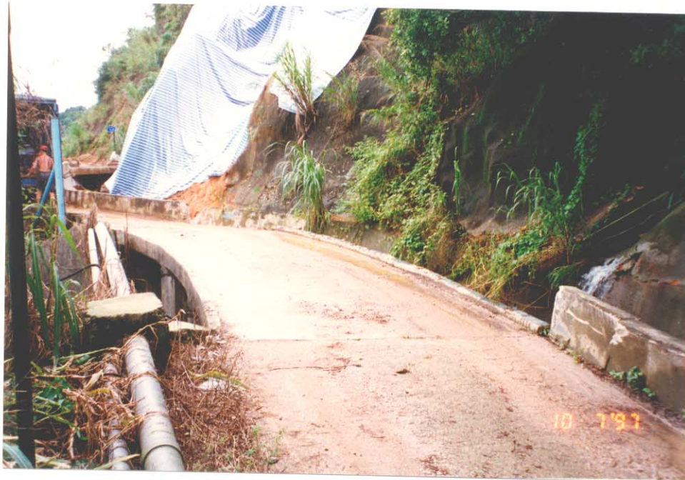
Plate 1 - View Showing Overflow Weir 'X' and Landslide 'A' on the Tai Lam Chung Catchwater Cut Slope No. 6SE-D/CR135 (Photograph Taken on 10 July 1997)
