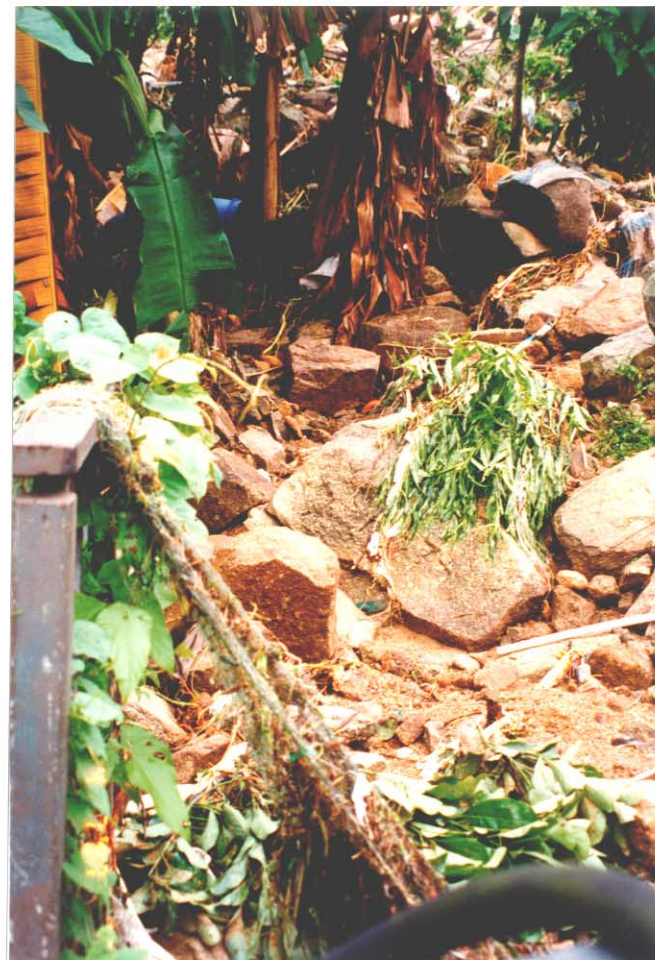
Plate 8 - Trapezoidal Drainage Channel 'D' Completely Blocked with Flood Debris (Photograph Taken on 4 July 1997)
