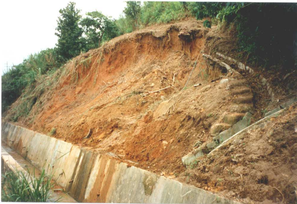
Plate 3 - Landslide 'C' on the Tai Lam Chung Catchwater Cut Slope No. 6SE-D/CR135 (Photograph Taken on 7 August 1997)
