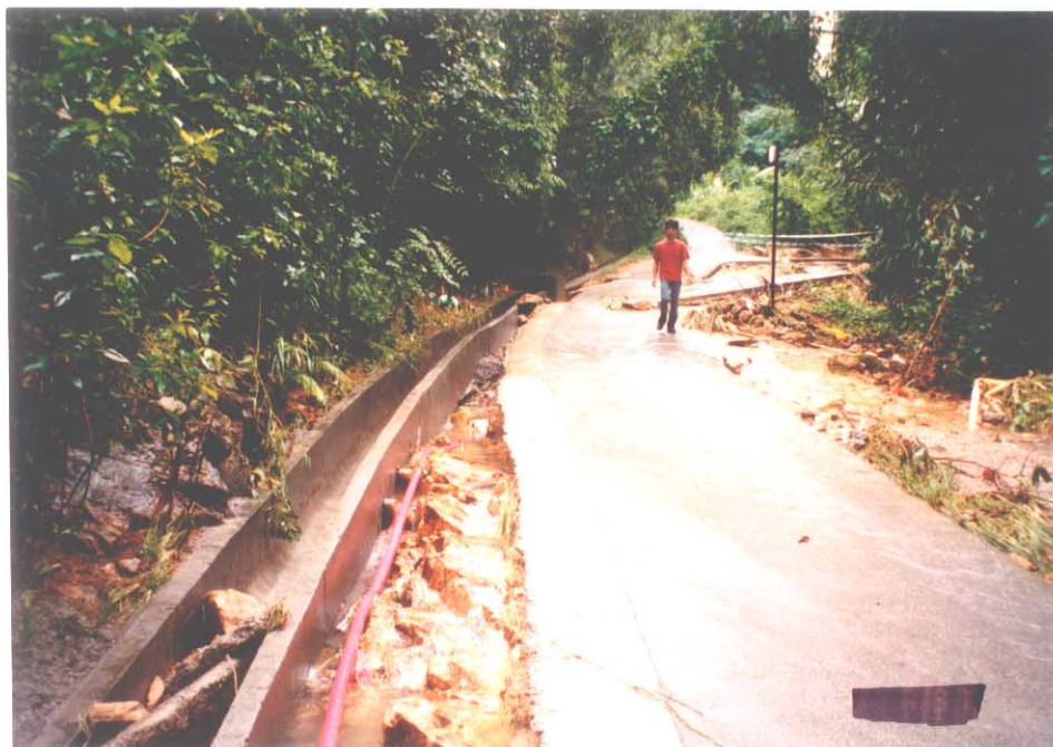
Plate 7 - Gully Erosion alongside Fuk Lok Tsuen Footpath (Photograph Taken on 3 July 1997)
