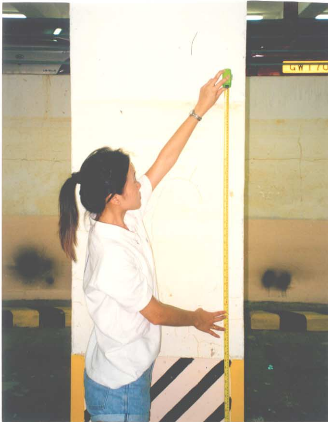
Plate 2 - View of Floodwater Staining, up to 1.7 m, in Car Park (Photograph Taken in August 1997)
