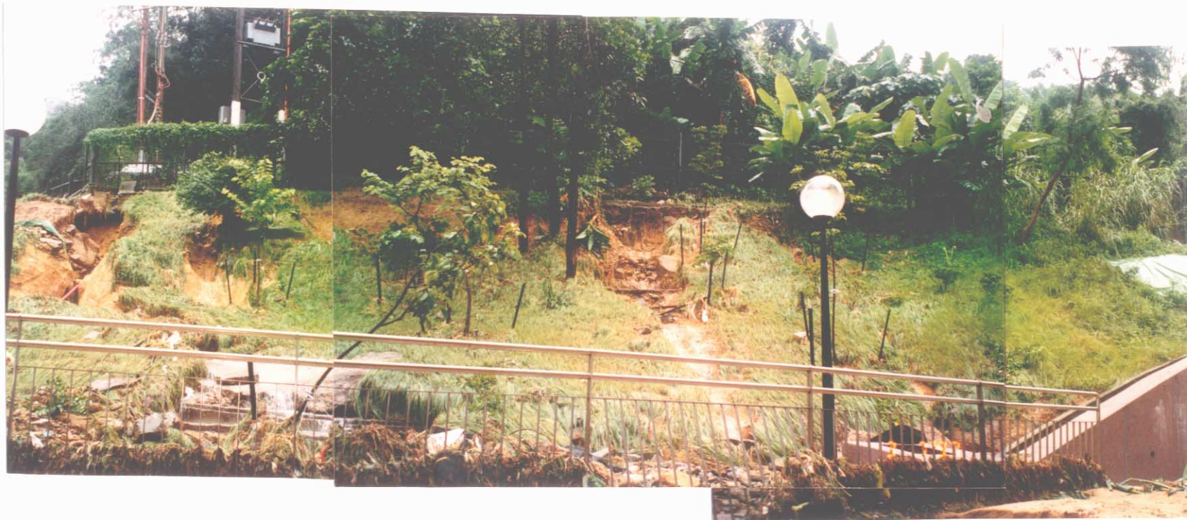
Plate 9 - Photograph Showing Flood Damage to Cut Slope No. 7SW-D/C791 at Mei Chung Court (Photograph Taken on 3 July 1997)
