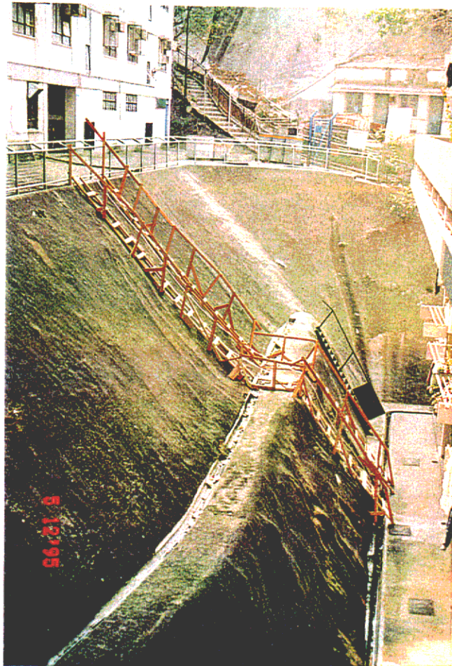
Plate 1 - Trial Site A - View looking south west at shotcreted section of slope. Note zones of seepage from weepholes adjacent to the access ladder. (EG95/143/1)
