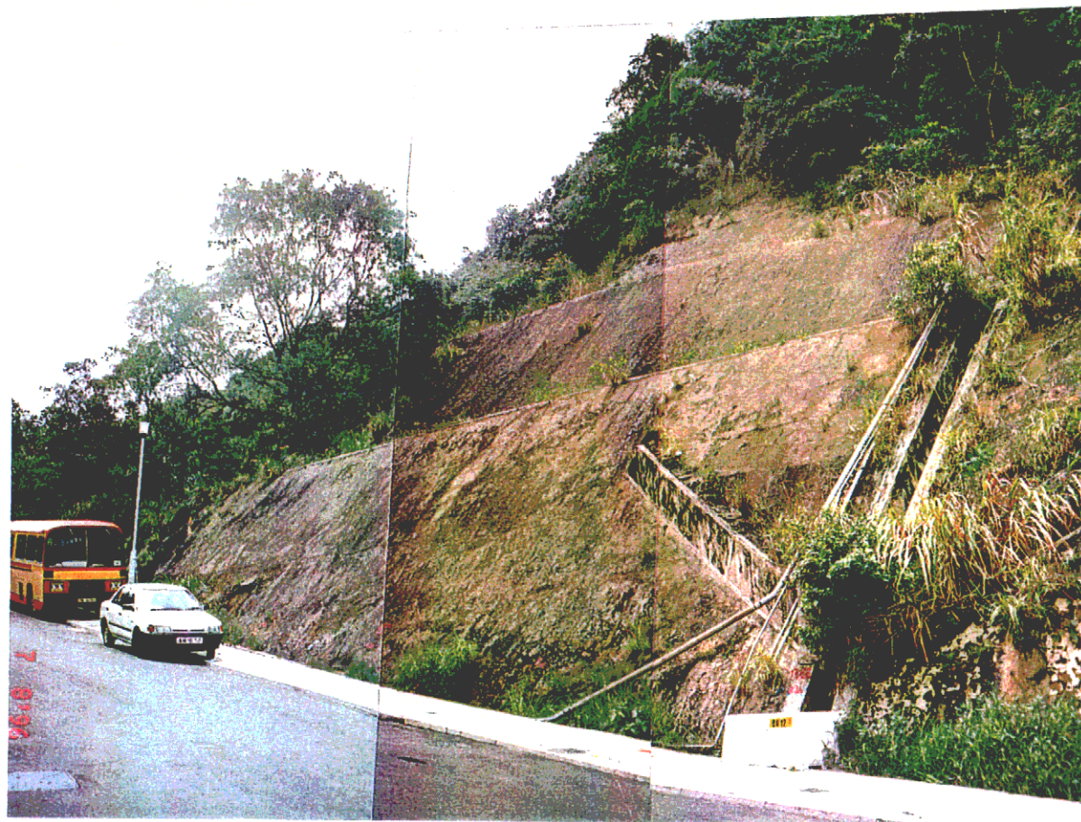
Plate 9 - Trial Site G - View of cut slope looking south east. Note single corestone protruding from slope face close to white motor car. (EG96/68/13,14,15)
