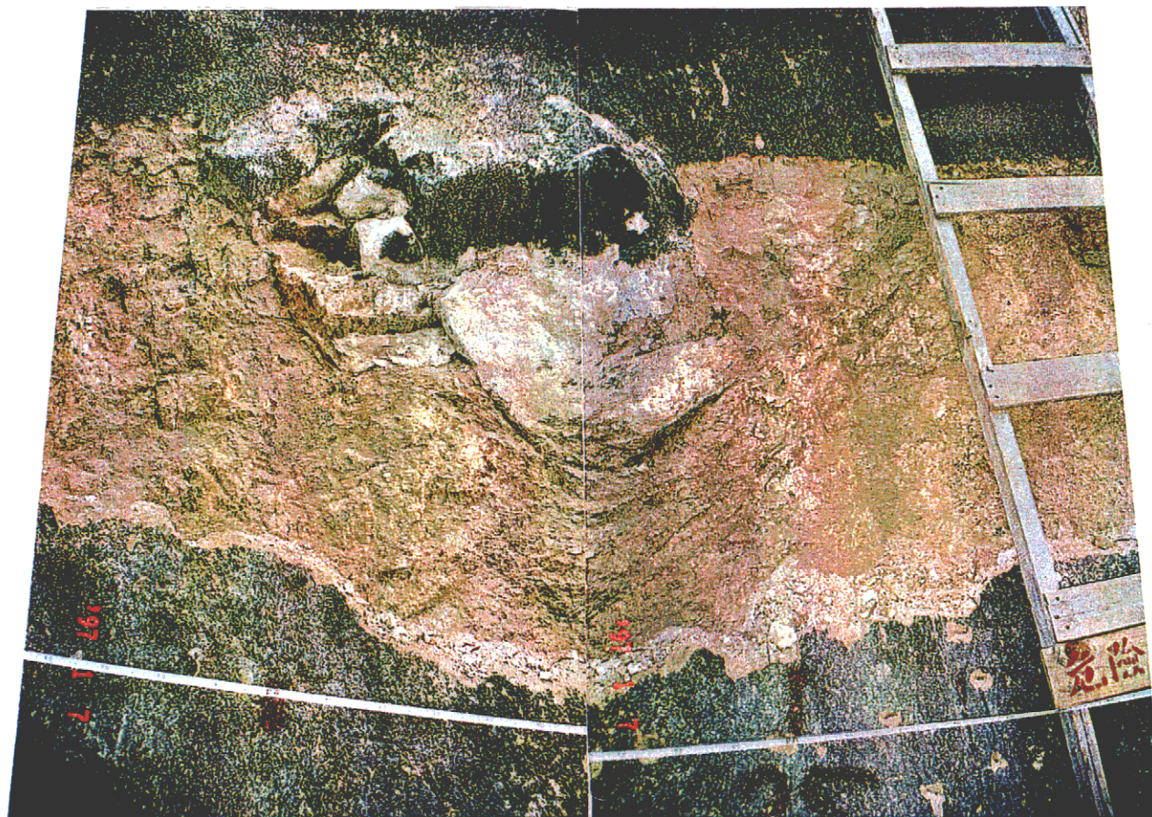
Plate 12 - Corestone of moderately decomposed granite exposed along chunam strip CSG1 at Site G. (EG97/03/4,5)
