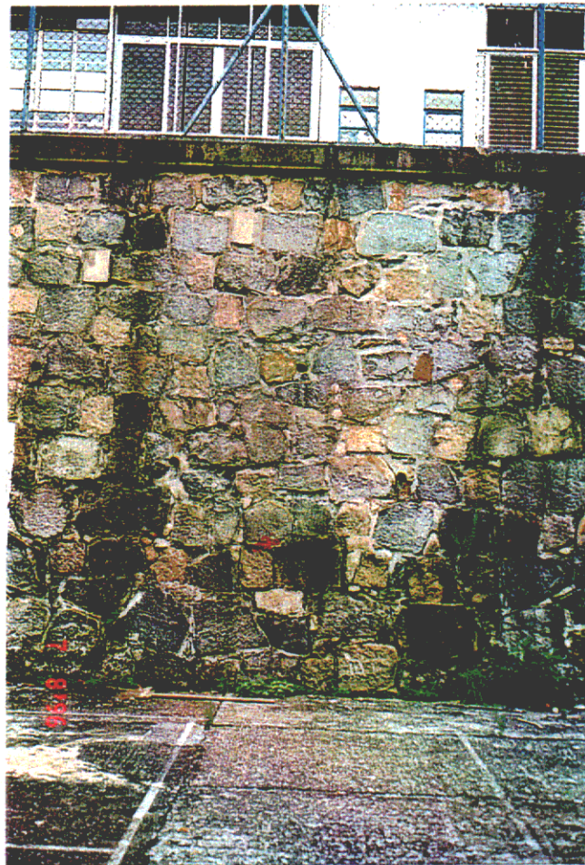
Plate 8 - Trial Site F - Granite headers in tied masonry wall. (EG96/69/21)
