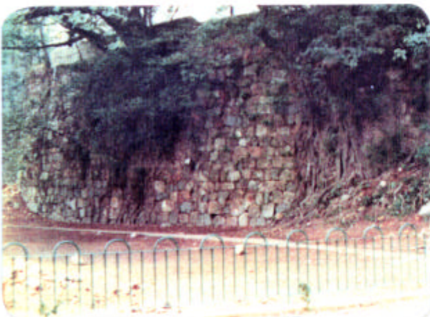
Plate D3 - Dry Packed Squared Rubble Wall (11SW-A/R109)
