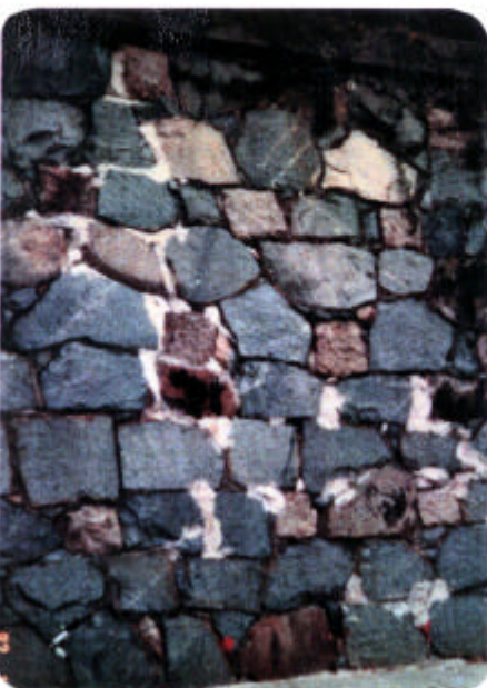
Plate D11 - Random Rubble Wall with Stone Ties
