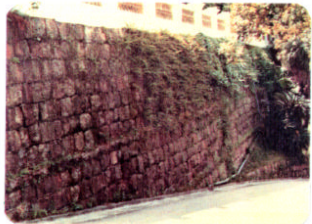
Plate D4 - Dry Packed Squared Rubble Wall with Horizontal Beams (11SW-A/R163)
