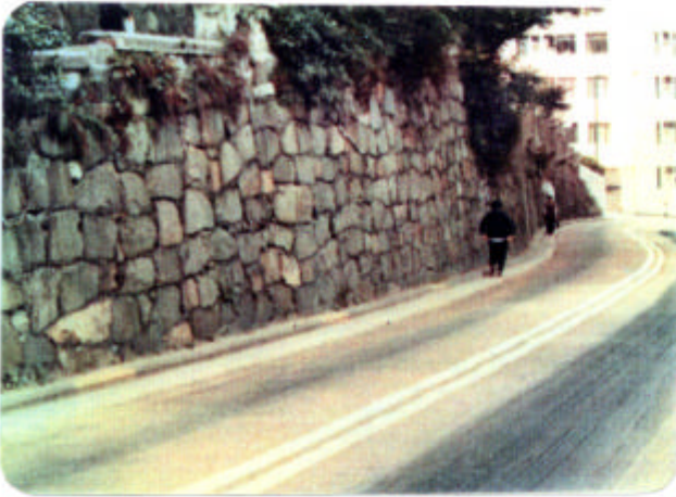
Plate D1 - Dry Packed Random Rubble Wall (11SW-A/R389)
