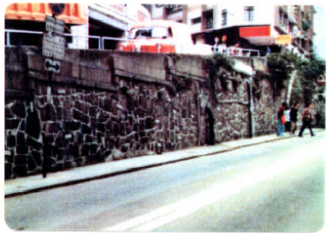
Plate D2 - Pointed Random Rubble Wall (11SW-A/R116)
