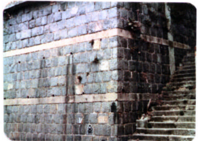
Plate D8 - Dressed Block Wall with Horizontal Beams (11SW-A/R423)
