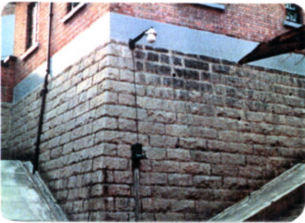
Plate D7 - Dressed Block Wall (11SW-A/R46)
