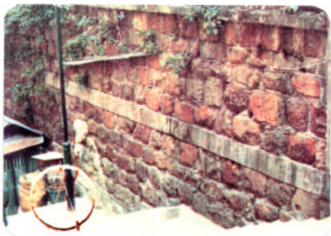
Plate D6 - Pointed Squared Rubble Wall with Horizontal Beams (11SW-A/R194)
