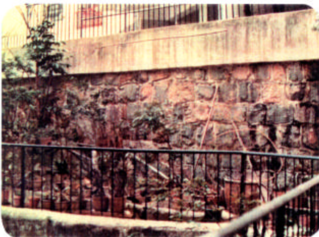
Plate D5 - Pointed Squared Rubble Wall (11SW-A/R295)
