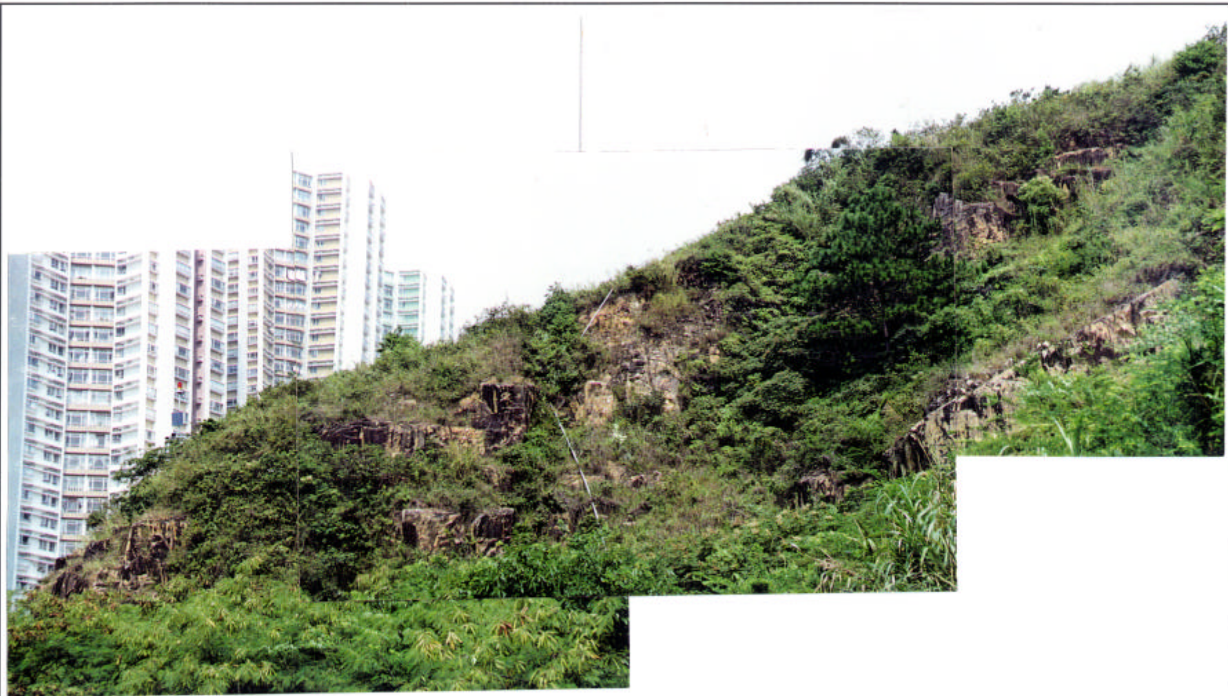
Plate 2 - North Flank of Large Ancient Landslide Scar (833335E 811350N) Along the Former Coastline, North of Slope 15NW-A/C3, Showing the Relationship of the Soil Profile to Joints (Subvertical, Subhorizontal and Inclined Parallel to the Natural Slope); the Inclined Planar Discontinuity (Lower Right) is at or near to the Basal Surface of Rupture of the Landslide. (Taken 3/10/96)
