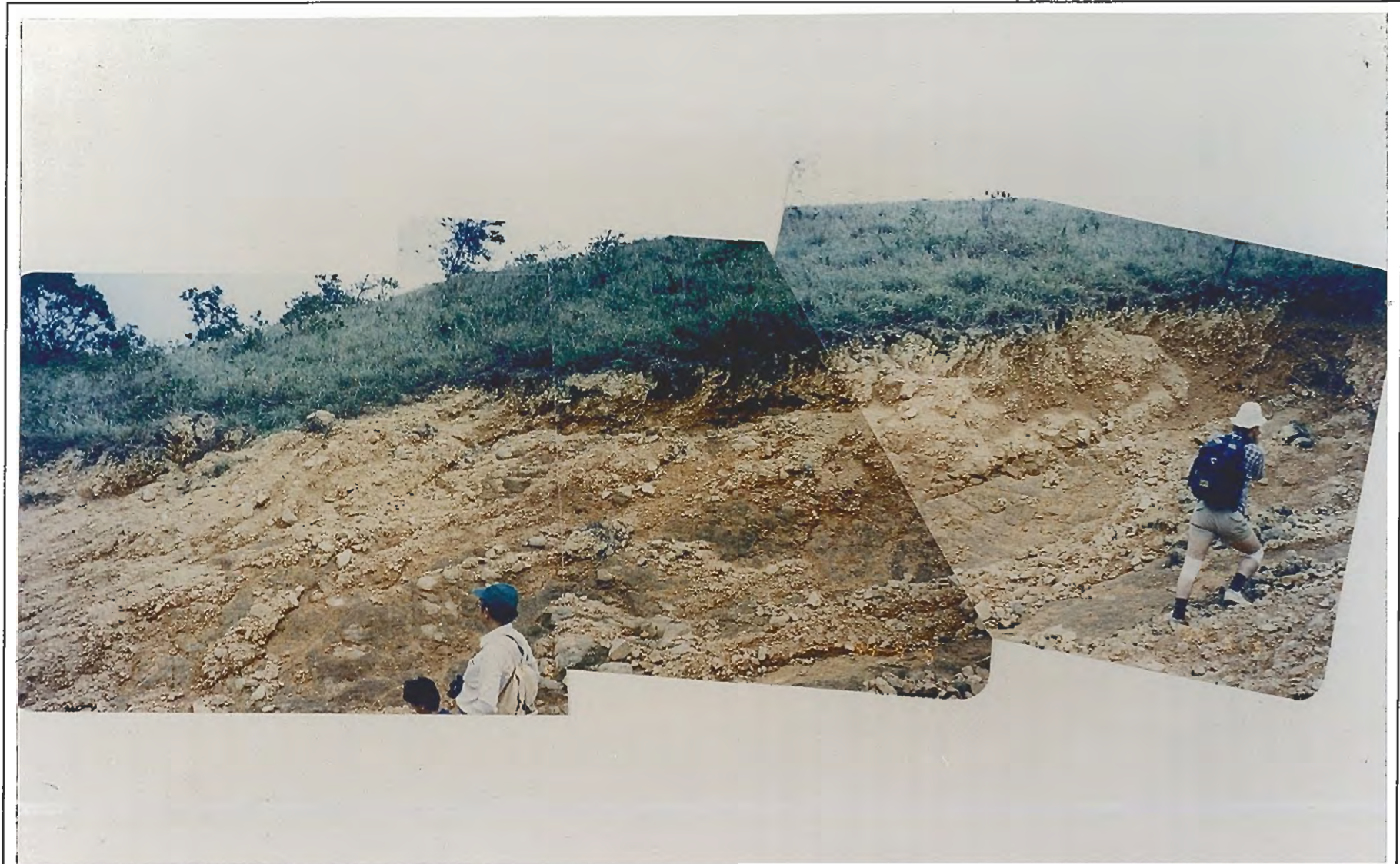
Plate C3 - Main Scarp of Landslide C1
