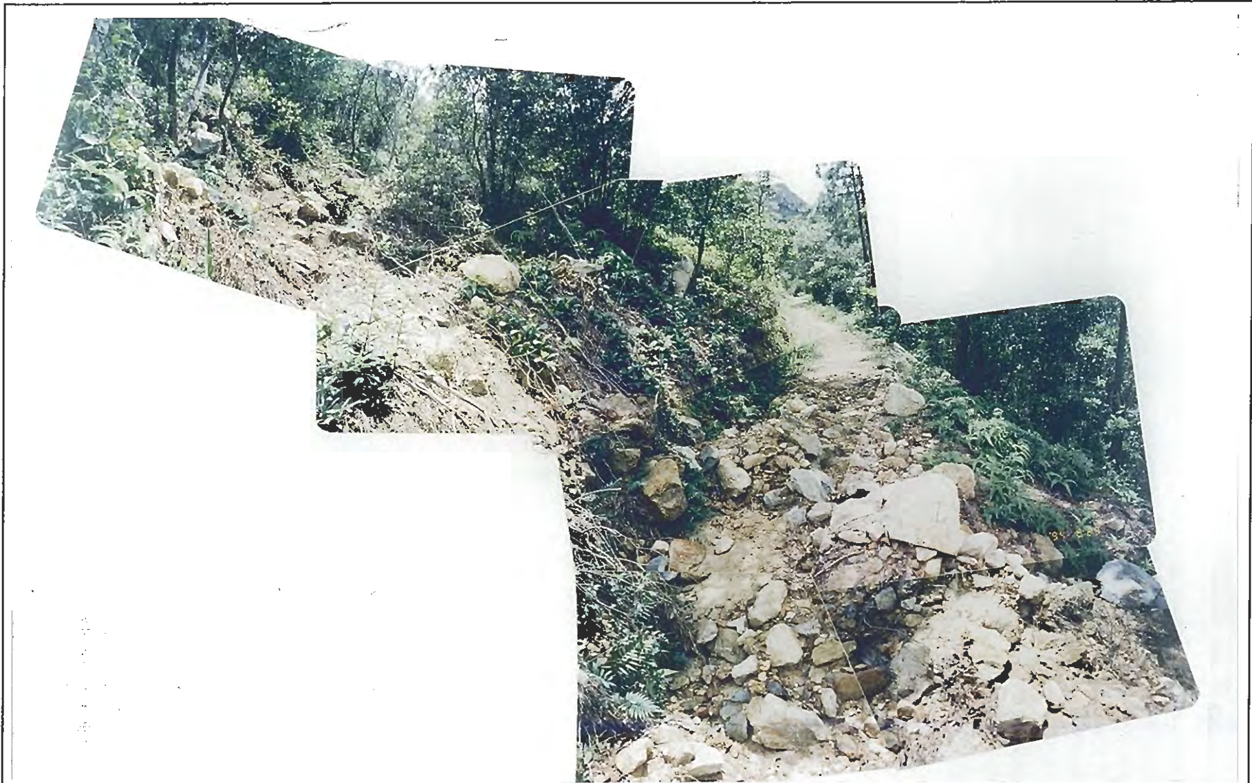
Plate B9.9 - Debris Trail at Footpath Level
