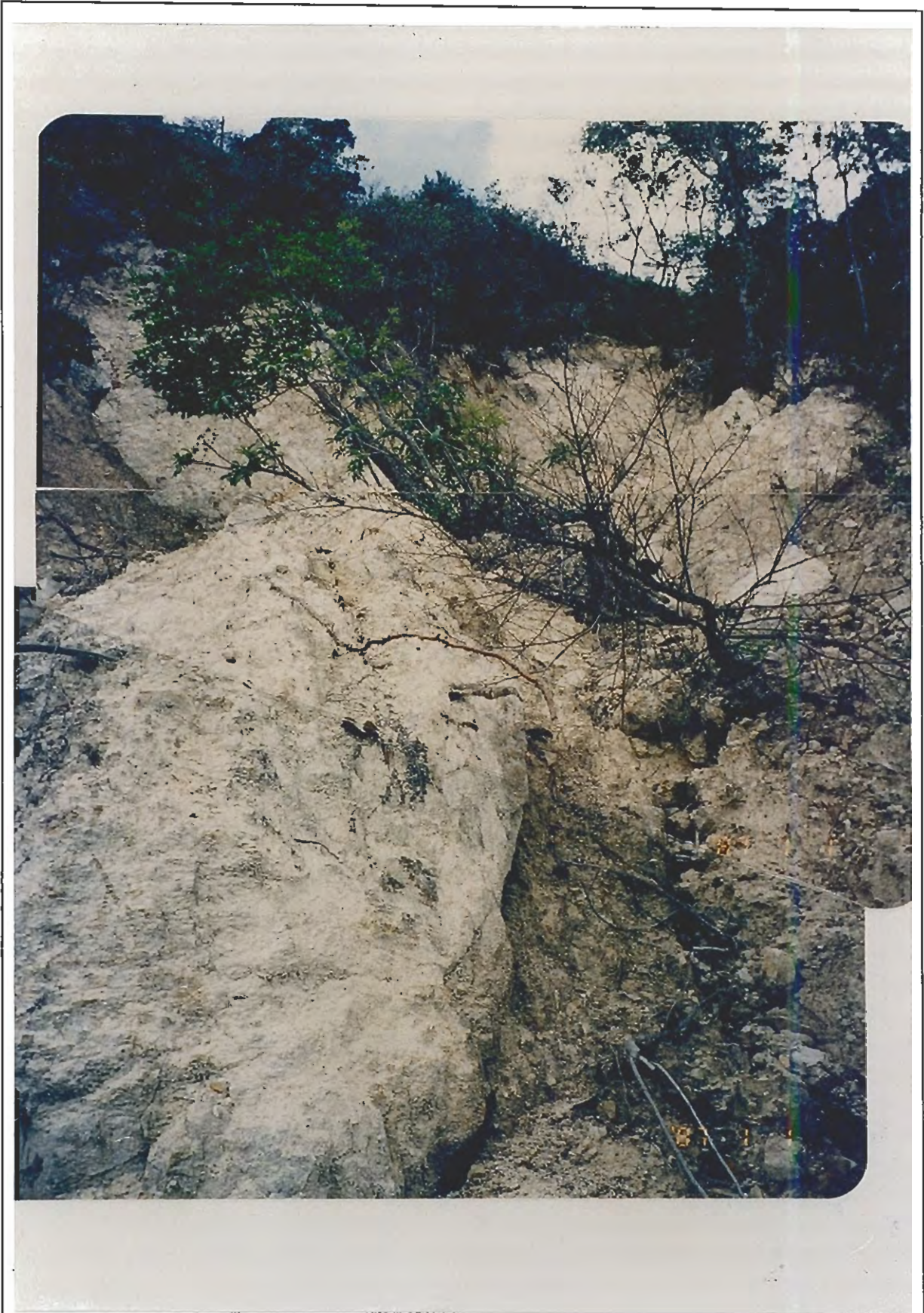
Plate B13.4 - Uphill View of Debris Trail of Landslide B13
