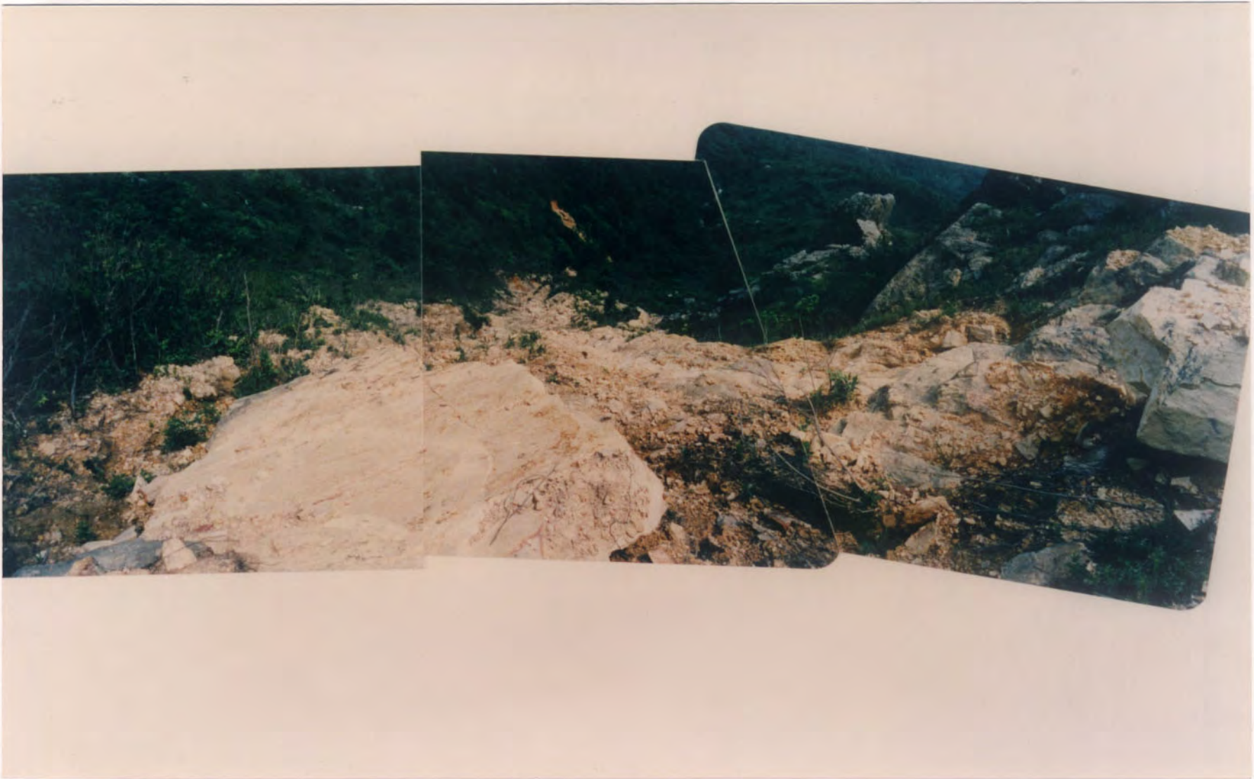
Plate B4.8 - Downhill View from Main Scarp B4E
