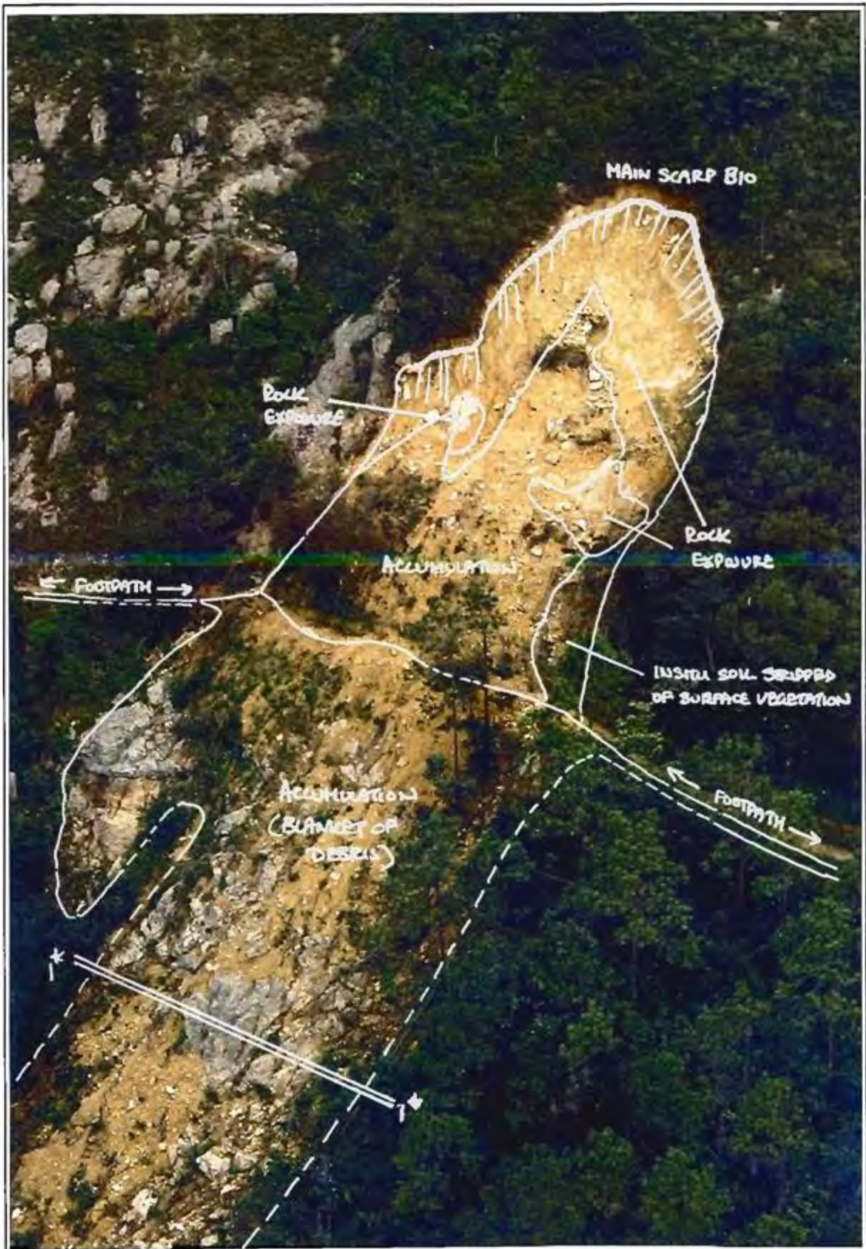
Plate B10.3 - Oblique View of Landslide B10
