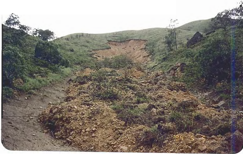
Plate C6 - Uphill View of Debris Trail
