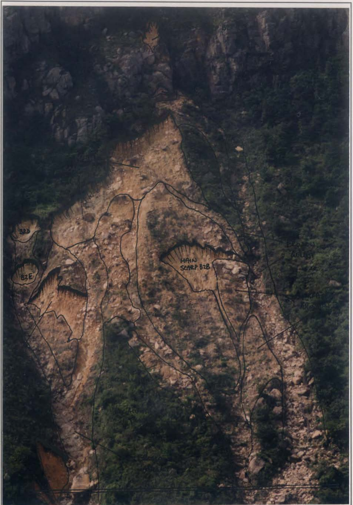
Plate B2.3 - Oblique View of Main Scarps of Landslide B2
