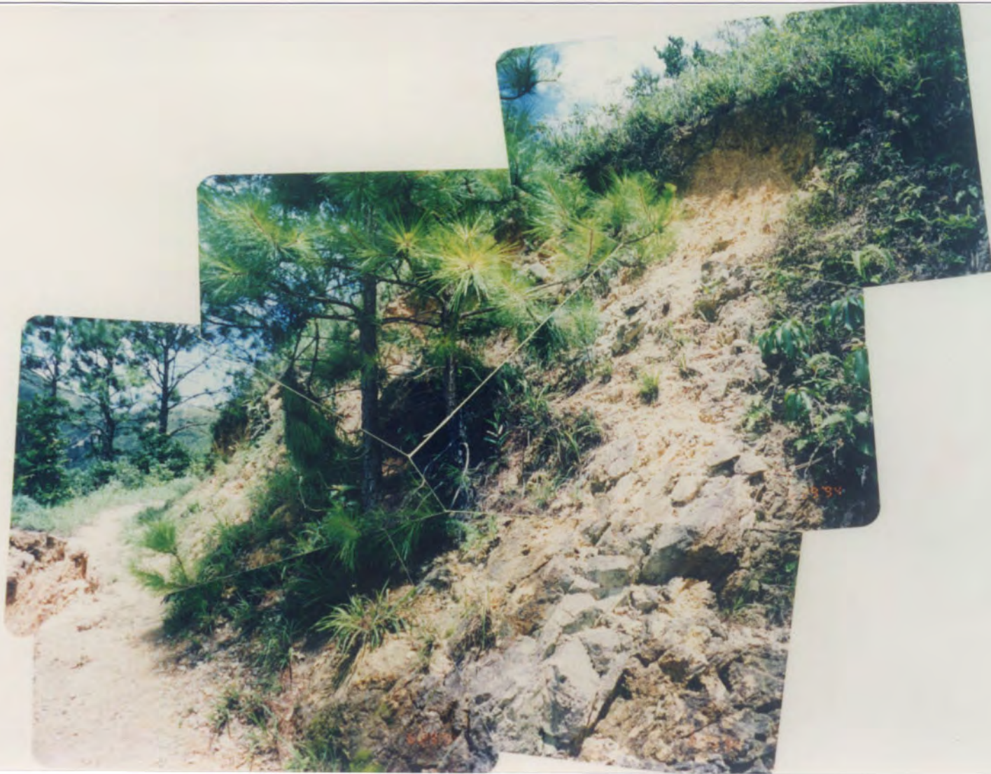
Plate B6.9 - Minor Landslide at Footpath above Landslide B6
