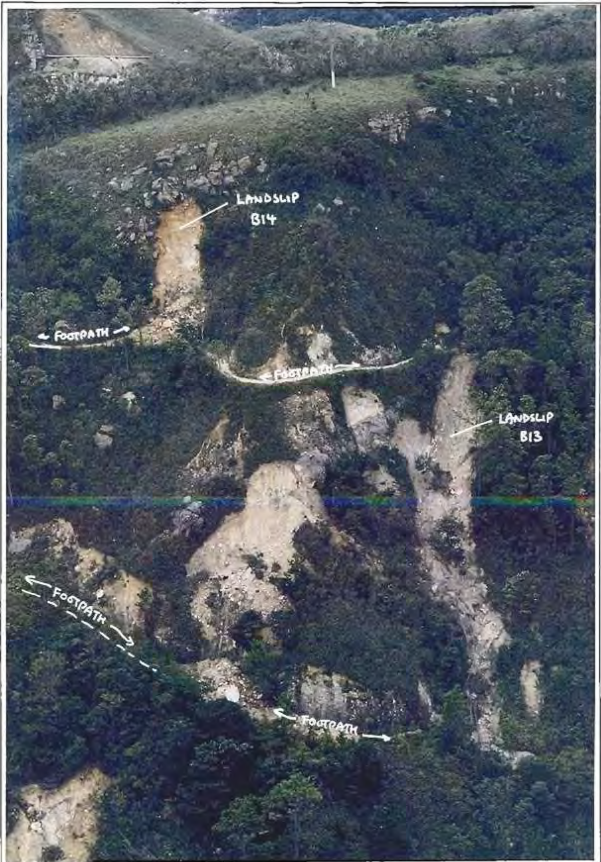
Plate B13.1 - Oblique View of Landslides B13 & B14
