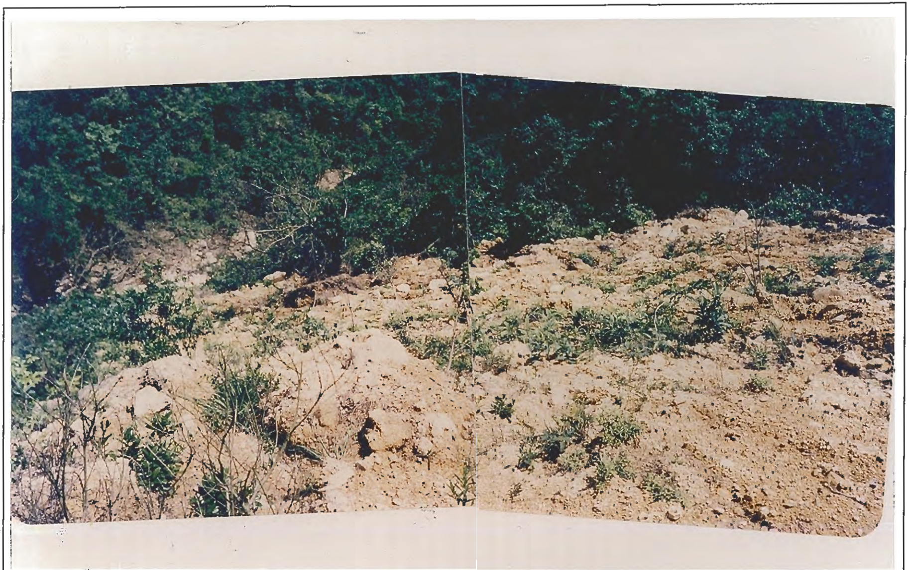
Plate B8.7 - Downhill View of Debris Trail from Scarp B8
