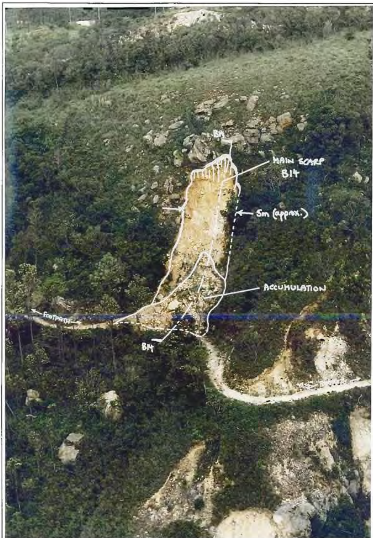
Plate B14.1 - Oblique View of Landslide B14
