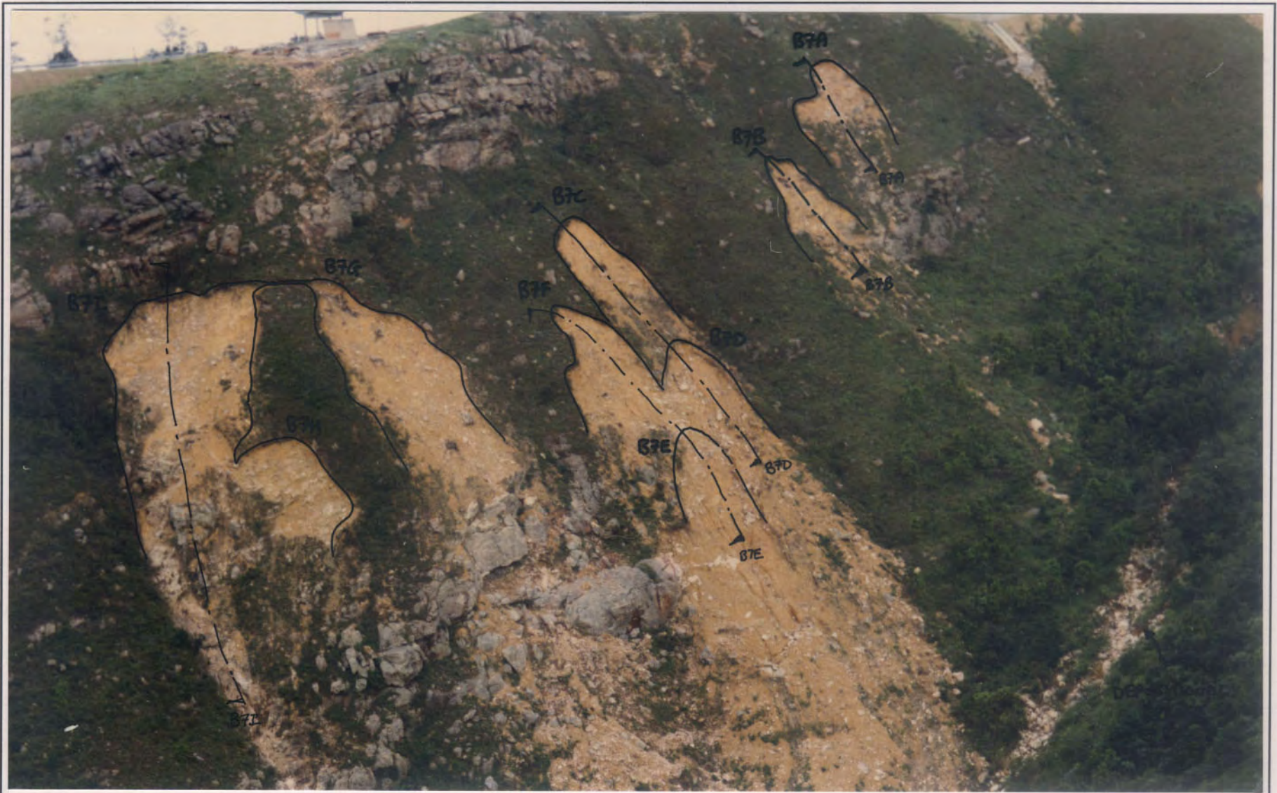
Plate B7.2 - Oblique View of Landslide Group B7
