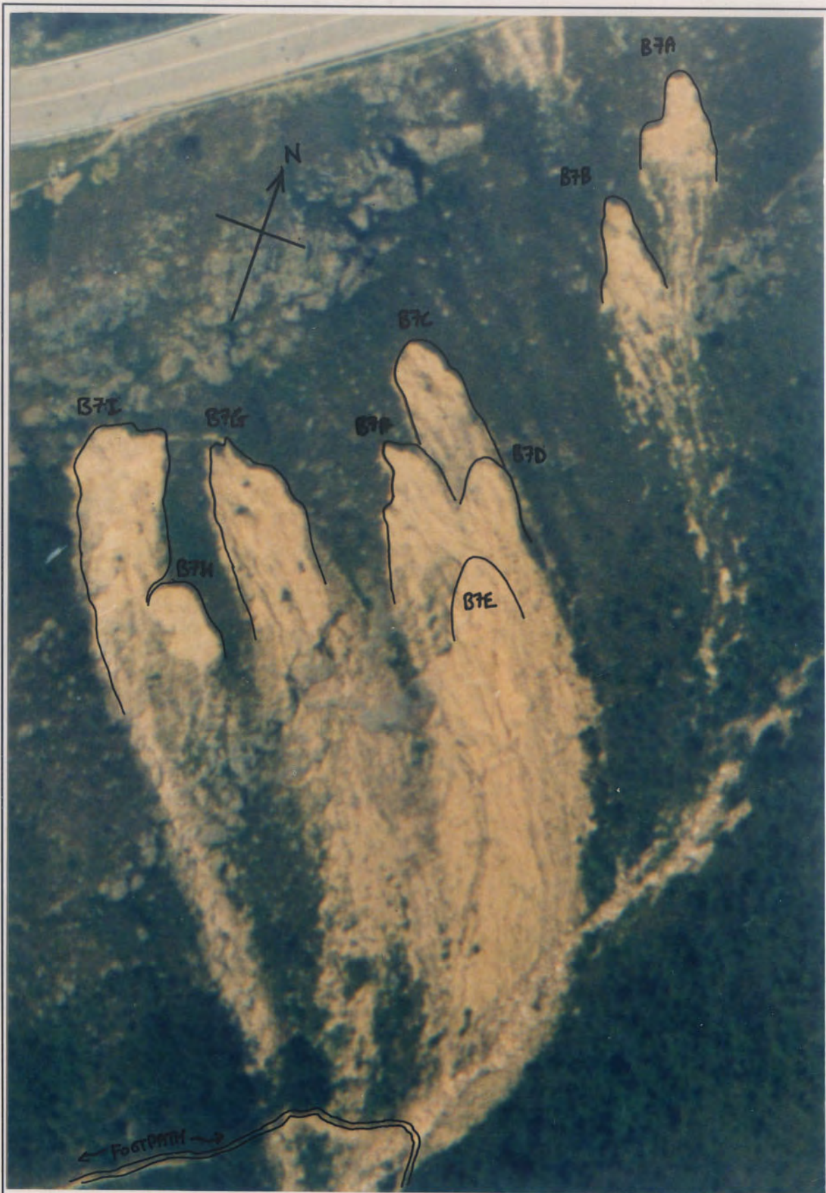
Plate B7.1 - Aerial View of Landslide Group B7
