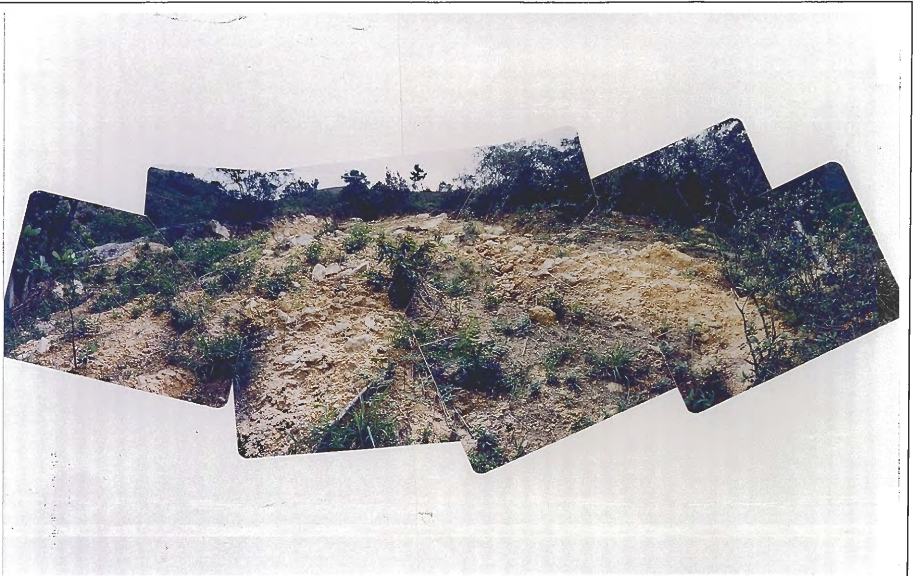
Plate B10.7 - Main Scarp of Landslide B10
