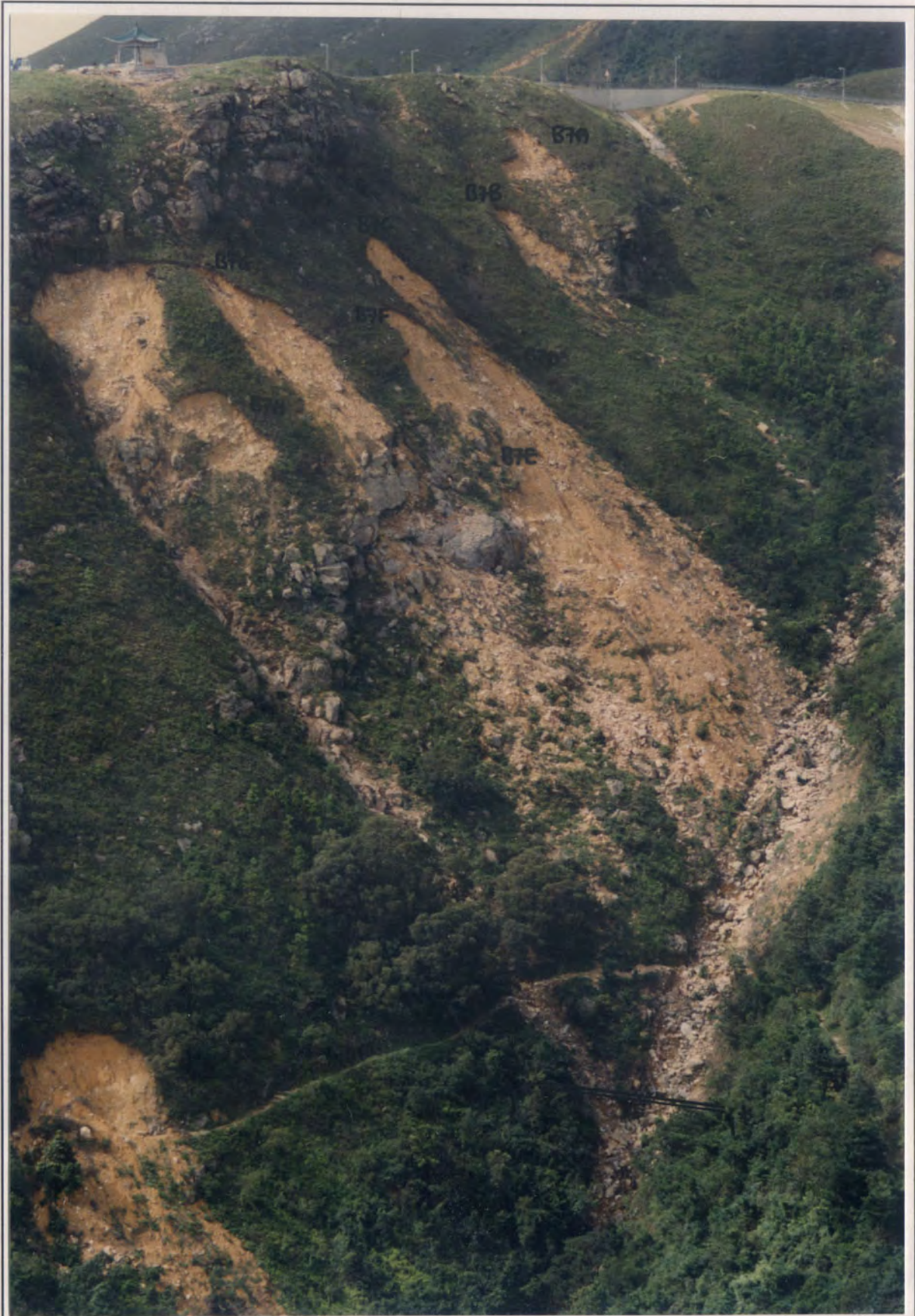
Plate B7.4 - Oblique View of Landslide Group B7
