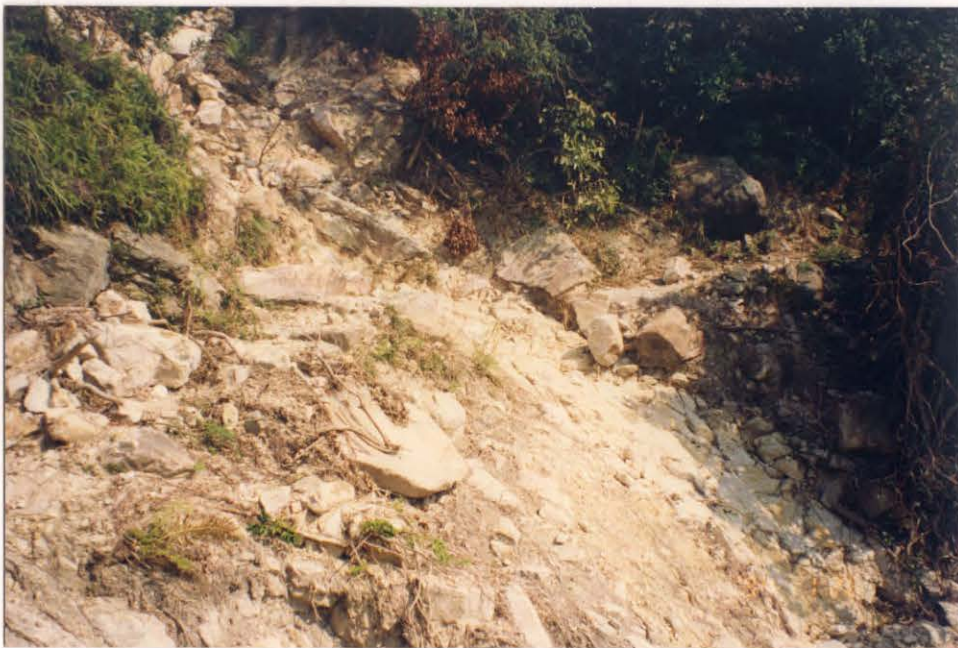
Plate B2.24 - Debris Trail of Landslide B2 at Footpath Level
