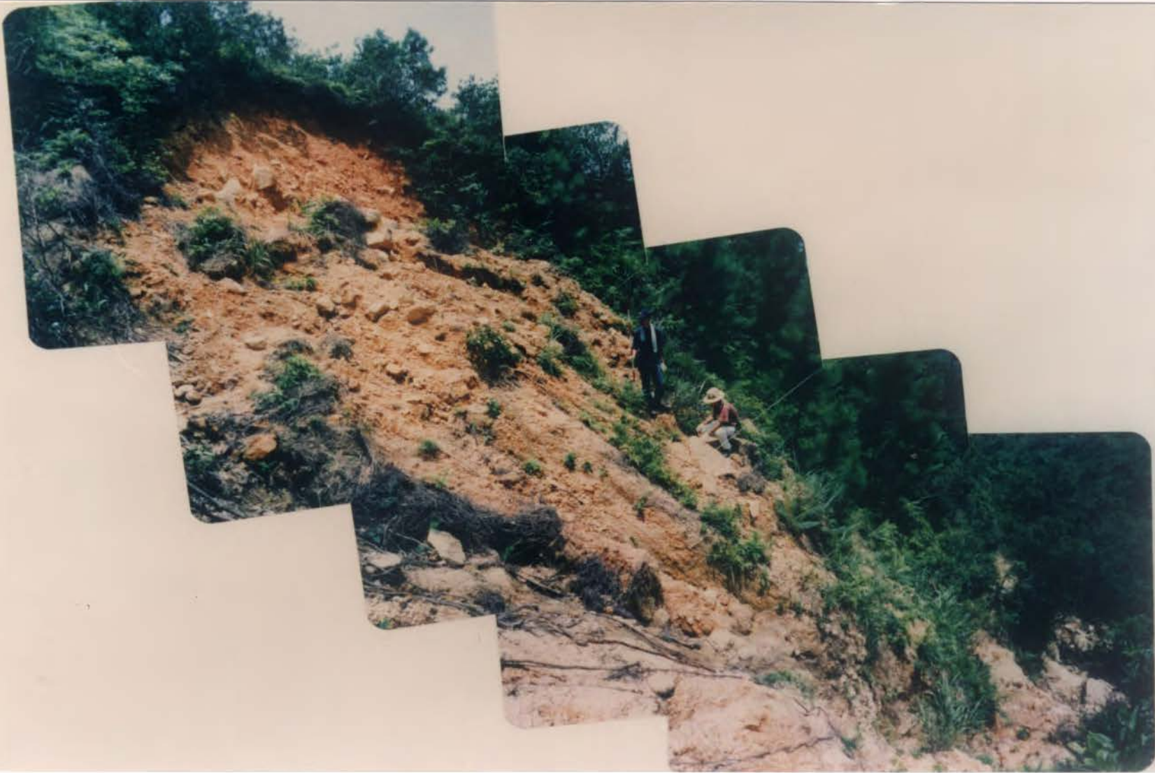
Plate B3.4 - Side View of Main Scarp B3A
