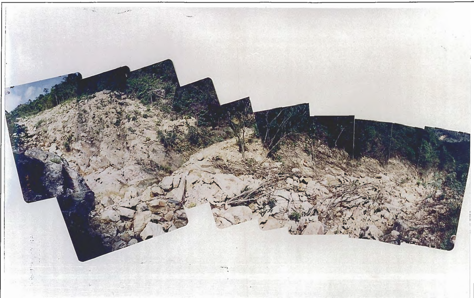
Plate B7.9 - View of Debris Trail of Landslide B7 from Footpath
