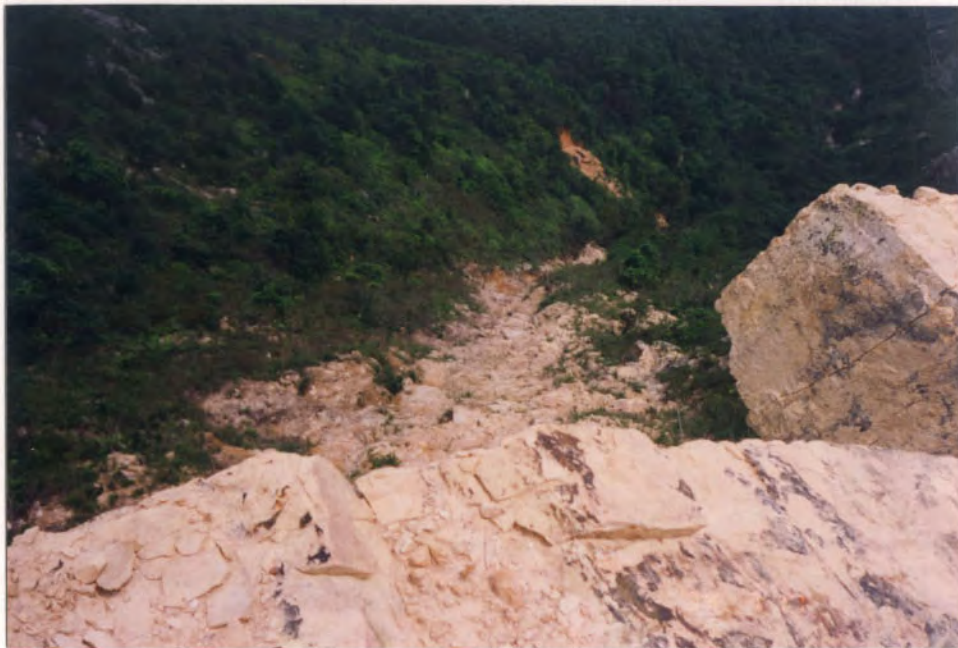
Plate B4.10 - Debris Trail View from Main Scarp B4E
