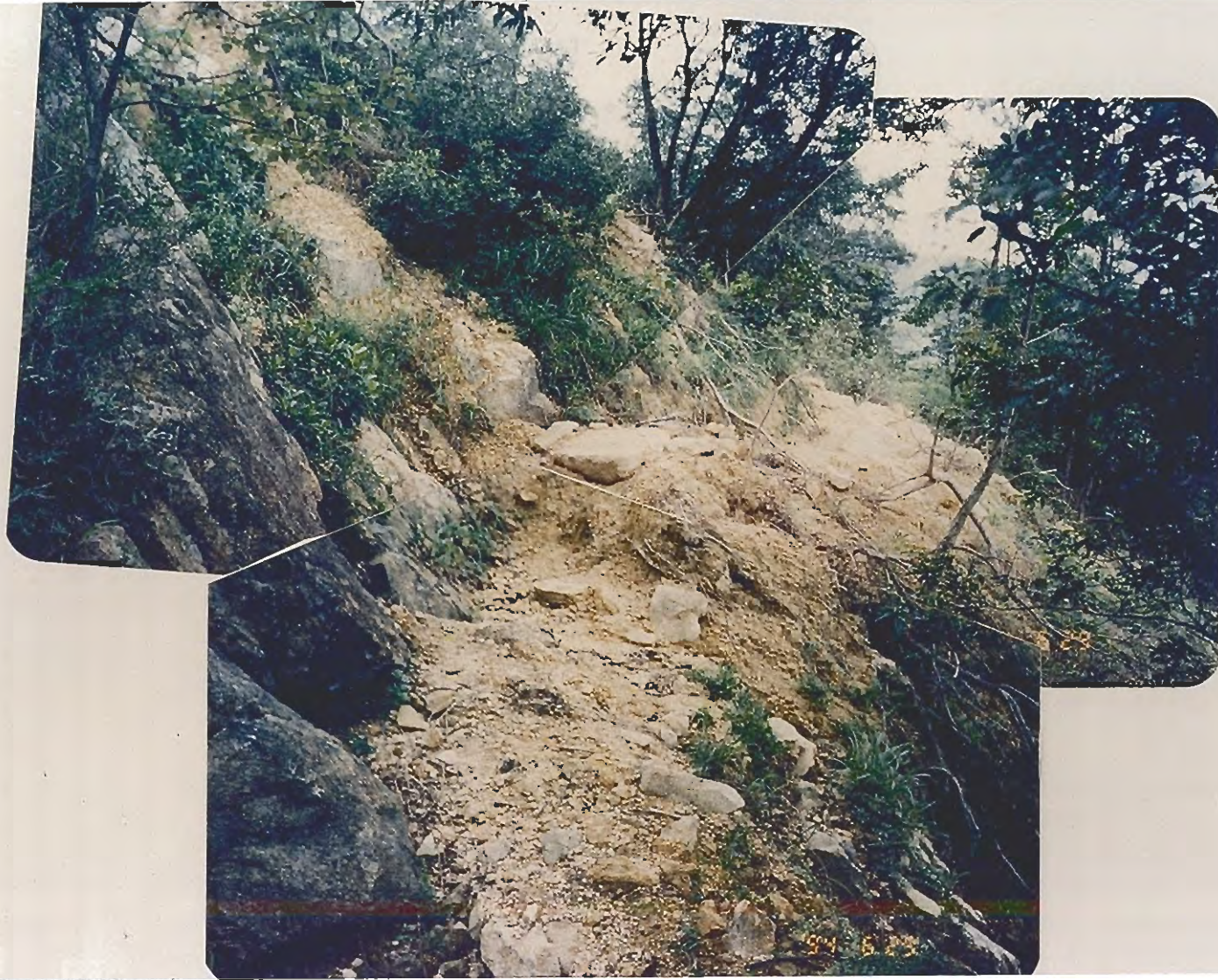
Plate B10.5 - Debris at Footpath
