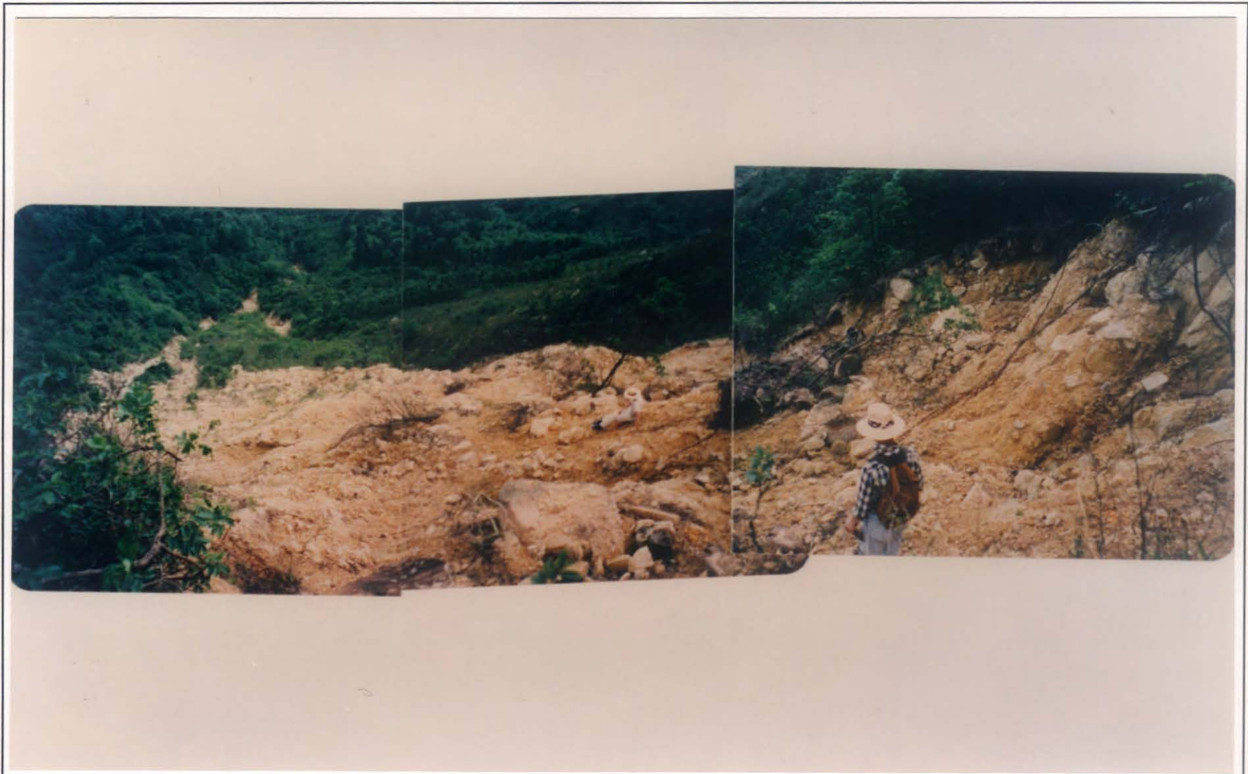
Plate B2.14 - Downhill View of Debris Trail from Main Scarp B2A
