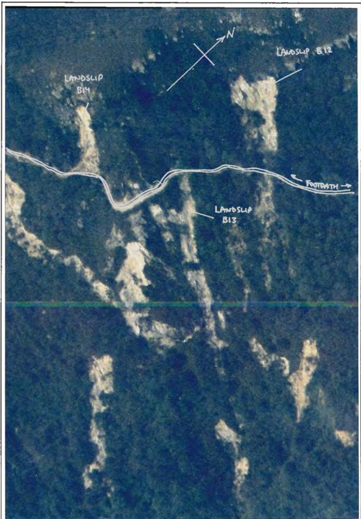
Plate B12.1 - Aerial View of Landslides B12, B13 & B14
