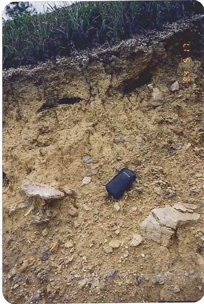
Plate B9.6 - Close-up of Main Scarp B9
