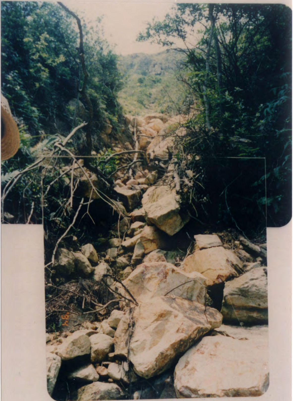
Plate B4.15 - Debris Trail of Landslide B4 Viewed from Footpath Level
