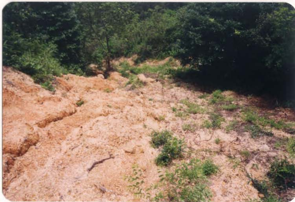
Plate B3.11 - Downhill View of Debris Trail from Main Scarp B3B
