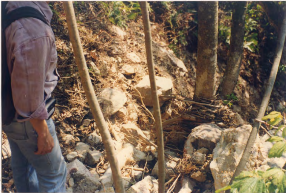
Plate B5.15 - Bouldery Deposit on Footpath and Signs of Surface Water Flow along Debris Trail of Landslide B5
