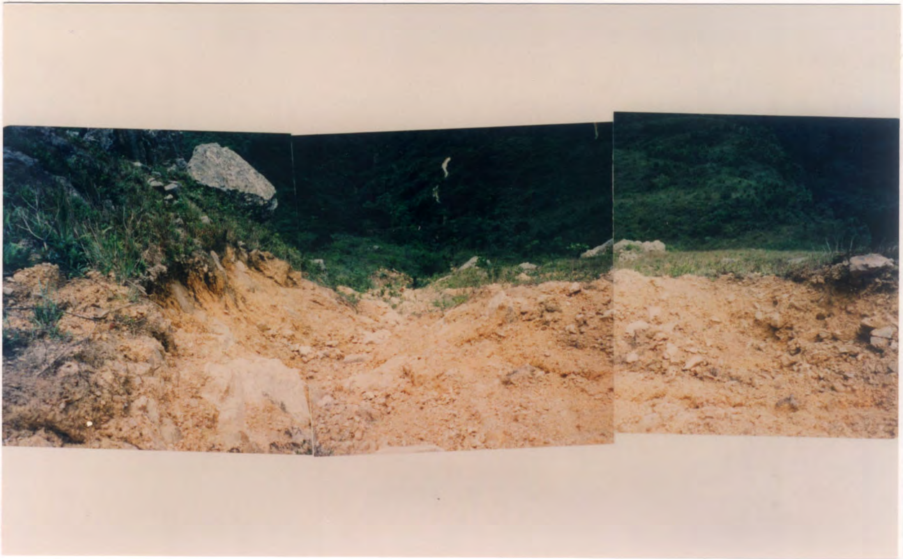
Plate B5.8 - Downhill View from Main Scarp B5A
