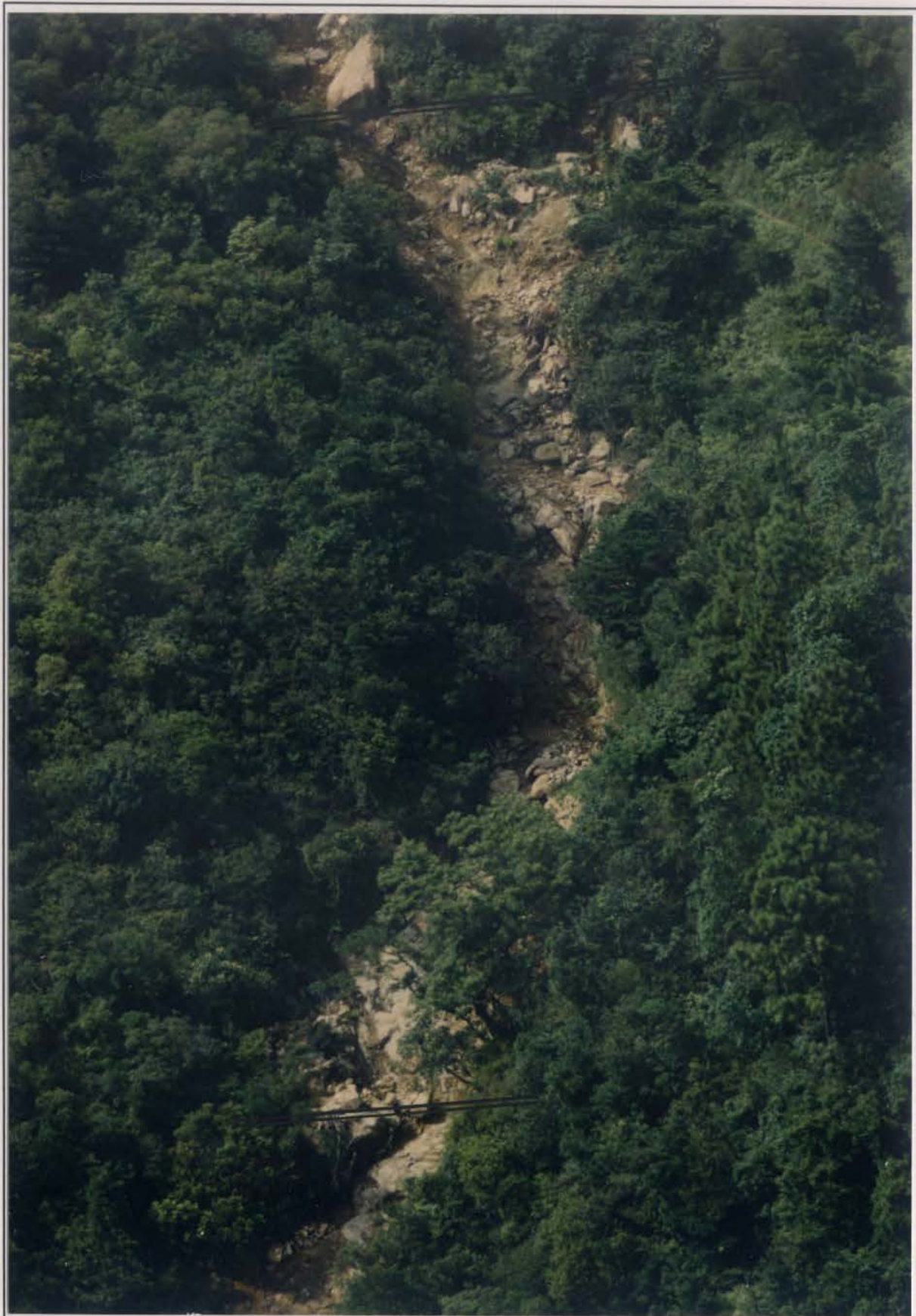
Plate B2.6 - Debris Trail (CH230 - CH260) of Landslide B2
