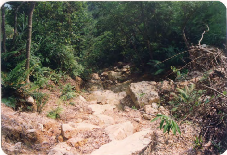
Plate B4.14 - Downhill View of Debris Trail of Landslide B4
