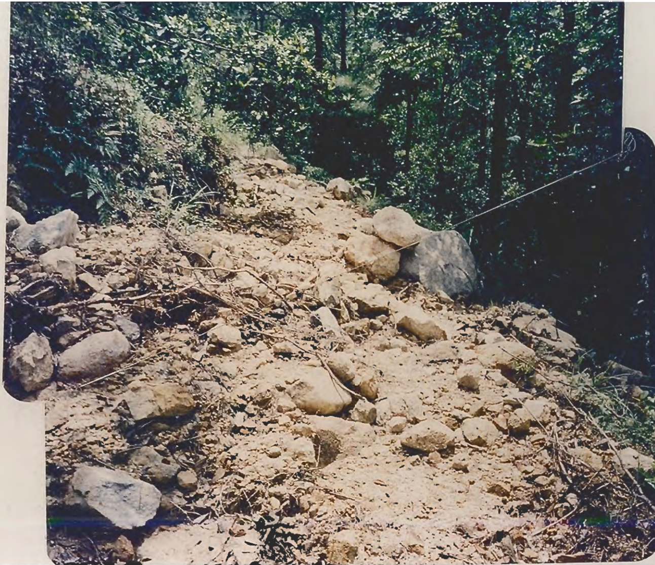
Plate B9.7 - Debris Trail of Landslide B9 Viewed from Footpath
