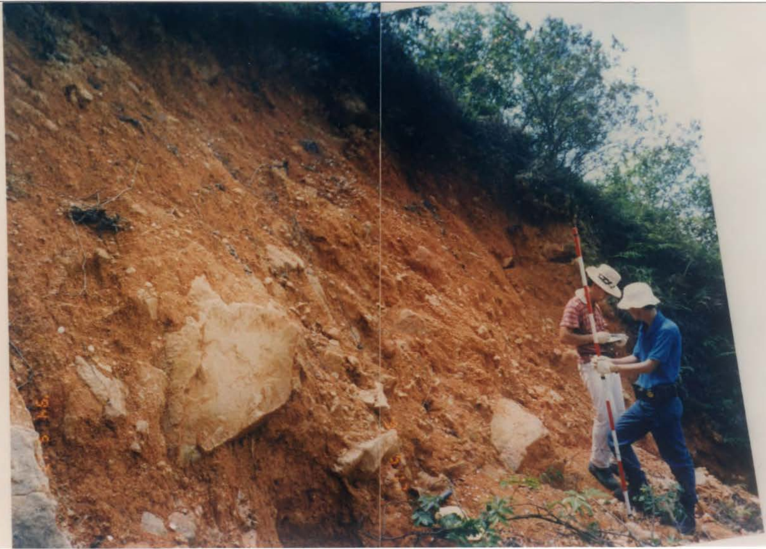
Plate B3.6 - Close-up of Main Scarp B3A
