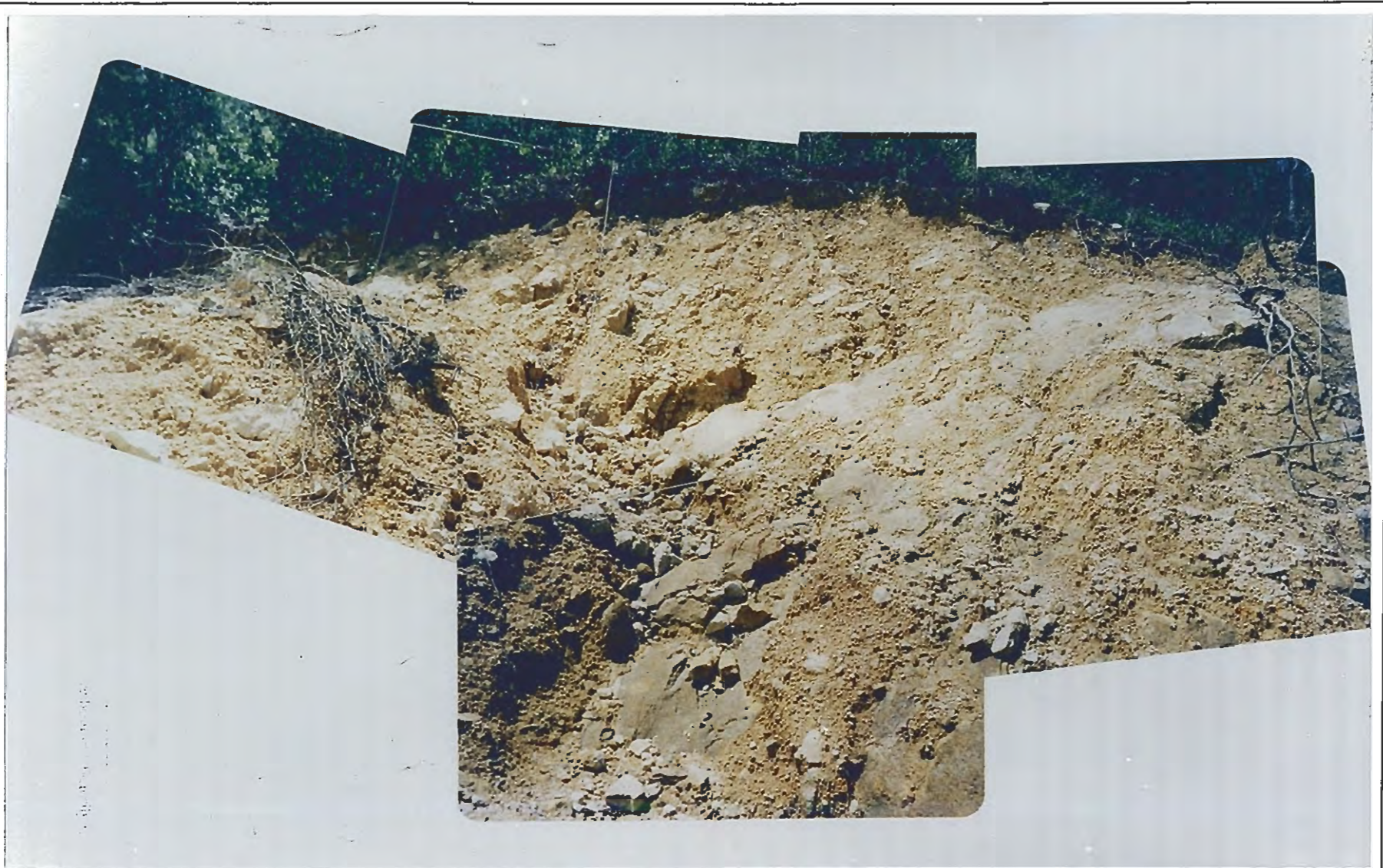
Plate B8.5 - Close-up of Main Scarp B8
