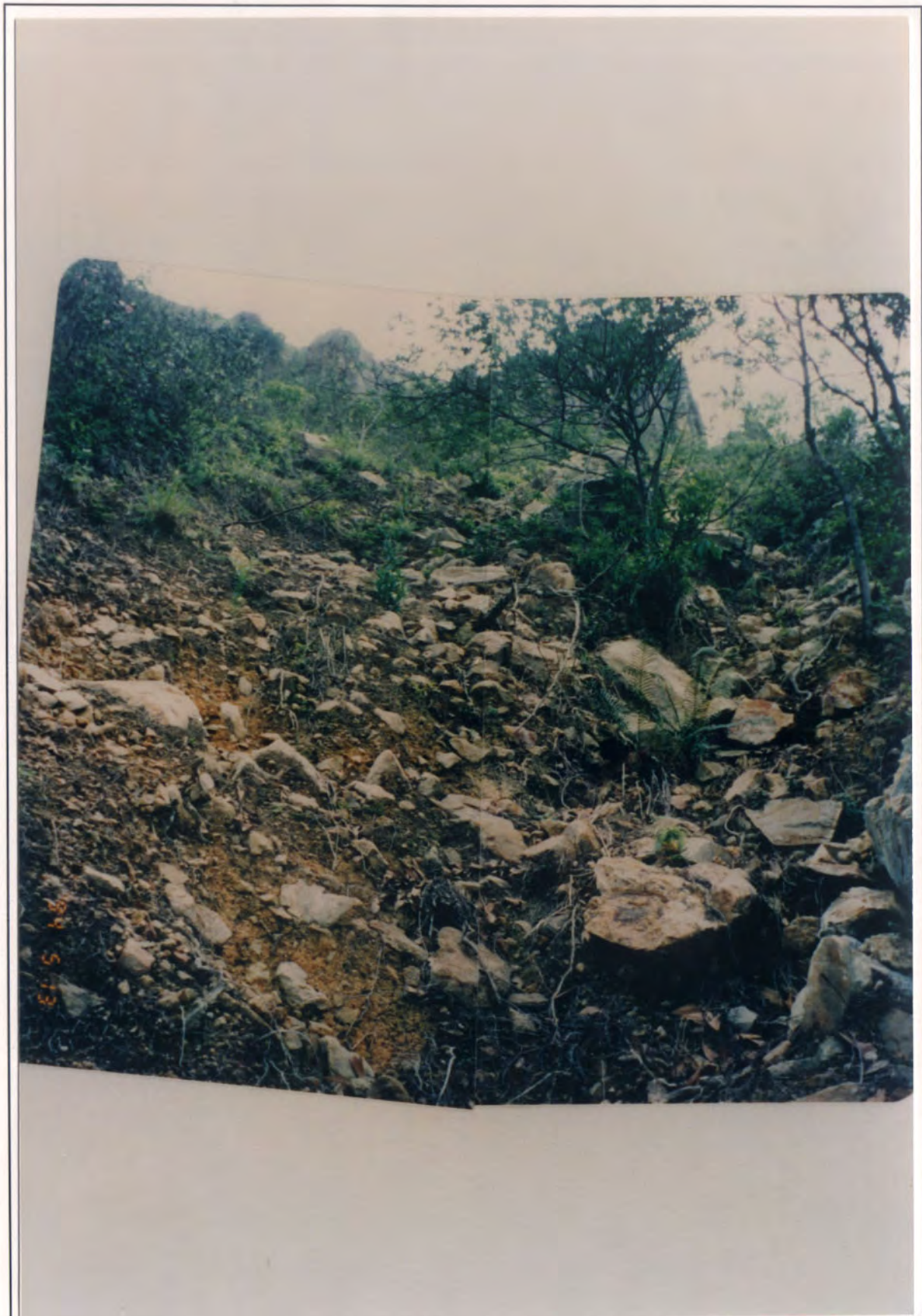
Plate B5.4 - Uphill View of Debris Trail of Landslide B5
