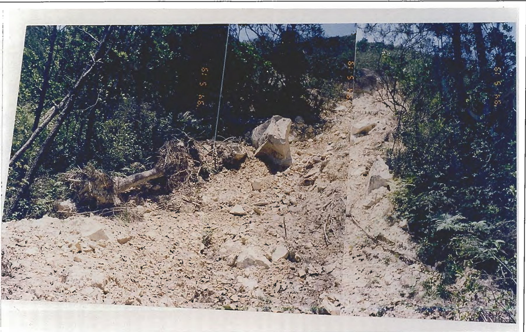
Plate B12.6 - Uphill View of Debris Trail of Landslide B12
