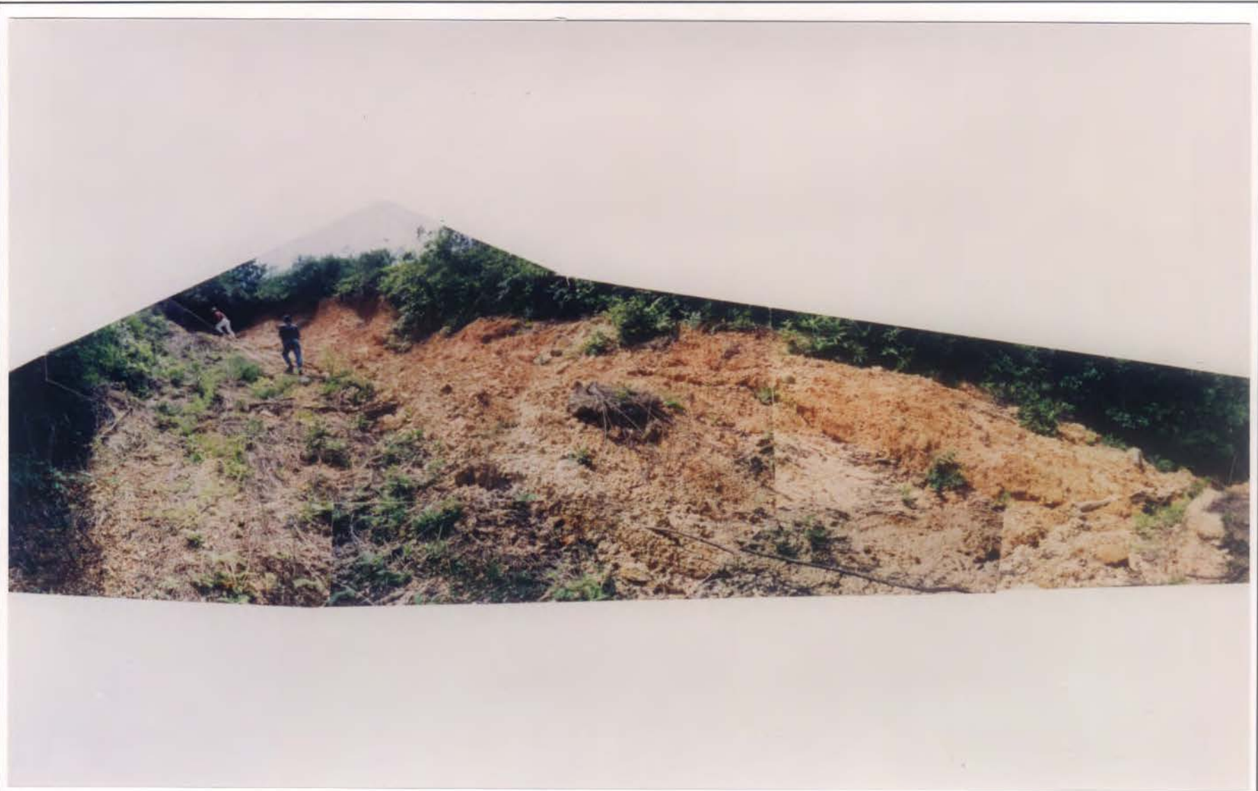
Plate B3.12 - Uphill View toward Main Scarp B3D
