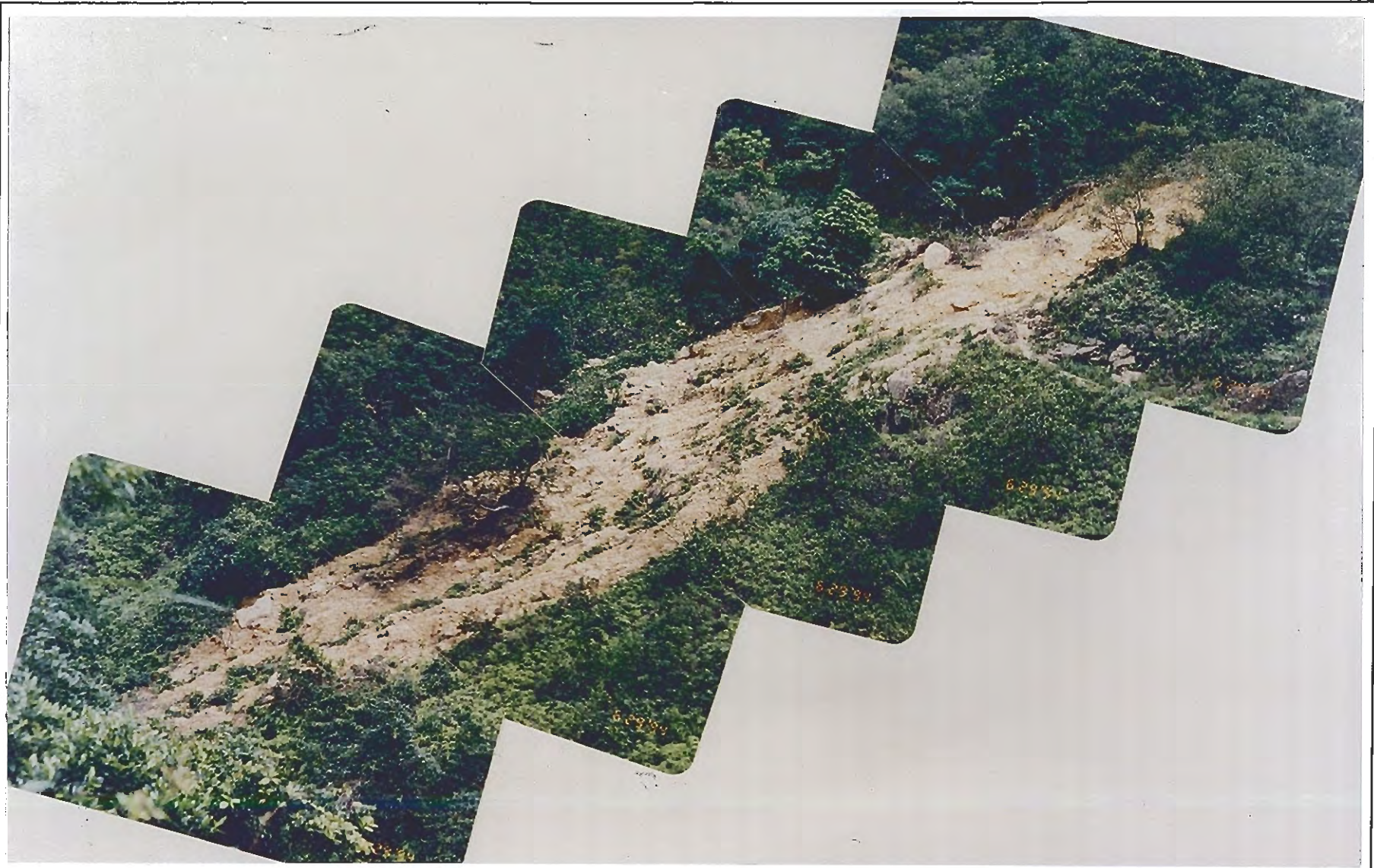
Plate B8.3 - View of Landslide B8
