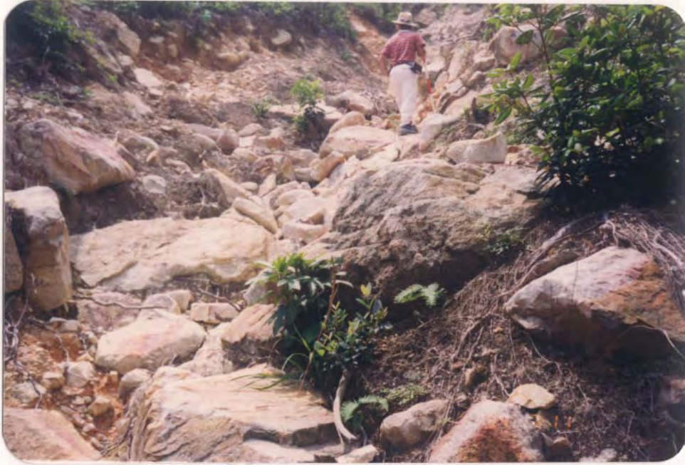
Plate B4.13 - Uphill View of Debris Trail of Landslide B4
