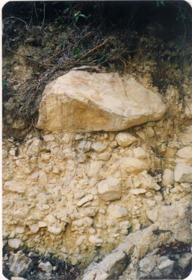
Plate B2.22 - Older Colluvium Exposed along Debris Trail of Landslide B2
