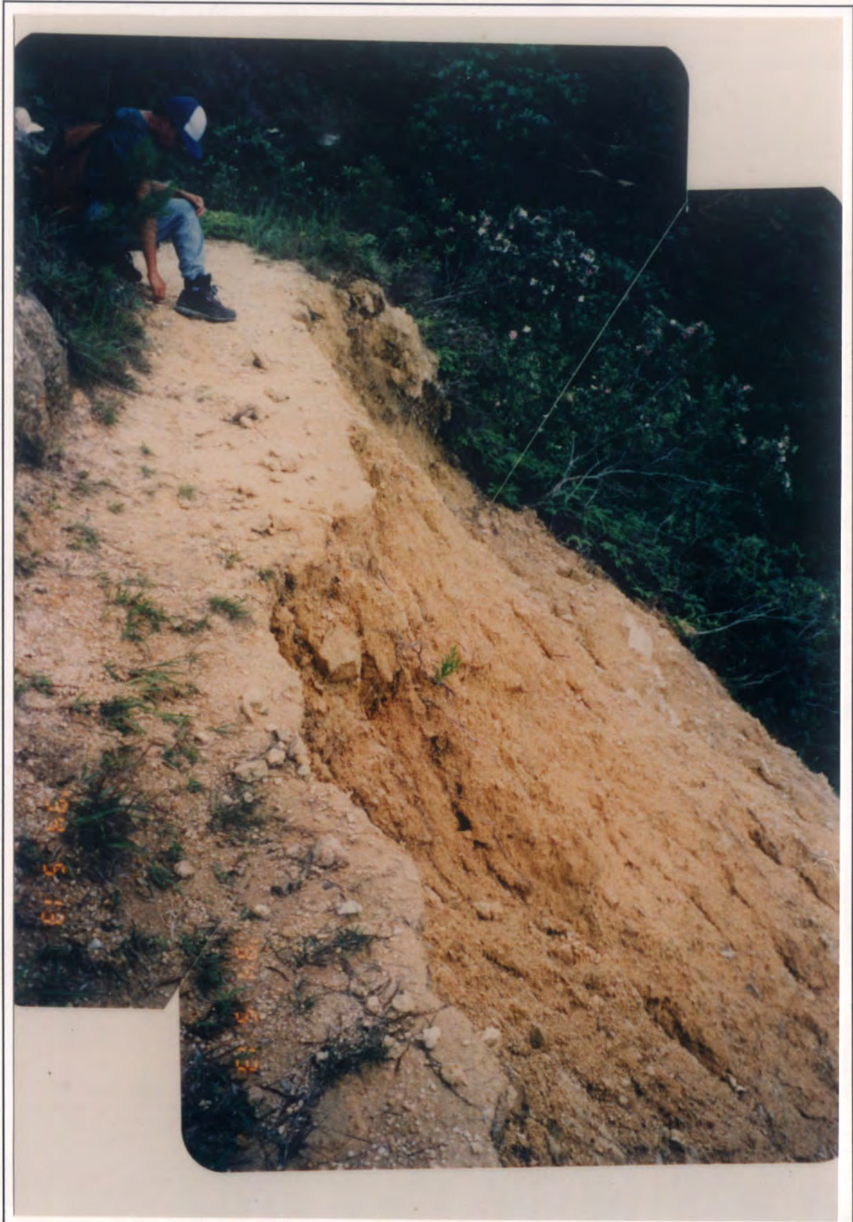
Plate B6.4 - Crown of Landslide B6 as Seen from Footpath
