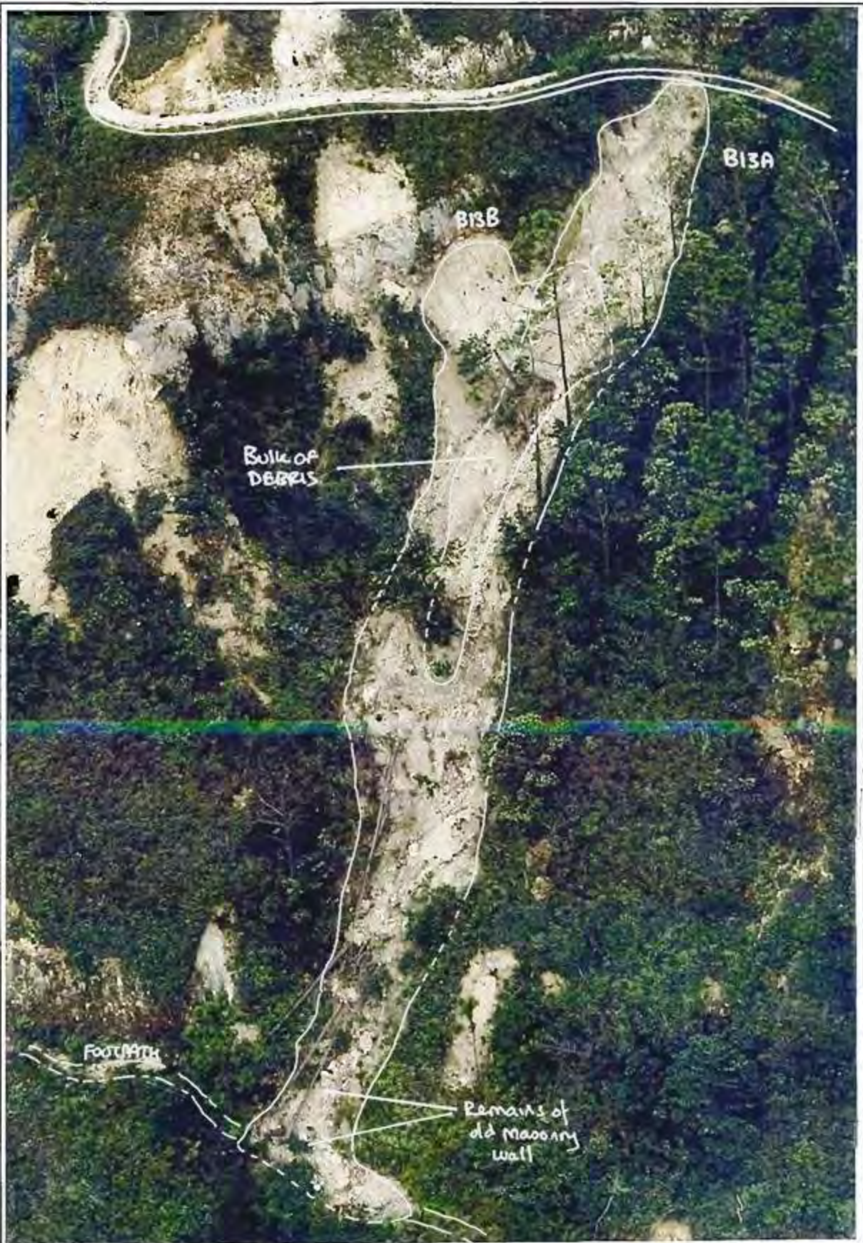
Plate B13.2 - Oblique View of Landslide B13
