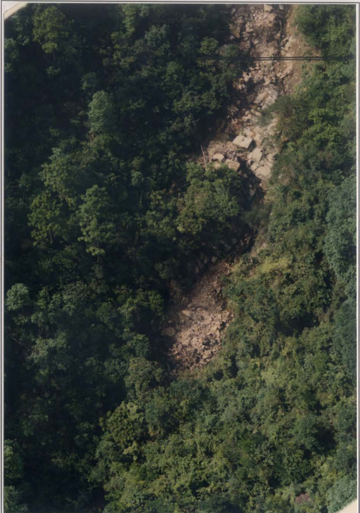
Plate B1.12 - Oblique View of Debris Trail (Approximate CH280+) of Landslide B1
