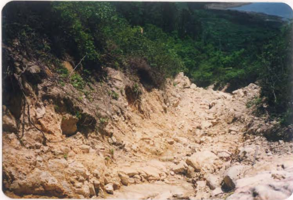
Plate B2.29 - Downhill View of Erosion Gully along Debris Trail of Landslide B2
