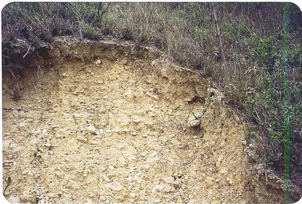
Plate B13.7 - Minor Landslide adjacent to Footpath above Landslide B13
