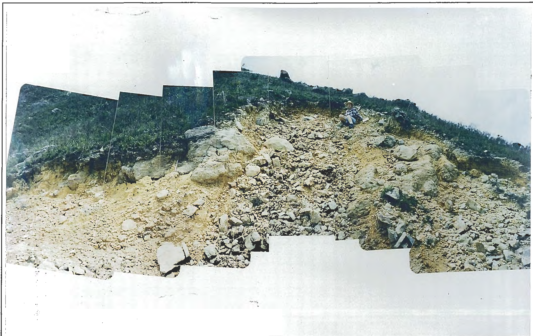
Plate B7.5 - Close-up of Main Scarp B7A
