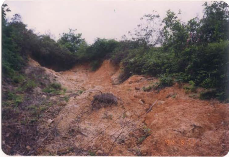
Plate B3.13 - Uphill View of Debris Trail of Landslide B3D
