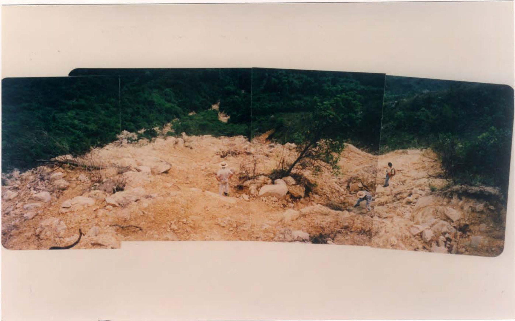
Plate B2.25 - Downhill View of Debris Trail from Main Scarp B2A
