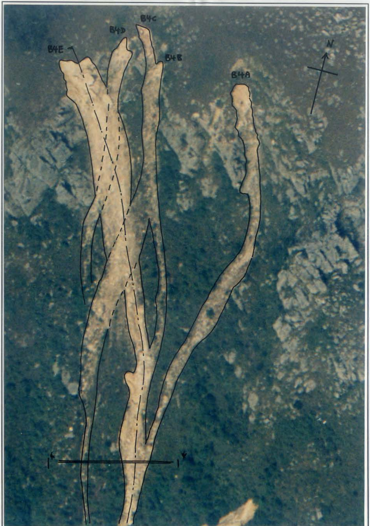
Plate B4.3 - Aerial View of Landslide Group B4
