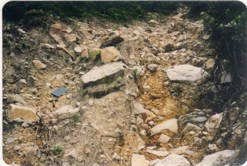
Plate B2.21 - Older Colluvium Exposed along Debris Trail of Landslide B2
