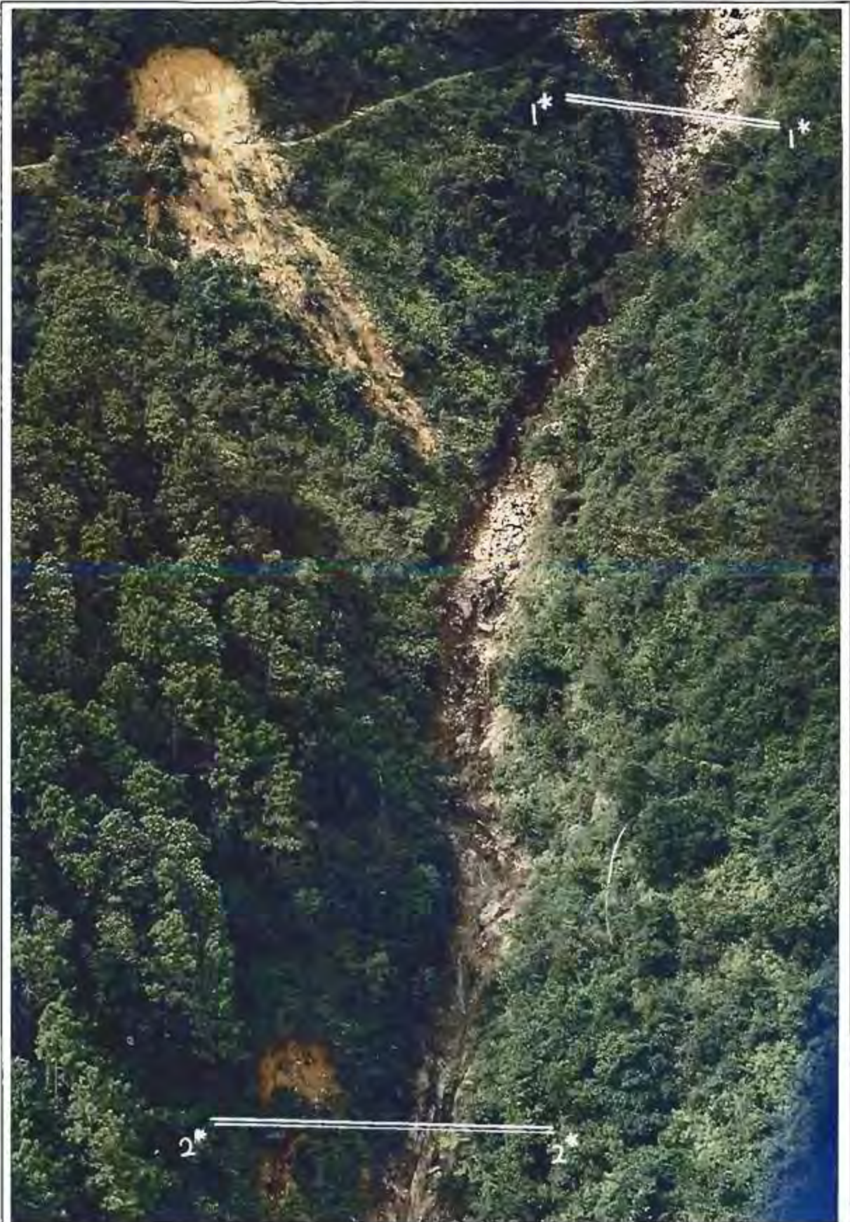
Plate B7.19 - Debris Trail (CH130 - CH210 Approximate) of Landslide B7
