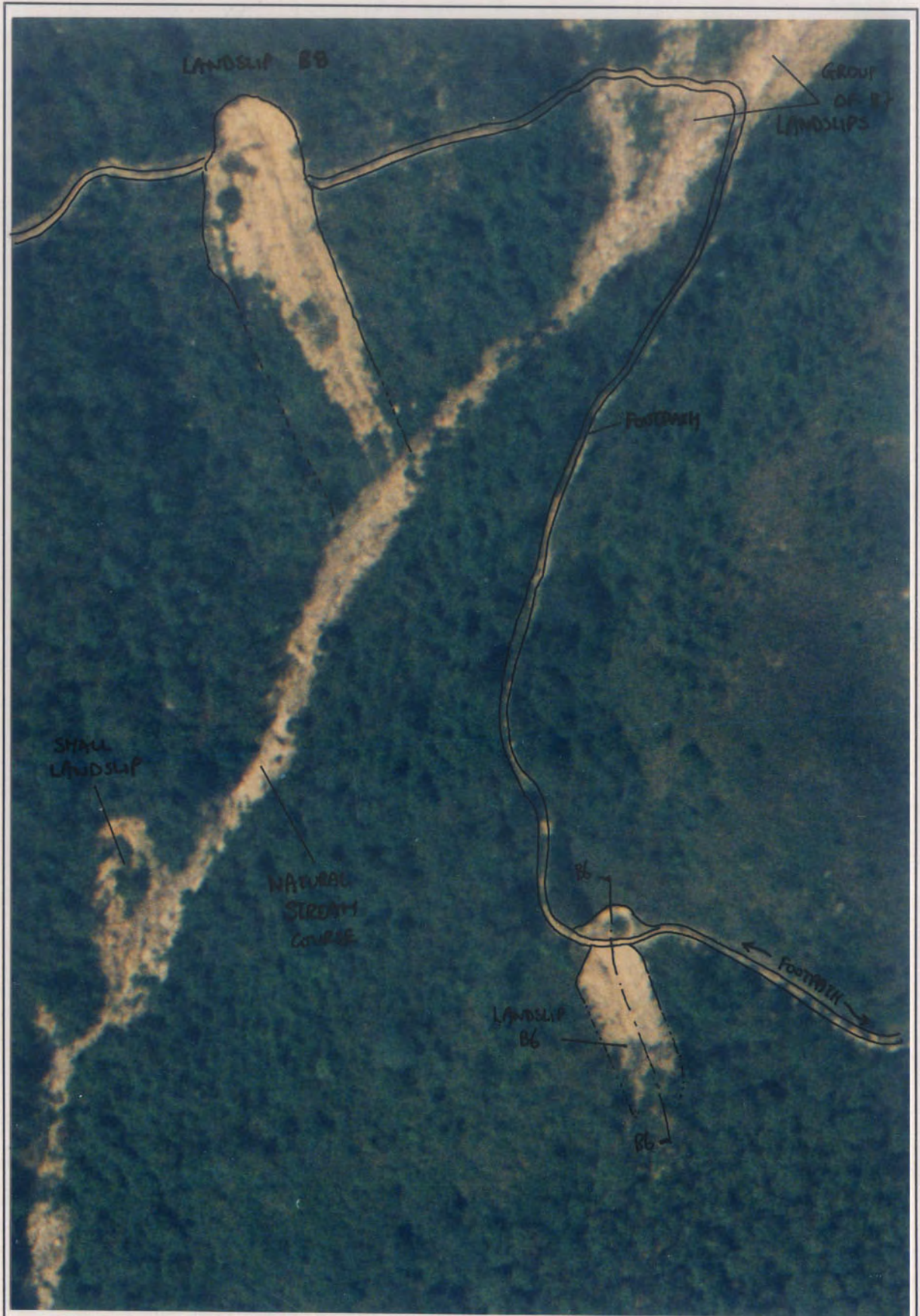
Plate B6.1 - Aerial View of Landslide Groups B6 and B8
