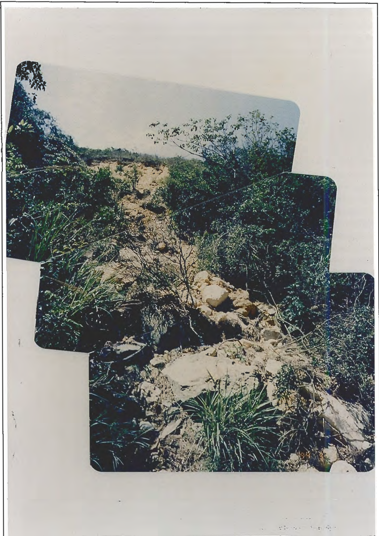
Plate B11.6 - Uphill View of Debris Trail of Landslide B11
