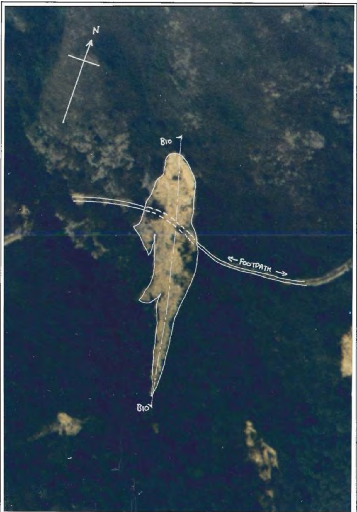
Plate B10.1 - Aerial View of Landslide B10
