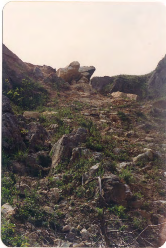
Plate B4.11 - Uphill View toward Main Scarp B4E
