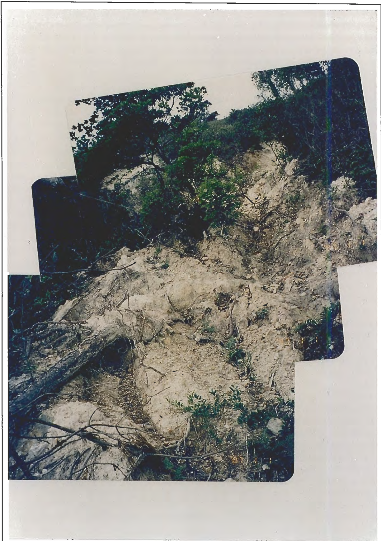
Plate B13.5 - Uphill View of Debris Trail of Landslide B13
