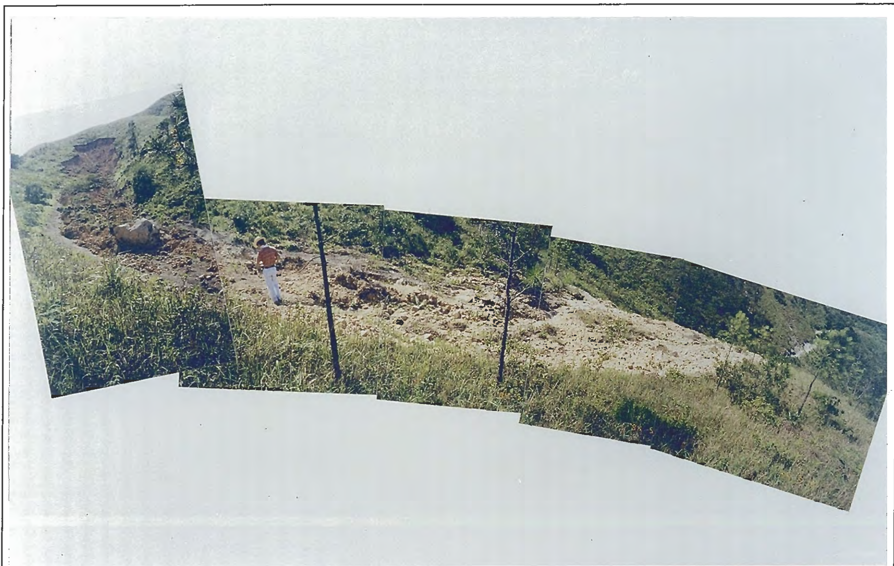
Plate C11 - View of Debris Trail
