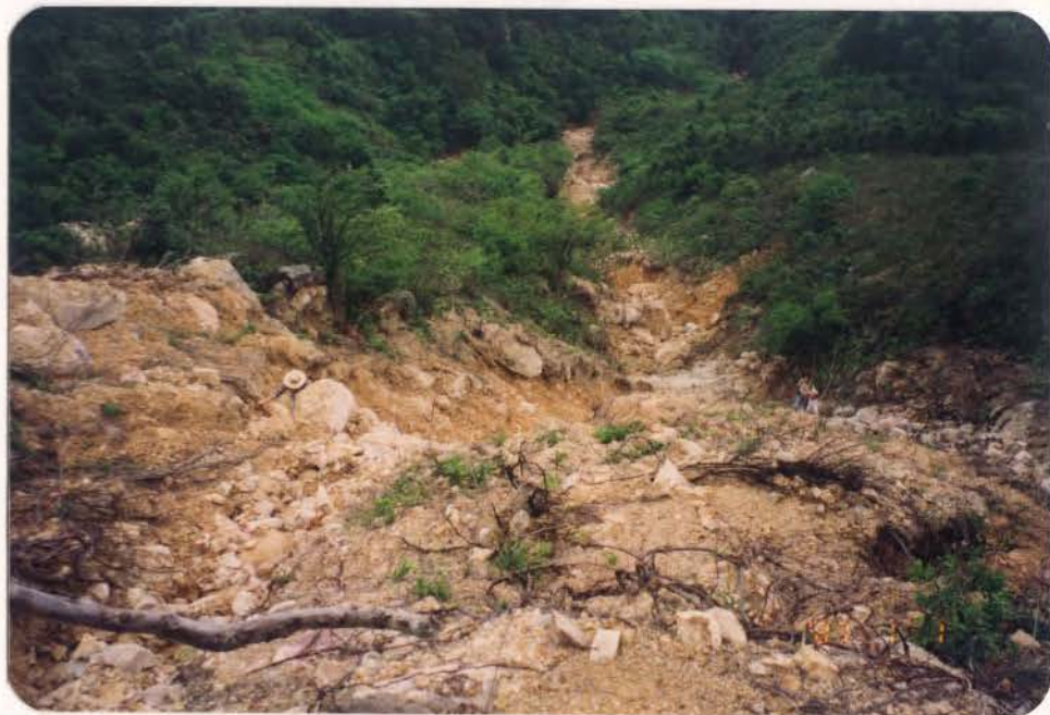
Plate B2.27 - Debris Trail Viewed Downhill from Scarp B2C
