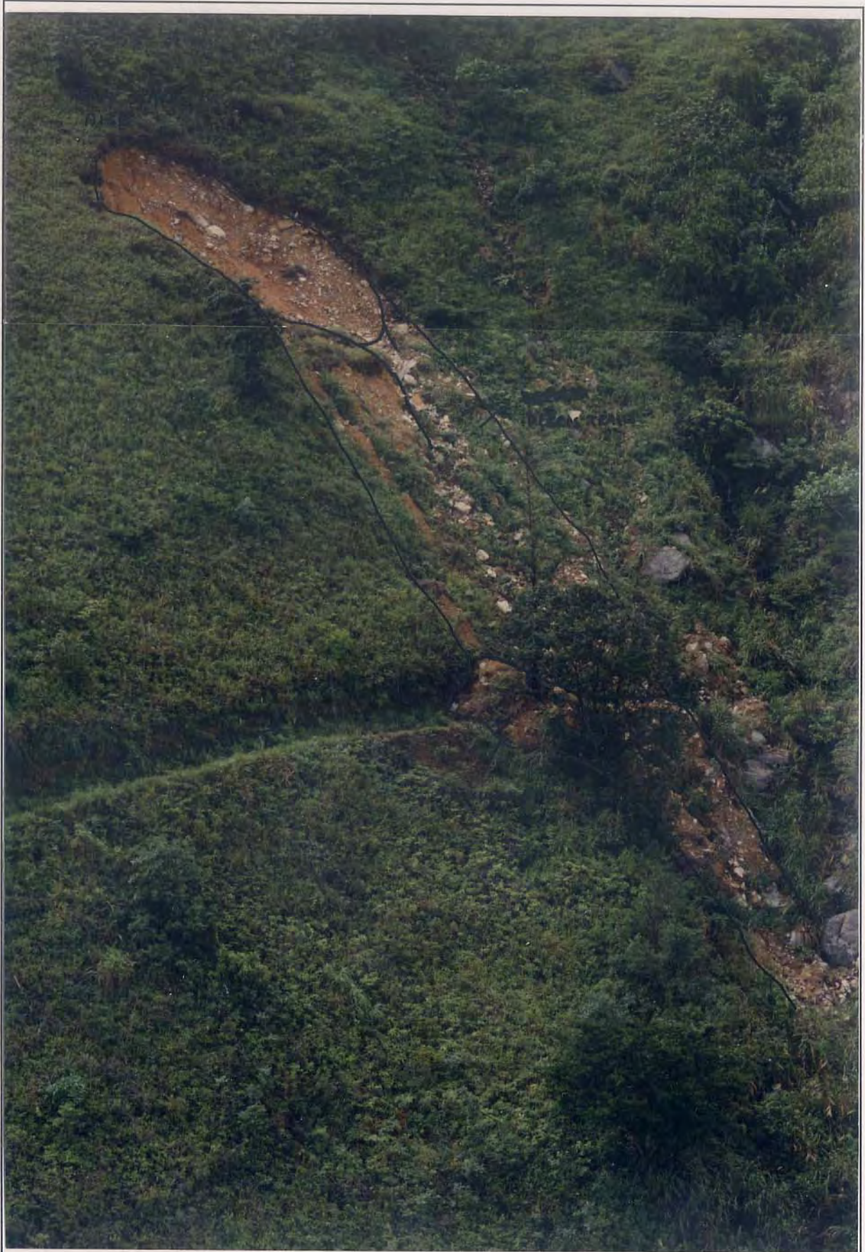
Plate A13.10 - Oblique View of Landslide A13B
