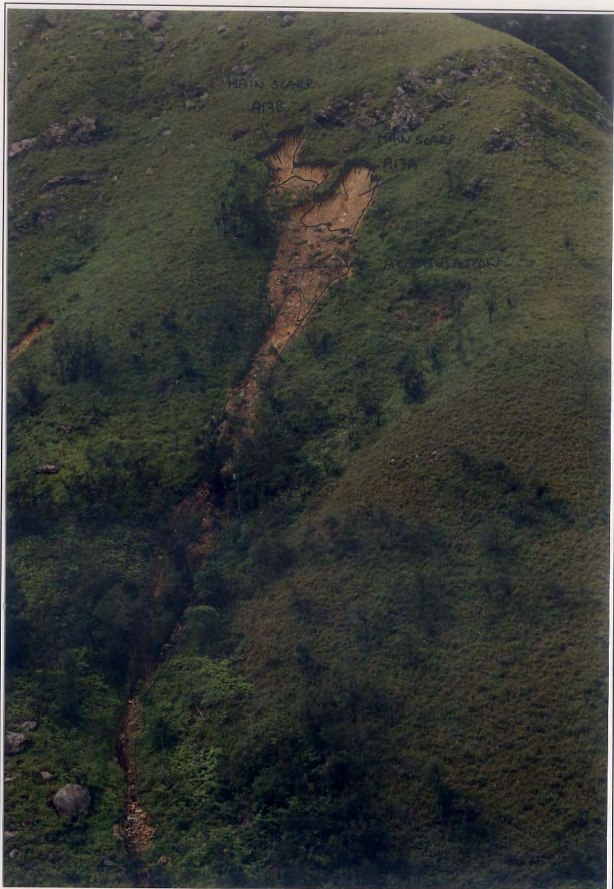
Plate A17.5 - Oblique View of Landslide A17
