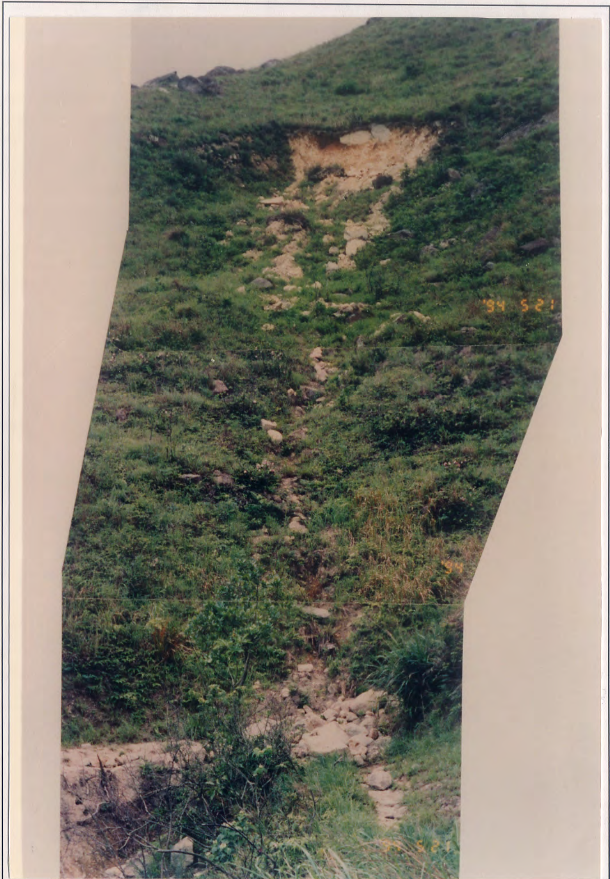
Plate A3.1 - Uphill View of Landslide A3 from Footpath
