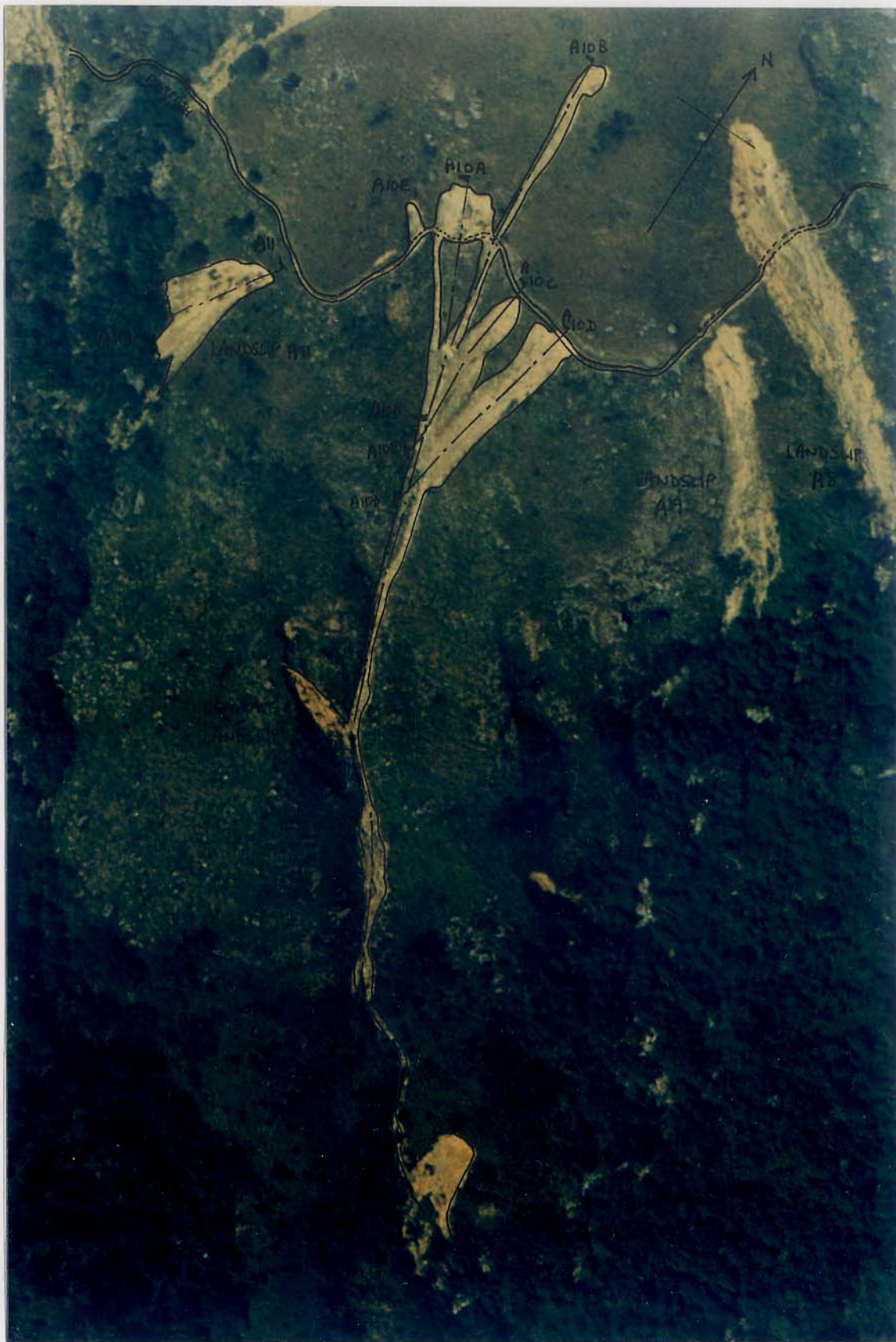
Plate A10.1 - Aerial View of Landslides A10 & A11
