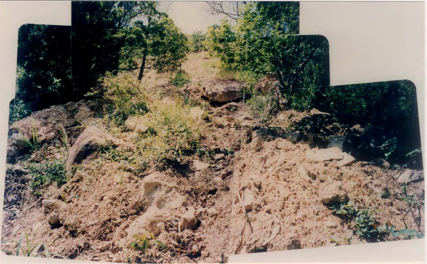
Plate A15.2 - Uphill View of Landslide A15
