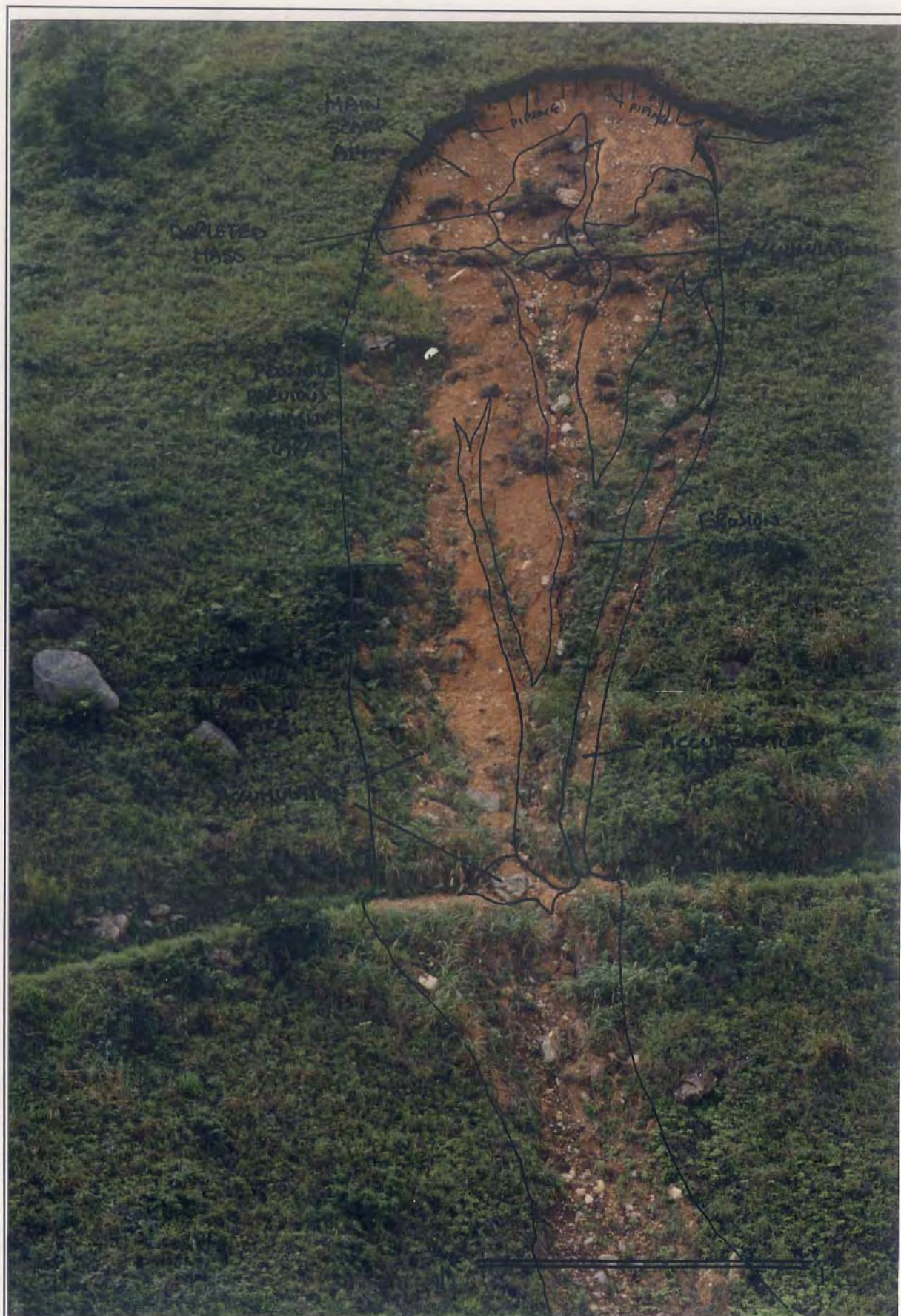
Plate A14.4 - Close-up of Landslide A14
