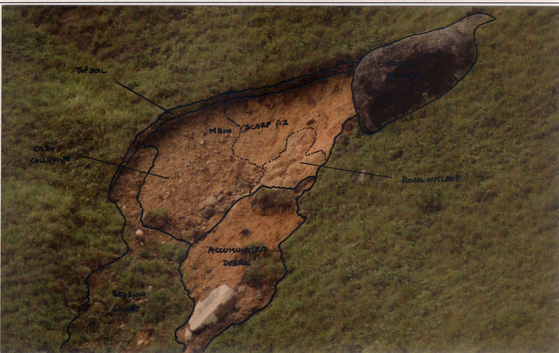
Plate A2.7 - Close-up of Landslide A2
