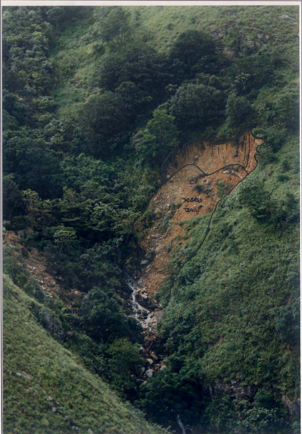
Plate A16.2 - Oblique View of Landslide A16A
