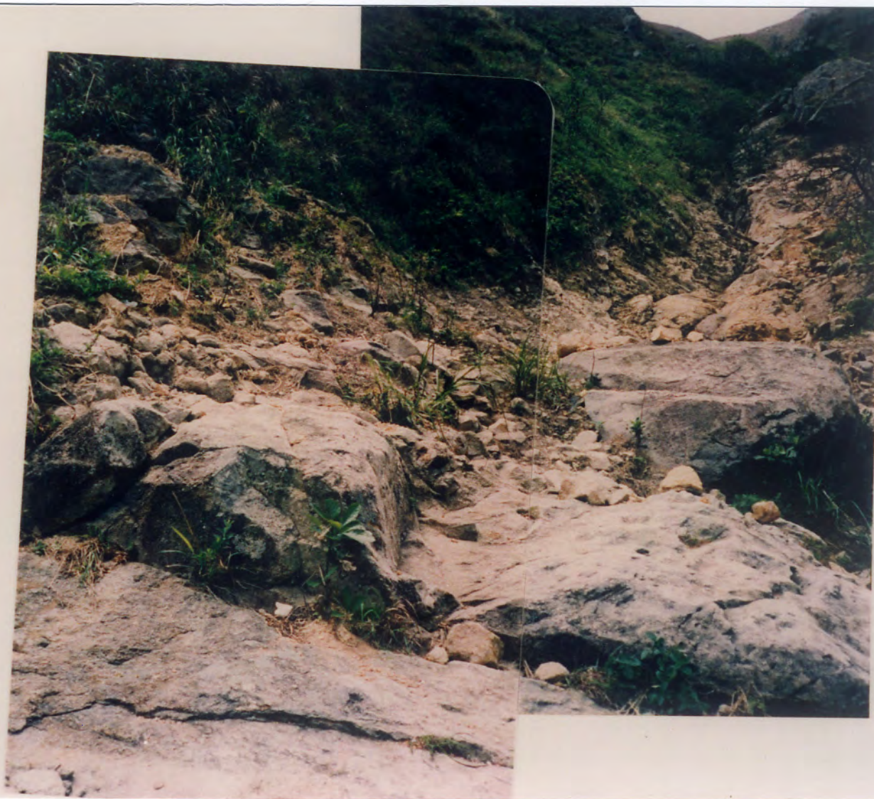
Plate A1.8 - Uphill View of Debris Trail of Landslide A1B from Footpath
