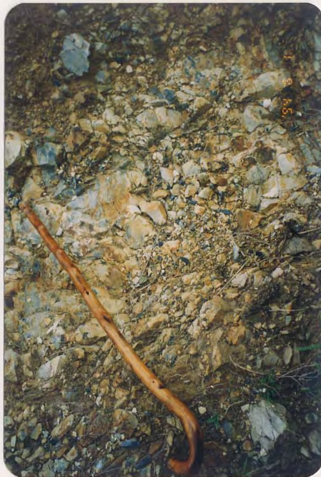
Plate A10.8 - Volcanic Rock Exposed at Footpath below Landslide A10B
