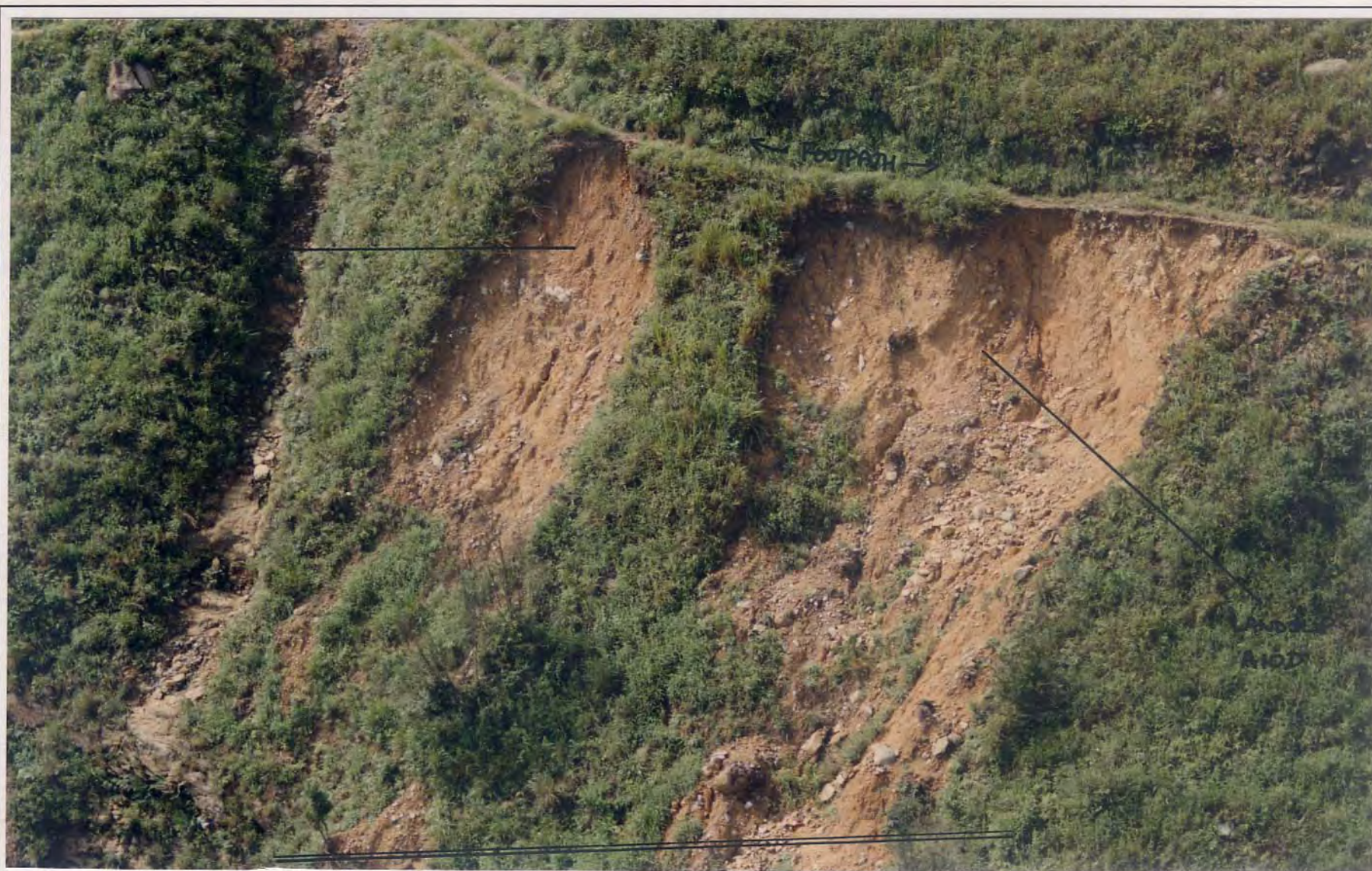
Plate A10.9 - Oblique View of Landslides A10C & A10D
