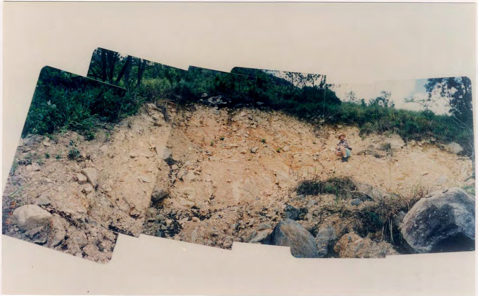
Plate A15.5 - Close-up of Landslide Scarp A15
