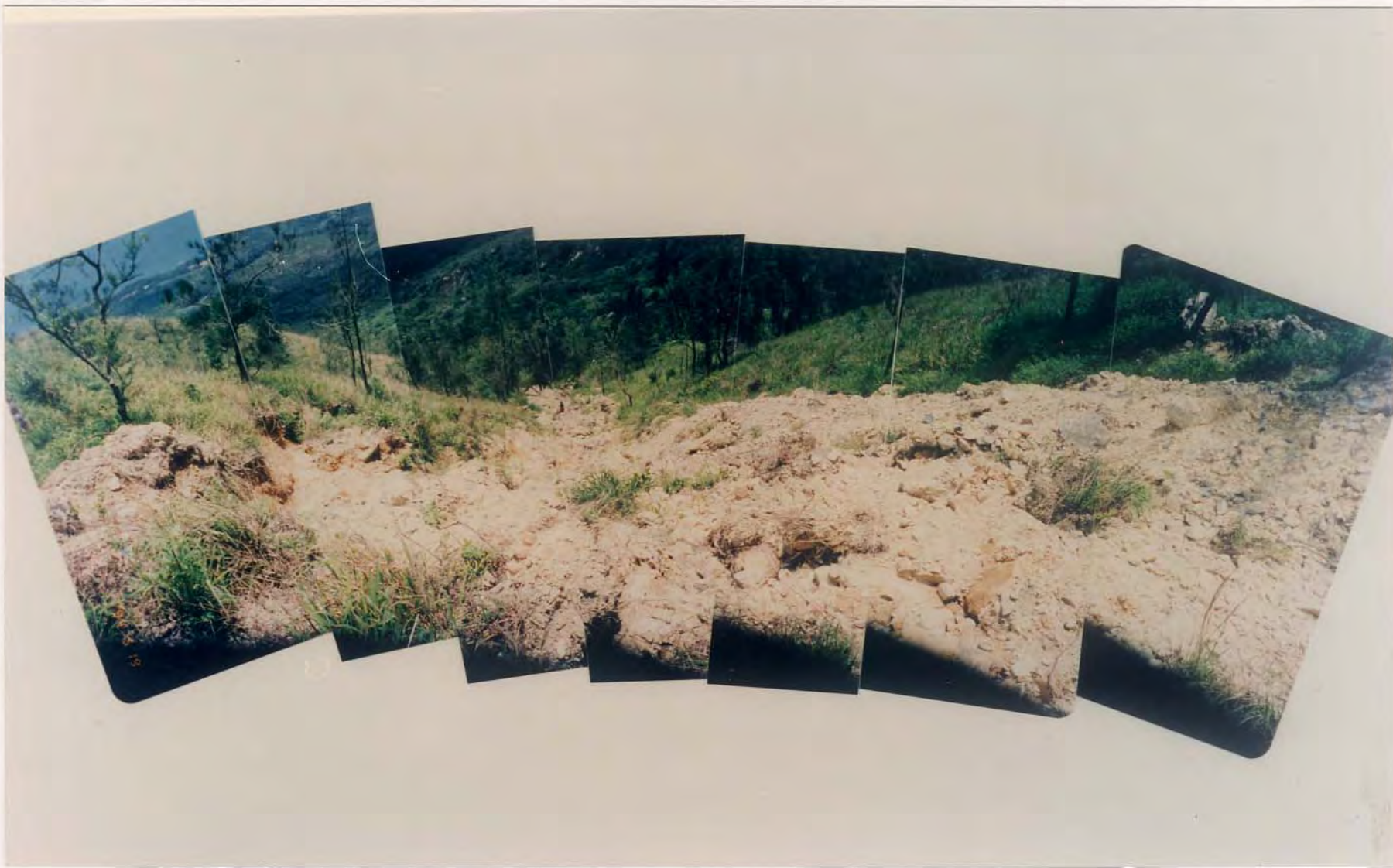
Plate A17.4 - Downhill View of Debris Trail of Landslide A17
