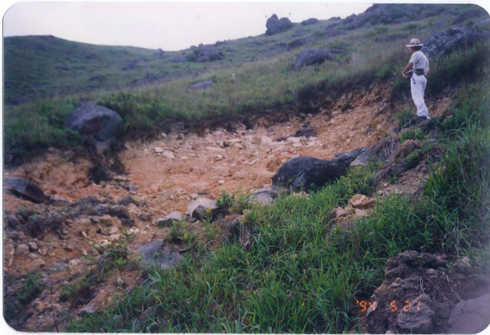
Plate A1.4 - Main Scarp of Landslide A1A
