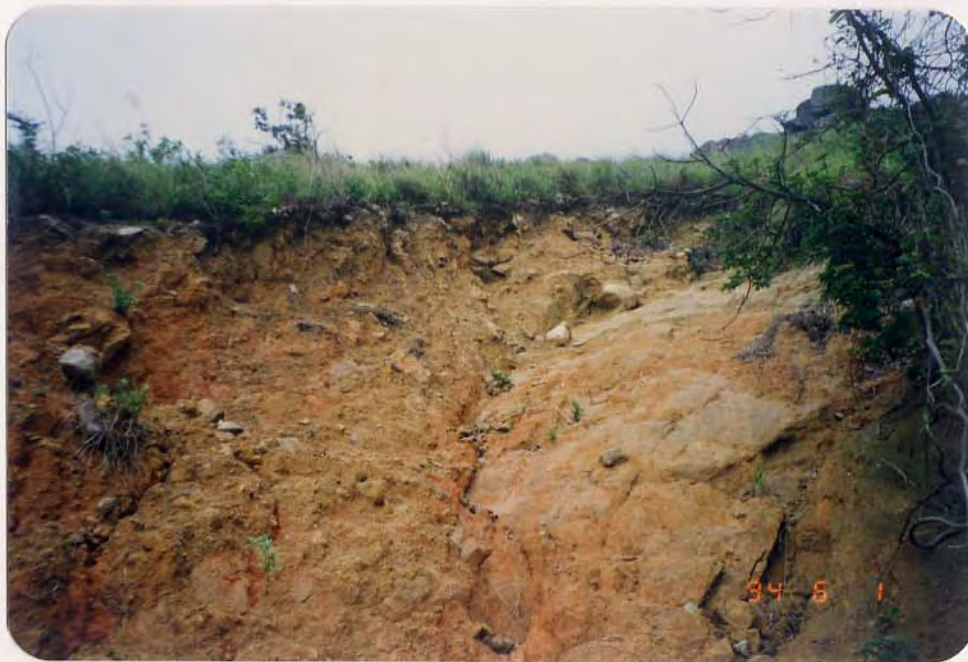
Plate A13.8 - Close-up of Crown of Landslide A13A
