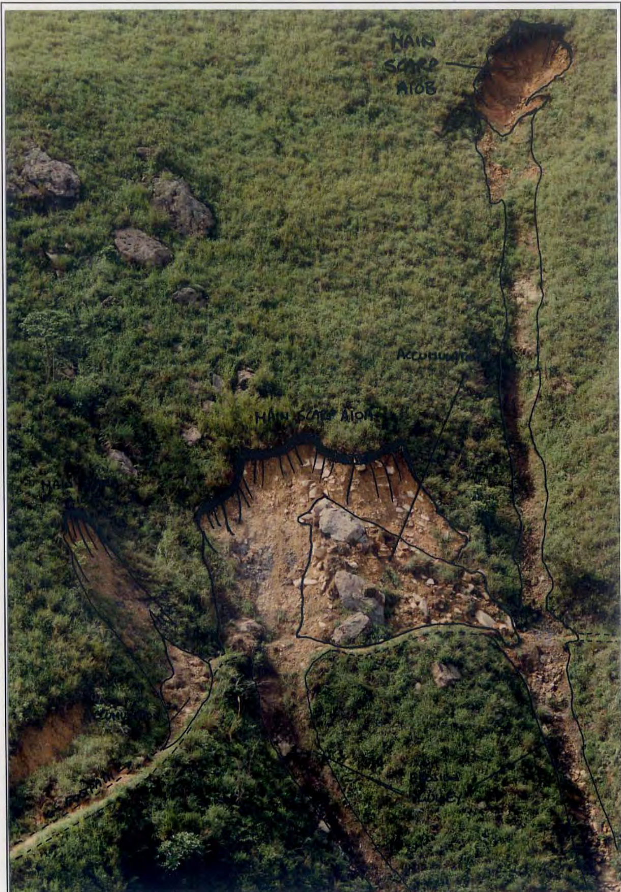
Plate A10.5 - Oblique View of Landslides A10A & A10B
