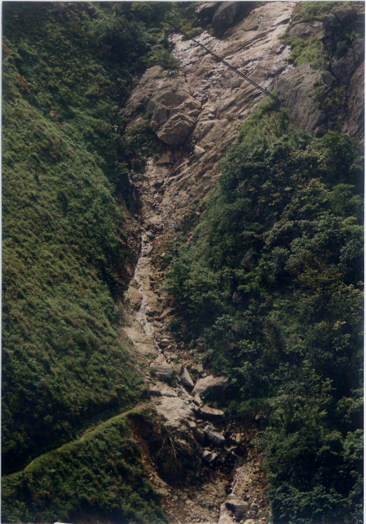
Plate A1.20 - Stream Course below Landslide A1B (CH139 - CH180)
