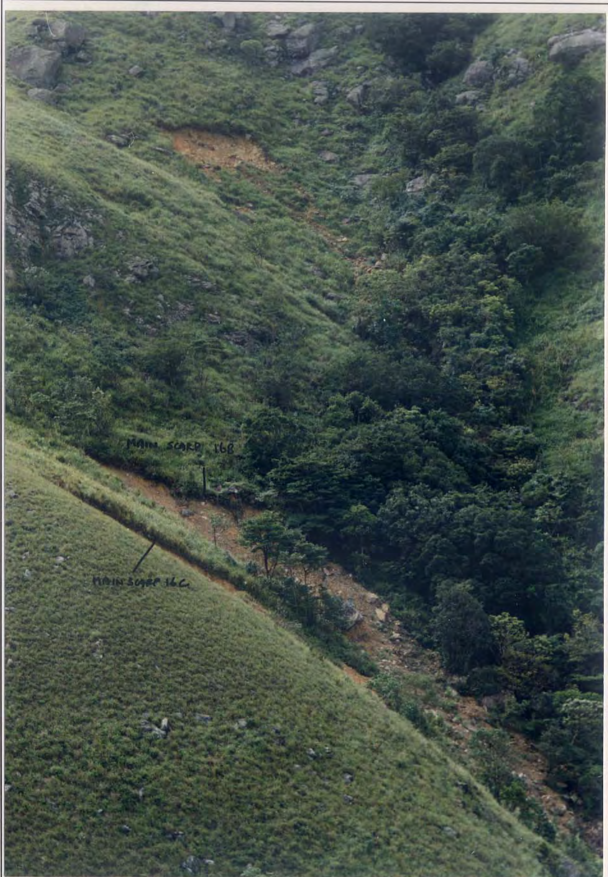
Plate A16.7 - Oblique View of Landslides A16B & A16C
