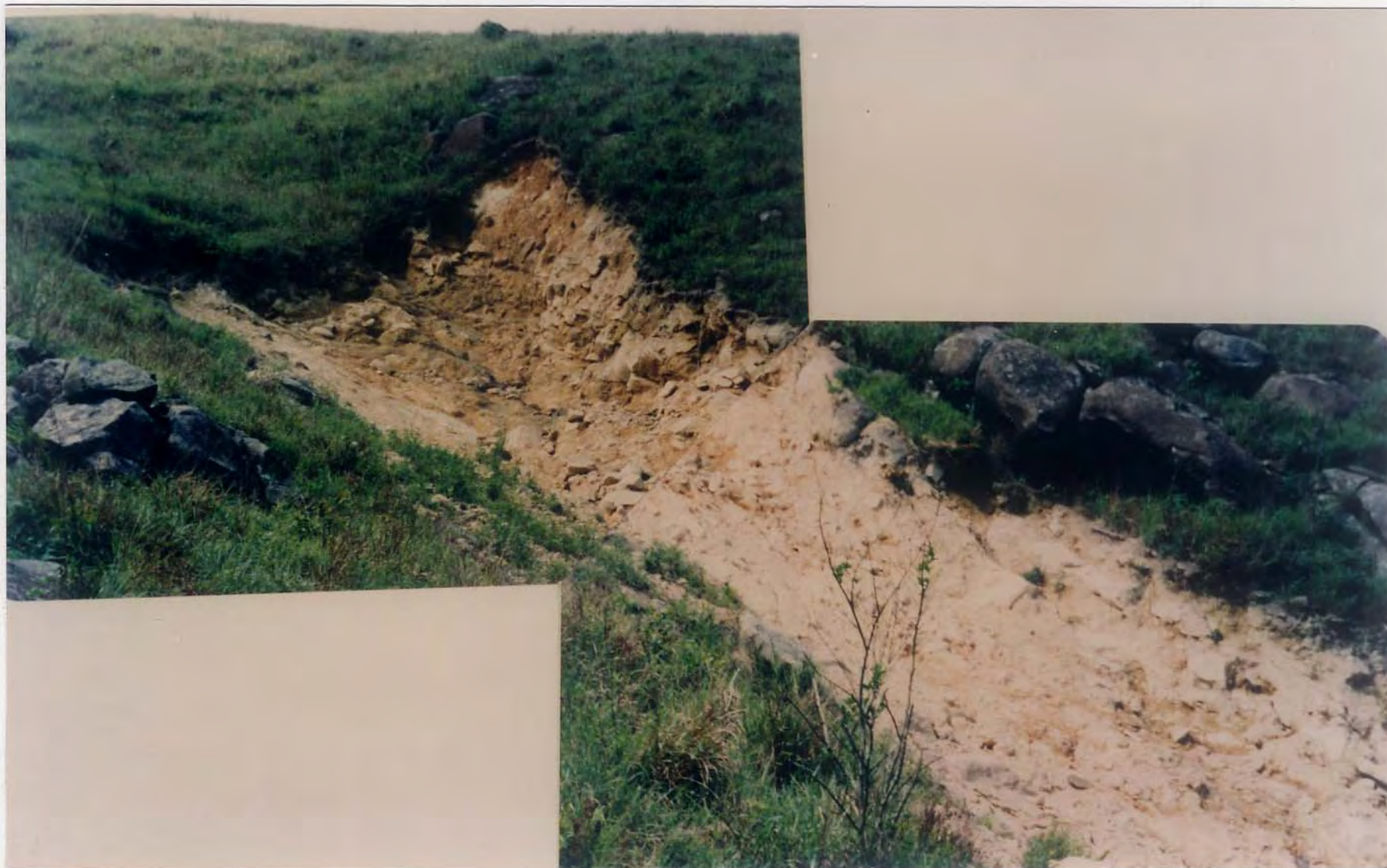
Plate A7.6 - Close-up of Landslide Scarp A7
