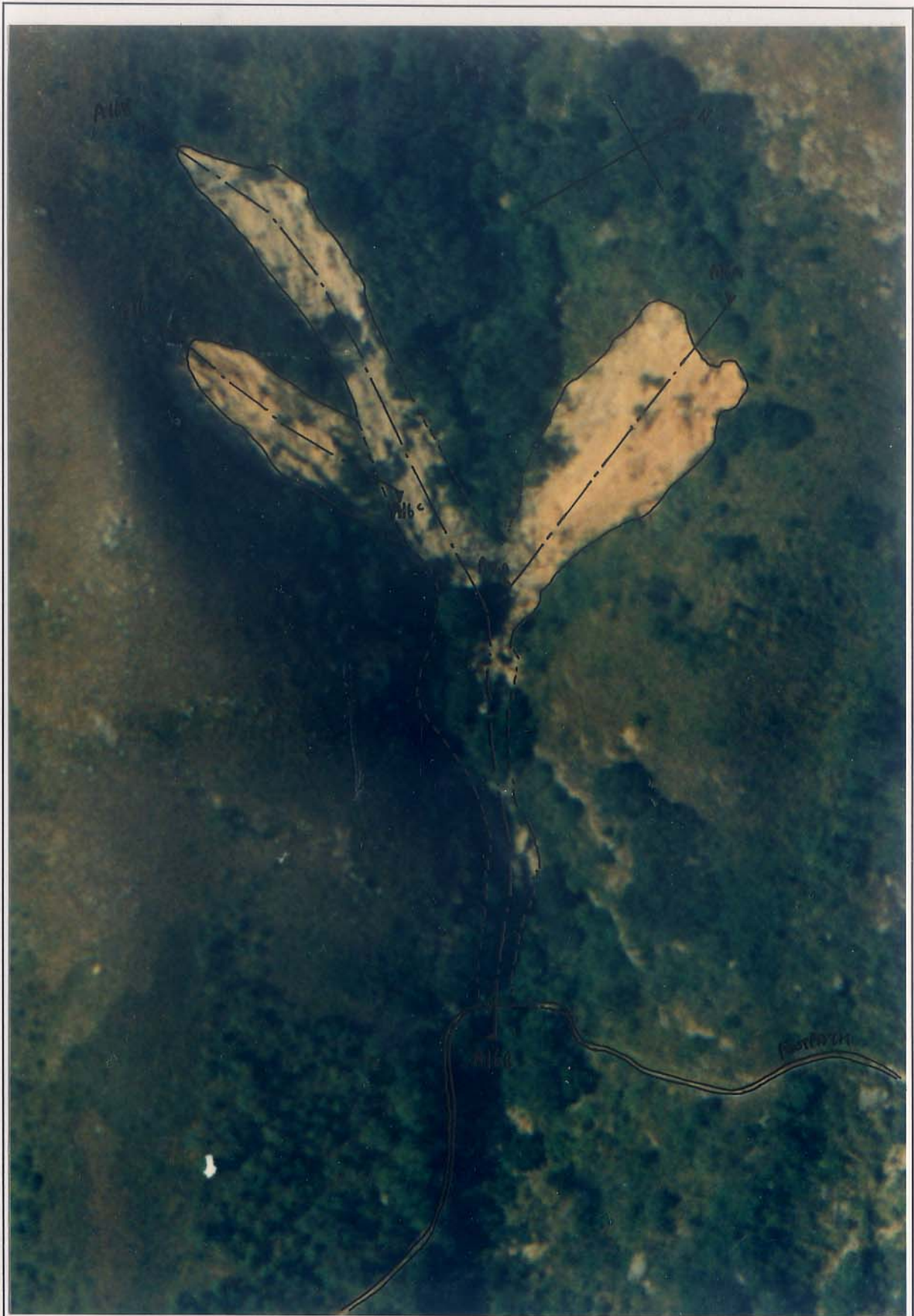
Plate A16.1 - Aerial View of Landslide Group A16
