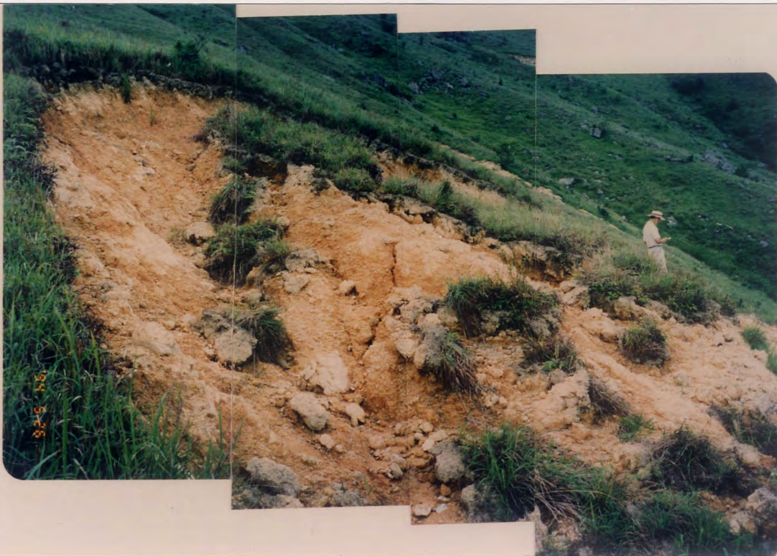
Plate A6.7 - Side View of Landslide Scarp A6
