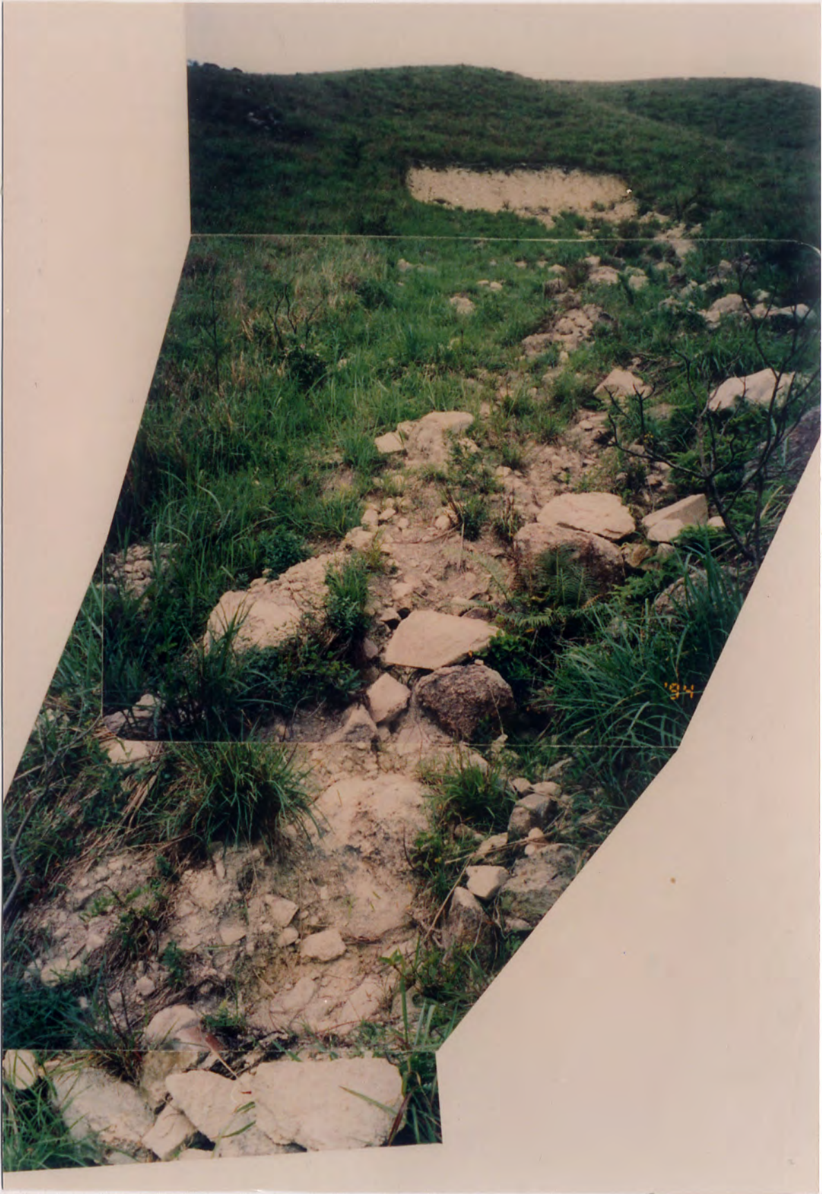
Plate A4.2 - Uphill View of Debris Trail of Landslide A4
