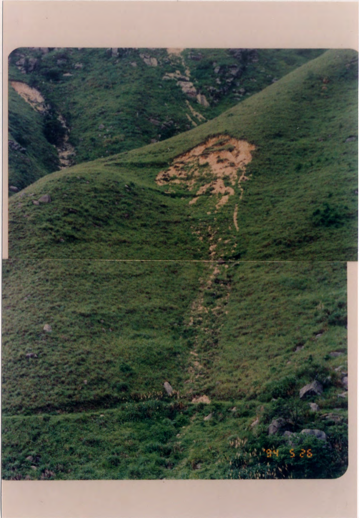
Plate A6.1 - Oblique View of Landslide A6
