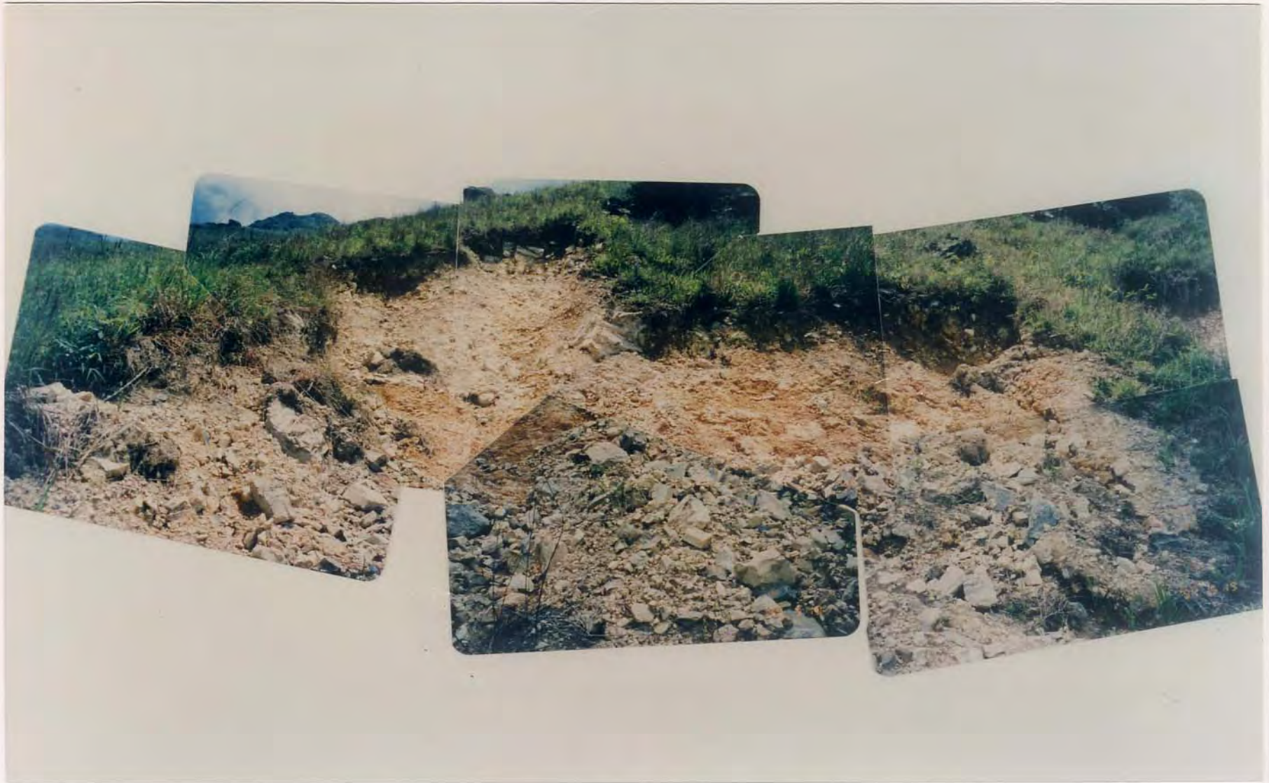
Plate A17.7 - Close-up of Landslide Scarp A17B
