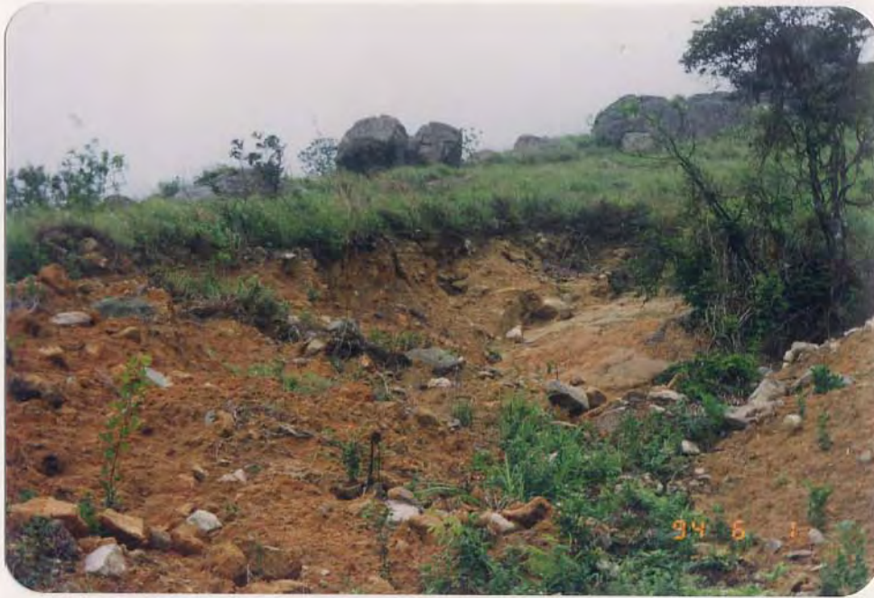
Plate A13.7 - Close-up of Landslide Scarp A13A
