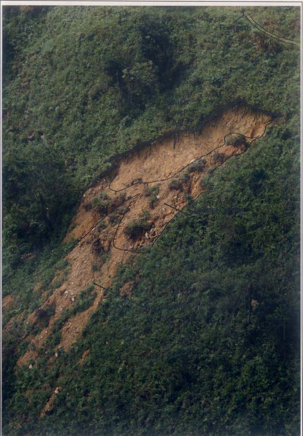
Plate A11.2 - Oblique View of Landslide A11
