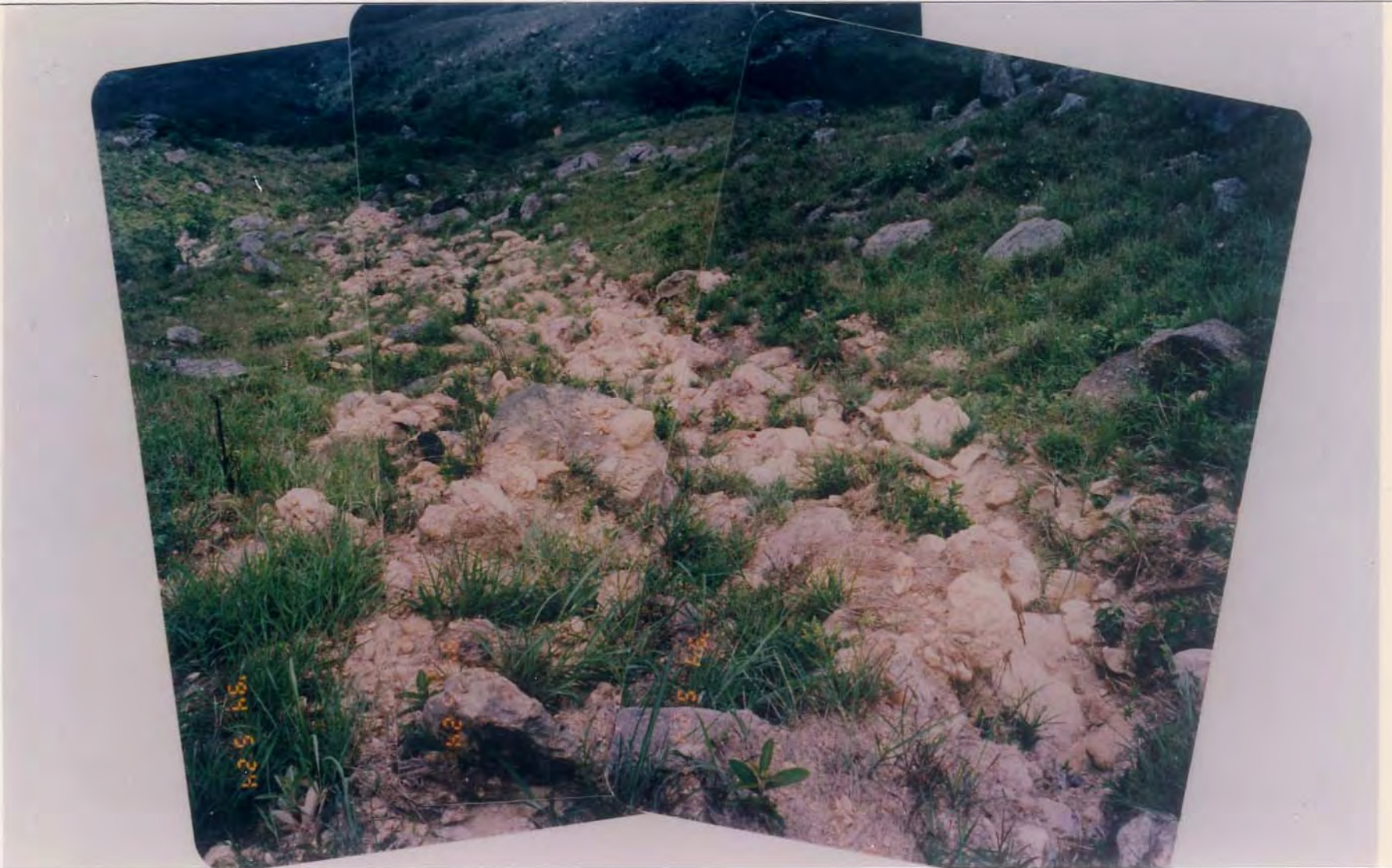
Plate A18.10 - Downhill View of Debris Trail from Landslide A18C
