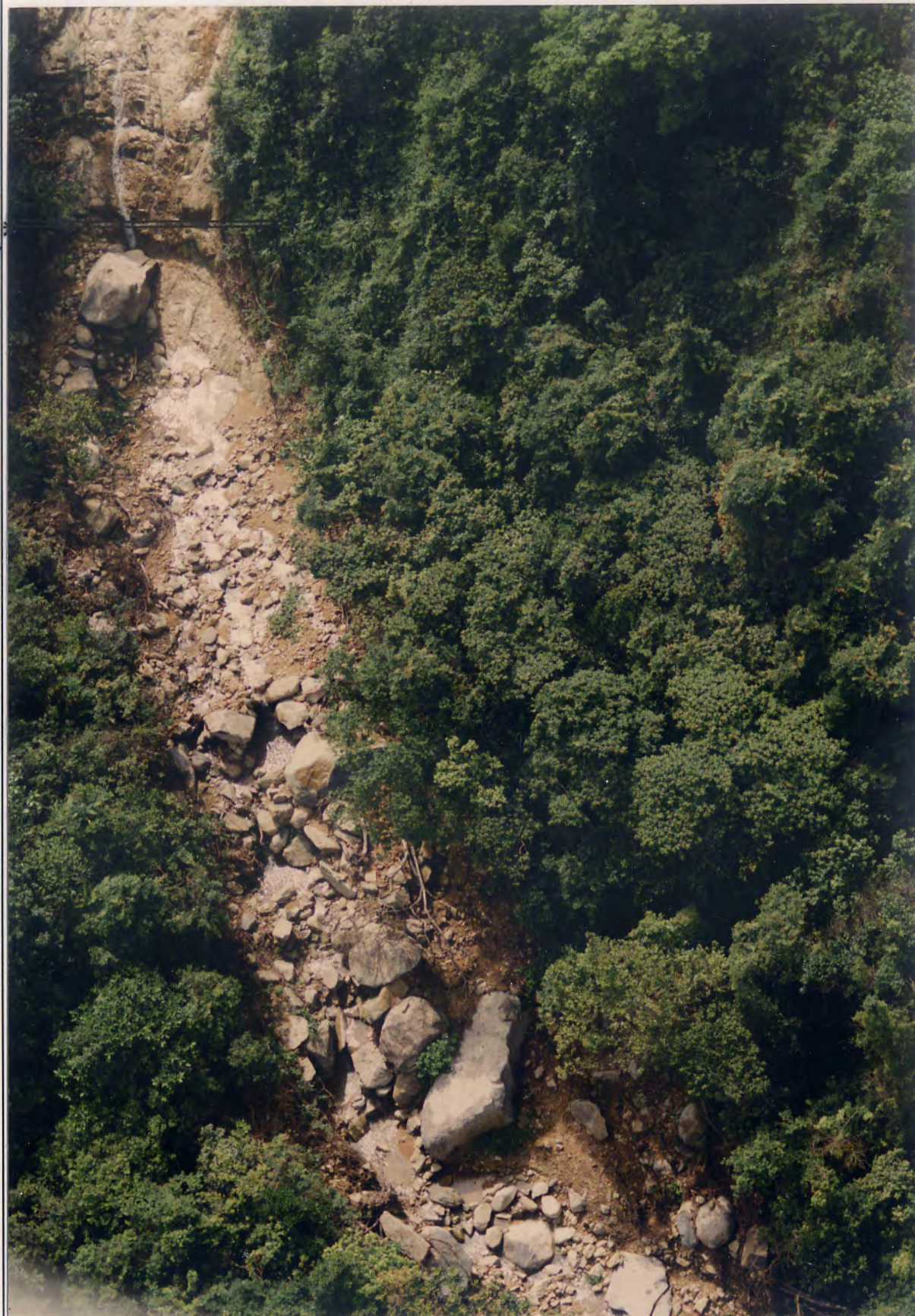
Plate A1.23 - Stream Course below Landslide A1B (from about CH270 onward)
