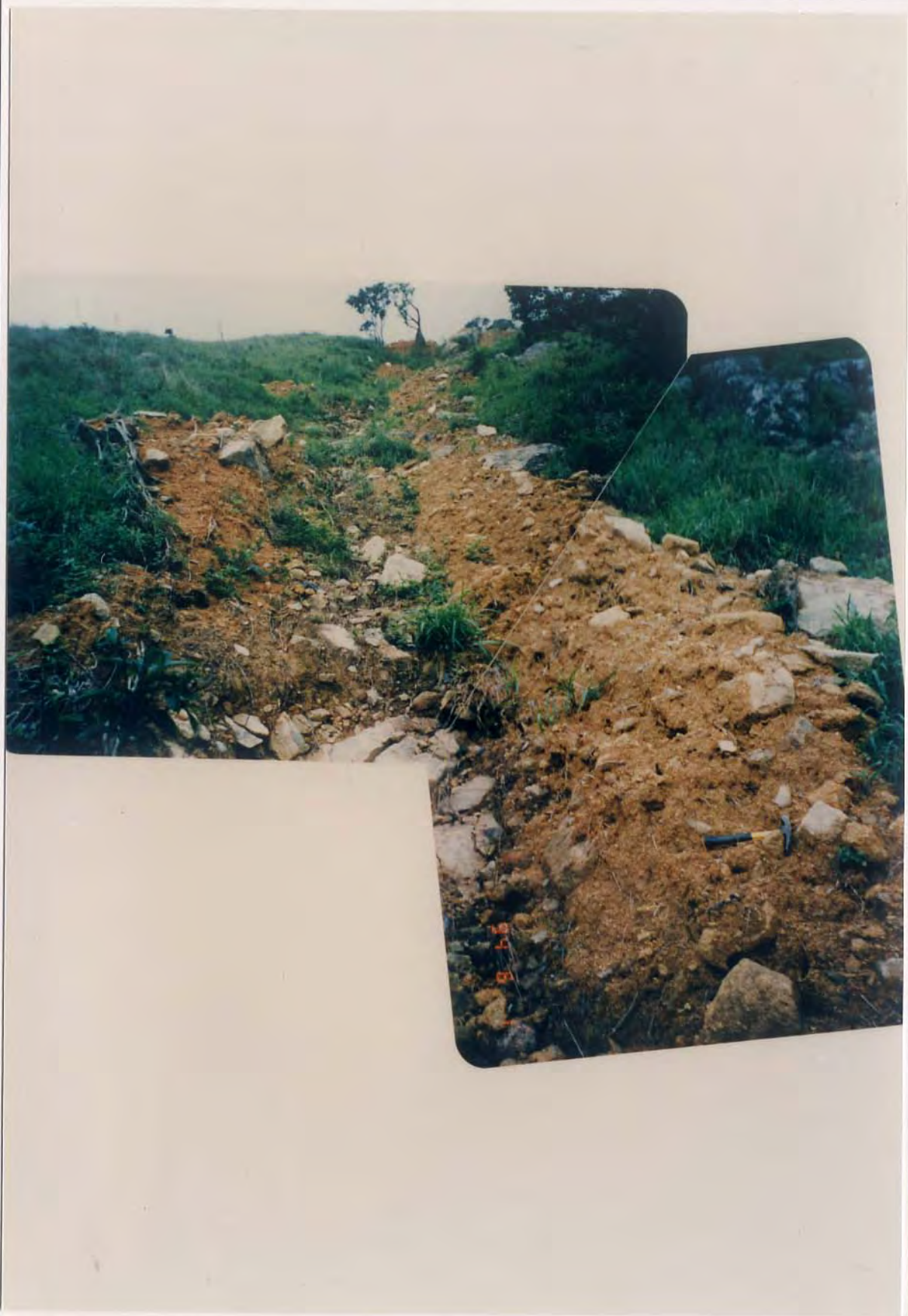
Plate A13.2 - Uphill View of Debris Trail of Landslide A13A
