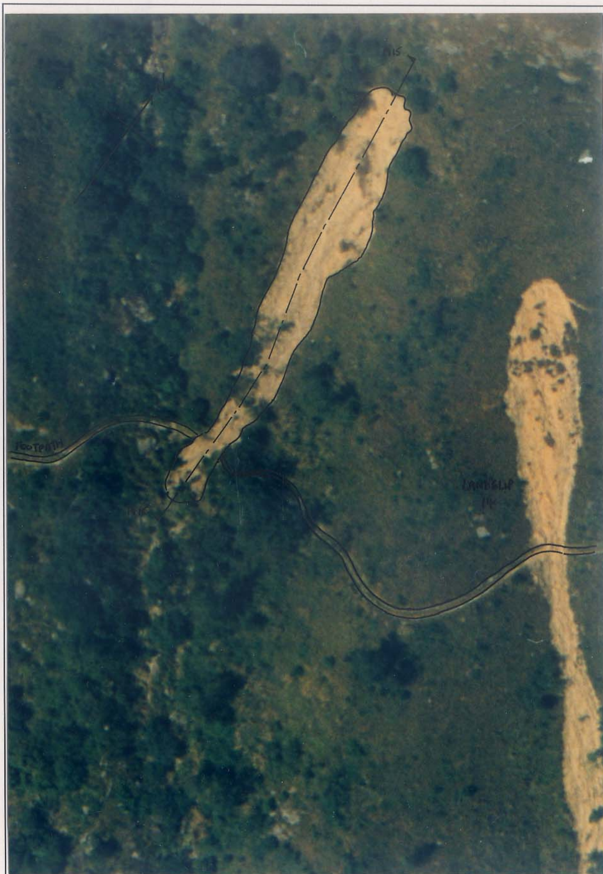
Plate A15.1 - Aerial View of Landslides A14 & A15
