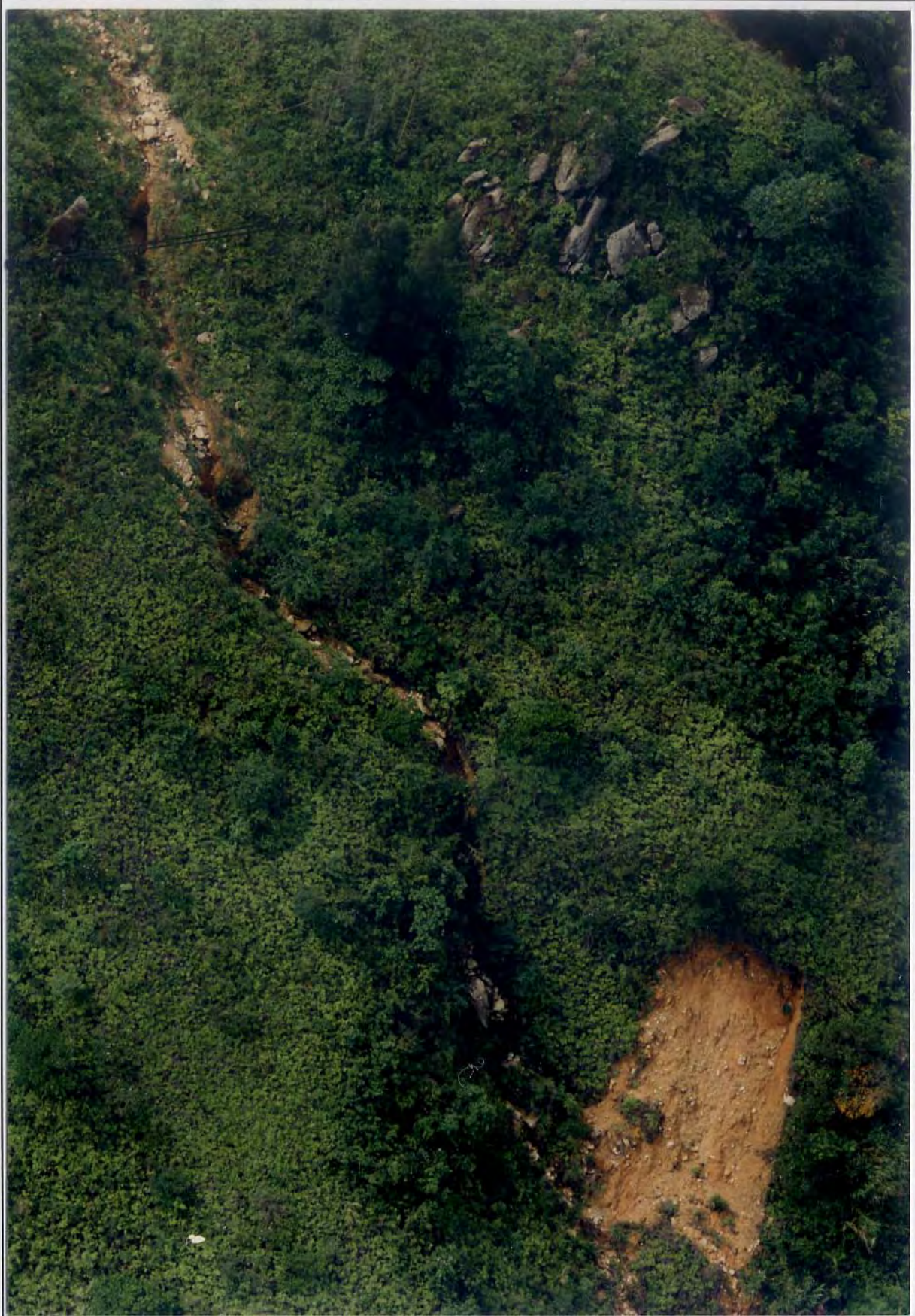
Plate A10.4 - Oblique View of Debris Trail of Landslide Group A10
