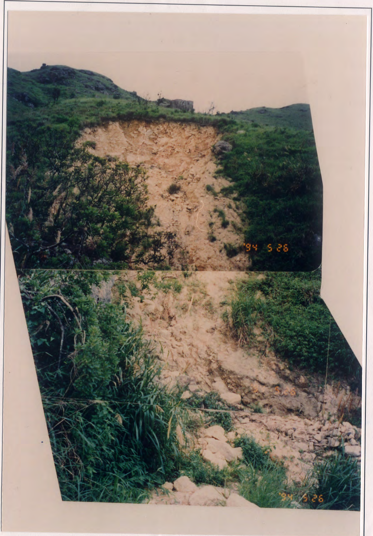
Plate A5.4 - Uphill View of Landslide A5A
