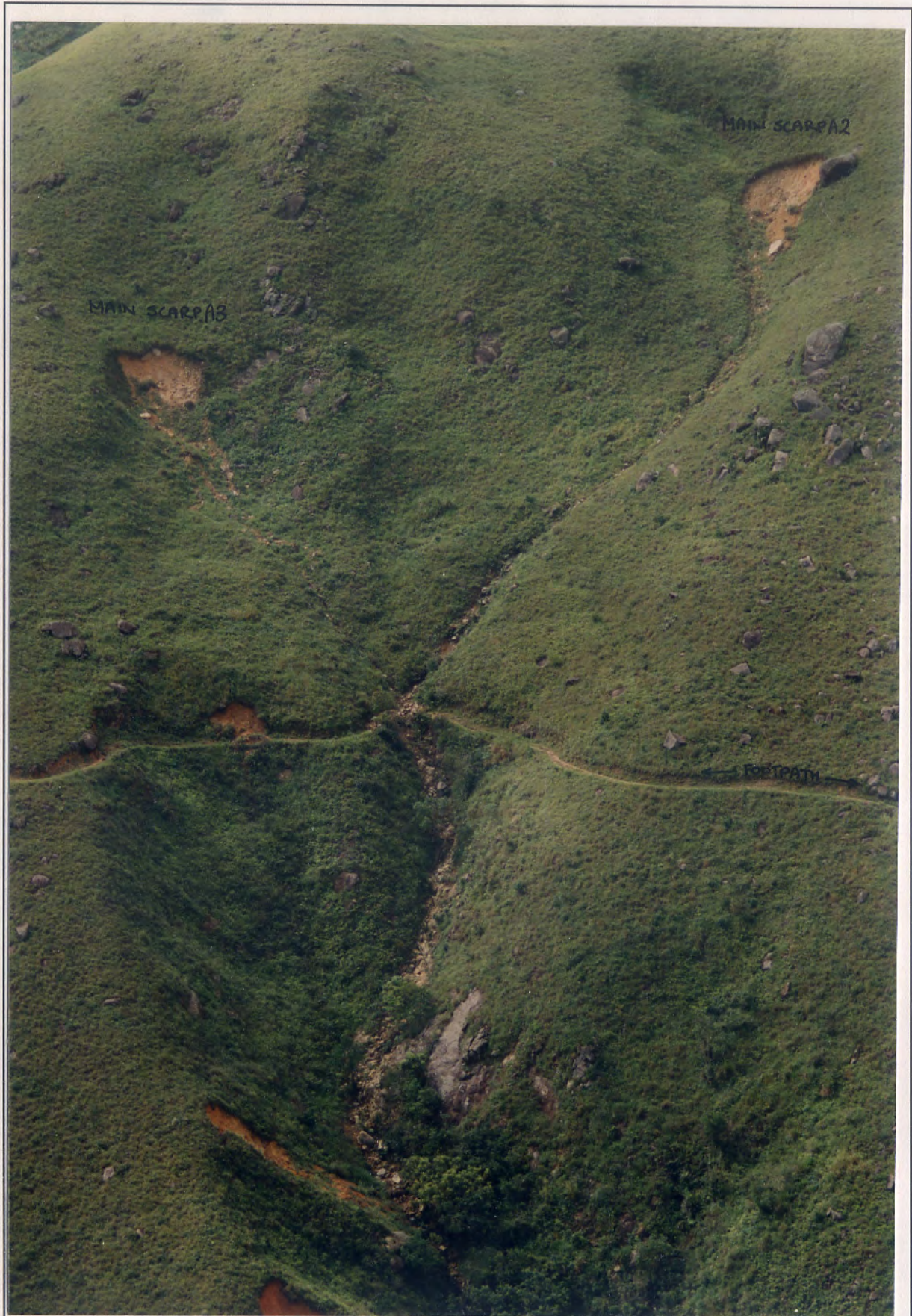
Plate A2.2 - Oblique View of Landslides A2 & A3
