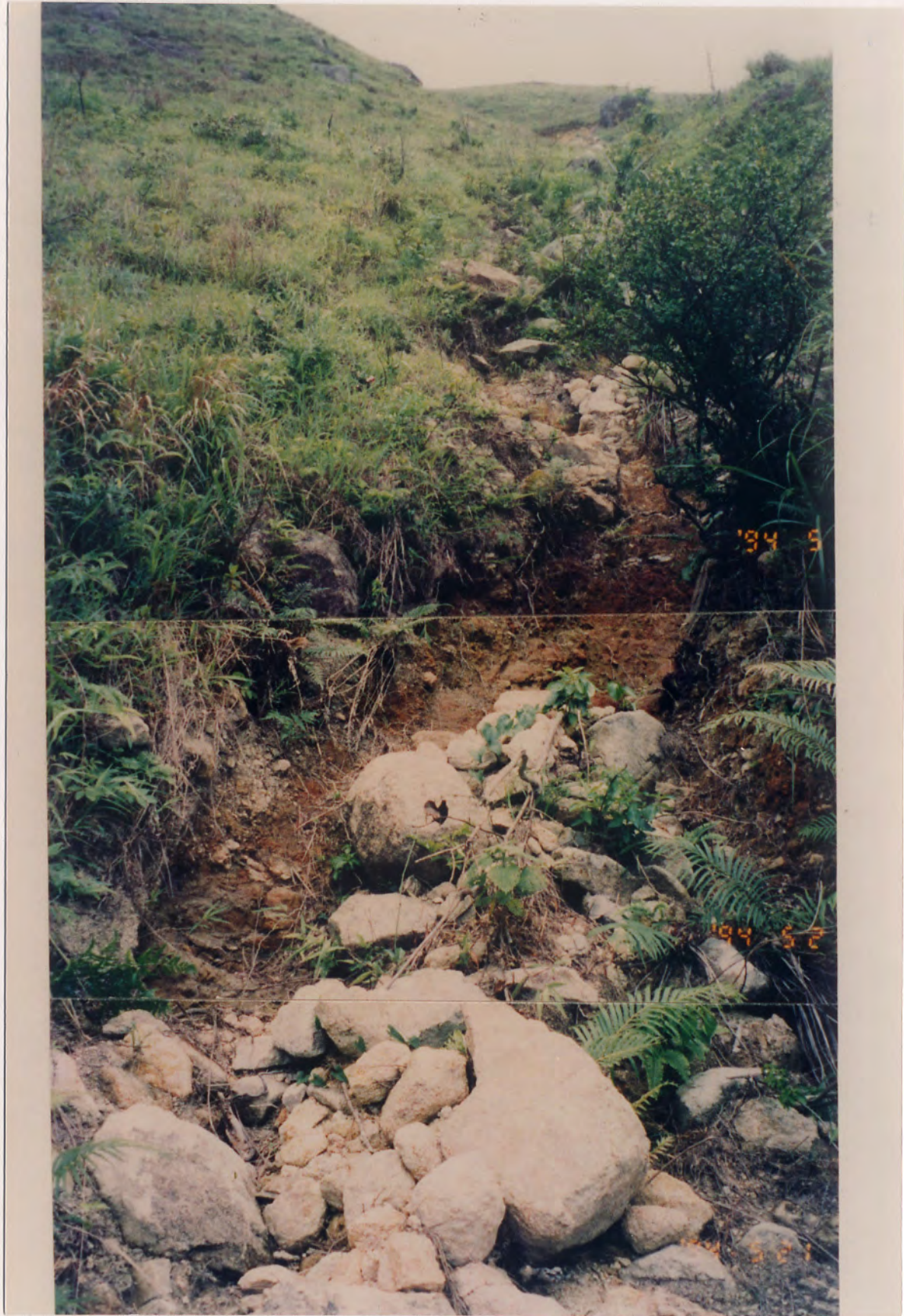
Plate A2.3 - Uphill View of Debris Trail of Landslide A2
