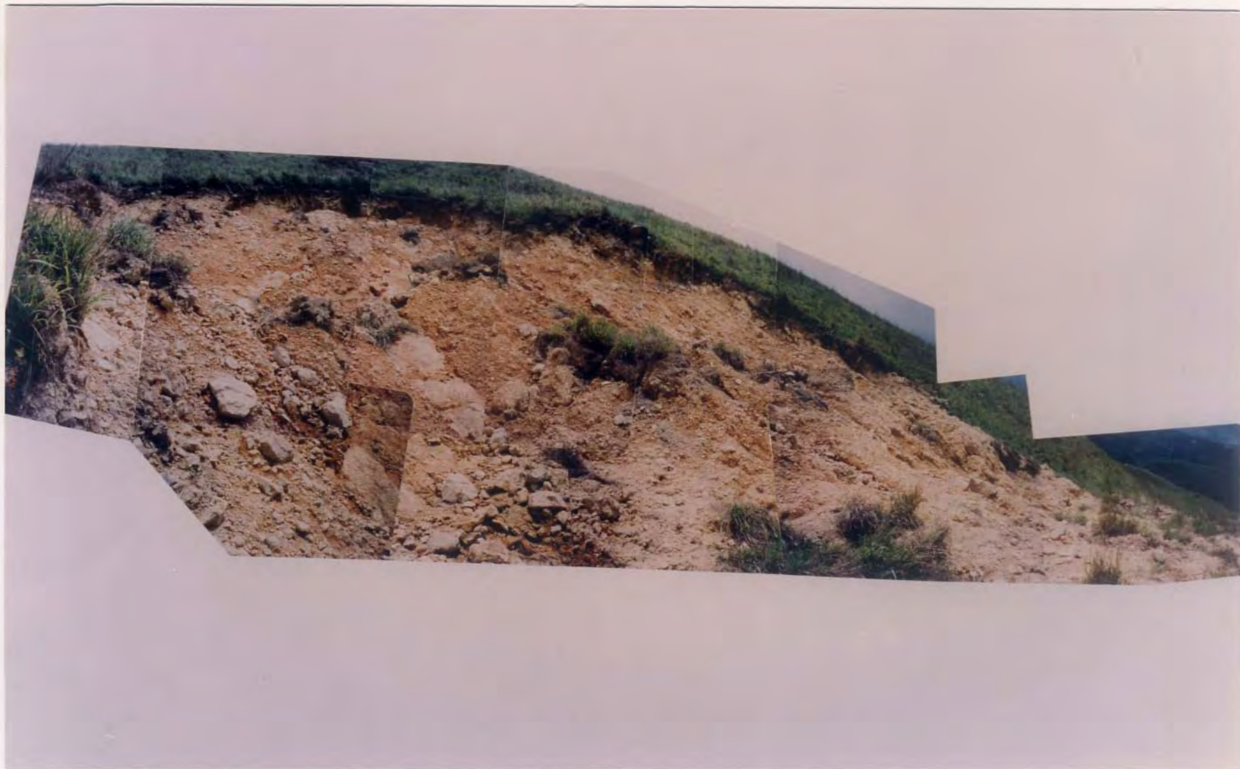
Plate A18.13 - Close-up of Landslide Scarp A18B
