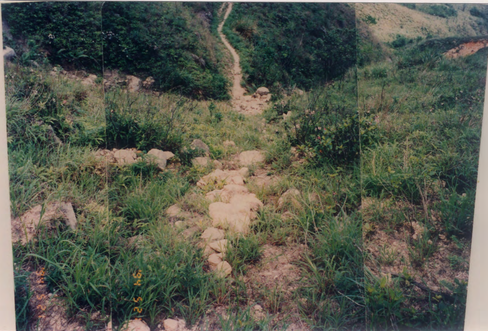
Plate A3.2 - Downhill View of Debris Trail of Landslide A3
