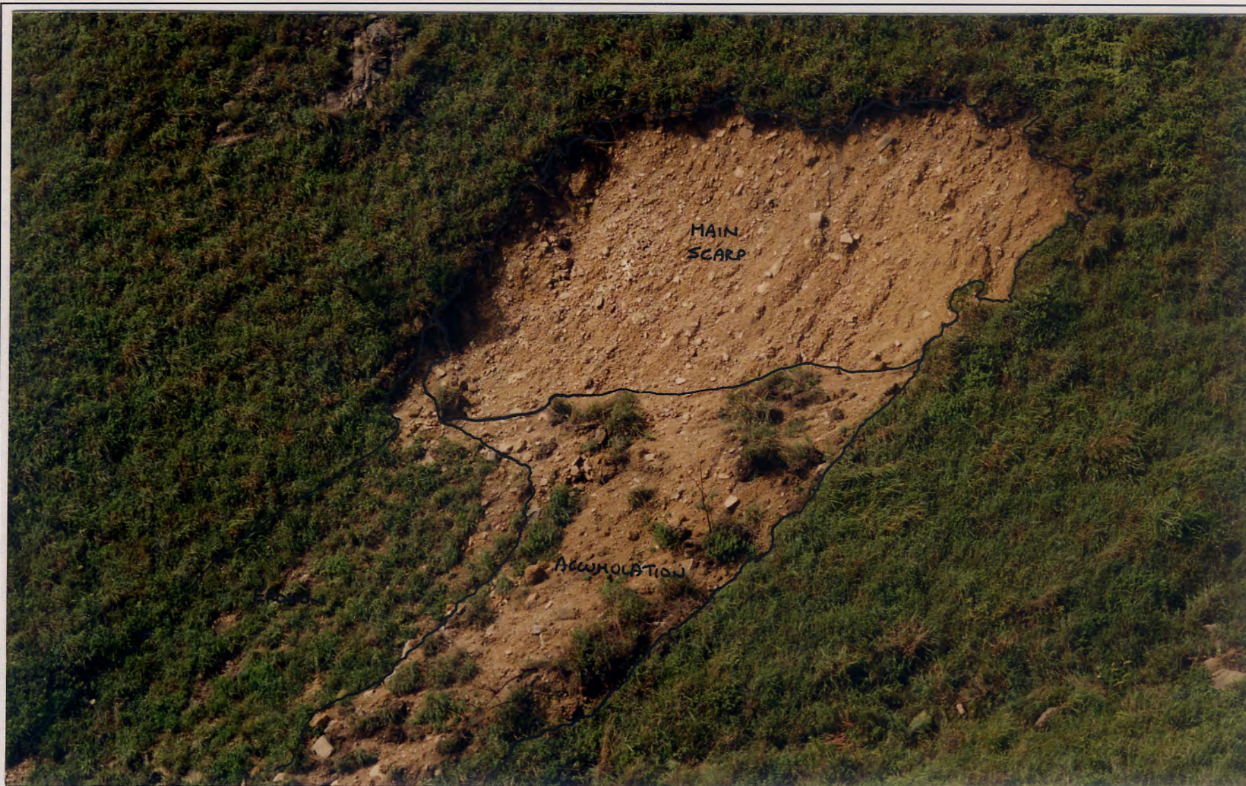
Plate A4.5 - Close-up of Landslide Scarp A4
