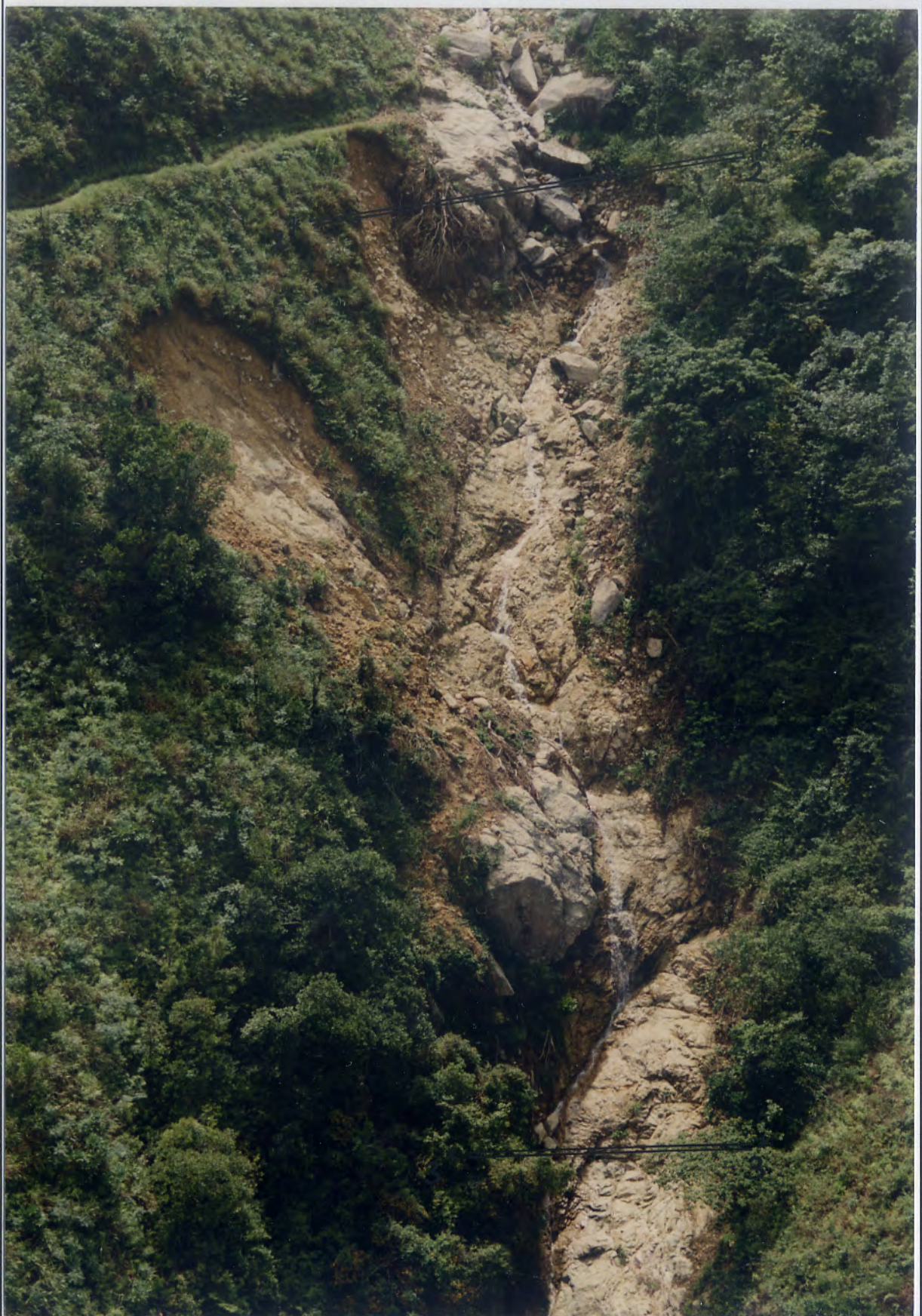
Plate A1.21 - Stream Course below Landslide A1B (CH180 - CH225)
