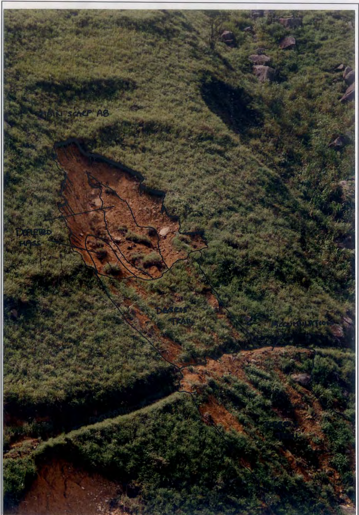
Plate A8.2 - Oblique View of Landslide A8
