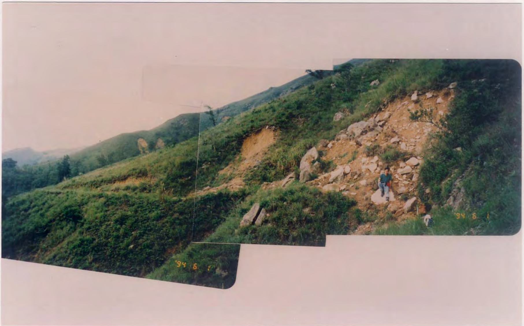
Plate A10.7 - View of Landslide Scarp A10A
