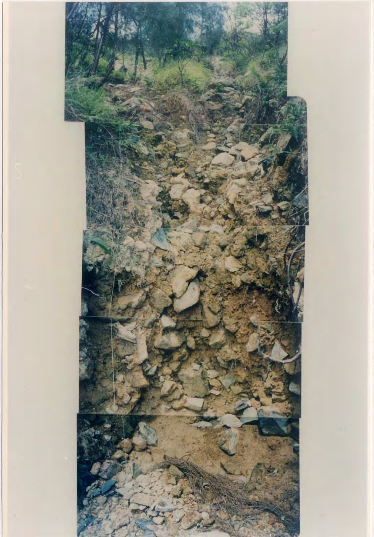
Plate A17.3 - Extensive Erosion along the Debris Trail of Landslide A17
