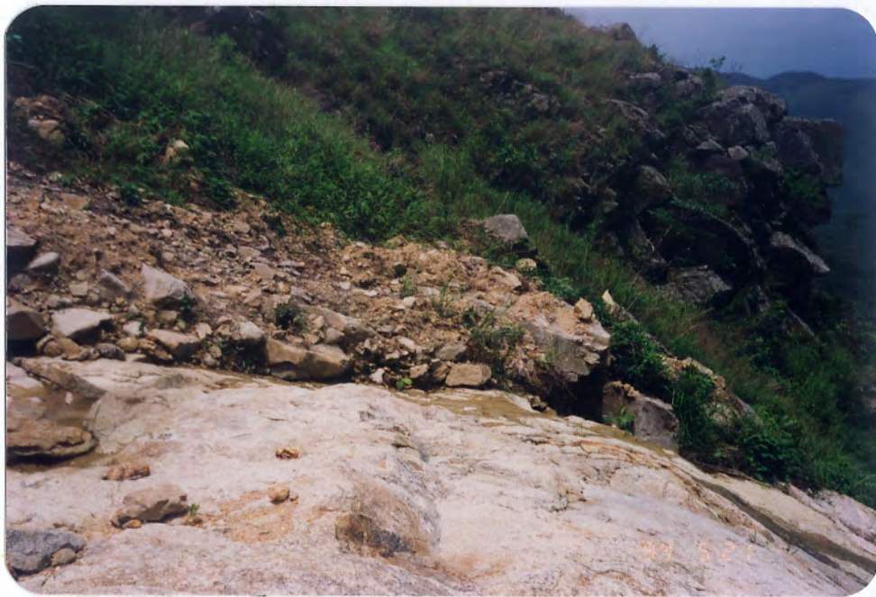
Plate A1.13 - Side View of Debris Trail of Landslide A1B from Top of Rock Cliff
