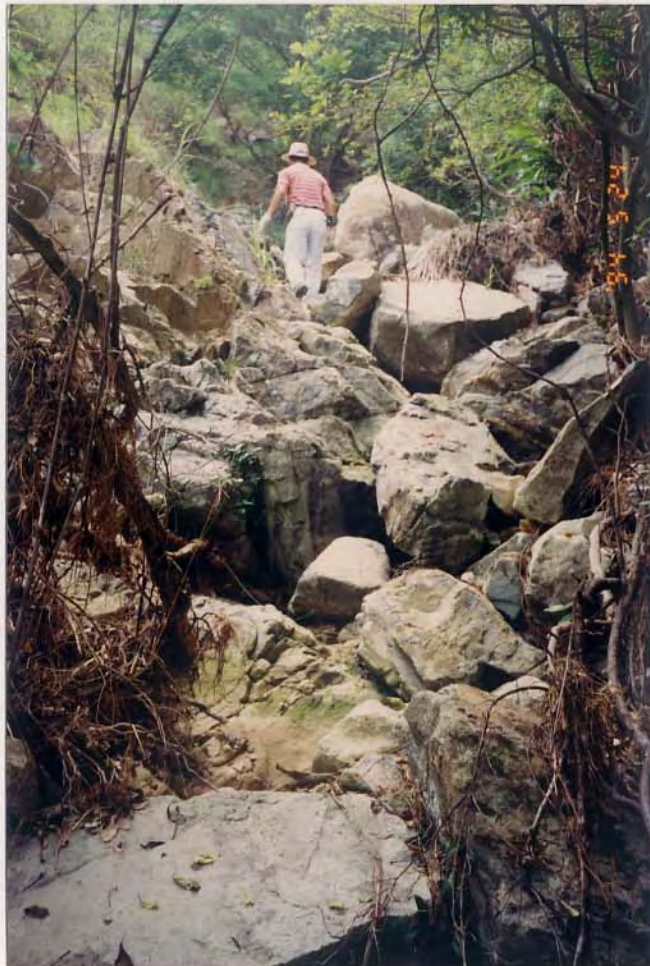
Plate A16.3 - View of Debris Trail of Landslide Group A16 from Footpath
