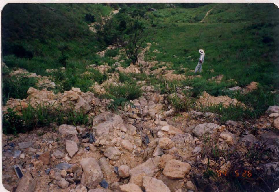
Plate A5.10 - Downhill View of Debris Trail of Landslide A5B
