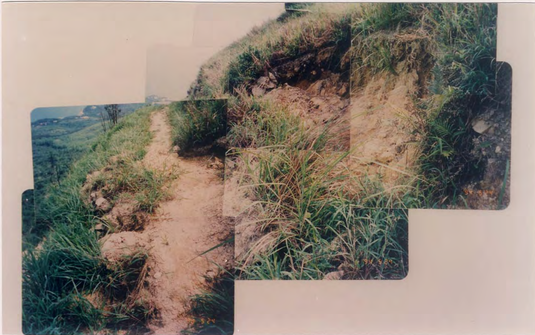
Plate A9.2 - Minor Landslide Adjacent to Footpath above Landslide A9
