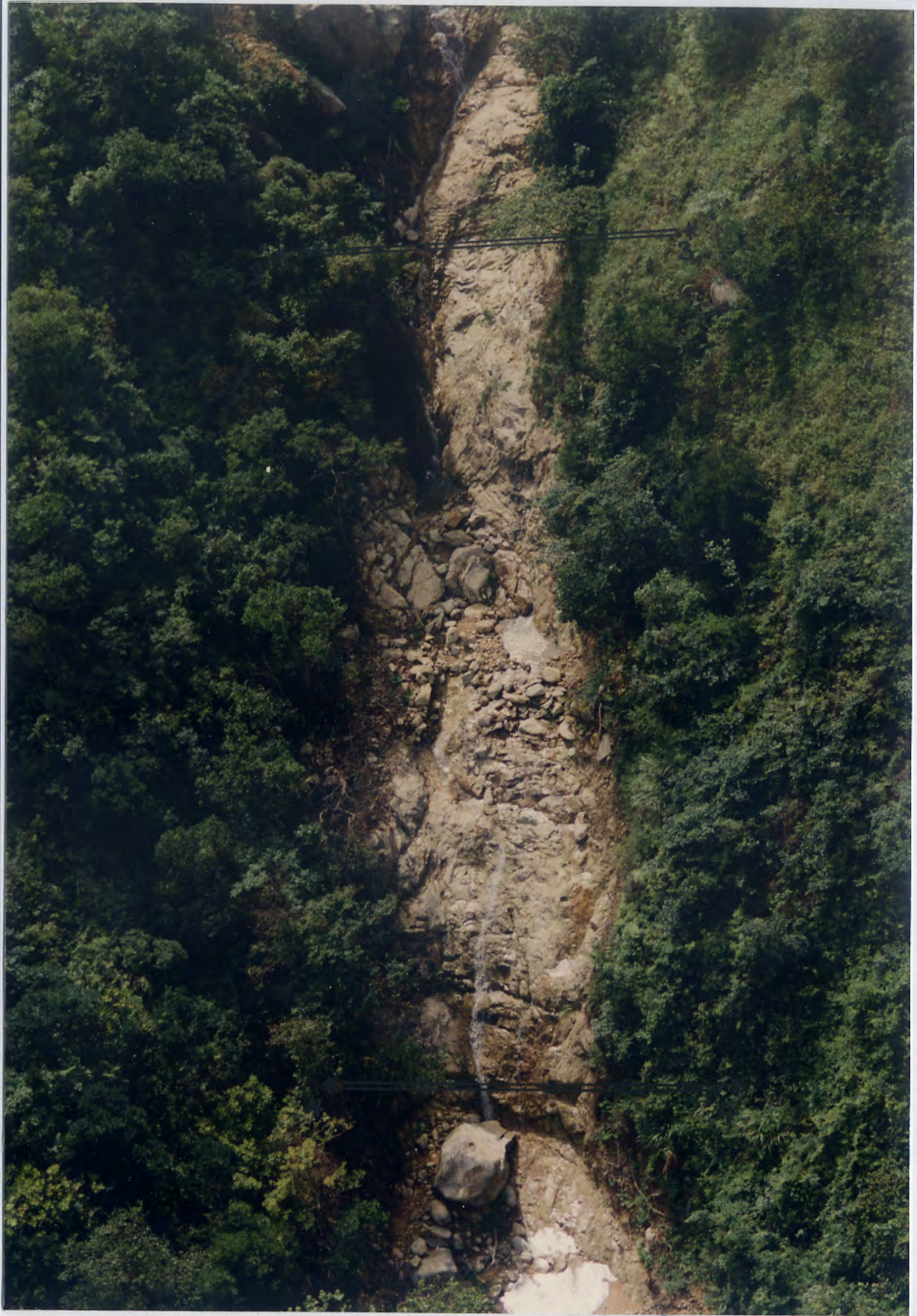
Plate A1.22 - Stream Course below Landslide A1B (CH225 - CH270)
