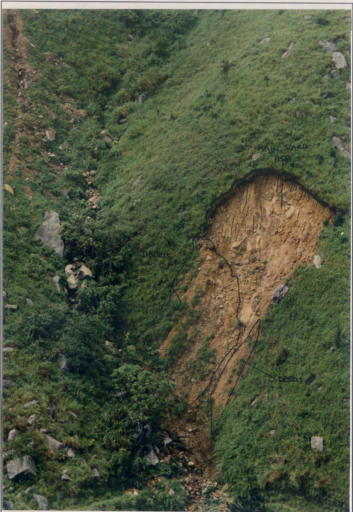
Plate A5.6 - Oblique View of Landslide A5A
