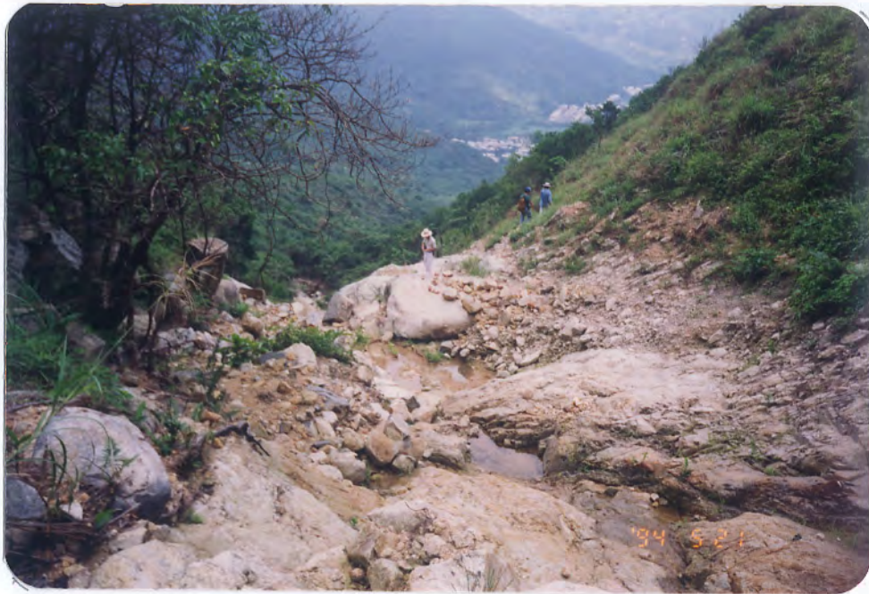
Plate A1.9 - Downhill View of Debris Trail of Landslide A1B
