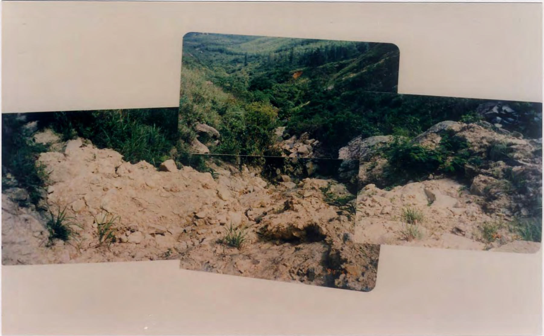
Plate A7.3 - Downhill View of Debris Trail from Footpath
