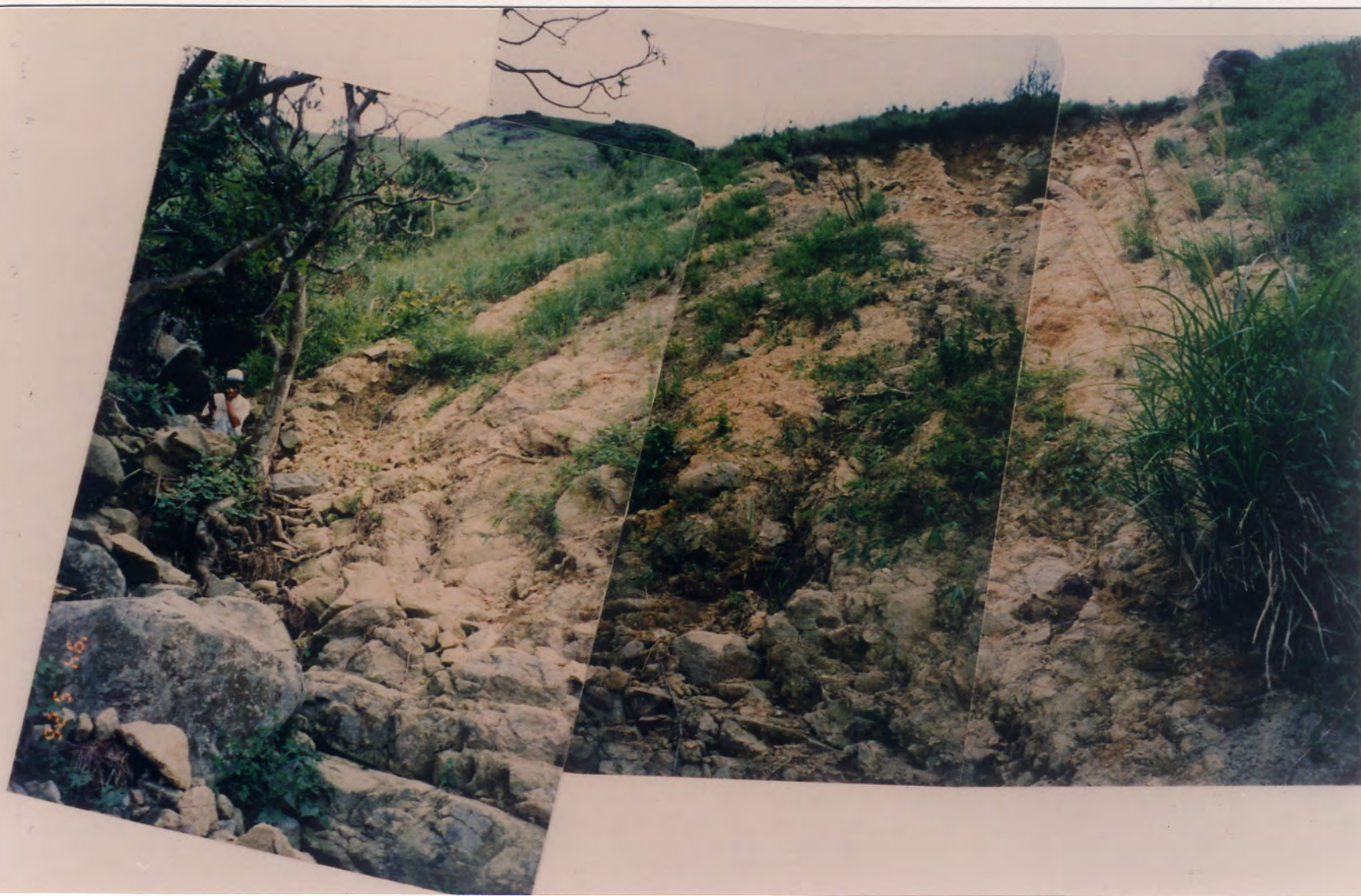
Plate A5.3 - Uphill View of Debris Trail toward Main Scarp A5A
