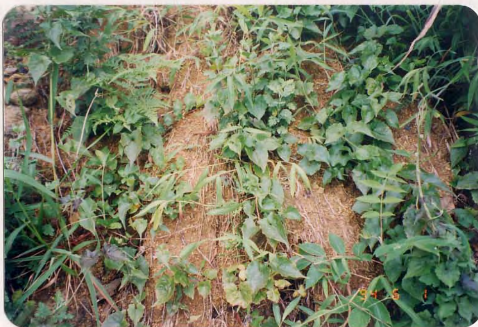
Plate A13.6 - Signs of Surface Water Action along Debris Trail of Landslide A13A
