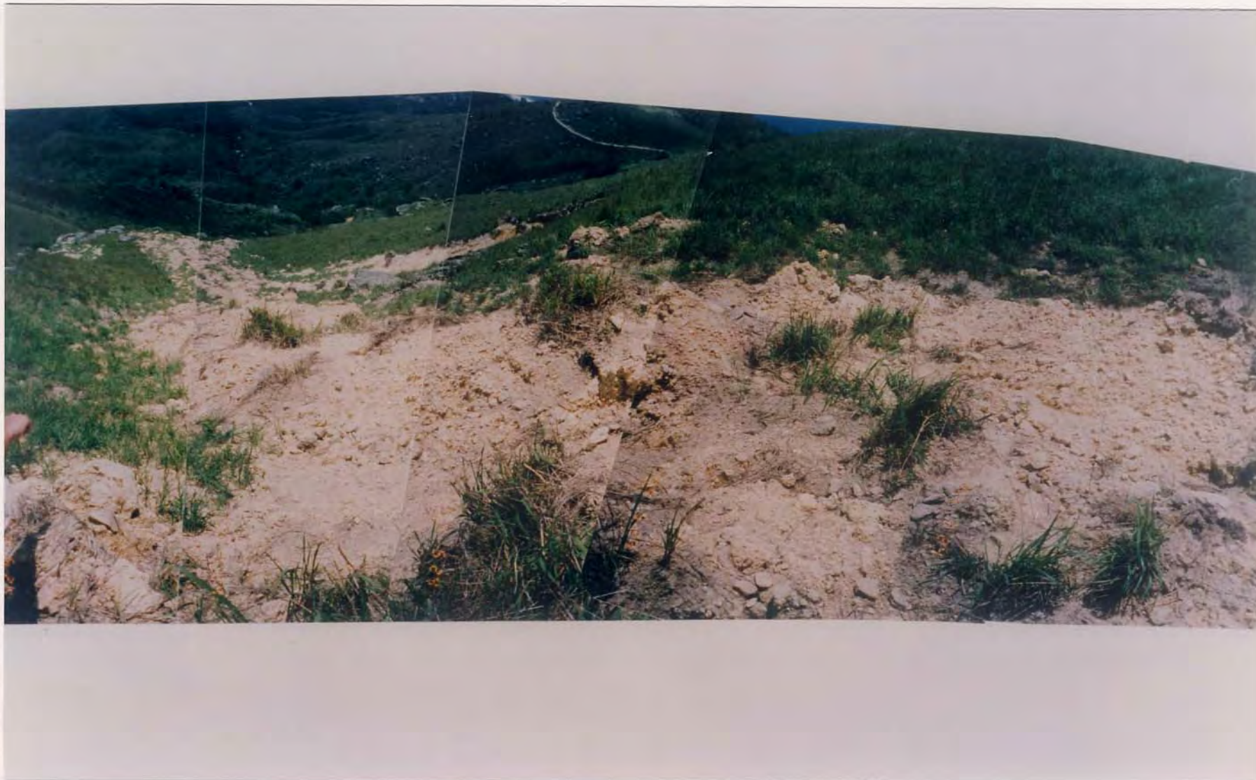
Plate A18.11 - Downhill View of Debris Trail from Landslide A18B
