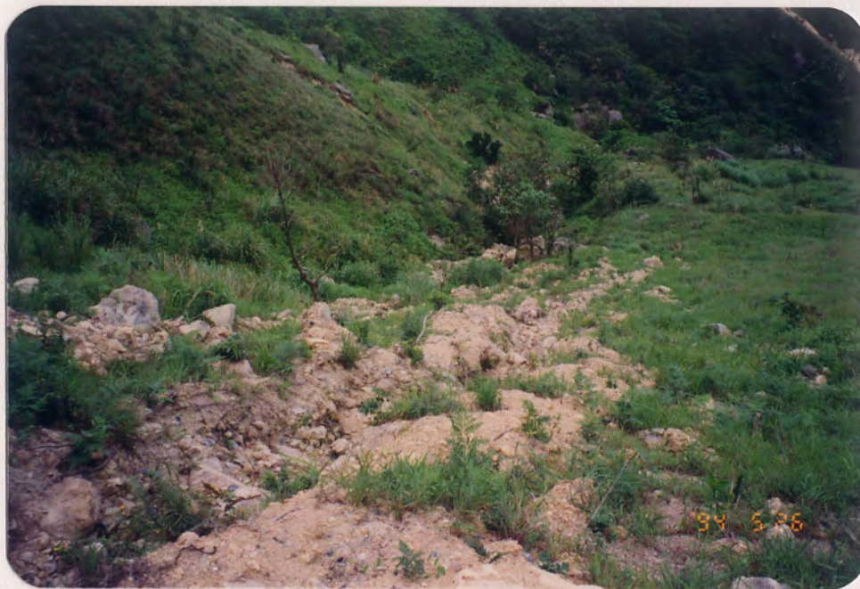
Plate A5.9 - Downhill View of Debris Trail from Main Scarp A5B
