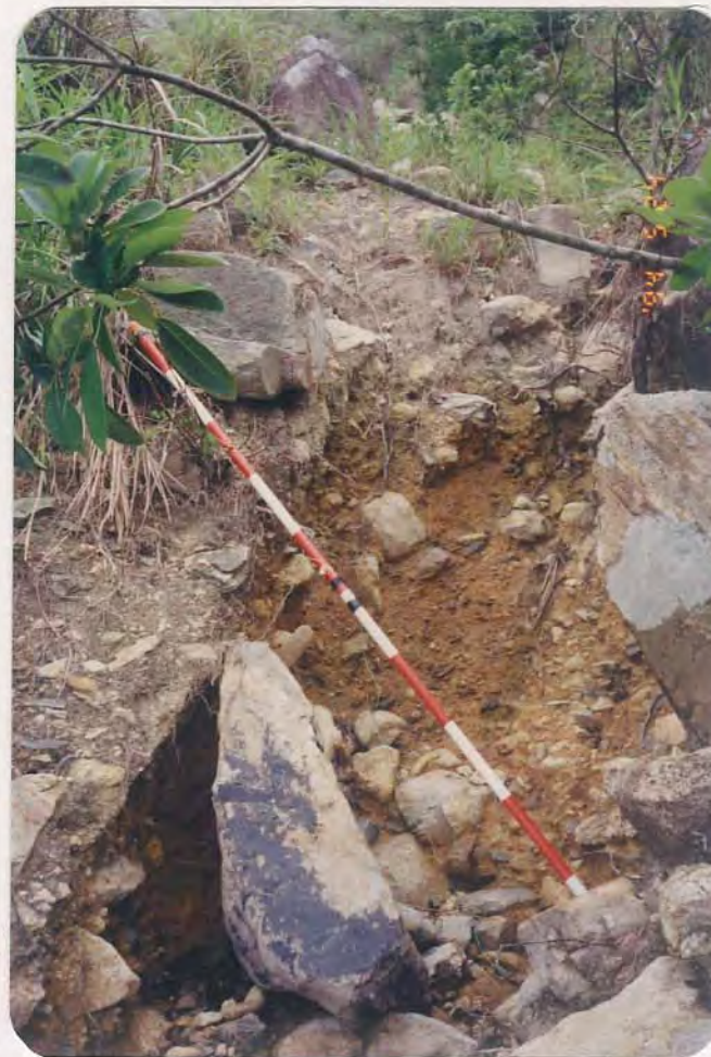
Plate A18.9 - Signs of Surface Water Action along Debris Trail of Landslides A18B & A18C
