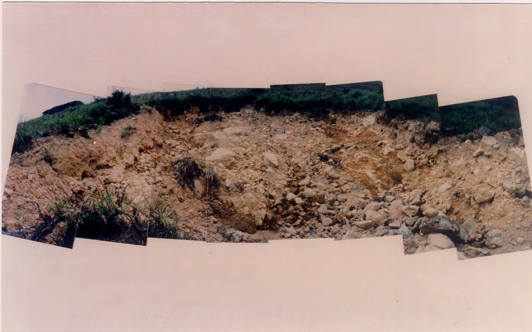
Plate A5.13 - Close-up of Main Scarp of Landslide A5B
