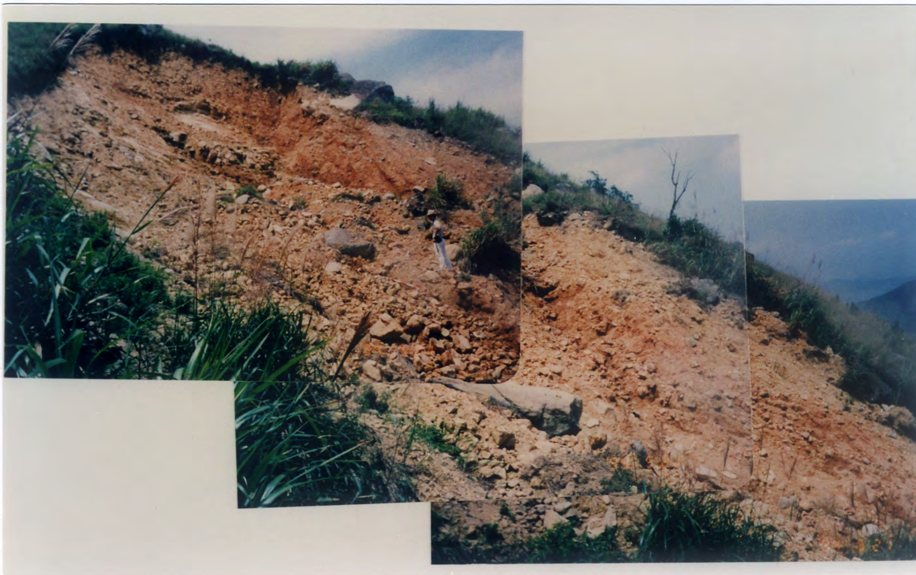
Plate A1.17 - View of Landslide Scarp A1B
