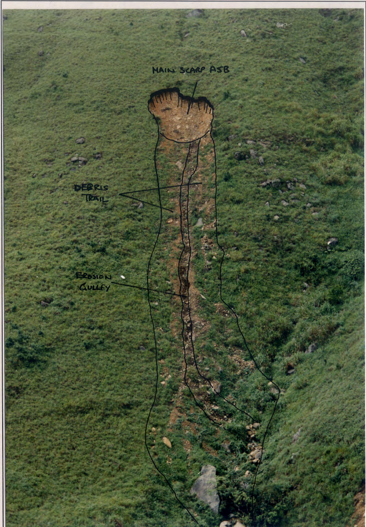
Plate A5.12 - Oblique View of Landslide A5B
