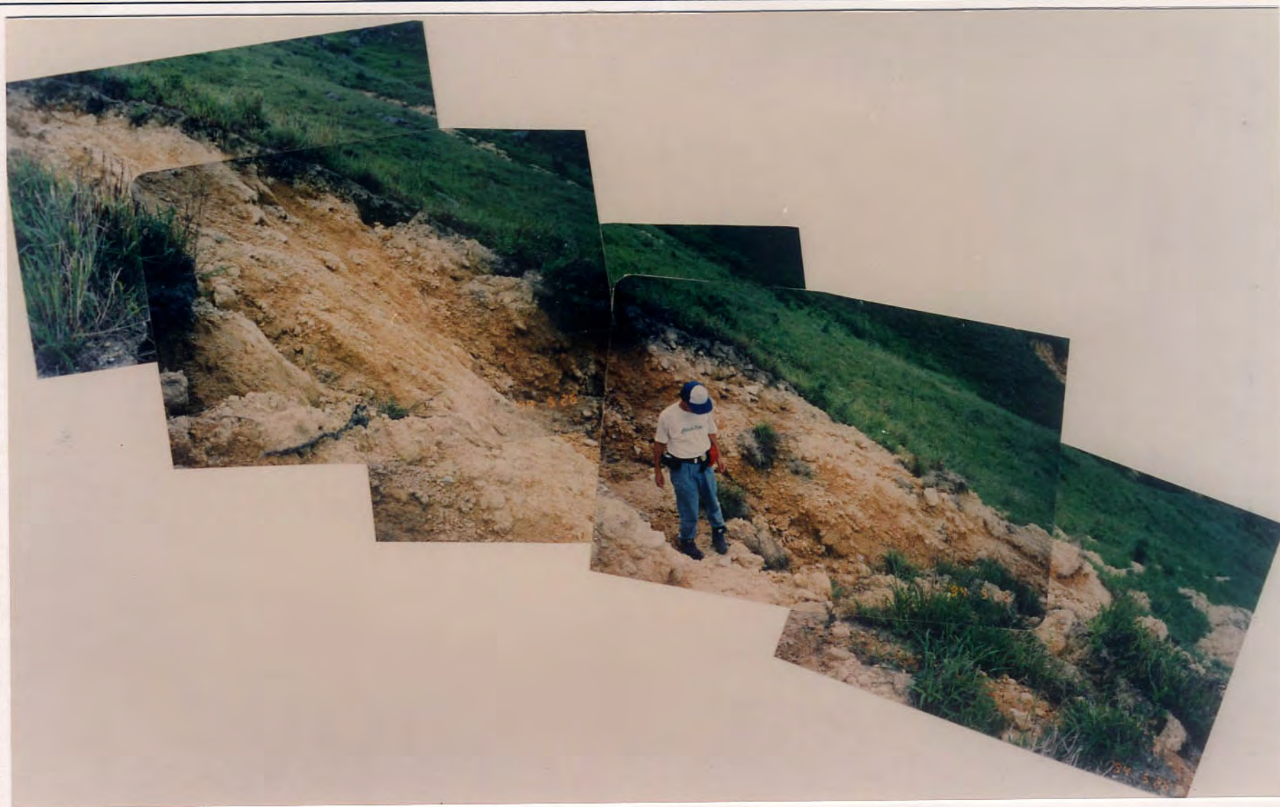
Plate A6.5 - Eastern Side of Landslide Scarp A6
