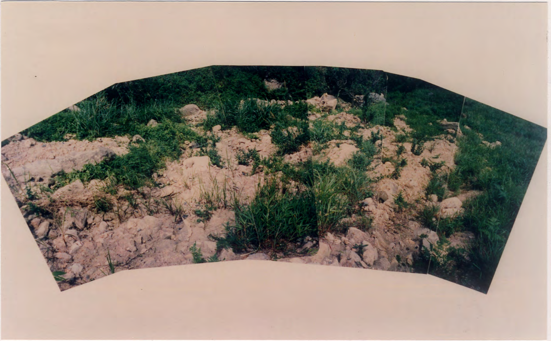
Plate A5.11 - Debris Deposited along Trail of Landslide A5B
