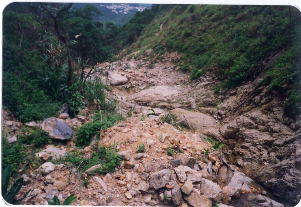
Plate A1.10 - Downhill View of Debris Trail of Landslide A1B
