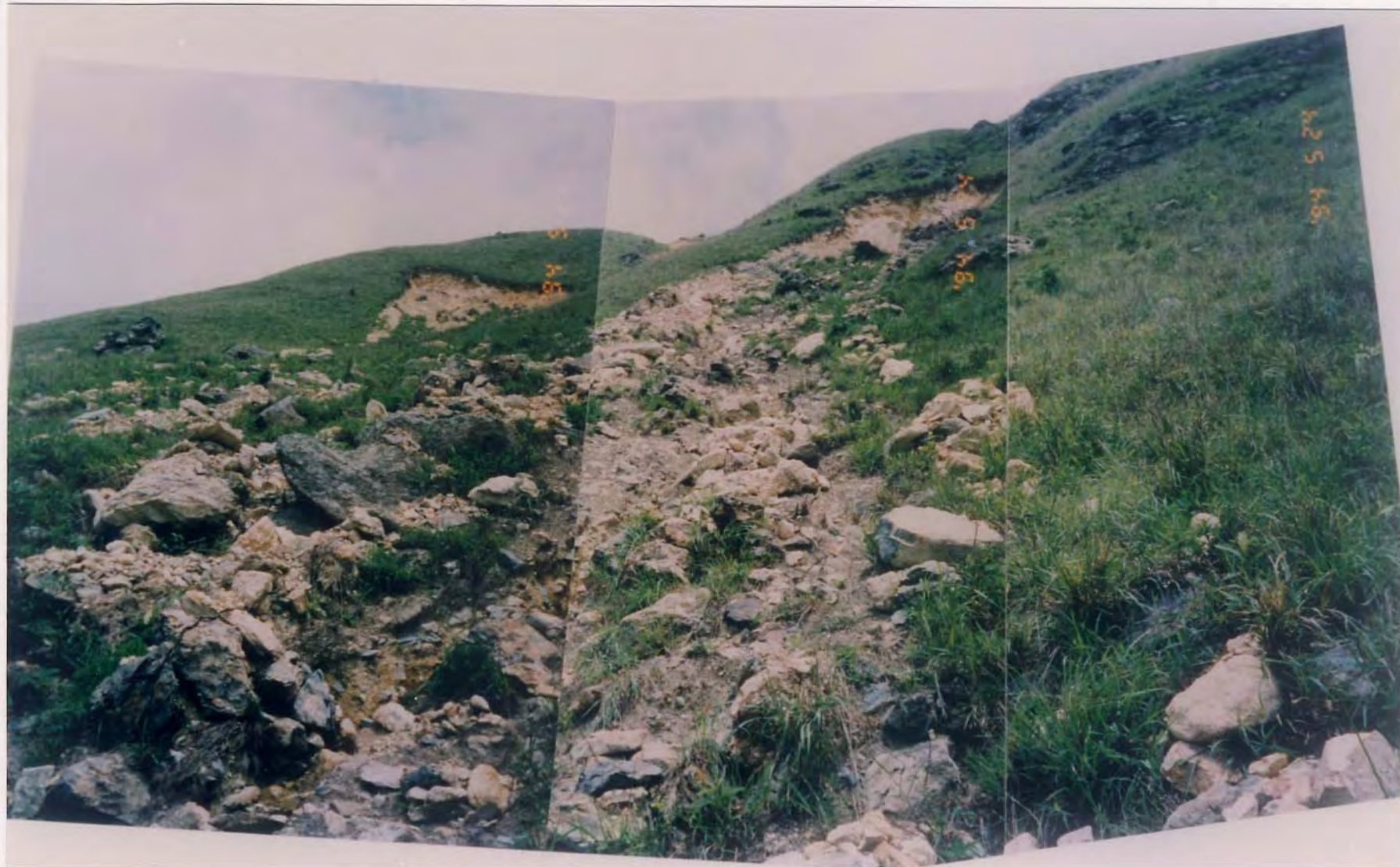
Plate A18.3 - Uphill View of Debris Trail of Landslide A18A
