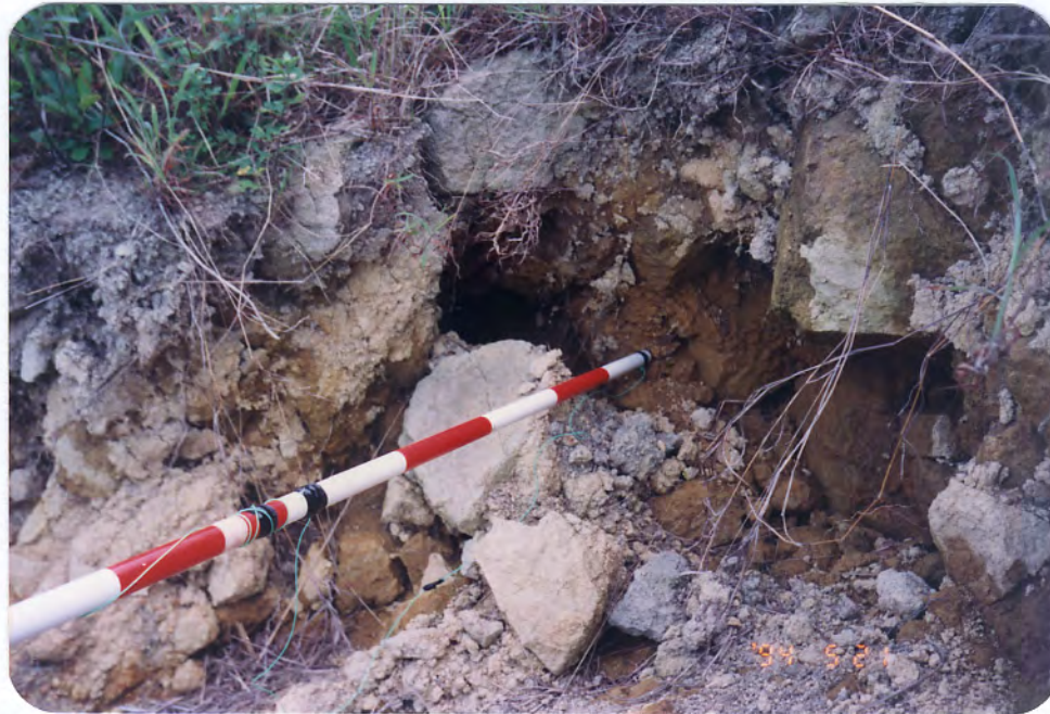
Plate A1.6 - Pipe Holes at Crown of Landslide A1A
