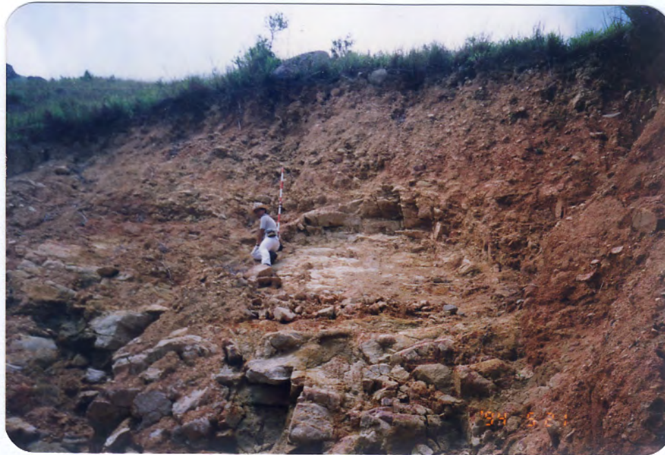
Plate A1.19 - Close-up of Landslide Scarp A1B
