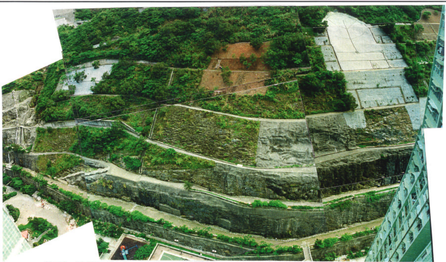
Plate 5 - High-level Oblique View to the West, of Slope 11SE-D/C188 on the West Side of Siu Sai Wan Estate, Showing the PW0/30 and PW90/100 Rock Mass Weathering Zone Interface, and Associated with Seepage and Kaolinitic Clay Development (Taken 2/7/96)
