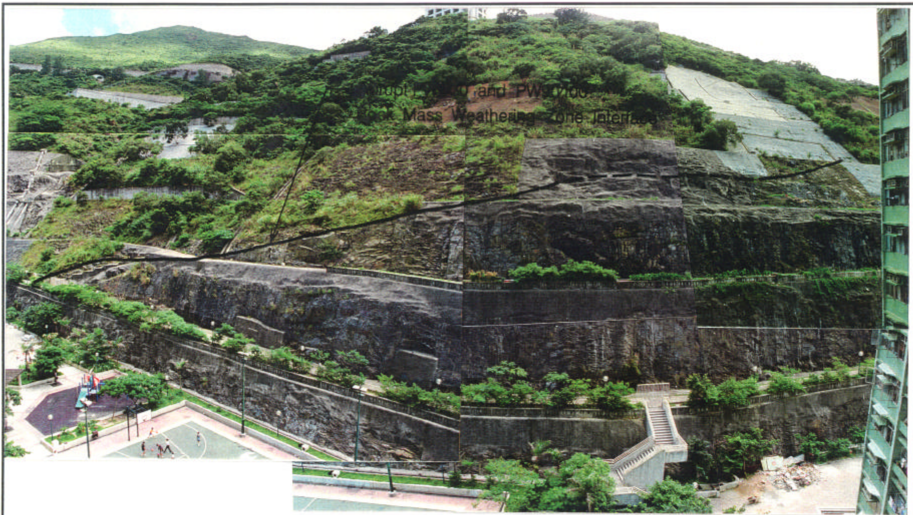
Plate 4 - Low-level Oblique View to the West, of Slope 11SE-D/C188, on the West Side of Siu Sai Wan Estate, Showing the PW0/30 and PW90/100 Rock Mass Weathering Zone Interface, and Associated with Seepage and Kaolinitic Clay Development (Taken 2/7/96)
