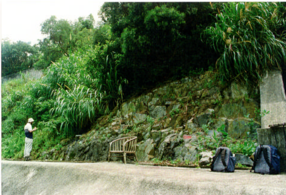
Plate 3 - General View of Planar, Obliquely Outward-dipping PW0/30 and PW90/100 Rock Mass Weathering Zone Interface (84356 81362), Associated with Kaolinitic Clay Development, in Slope 11SE-D/C188, West of Siu Sai Wan Estate (Taken 17/7/96)
