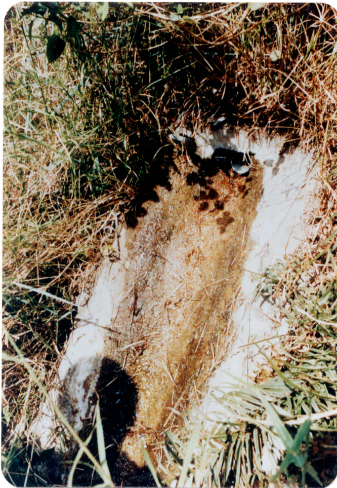
Plate 14 - Drain Outlet Showing Seepage Stains, New Clear Water Bay Road
