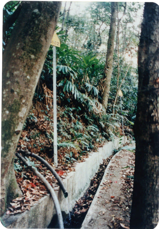
Plate 6 - Typical Drain Outlet in Natural Slope at Po Shan
