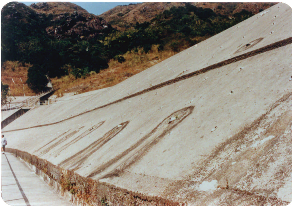
Plate 28 - Flow Scour on Chunam Surface Below Drain Outlets at Tsz Wan Shan Estate
