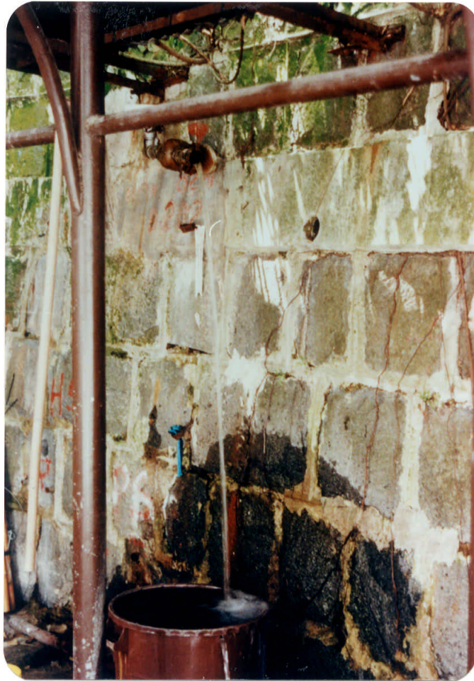
Plate 7 - Typical Drain Outlet Through Retaining Wall at Po Shan
