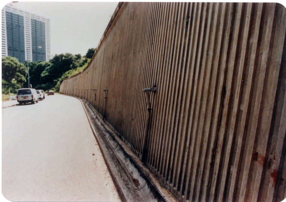
Plate 20 - Drain Outlets Through Retaining Wall, Tin Wan Hill Road
