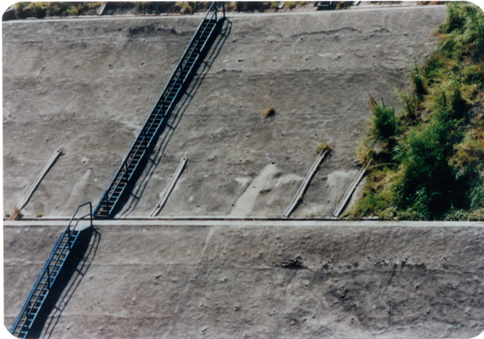
Plate 21 - Drain Outlets in Centre of Slope, Tin Wan Hill Road
