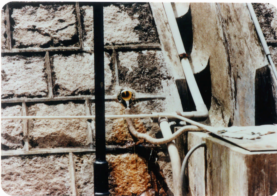
Plate 11 - Flowing Drain at Base of Slope Behind Grenville House
