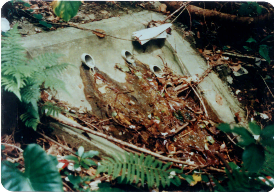
Plate 24 - Close-up View of Group of Drain Outlets, Hing Man Estate
