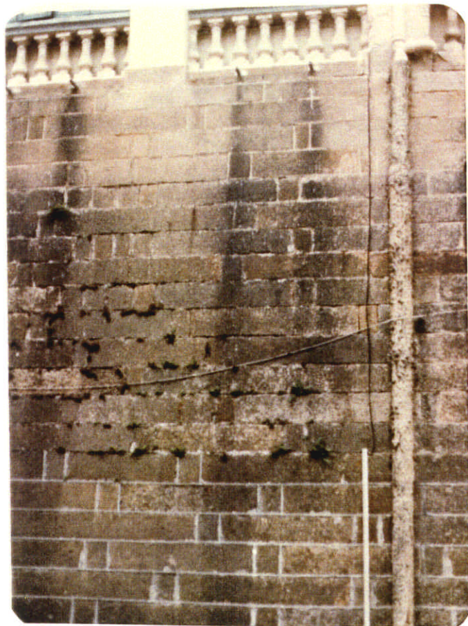
Plate 3.3 - Tied Face Retaining Wall at Caine Road J/o Castle Road
