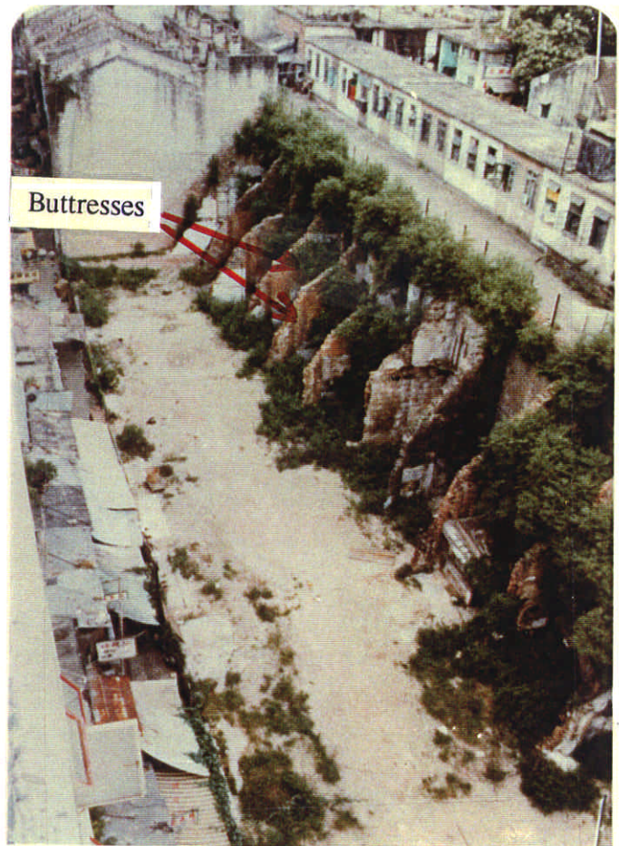
Plate D8.2 - Retaining Wall at Fat Hing Street - View of the Wall before Work Commenced on the Adjacent Site (II)
