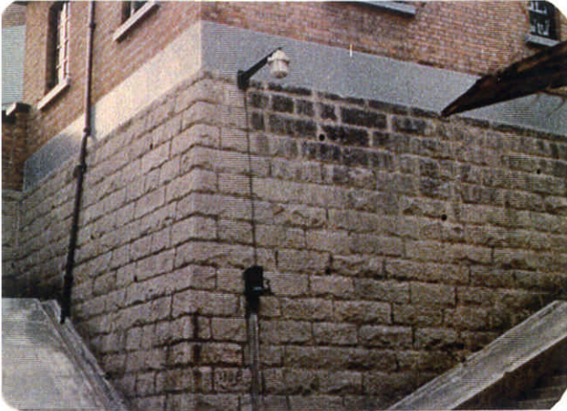
Plate B7 - Dressed Block Wall (11SW-A/R46)
