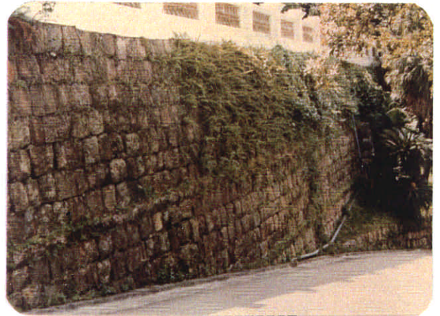
Plate B4 - Dry Packed Squared Rubble Wall with Horizontal Beams (11SW-A/R163)
