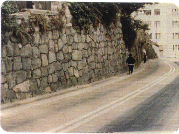
Plate B1 - Dry Packed Random Rubble Wall (11SW-A/R389)
