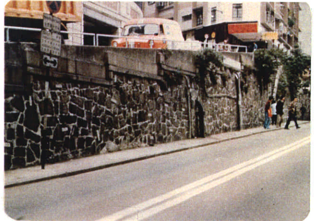
Plate B2 - Pointed Random Rubble Wall (11SW-A/R116)
