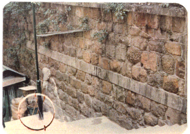
Plate B6 - Pointed Squared Rubble Wall with Horizontal Beams (11SW-A/R194)
