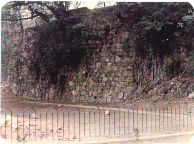
Plate B3 - Dry Packed Squared Rubble Wall (11SW-A/R109)
