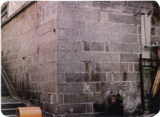
Plate B9 - Tied Face Wall (11SW-A/R74)
