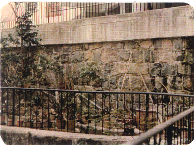
Plate B5 - Pointed Squared Rubble Wall (11SW-A/R295)
