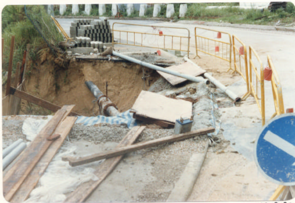
Plate 1 : Deep Water Bay Road : Minor failure of a (Incident No. HK/8/28) fill slope
