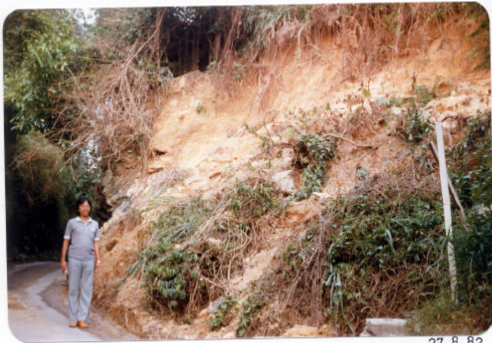
Plate 31 : Cheung Hang Road (A) : Road totally blocked (Incident No. NT/8/11) by debris
