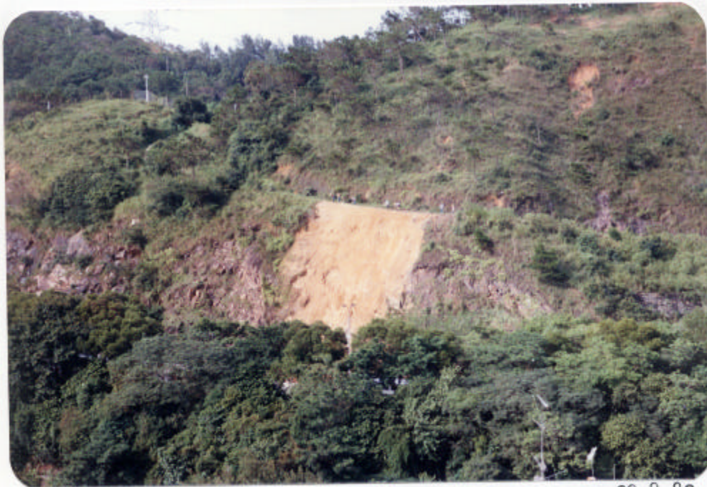
Plate 6 : 5 \frac{1}{2} MS Castle Peak Road : Major failure of a soil/rock (Incident No. NT/8/23) cut slope (11NW-A/C63)
