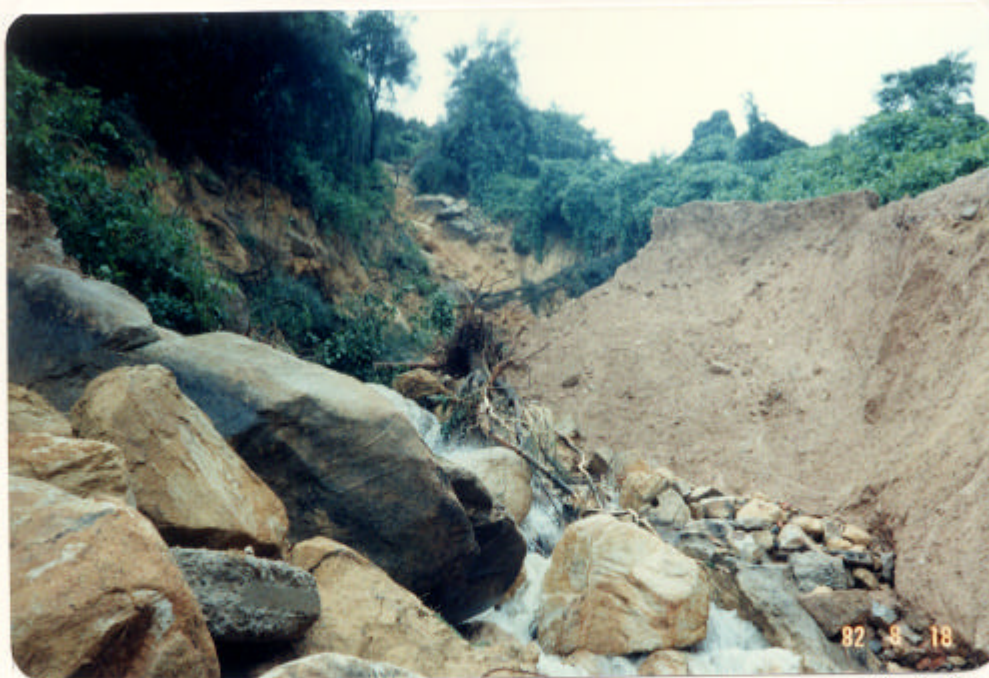
Plate 2 : Mount Butler Quarry : Major failure of a (Incident No. HK/8/23) fill slope
