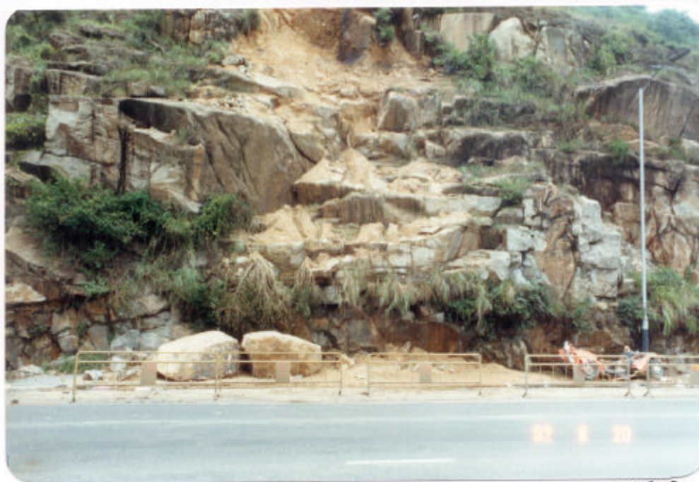
Plate 10 : Kwai Chung Road : Major failure of a rock (Incident No. NT/8/26) cut slope (11NW-A/C79)
