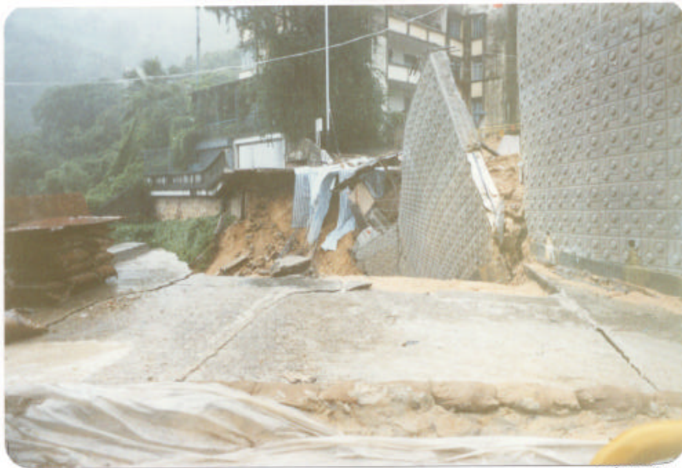
Plate 13 and 14 : 7, Chung Shan Terrace, NT : Major failure of (Incident No. GCB 6/8) a retaining wall
