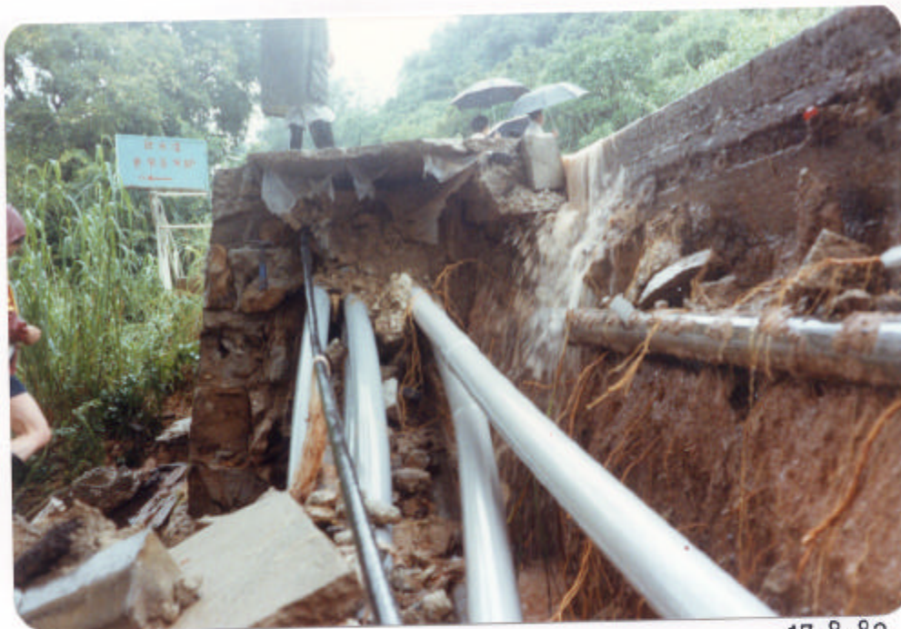
Plates 16 and 17 : 9½ MS Castle Peak Road : Major failure of a (Incident No. NT/8/16) retaining wall
