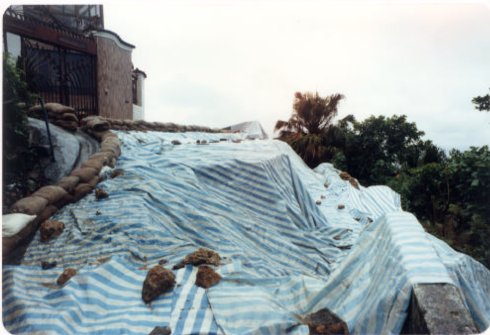
Plate 15 : 25, Lugard Road, HK : Major failure of (Incident No. GCB 1/8) a retaining wall
