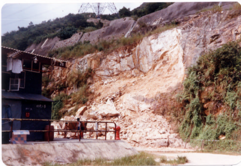
Plate 9 : Shek Yam Temporary Housing Area : Major failure of a (Incident No. NT/8/69) rock cut slope (7SW-C/C153)
