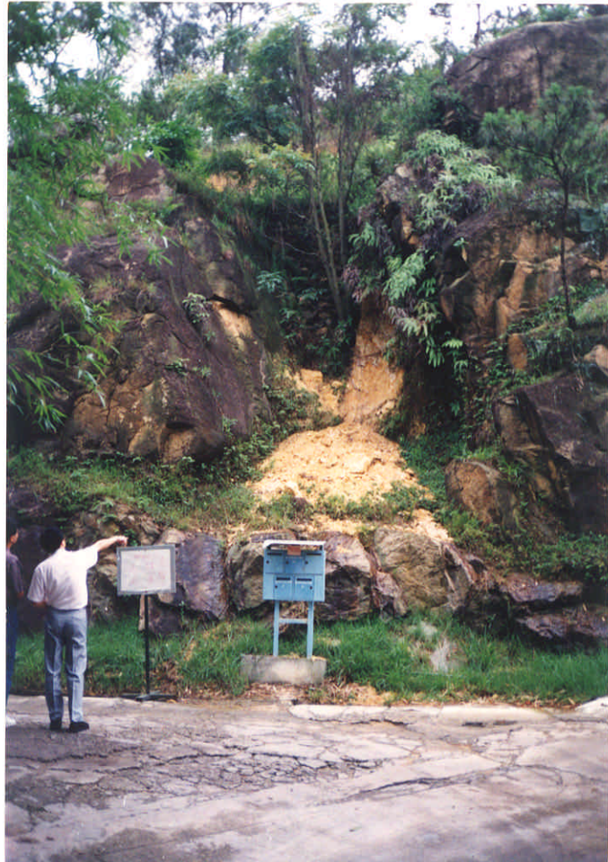
Description : Failure of a rock cut slope affecting a private access.
