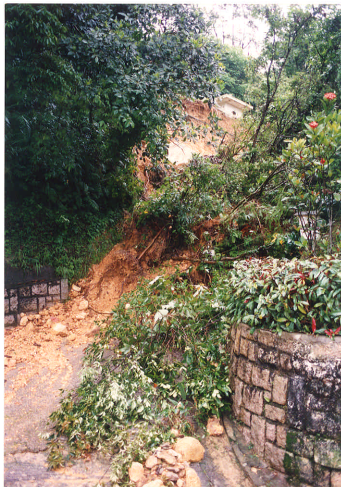
Plate 18 - 9 Middle Gap Road, Wan Chai Gap (Incident HK 5/39)
