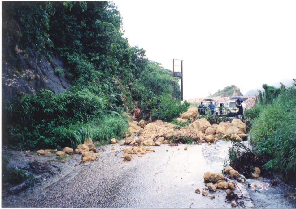
Negative No. ME9218819 Taken on : 8-5-92 Description : Failure of a soil cut slope resulting in the blockage of one road lane.
