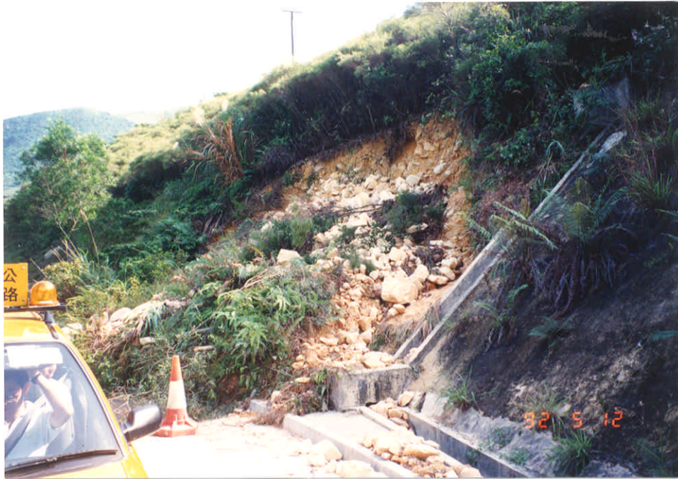
Negative No. MW9211524 Taken on : 12-5-92 Description : Failure of a soil cut slope resulting in the partial blockage of a road.
