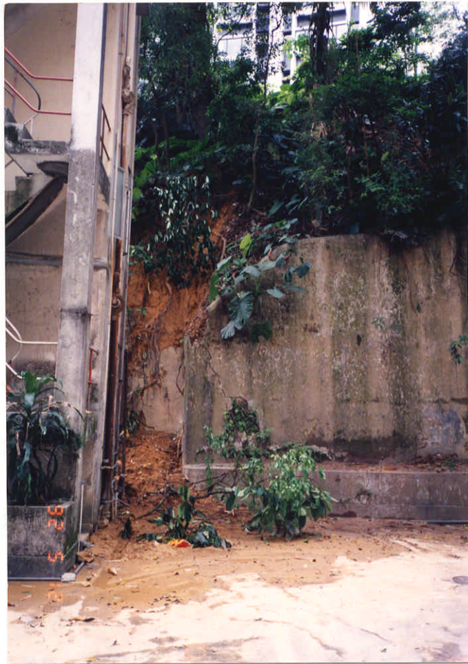
Description : Failure of a soil cut slope affecting a building lot.
