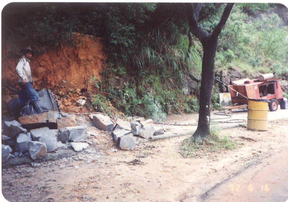
Negative No. I9235707 Taken on : 16-6-92 Description : Rock/boulder fall affecting a footpath.
