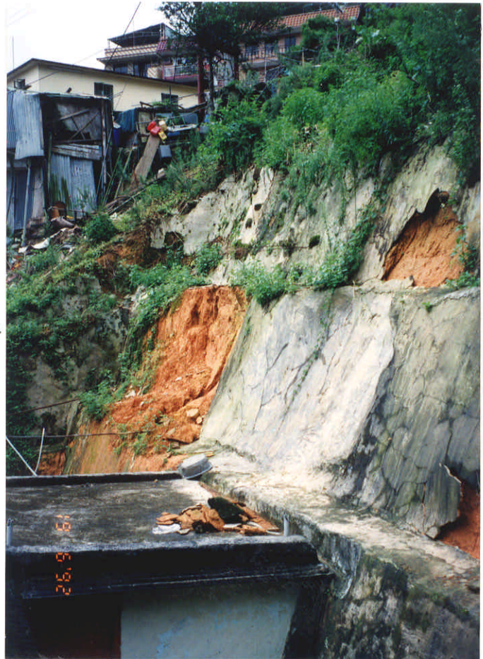
Description : Failure of a soil cut slope affecting a building lot.
