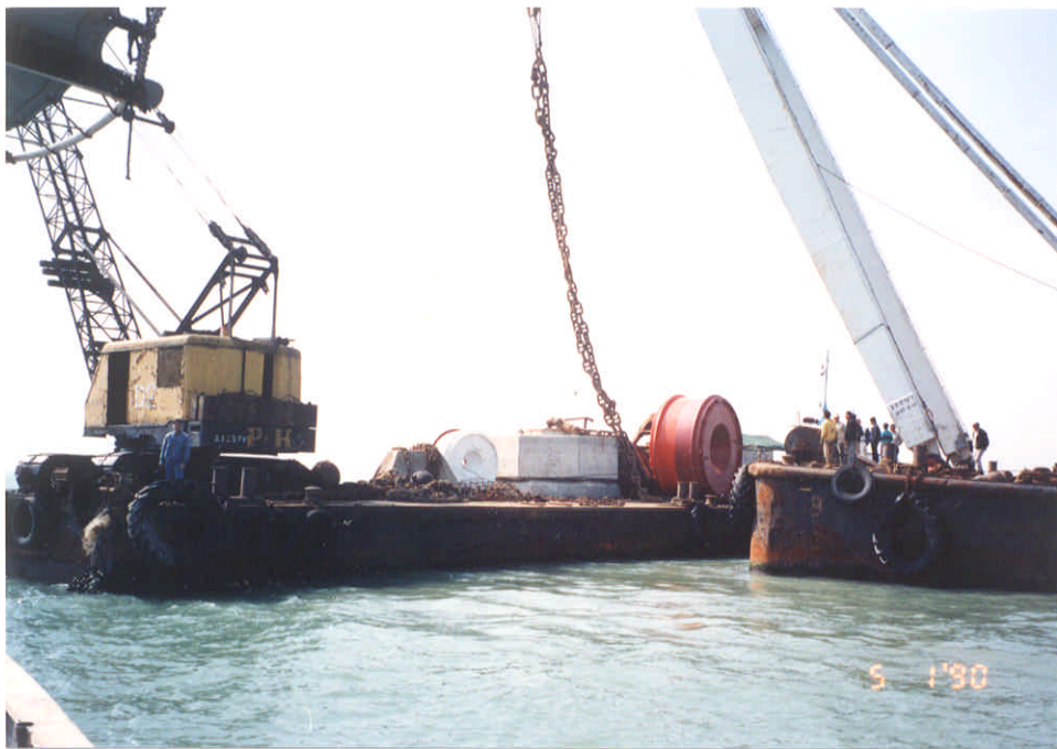
Plate 8 - 90-tonne Sinker and Harbour Mooring Buoy before Deployment at Urmston Road Borrow Area
