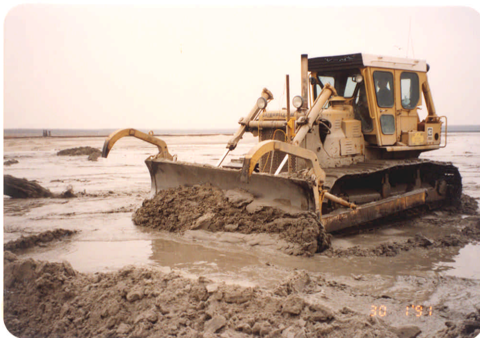
Plate 16 - Levelling Operations at Reclamation Site
