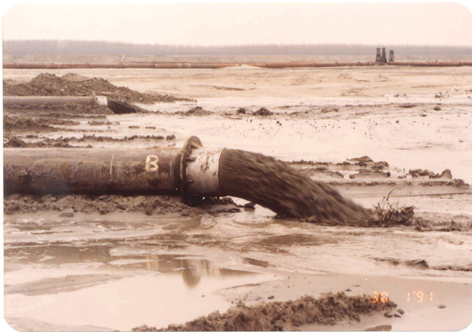
Plate 15 - Quick Coupling Discharge Pipes in use at Reclamation Site
