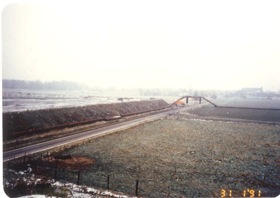
Plate 13 - Pipeline Transport of Dredged Sand over Low-Lying Land
