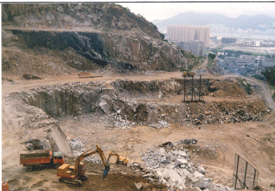
Plate 1 - General View of the Former Quarry Area Looking Southeast and Showing the Basalt Dyke Intrusion
