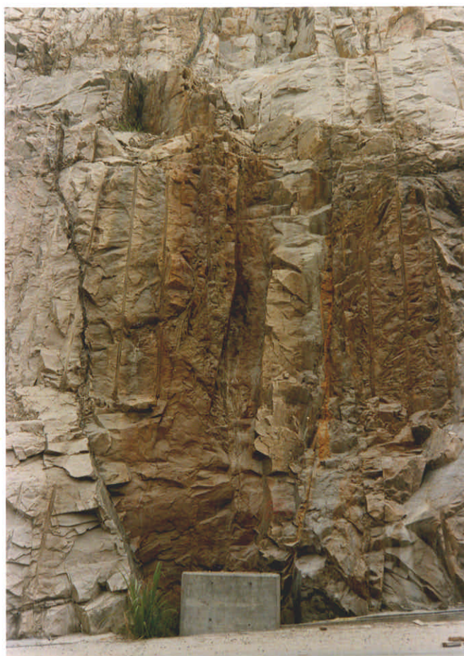
Plate 2 - Jointing Pattern in Fine- to Medium-Grained Granite
