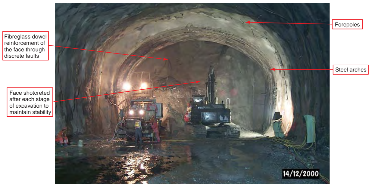
Figure 6.7.11 – Full face excavation, face reinforcement and forepoling during construction (photograph by Nishimatsu-Dragages Joint Venture)
