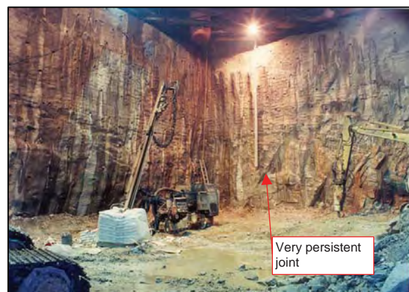
Figure 6.6.3 – MTRC North Point plant building during excavation showing limited support and occasional very persistent joints
