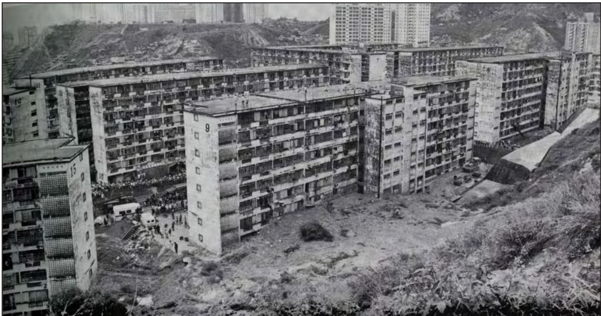
Figure 5.9.2 – View of the fill slope failure at Sau Mau Ping Estate in 1976
