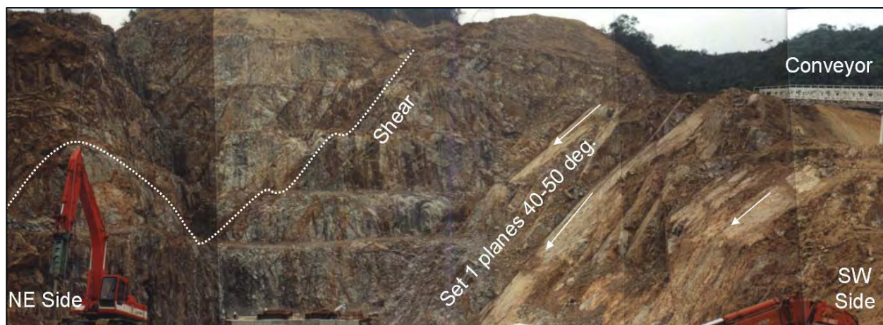
Figure 6.4.32 – Initial ‘box-cut’ of Ting Kau cutting showing continuous shear and persistent Set 1 joint planes (photograph by J.W. Tattersall)
