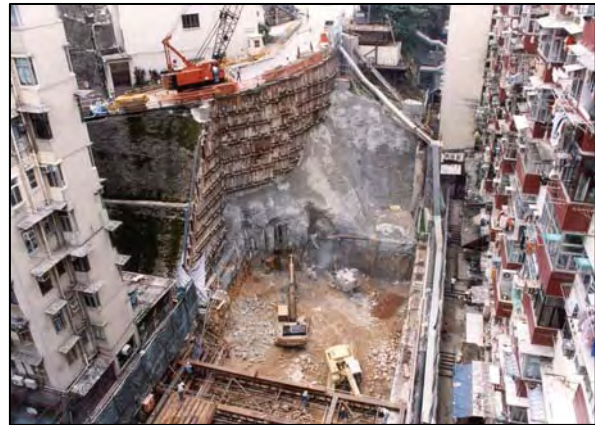
Figure 6.6.2 – Initial excavations for the MTRC North Point plant building
