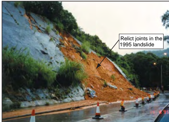
Figure 6.4.13 – 1995 landslide at Sai Sha Road with relict joints (Wong, 1997)
