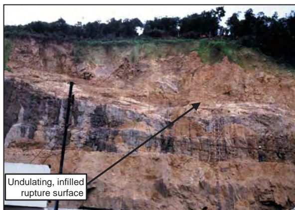
Figure 6.4.19 – 1982 South Bay Close landslide scar (Hencher, 1983b)
