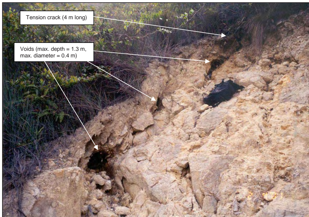
Figure 4.4.13 – Voids/soil pipes at the colluvium/bedrock interface in a landslide scar
