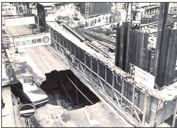
Figure 6.6.1 – Collapse of road due to boulders preventing adequate embedment of sheet piles retaining adjacent excavation
