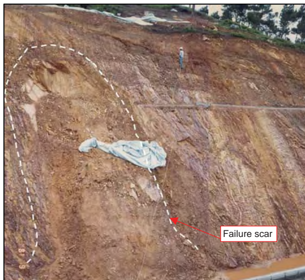
Figure 6.4.29 – 1981 failure on undulating foliation planes plunging steeply towards cutting at Lin Ma Hang Road
