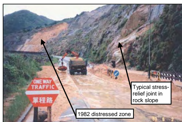
Figure 6.4.18 – Outwash from complete failure of the 1982 distressed zone of the ‘Pepco’ slope blocking Tsing Yi Road in 1983 following heavy rain (Choot, 1993b)
