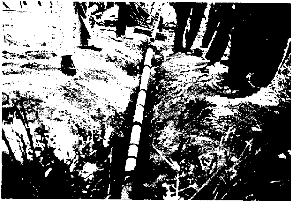
Plate 9 - Horizontal Drain after Exhumation Showing Successfully Grouted Invert (November, 1983)
