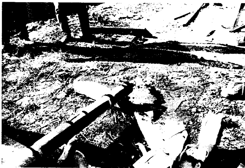
Plate 6 - Water Testing Grouting Nozzle before Drain Installation (November, 1983)
