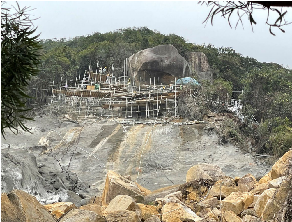
a) Emergency Repair Works at the Crest of the Lower Landslide Scar
