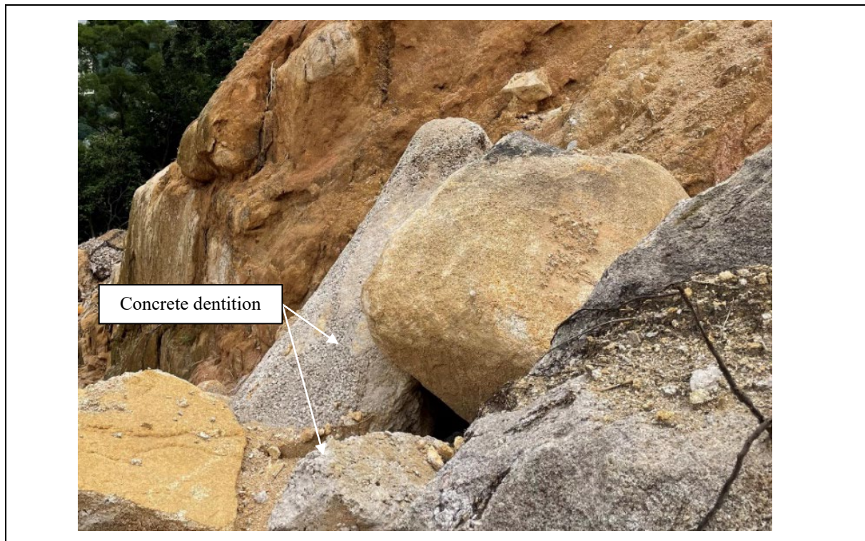
Figure 6.27 Remnants of Concrete Dentition at the Lower Landslide Scar (Photograph taken on 26 September 2023)
