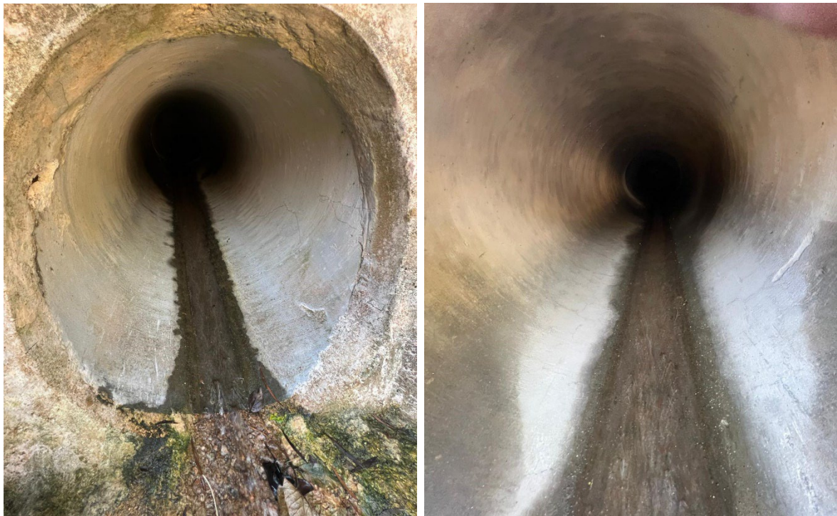
b) Partially Blocked Inlets of the Other Two Drainage Outlet Pipes
