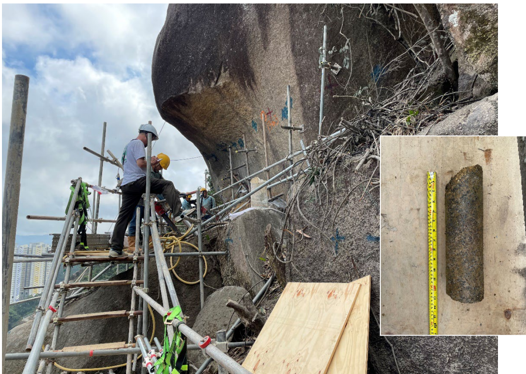
b) Drillholes for Installation of Dowel Bars at Tor and Coreslab
