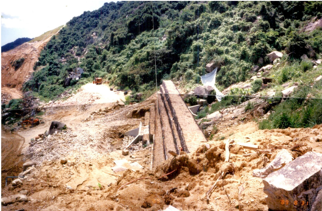
a) Overview of Gabion Wall ND9 Across the Rocky Stream Course
