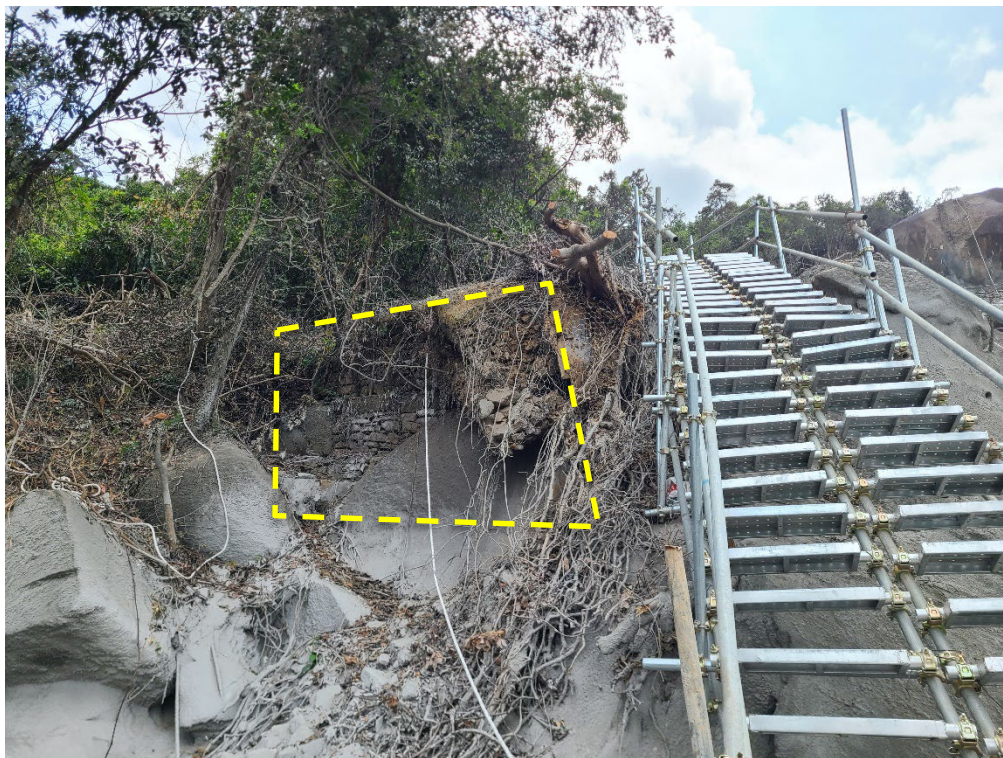
b) Remnant of Gabion Wall ND10
