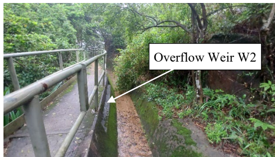
(c) Overflow Weir W2 (Photograph taken on 2 May 2024)
