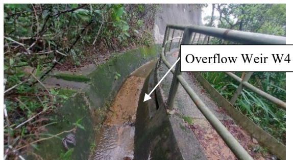
(e) Overflow Weir W4 (Photograph taken on 2 May 2024)
