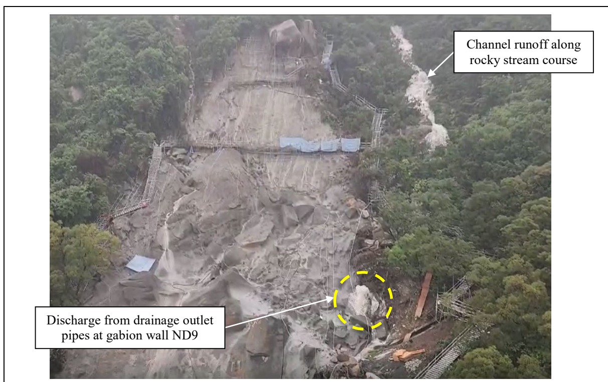
Figure 6.10 Channel Runoff along Cascade below Gabion Wall ND9 (Photograph taken on 4 May 2024)
