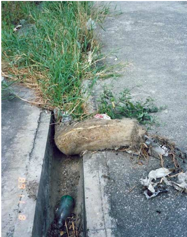
(a) U-channel along Crest of Slope
