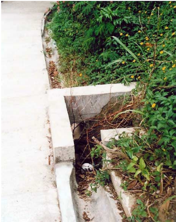
(c) Catchpit at Toe of Slope
