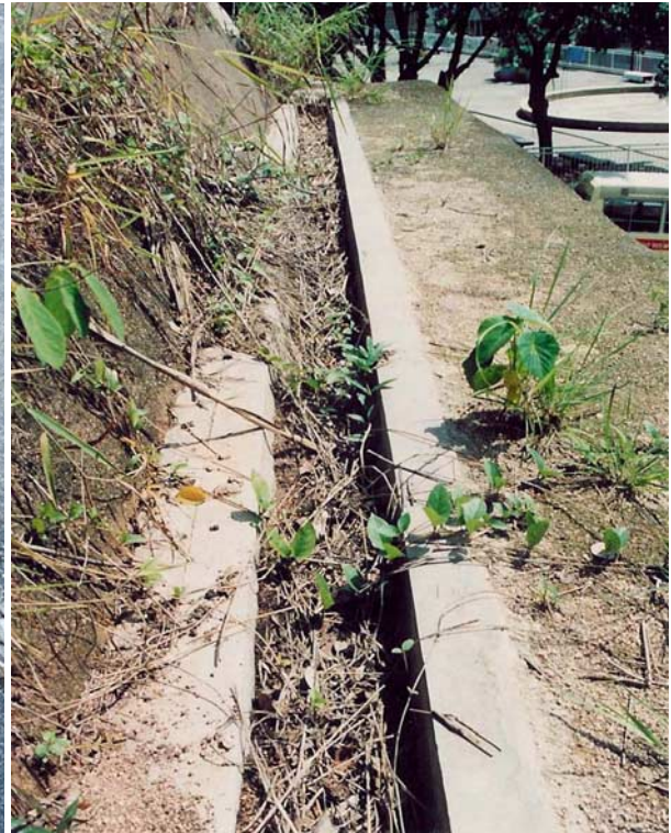
(b) U-channel along Berm of Slope
