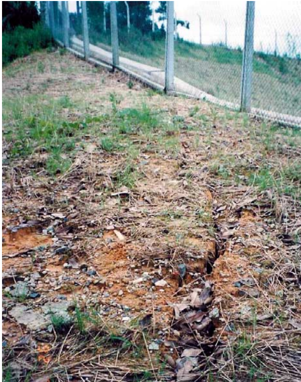
(a) Tension Crack on Slope
