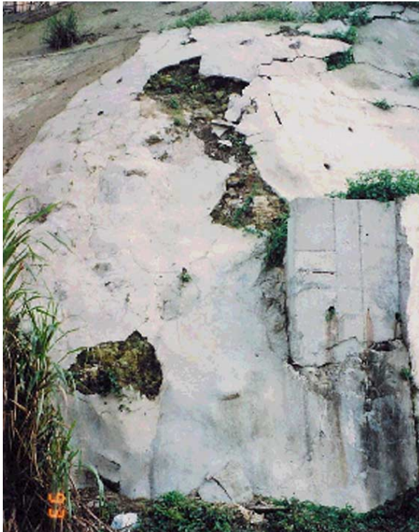
(c) Cracked Chunam Surface
