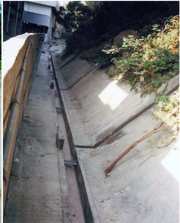
(b) U-channel along Toe of Slope
