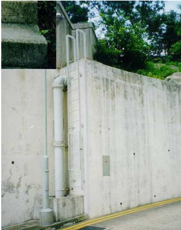
(a) Exposed Down Pipe on Retaining Wall
