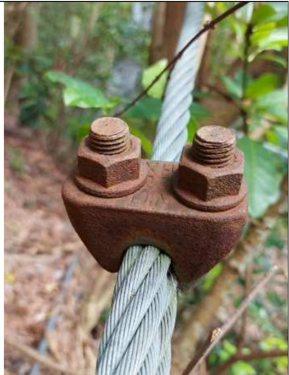
(b) Wire Rope Clips
