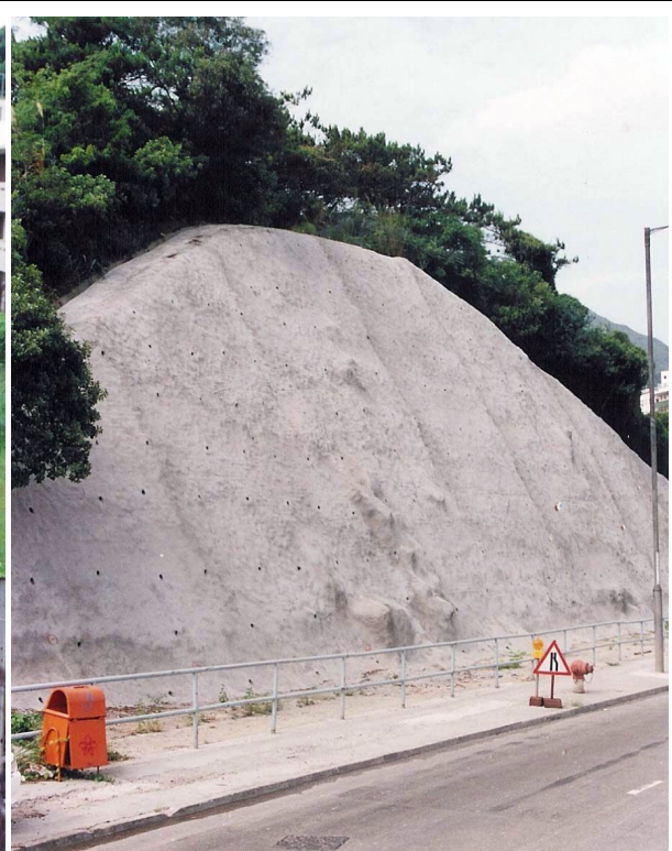
(b) Shotcreted Surface
