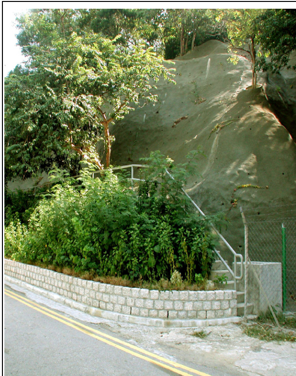
(a) Concealed Access to Stairway
