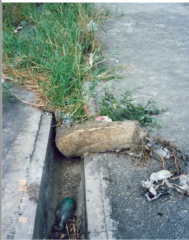
(a) U-channel along Crest of Slope
