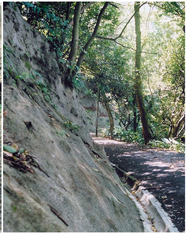
(b) Shotcreted Surface
