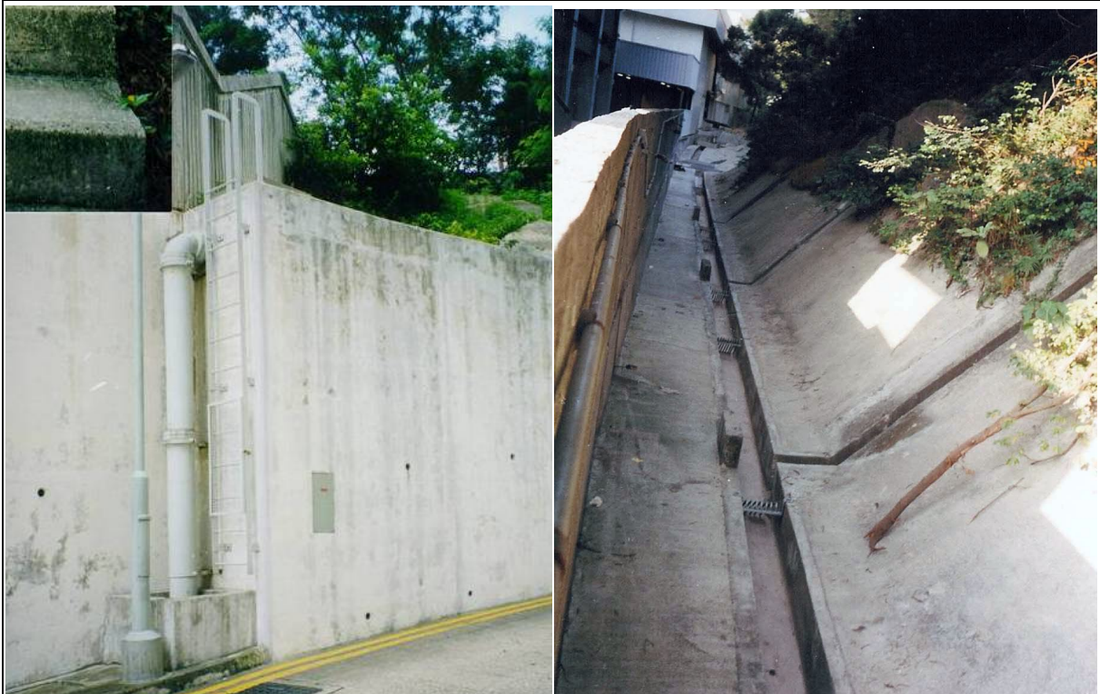
(a) Exposed Down Pipe on Retaining Wall
