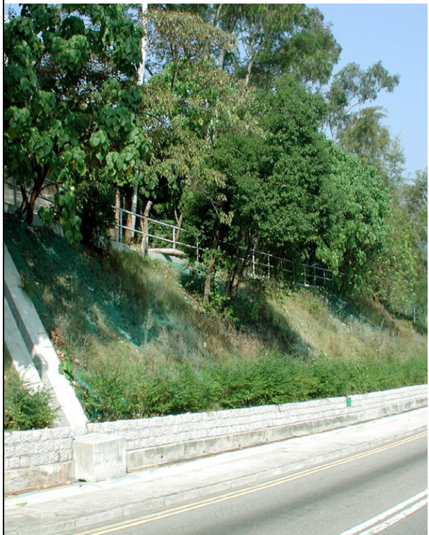
(c) Fencing Recessed into Vegetated Land
