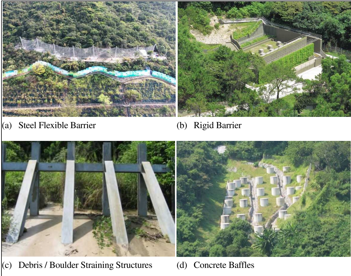
Plate 6.1 Examples of Natural Terrain Hazard Mitigation Measures
