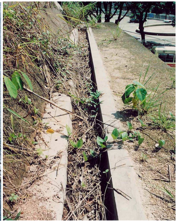
(b) U-channel along Berm of Slope
