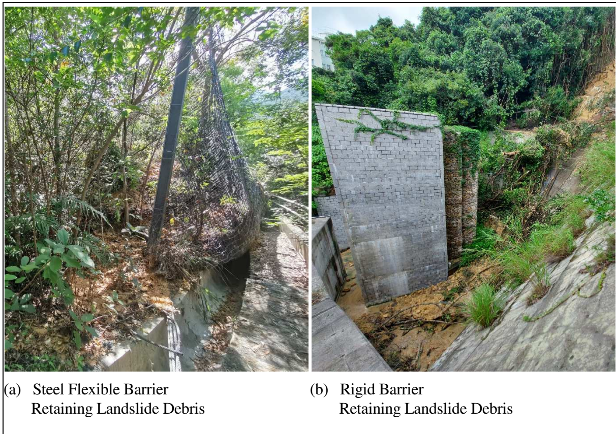
Plate 7.1 Examples of Landslide Debris Accumulated behind Defence Measures
