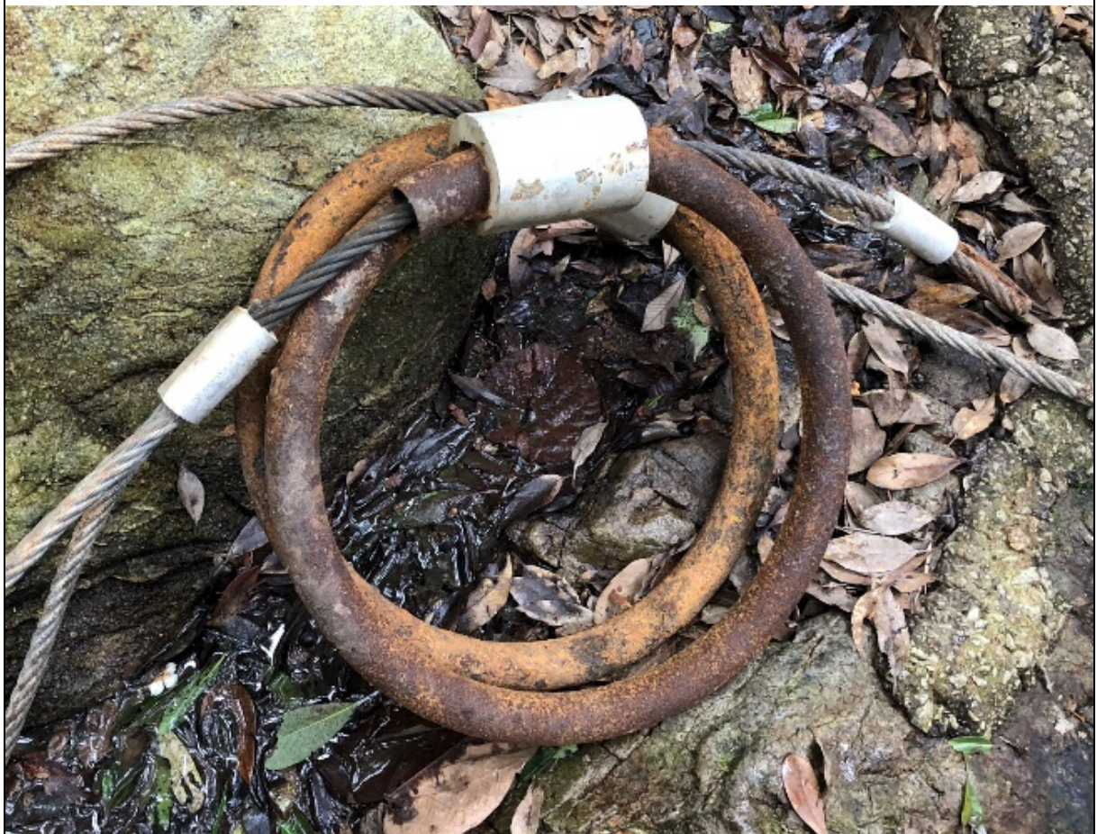
(c) Energy Dissipating Devices
