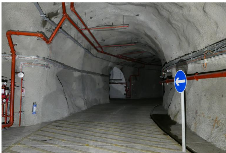
Figure A3 One of the Explosive Storage Niches (Left), and a Section of the Horseshoe-shaped Access Adit at the West Island Line Explosives Magazine (Right) (courtesy of ARUP)
