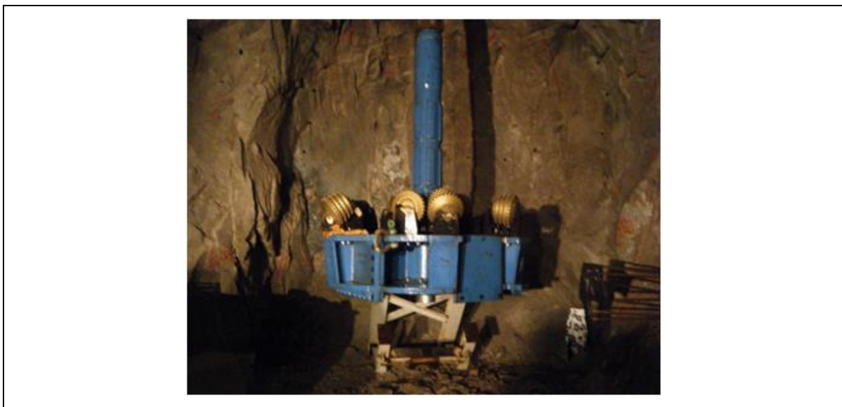
Figure 8.2 Installation of Raise Bore Cutter-head Underground (courtesy of ARUP)
