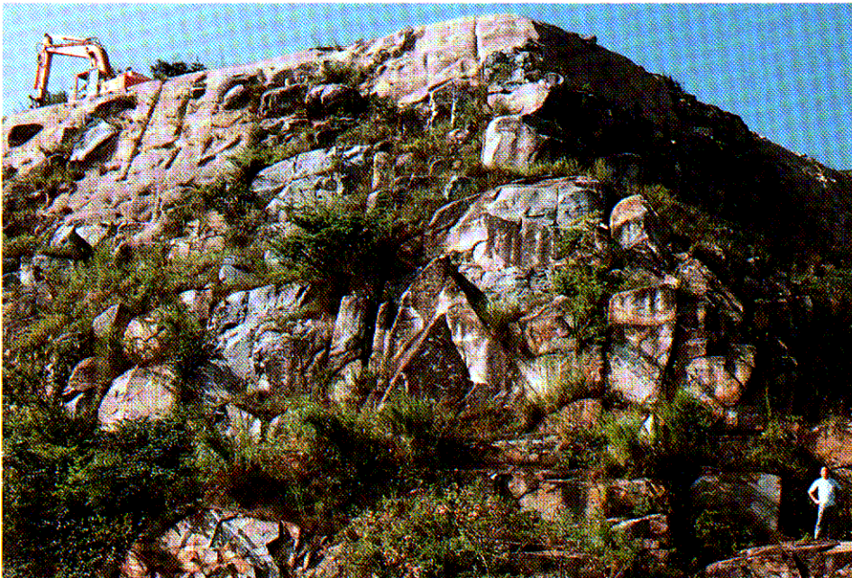
B: Cutslope in Coarse Ash Tuff at Mt. Davis, Hong Kong Island, Showing Variation in Degree of Rock Mass Weathering and Spacing / Orientation of Major Discontinuities ( Vegetation and chunam surfacing obscure the relatively more weathered zones )
