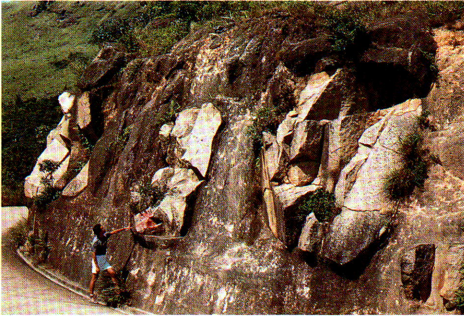
A: Granite Cutslope at Jat's Incline, East Kowloon, Showing a Partially Weathered PW 30/50 Rock Mass Zone with Large Corestones Overlying a Partially Weathered PW 0/30 Rock Mass Zone
